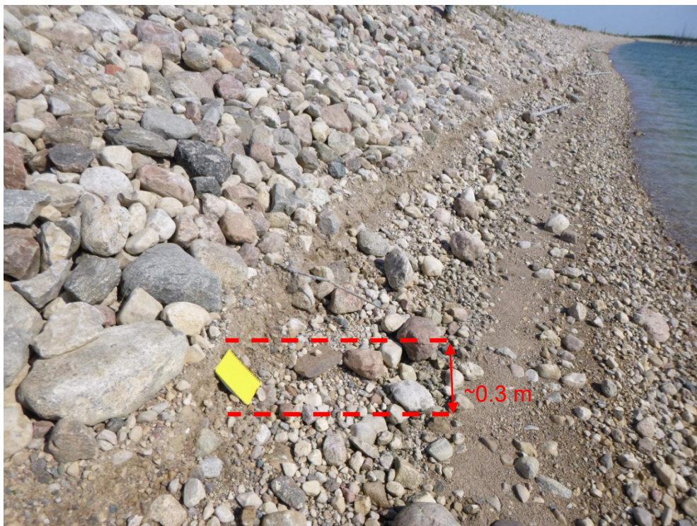
Photograph 12: North Dyke – Upstream Slope, ~0.3 m Scarp Below Riprap Placed In 2018, Looking Northeast, 12 August 2019
