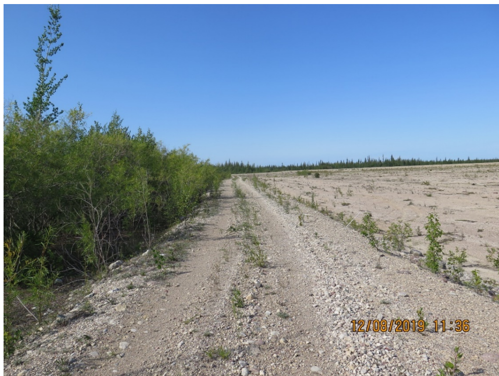
Photograph 3: South Dyke – Crest at West End with Vegetation on Downstream Slope, Looking West, 12 August 2019
