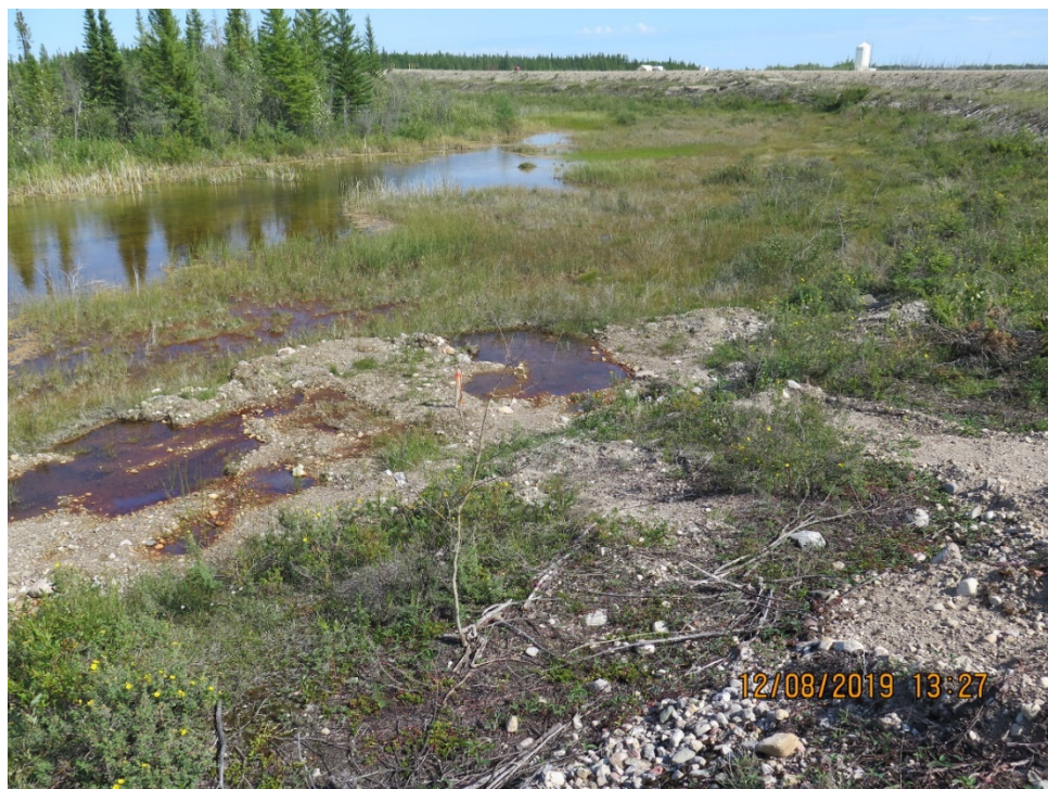
Photograph 14: North Dyke – Downstream Toe Area at Dogleg, Red Staining, Looking East, 12 August 2019
