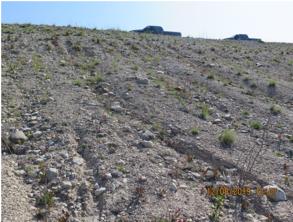
Photograph 7: West Dyke – Downstream Toe and Slope Near North End, Looking East, Minor Erosion Rills, 12 August 2019
