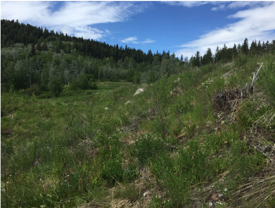
Photo II-18 Tailings Dam – west leg, looking north along dam slope towards Closure Spillway.
