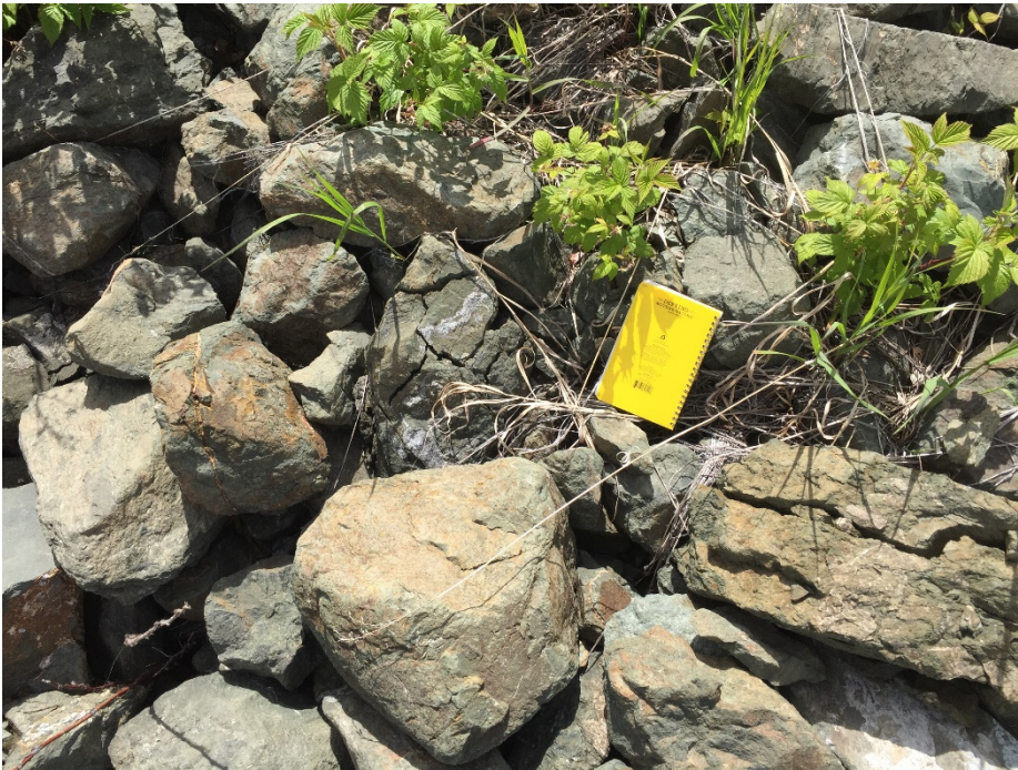
Photo II-44 Ed Creek Diversion Channel – Riprap on right bank, showing weathering and breakage.
