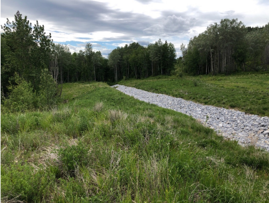
Photo II-23 Closure Spillway – looking downstream from dam crest.
