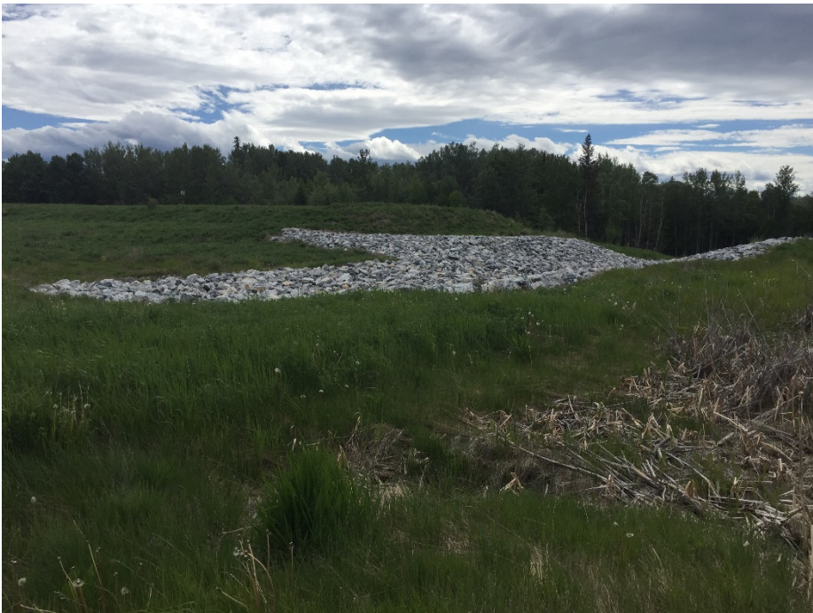
Photo II-24 Closure Spillway – looking southwest from upstream of dam crest.
