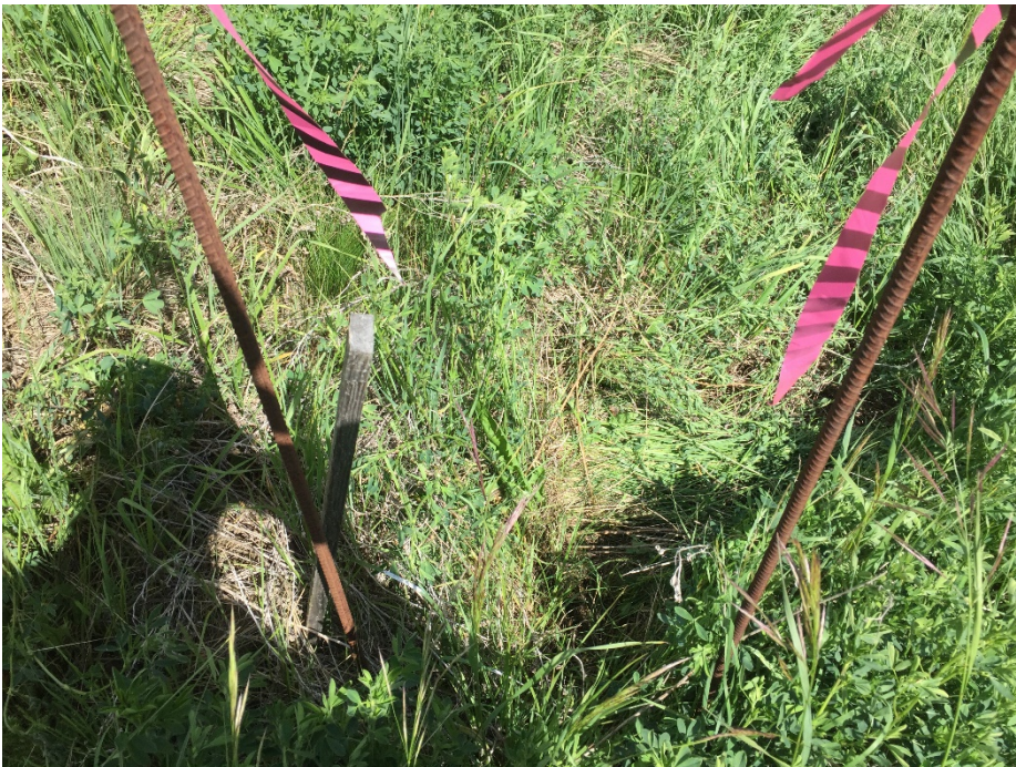
Photo II-36 Borrow Area A – crack monitoring rod location 103 (crack not visible).
