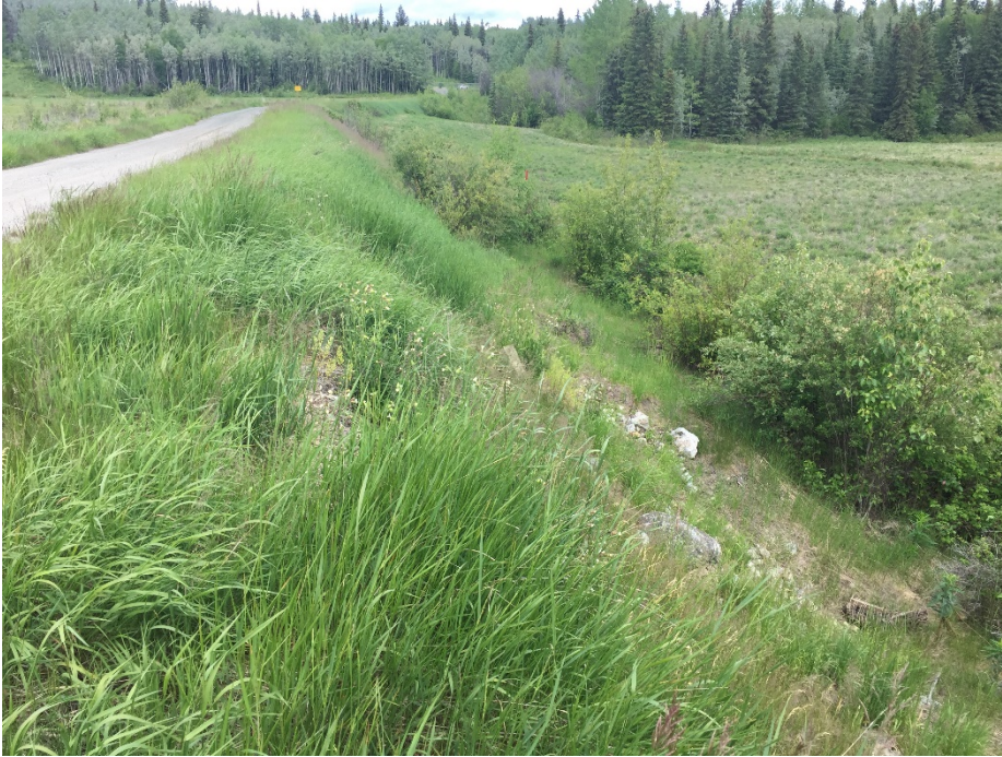
Photo II-5 Tailings Dam – east leg, looking north. Note vegetation on dam slope.
