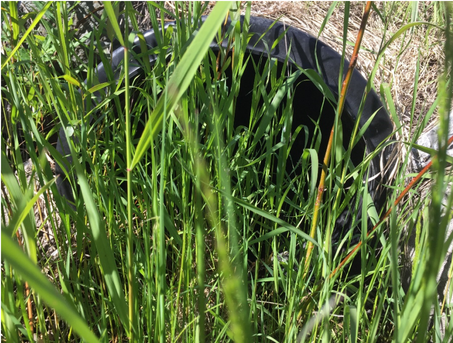
Photo II-31 Spillway Downstream Channel – close up of inlet to culvert beneath road to on-site residence. Note vegetation growth.
