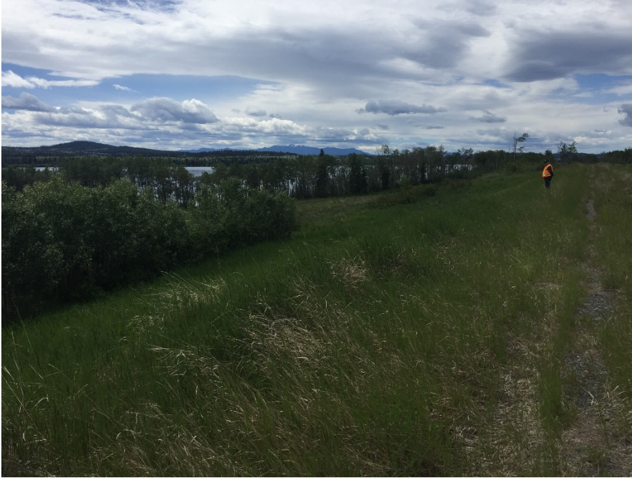
Photo II-9 Tailings Dam – south leg, looking west along downstream slope.
