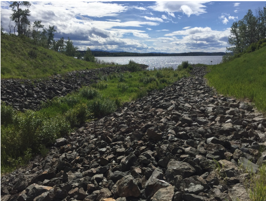
Photo II-42 Ed Creek Diversion Channel – outlet at Pinchi Lake.
