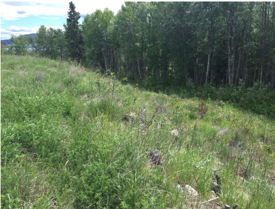
Photo II-16 Tailings Dam – west leg, looking south along downstream slope.
