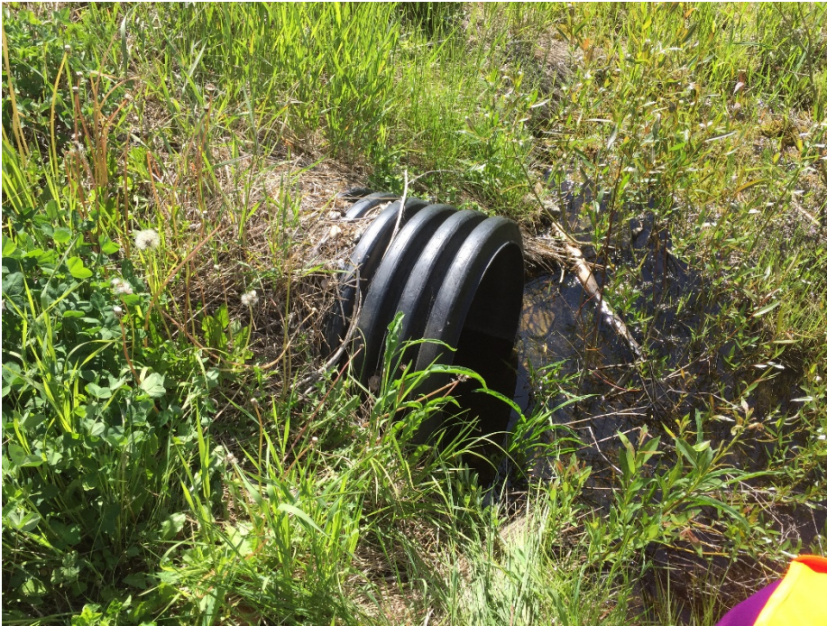
Photo II-33 Spillway Downstream Channel – outlet of culvert beneath road to former caretaker’s house.
