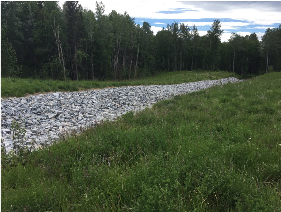
Photo II-26 Closure Spillway – looking downstream.
