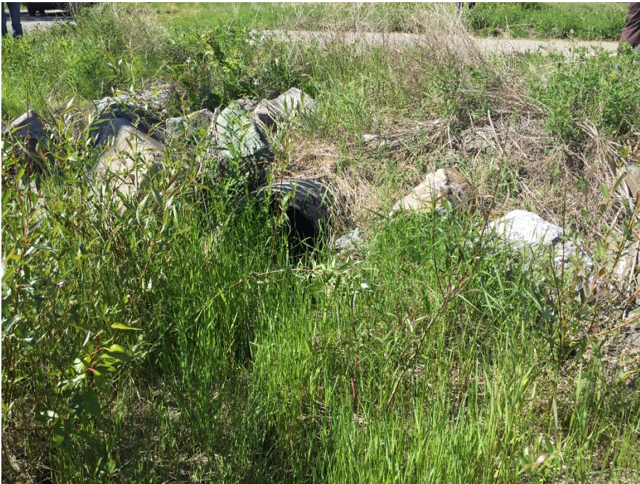
Photo II-30 Spillway Downstream Channel – inlet to culvert beneath road to on-site residence. Note vegetation growth.
