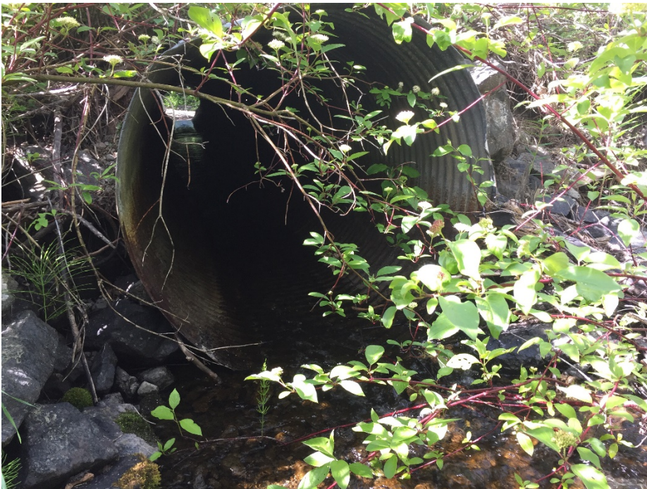
Photo II-56 Inlet of east culvert under Pinchi Lake Road.
