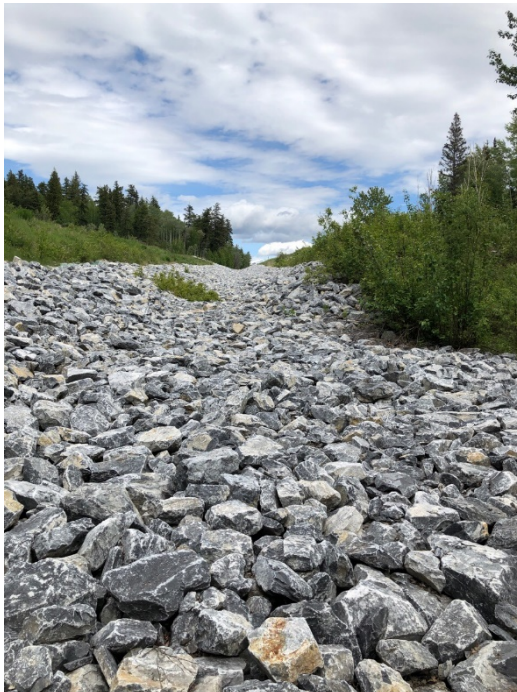
Photo II-28 Closure Spillway – looking upstream from downstream end of riprap.
