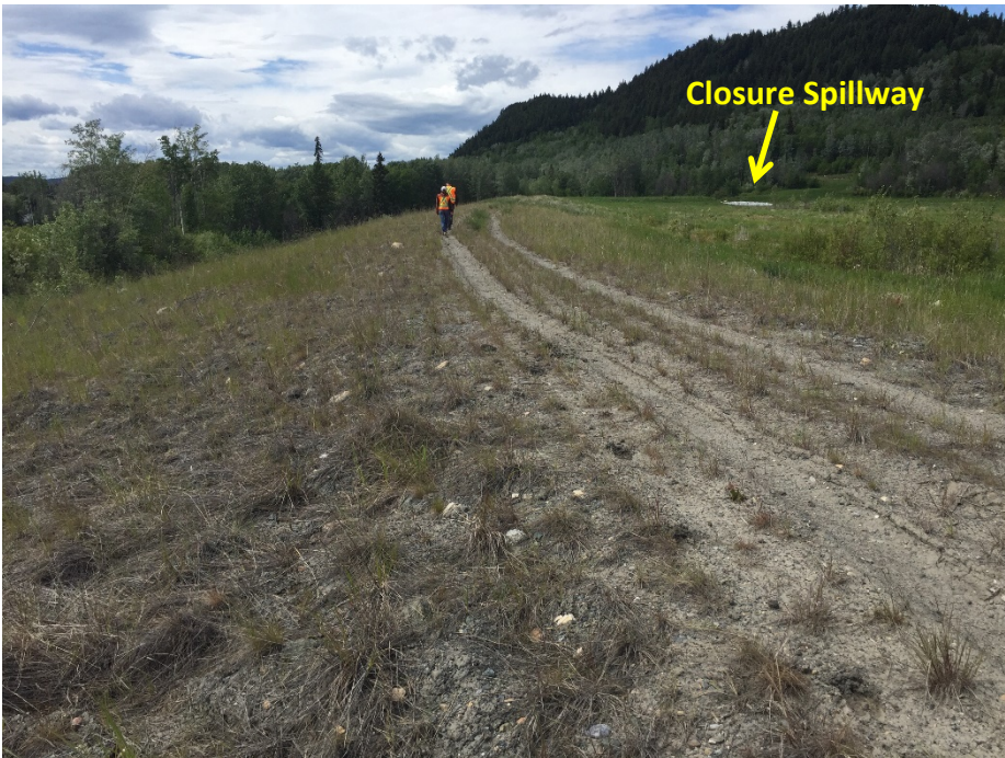
Photo II-10 Tailings Dam – southwest leg, looking northwest along the crest.
