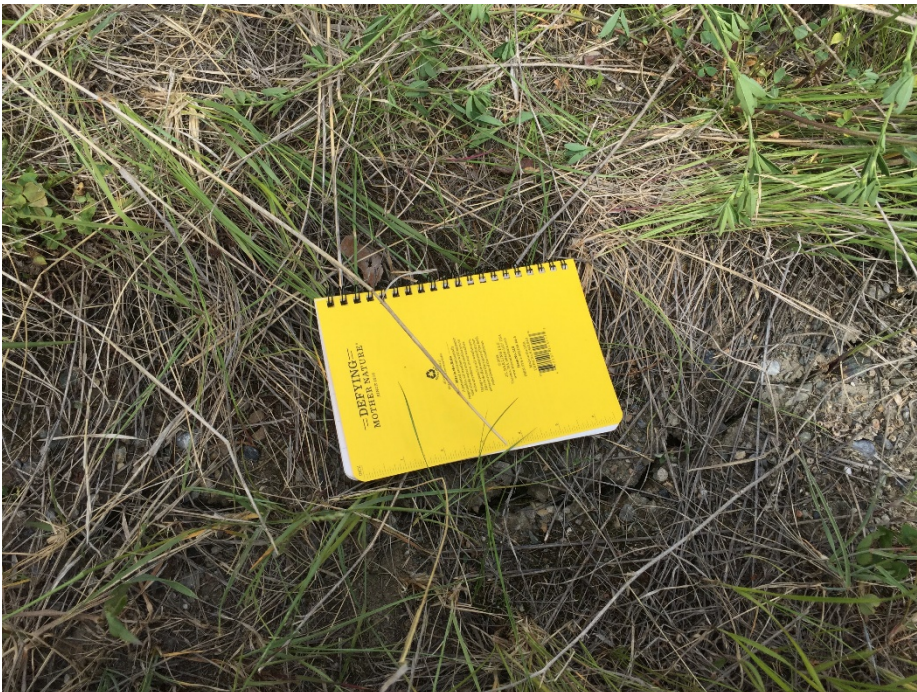
Photo II-14 Tailings Dam – southwest leg, crack on dam crest in tire track.
