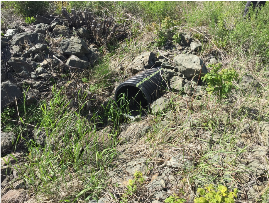
Photo II-52 Outlet of 460 mm culvert on north bank of Ed Creek Diversion Channel.
