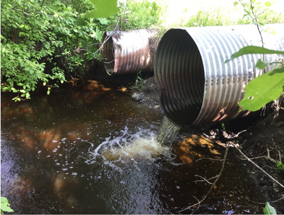
Photo II-57 Outlets of Ed Creek culverts under Pinchi Lake Road. Note only one culvert is flowing.
