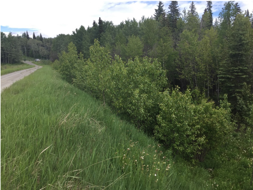
Photo II-2 Tailings Dam – east leg, looking north. Note vegetation on dam slope.
