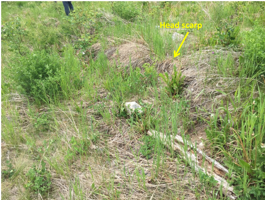
Photo II-27 Closure Spillway – head scarp of slump above right bank, 90 m downstream of centreline
