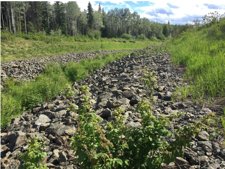
Photo II-48 Ed Creek Diversion Channel – looking downstream from between first and second bends.
