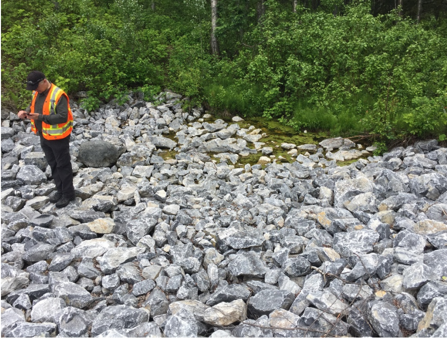
Photo II-29 Closure Spillway – pond at downstream end of riprap.
