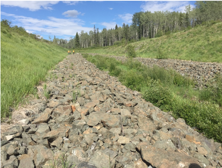
Photo II-46 Ed Creek Diversion Channel – looking upstream from between second and third bends.
