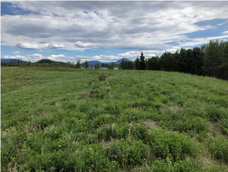
Photo II-17 Tailings Dam – west leg, looking south along upstream slope. Covered tailings surface is on the left.
