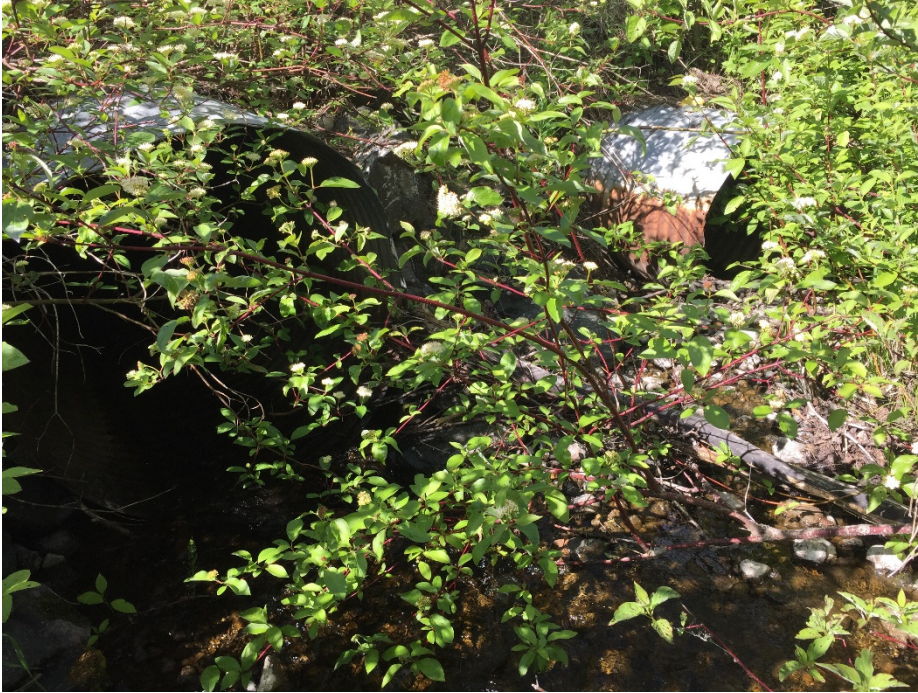
Photo II-55 Inlets of Ed Creek culverts under Pinchi Lake Road.
