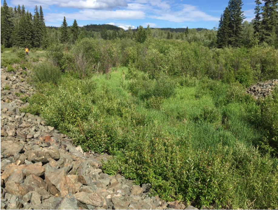
Photo II-51 Ed Creek Diversion Channel – looking upstream towards first bend.
