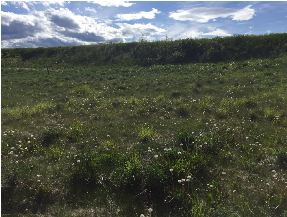
Photo II-4 Tailings Dam – east leg, looking upstream from toe.
