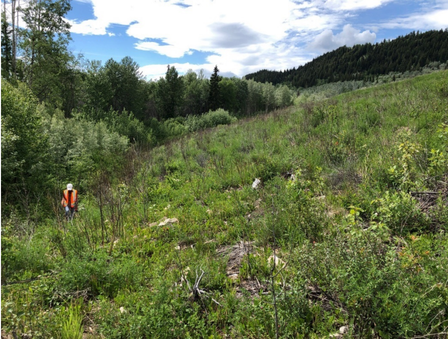
Photo II-13 Tailings Dam – southwest leg, looking northwest along the downstream slope.
