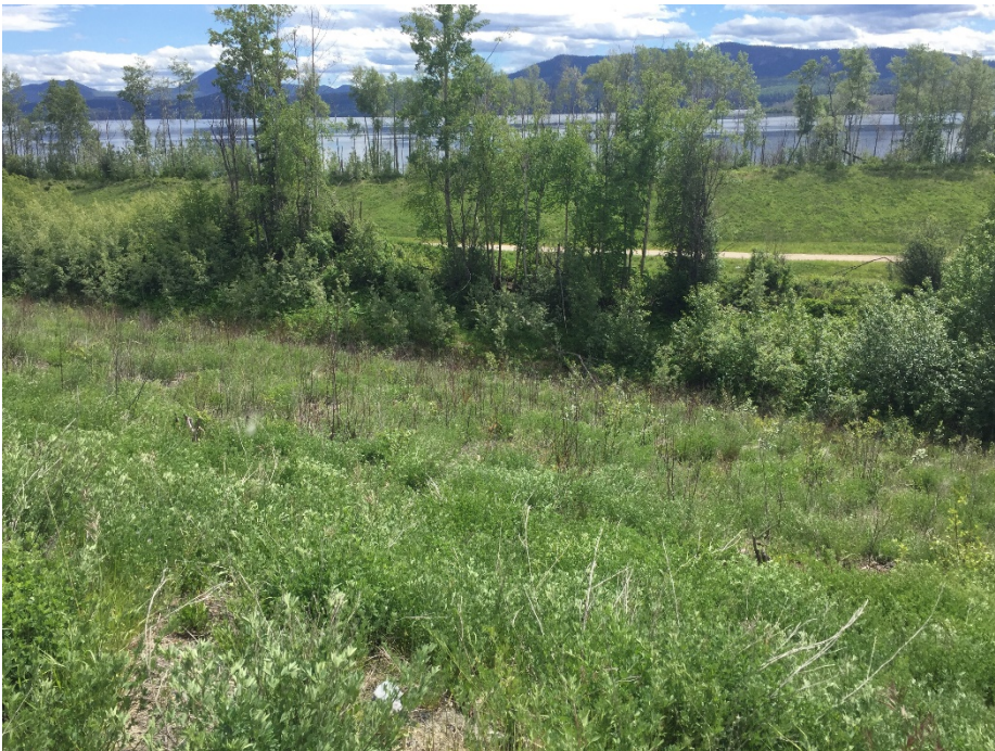
Photo II-12 Tailings Dam – southwest leg, looking downstream from the crest.
