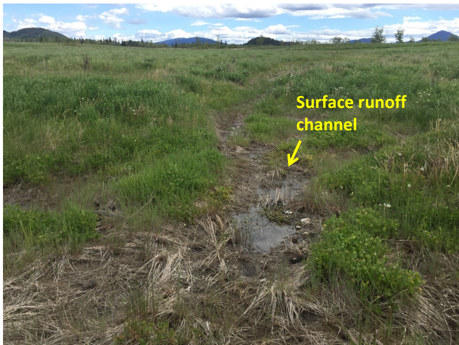
Photo II-22 Downstream end of surface runoff channel in tailings cover, looking southeast from Closure Spillway.
