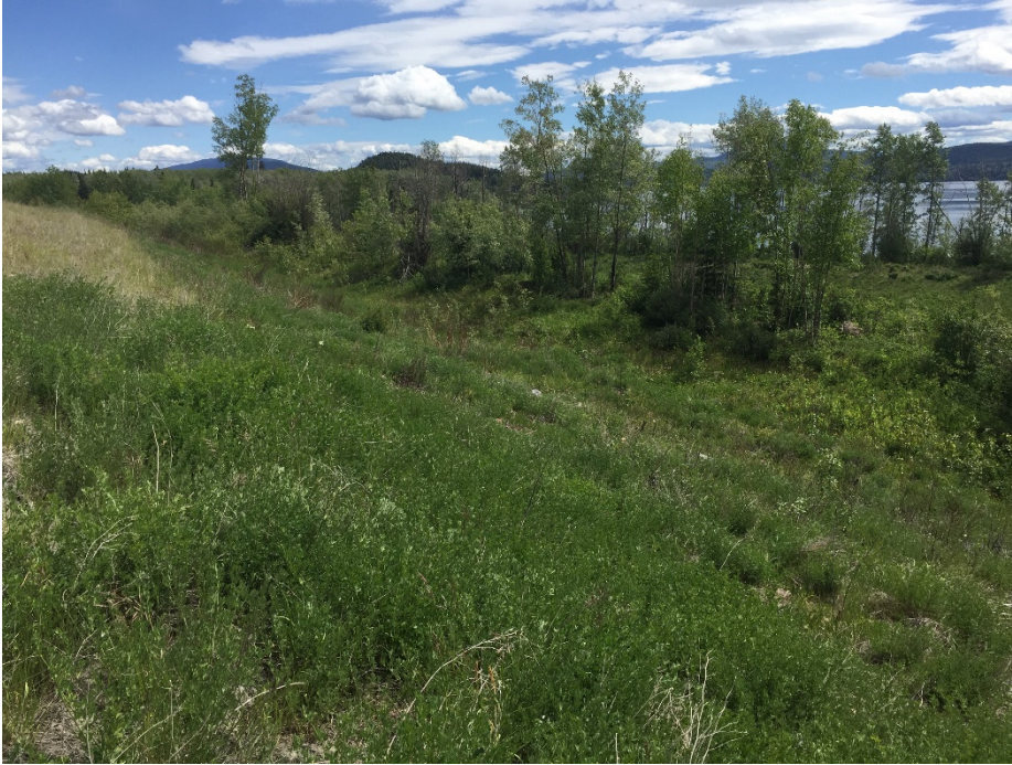
Photo II-11 Tailings Dam – southwest leg, looking southeast along the downstream slope.
