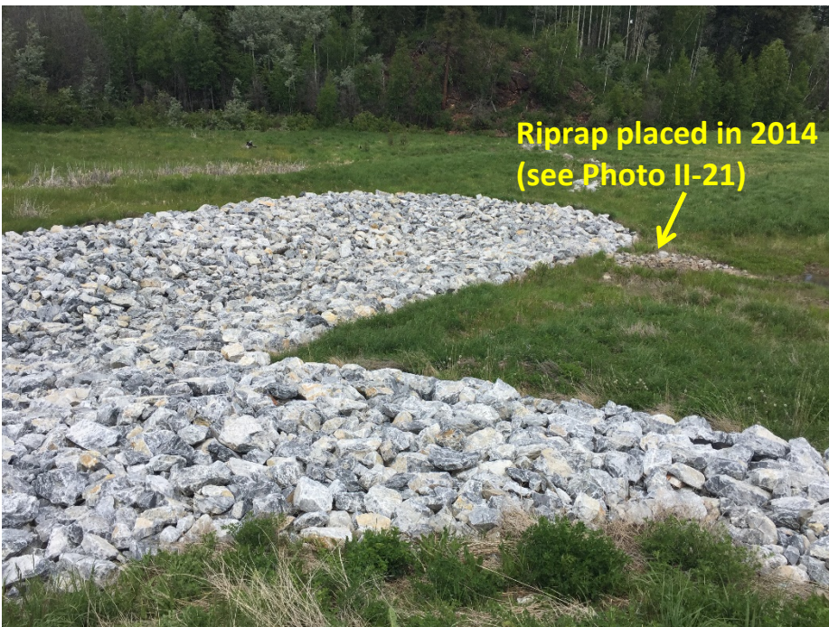
Photo II-20 Closure Spillway – inlet apron.
