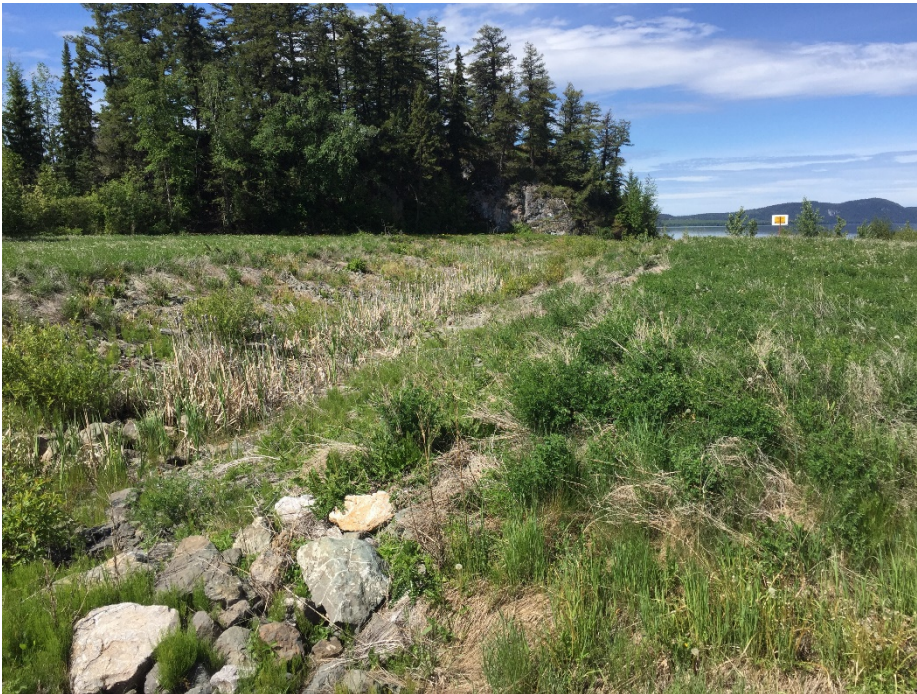
Photo II-34 Spillway Downstream Channel – Lower Reach, looking downstream.
