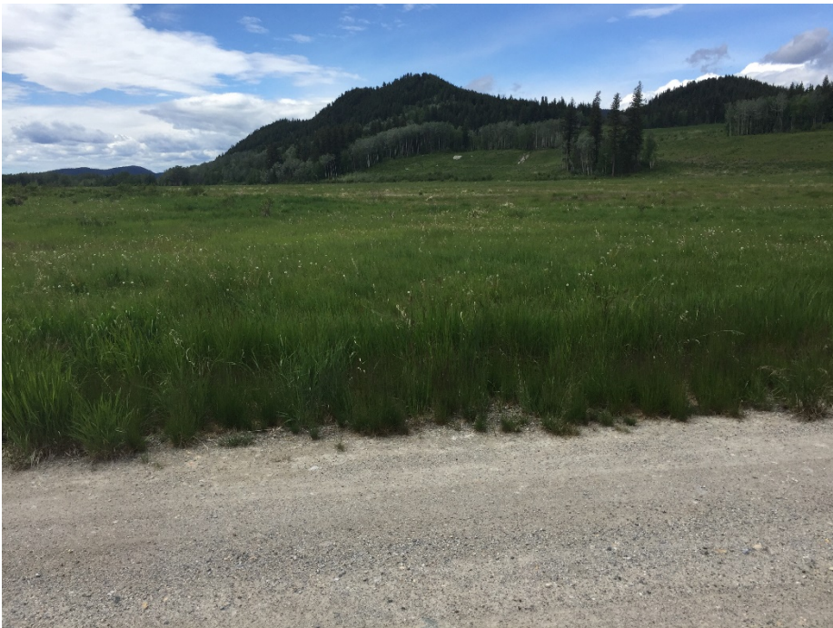
Photo II-6 Tailings Dam – east leg, looking west at the covered tailings surface.
