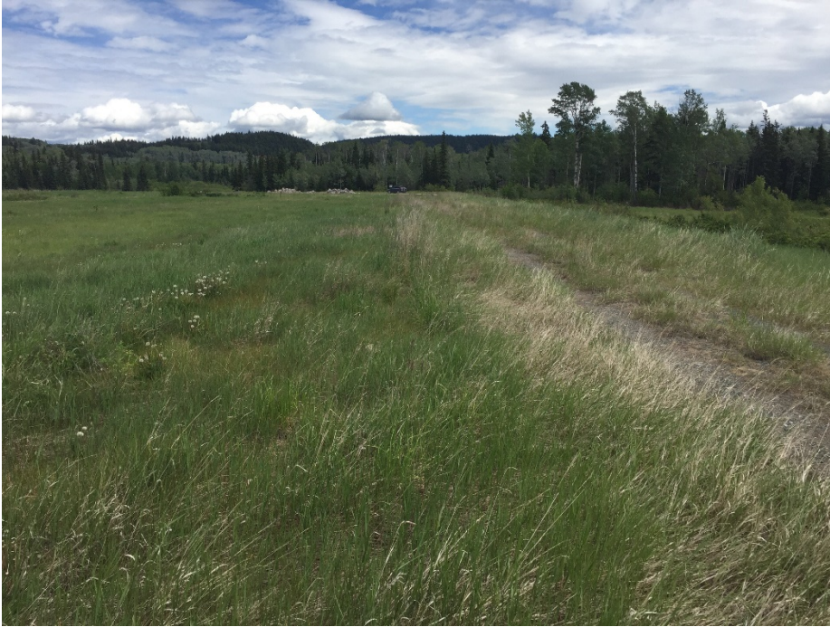
Photo II-7 Tailings Dam – south leg, looking east towards Ed Creek.
