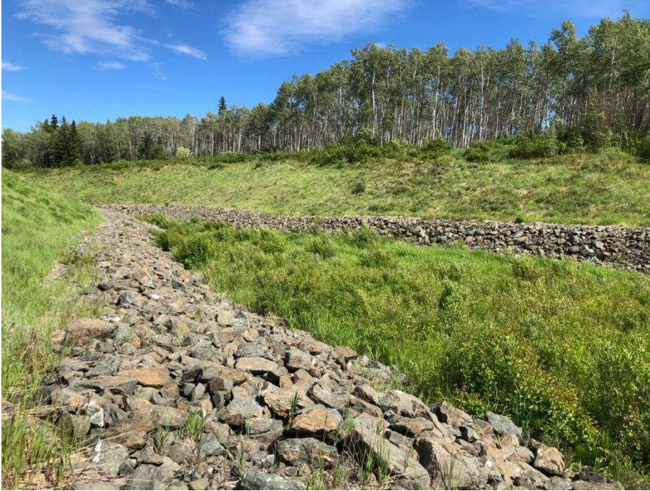
Photo II-43 Ed Creek Diversion Channel – looking upstream from near outlet.
