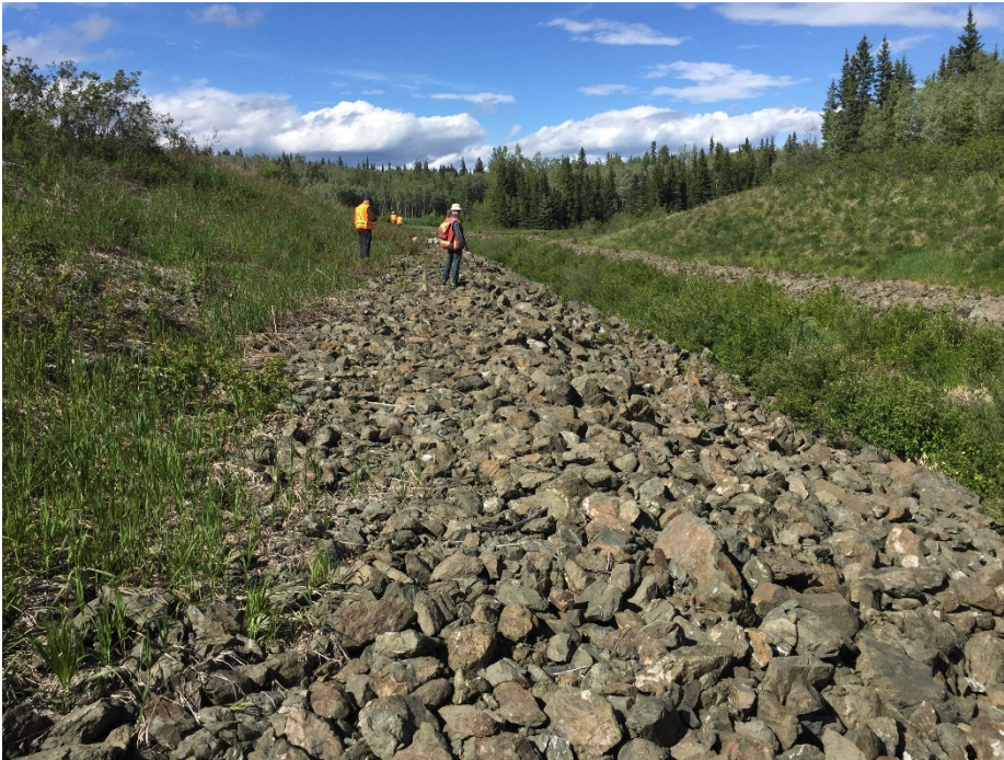
Photo II-49 Ed Creek Diversion Channel – looking upstream from between first and second bends.
