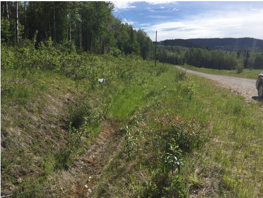
Photo II-40 Road ditch above tailings impoundment, looking east.
