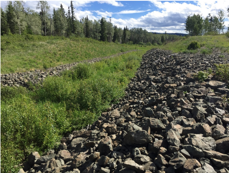
Photo II-50 Ed Creek Diversion Channel – looking downstream from near first bend.
