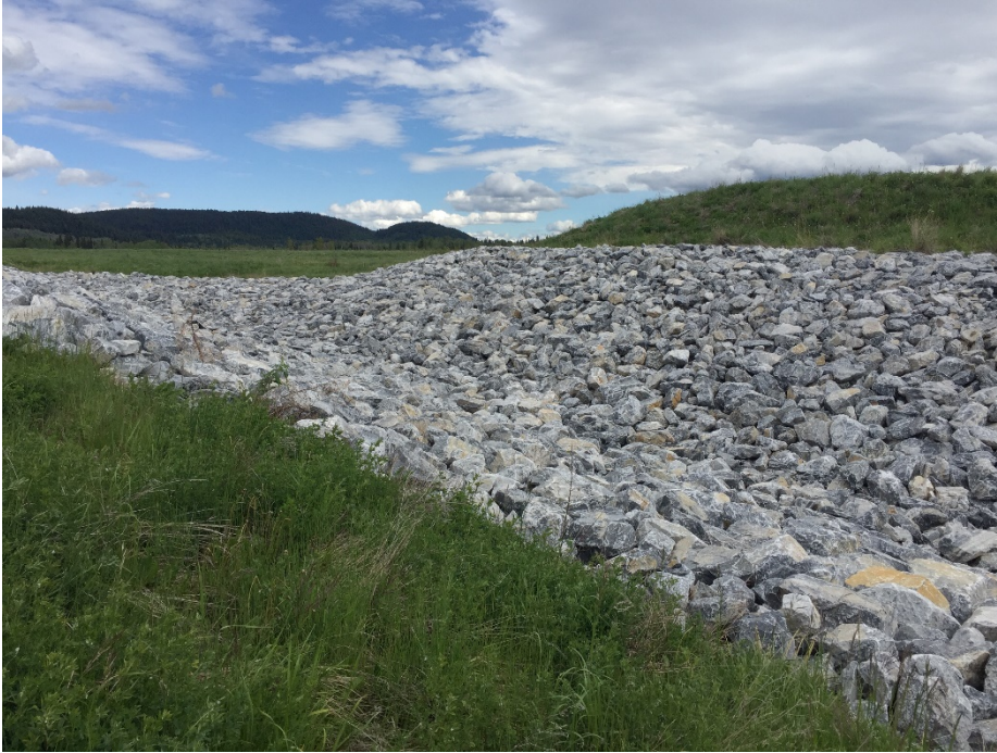
Photo II-25 Closure Spillway – looking upstream from dam toe area.
