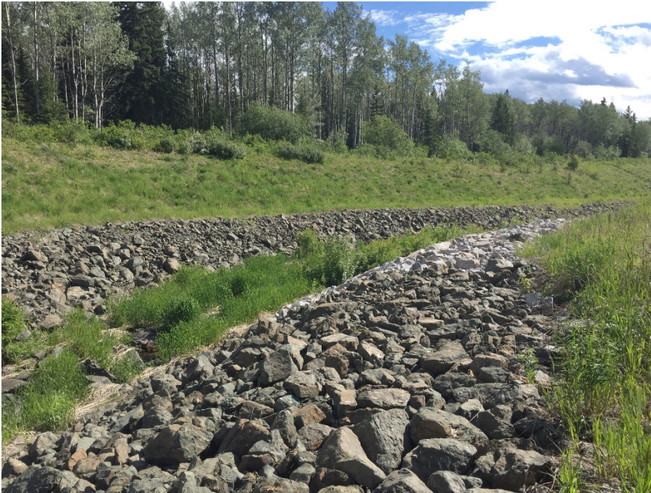
Photo II-47 Ed Creek Diversion Channel – looking downstream from near second bend. Light-coloured area of riprap was replaced in 2014, and is in good condition.
