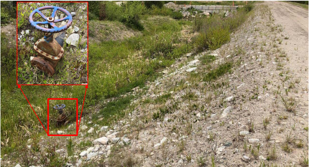
Photo II-B-30 S5 Pond: Overview of downstream slope and blocked outlet pipe daylighting at toe, looking north (HGH-2019-35)
