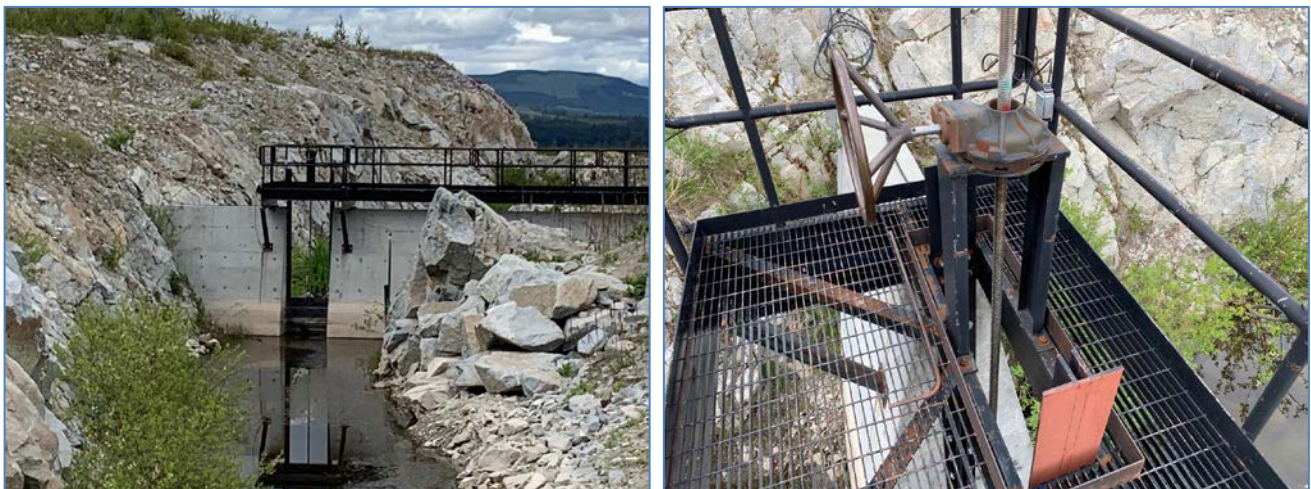
Photo II-A-17 Spillway flow control gate – No signage or safety grating is present at valve. (HGH-2019-15)
