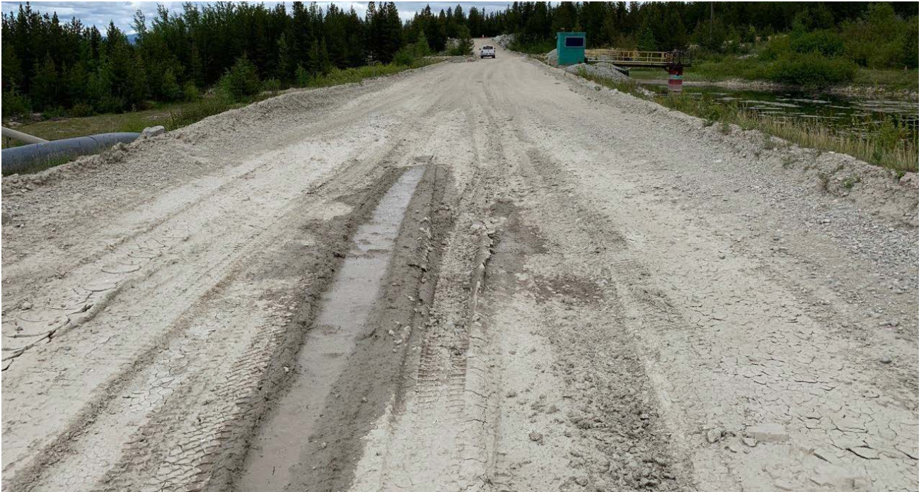
Photo II-B-32 S8 Pond: Downstream slope; looking east from left abutment. Pipe on slope is not connected to anything and should be removed (HGH-2019-40)
