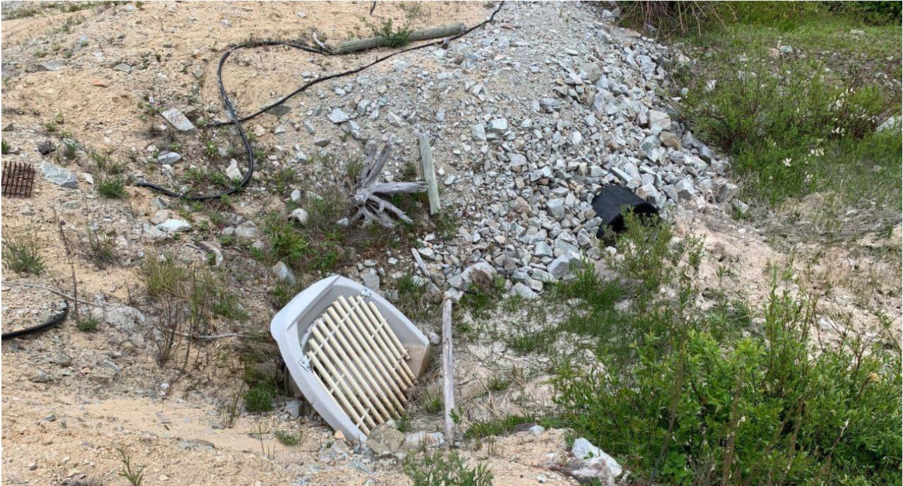
Photo II-B-35 S8 Pond: Overview of overflow pipe. Trash rack is clear of debris; and water level observed below invert. Second pipe discharges into pond from east ditch. (HGH-2019-39)
