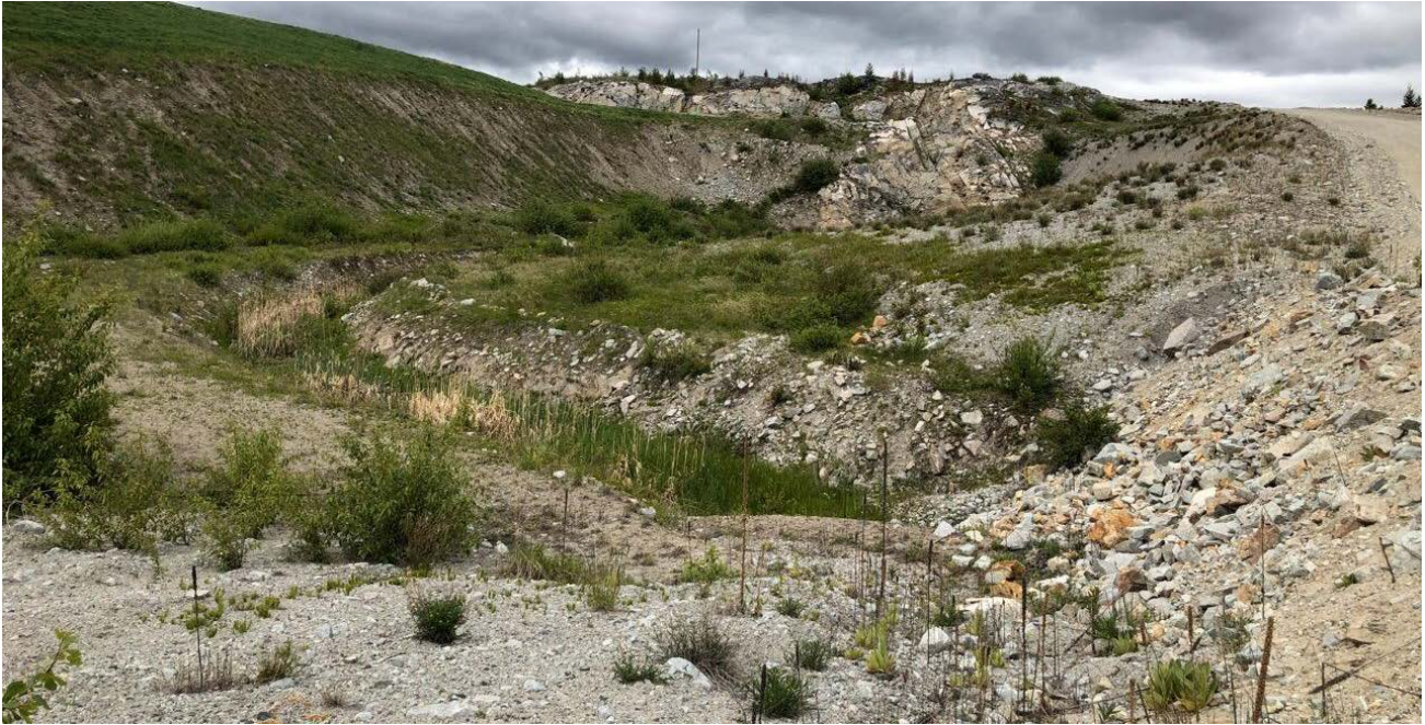
Photo II-A-21 Highmont Spillway channel downstream of rock chute, portion of channel where base is not in bedrock and has been covered with riprap (HGH-2019-17)
