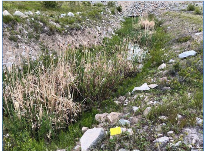
Photo II-A-23 Inlet of 33" ID Highmont Spillway culverts crossing toe access road. Channel is vegetated in this area. No flow was observed through the culverts. (HGH-2019-07)
