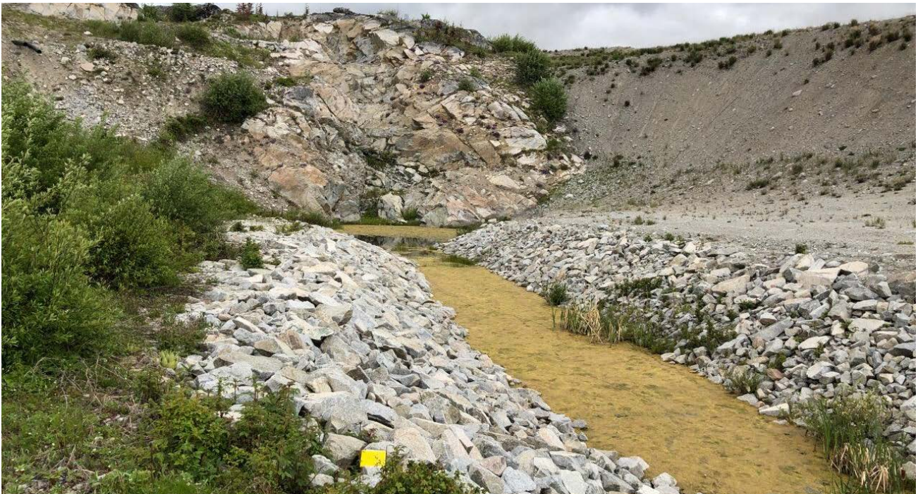
Photo II-A-21 Highmont Spillway channel downstream of rock chute, portion of channel where base is not in bedrock and has been covered with riprap (HGH-2019-17)
