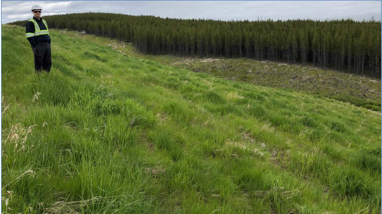
Photo II-A-6 Overview of East Dam downstream slope, looking northeast. Slope covered by vegetation (HGH-2019-04)
