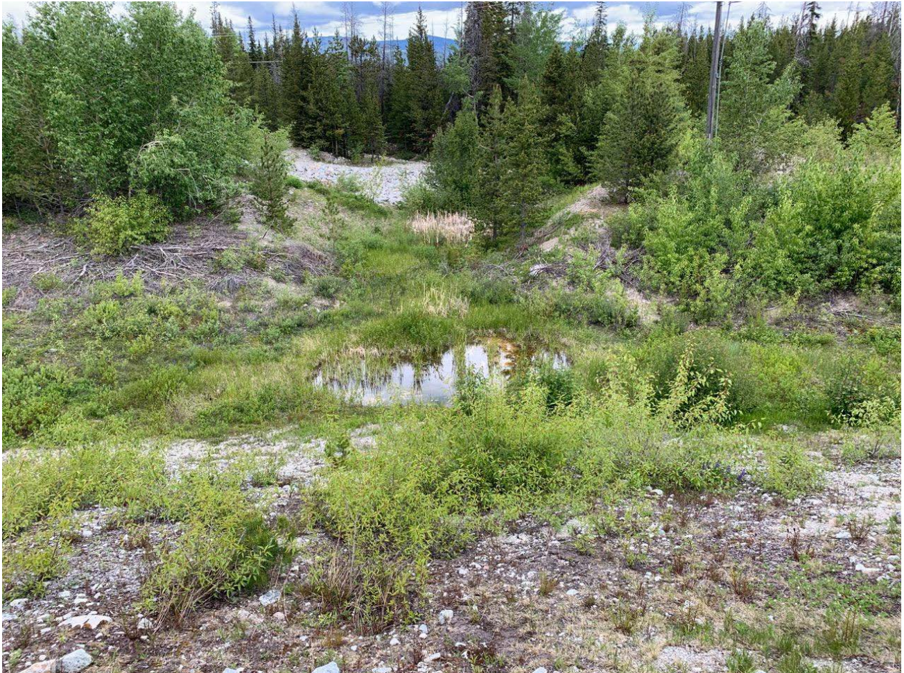
Photo II-B-14 S2 Pond: Ponded water at downstream toe, similar in size to the pond noted during previous year DSIs (HGH-2019-28)
