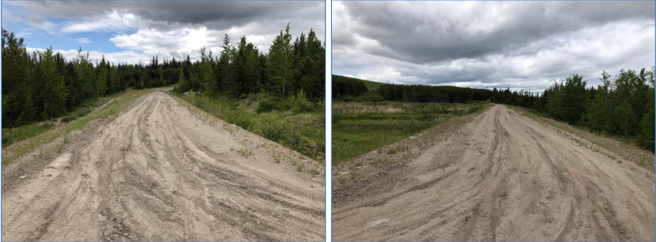
Photo II-B-22 S5 Pond: perimeter crest of pumping sub-cell, looking south, both outlet pipes are blocked and the low point of the crest is the right (south) abutment (HGH-2019-35)
