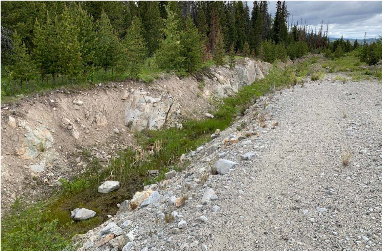
Photo II-A-26 Highmont Spillway plug across S2 Pond inlet channel. No sign of recent flow in spillway or inlet channel (HGH-2019-20)
