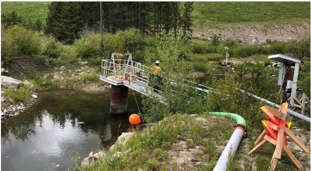
Photo II-B-18 S3 Pond: Catwalk and outlet pump to Highmont Distribution Box; personal flotation devices are in place (HGH-2019-32)
