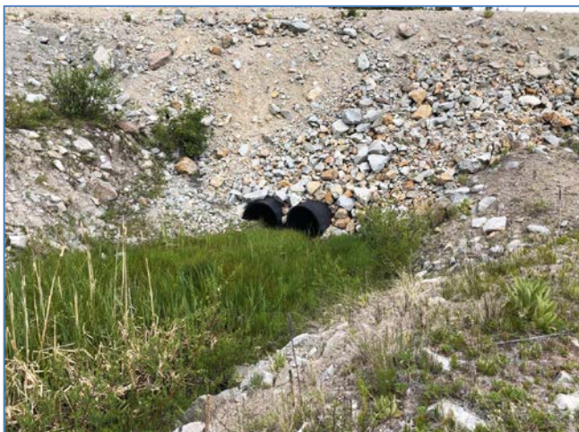
Photo II-A-23 Inlet of 33" ID Highmont Spillway culverts crossing toe access road. Channel is vegetated in this area. No flow was observed through the culverts. (HGH-2019-07)
