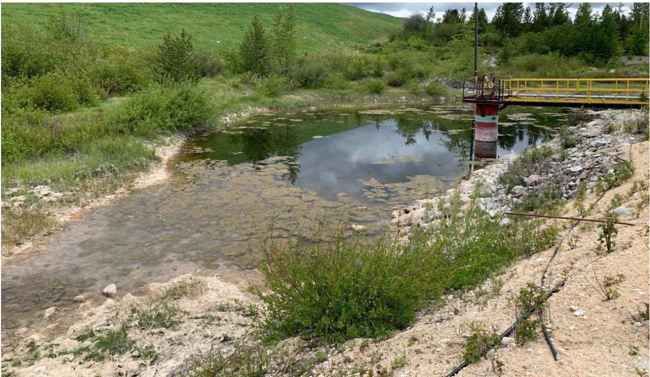
Photo II-B-34 S8 Pond: Overview of impoundment, catwalk and outlet pump to S1 Pond (HGH-2019-41)
