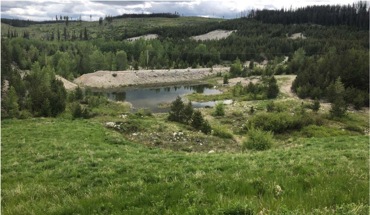
Photo II-A-10 Overview of the South Dam downstream slope and seepage weir upstream of S3 Pond. Flow is clear. No seepage face observed on dam slope (HGH-2019-09)
