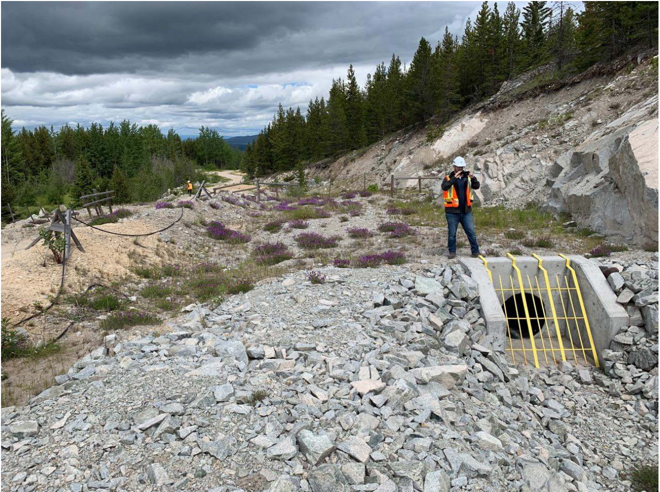
Photo II-B-6 S1 Pond: Spillway channel and pipe intake looking downstream. Pipe intake is clear with no sign of vegetation or any other obstructions. (HGH-2019-24)
