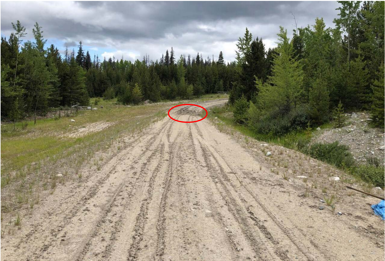
Photo II-B-22 S5 Pond: perimeter crest of pumping sub-cell, looking south, both outlet pipes are blocked and the low point of the crest is the right (south) abutment (HGH-2019-35)
