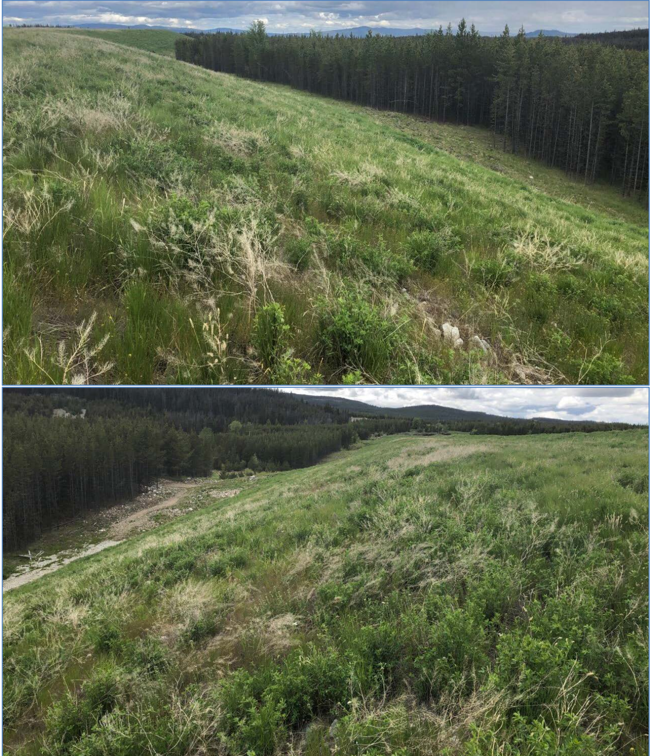
Photo II-A-7 Overview of South Dam downstream slope. Slope covered by vegetation (HGH-2019-05)
