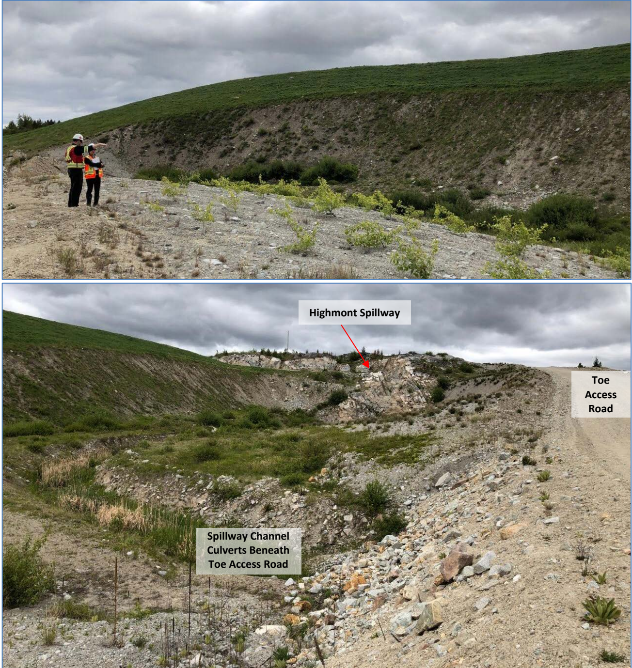
Photo II-A-8 Overview of North Dam downstream slope and toe, downstream of Highmont Spillway (HGH-2019-06 )
