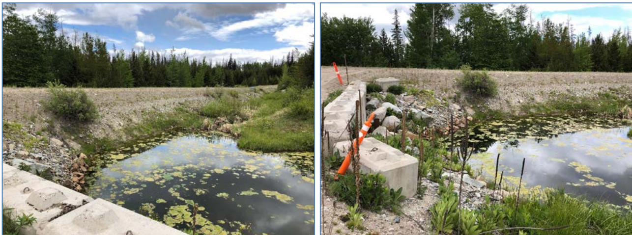
Photo II-B-28 S5 Pond: Overview of Pumping Sub-cell and overflow point over internal dyke which is below perimeter crest (HGH-2019-37)
