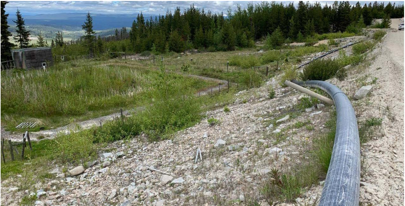
Photo II-B-32 S8 Pond: Downstream slope; looking east from left abutment. Pipe on slope is not connected to anything and should be removed (HGH-2019-40)
