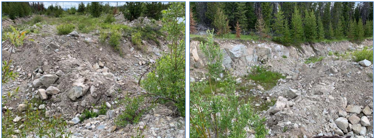
Photo II-A-26 Highmont Spillway plug across S2 Pond inlet channel. No sign of recent flow in spillway or inlet channel (HGH-2019-20)
