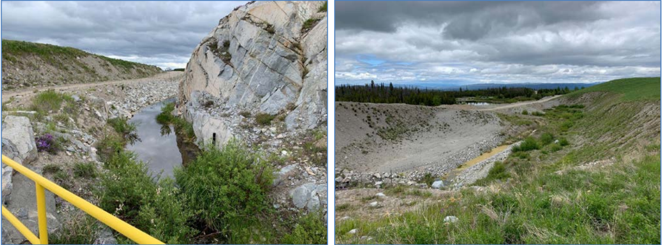
Photo II-A-19 Highmont Spillway channel looking at inlet to S1 Pond diversion – Trash rack on invert is clear of debris and water is flowing through diversion (HGH-2019-16)
