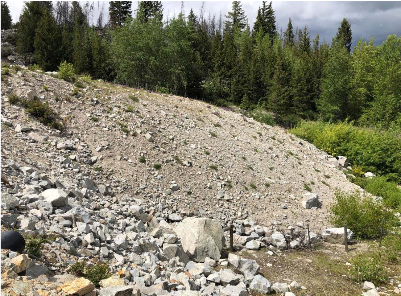
Photo II-B-2 S1 Pond: Overview of S1 Pond dam downstream slope (HGH-2019-22)
