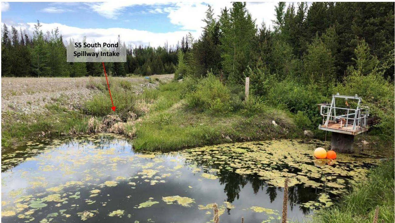
Photo II-B-28 S5 Pond: Overview of Pumping Sub-cell and overflow point over internal dyke which is below perimeter crest (HGH-2019-37)
