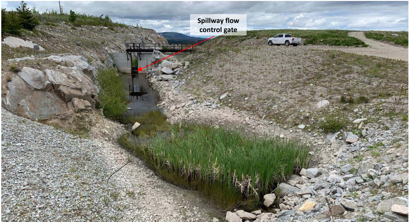
Photo II-A-17 Spillway flow control gate – No signage or safety grating is present at valve. (HGH-2019-15)
