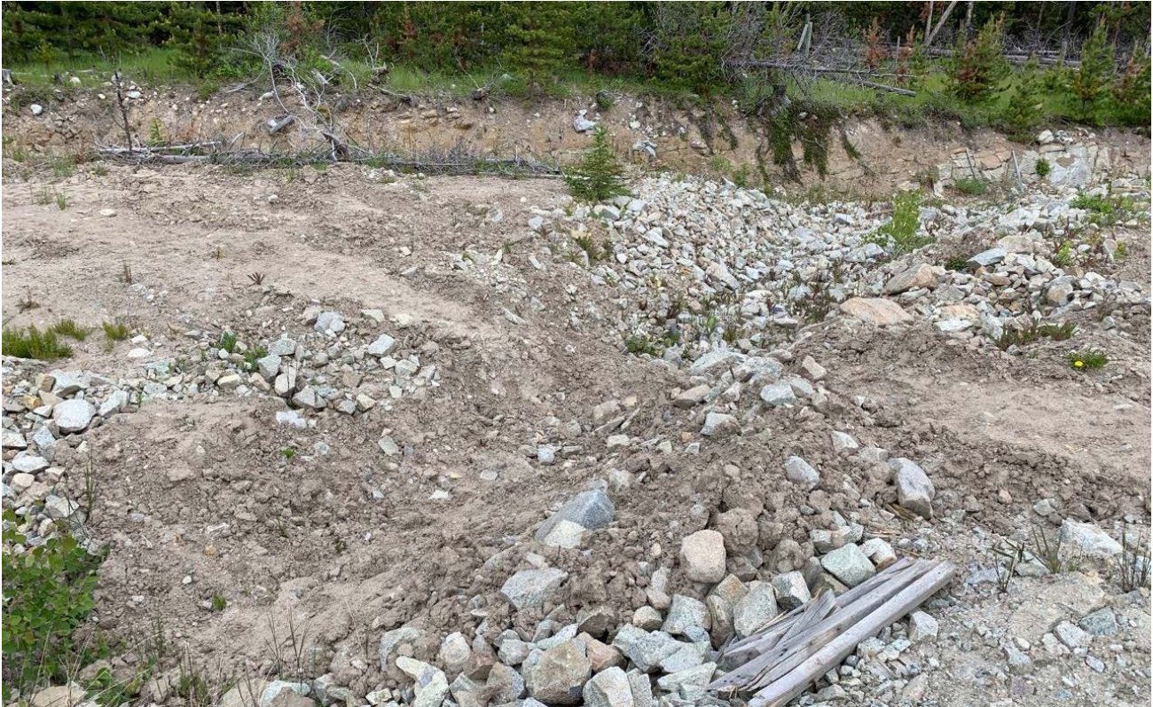
Photo II-B-13 S2 Pond: S2 Pond Spillway invert and channel; remnant of a temporary access built over the channel remains in place has reduced the spillway flow channel and should be removed as part of routine maintenance before freshet (HGH-2019-29)
