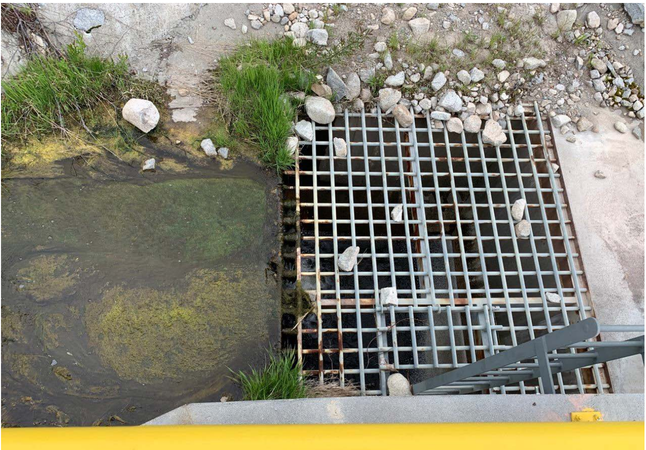
Photo II-A-19 Highmont Spillway channel looking at inlet to S1 Pond diversion – Trash rack on invert is clear of debris and water is flowing through diversion (HGH-2019-16)
