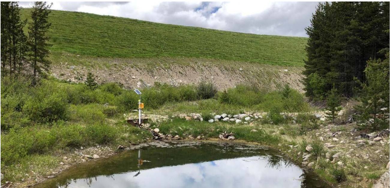
Photo II-A-10 Overview of the South Dam downstream slope and seepage weir upstream of S3 Pond. Flow is clear. No seepage face observed on dam slope (HGH-2019-09)
