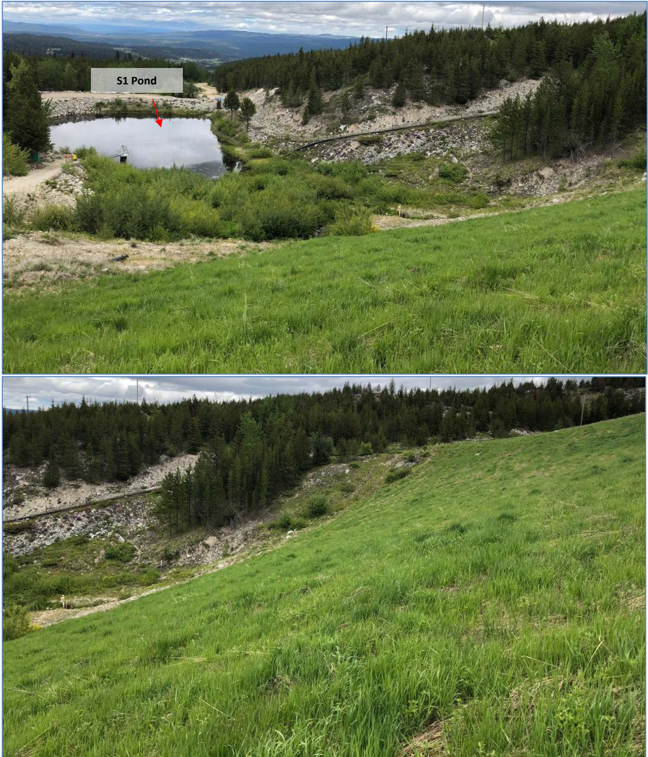
Photo II-A-4 Overview of North Dam downstream toe and S1 Pond. No signs of distress or deformations (HGH-2019-02)
