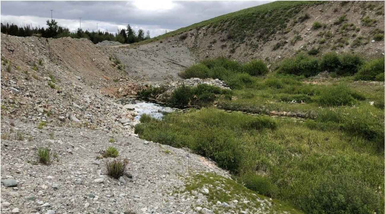
Photo II-A-23 Inlet of 33" ID Highmont Spillway culverts crossing toe access road. Channel is vegetated in this area. No flow was observed through the culverts. (HGH-2019-07)
