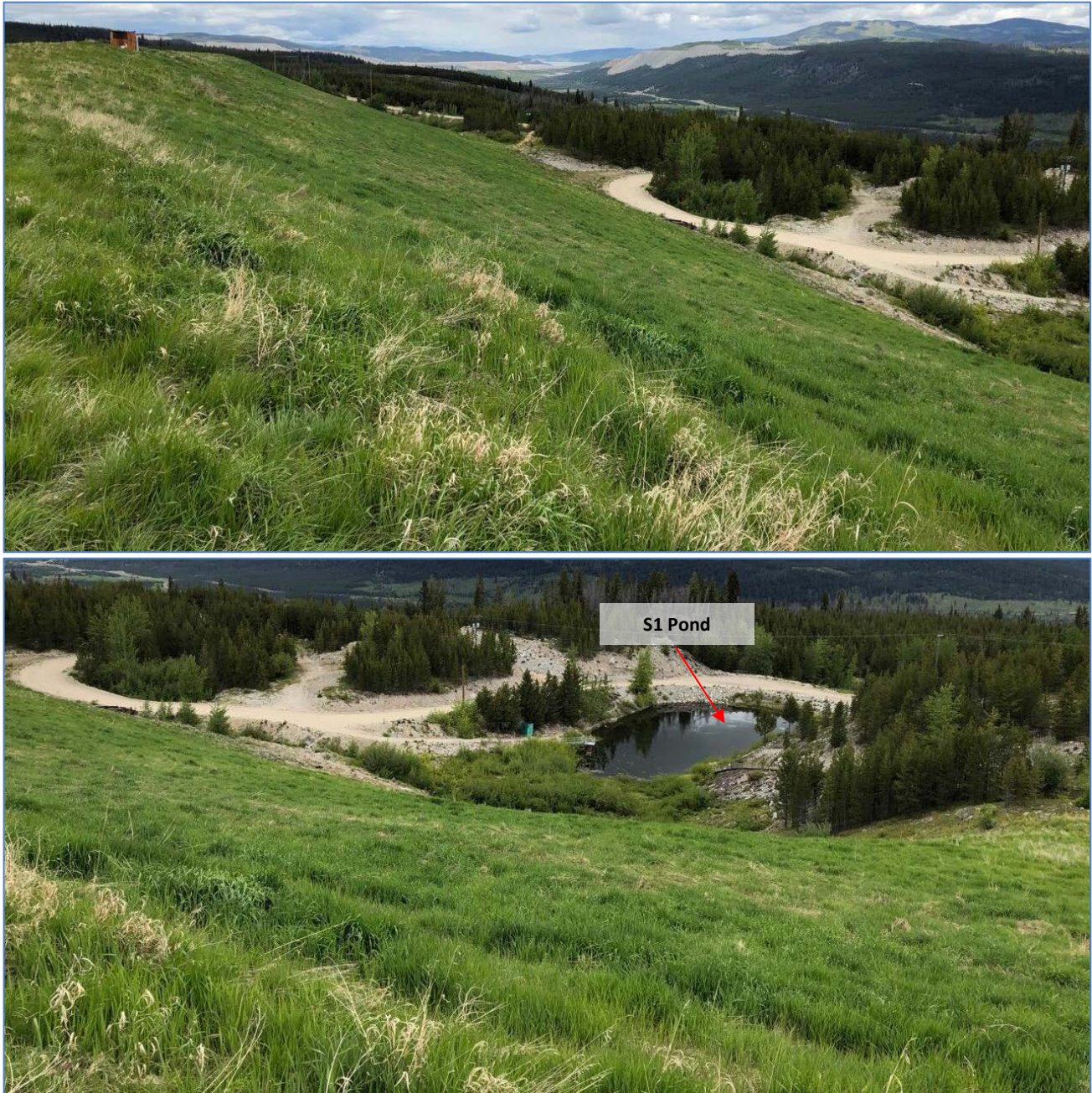
Photo II-A-5 Overview of North Dam downstream slope downstream of P2. No signs of distress or deformations. (HGH-2019-03)
