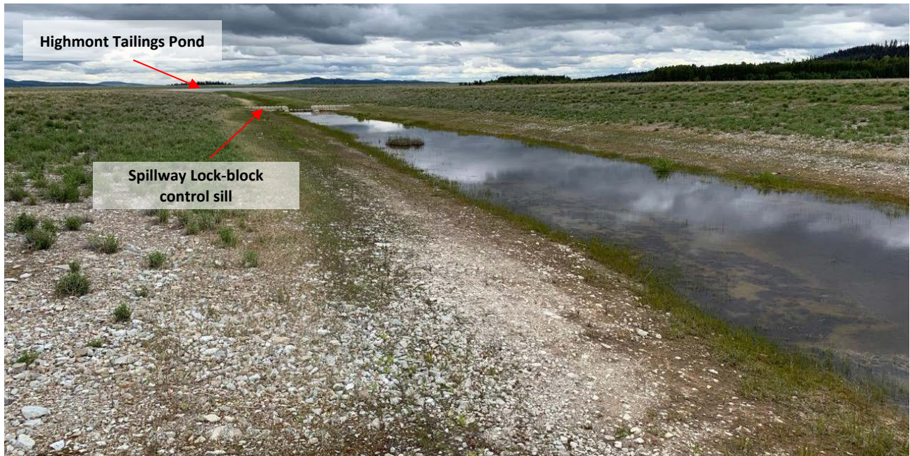
Photo II-A-14 Highmont Spillway approach channel, concrete lock-block control sill – Spillway is inactive. Water ponded downstream of sill is controlled by level at spillway flow control gate (HGH-2019-14)
