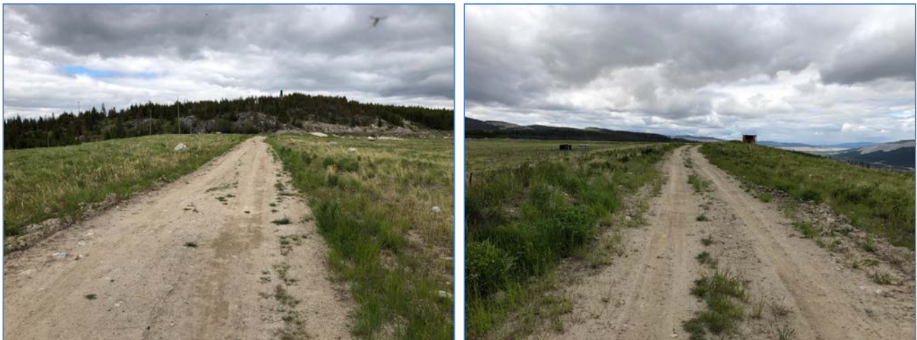
Photo II-A-2 Overview of North Dam crest. No signs of distress, settlement or depression. (HGH-2019-01)
