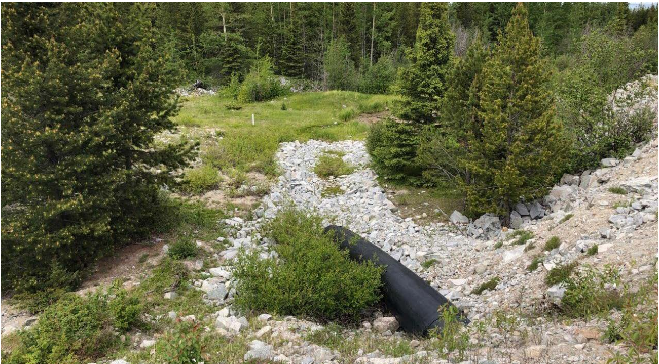
Photo II-B-8 S1 Pond: Spillway pipe outlet with no obstruction (HGH-2019-26)
