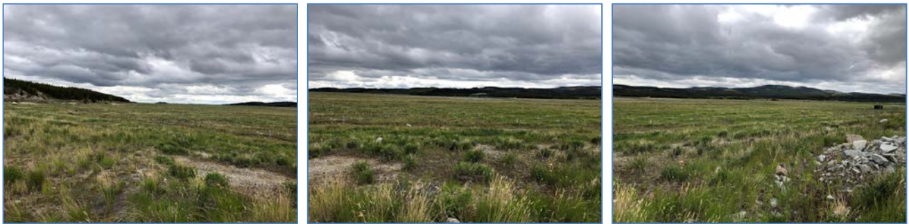
Photo II-A-2 Overview of North Dam crest. No signs of distress, settlement or depression. (HGH-2019-01)
