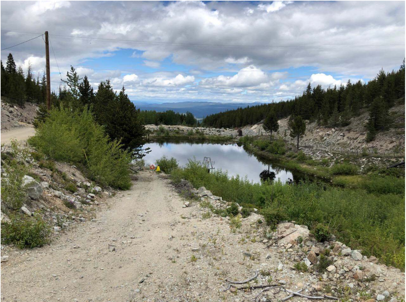
Photo II-B-3 S1 Pond: Overview of pond and upstream slope of dam, looking north. (HGH-2019-23)
