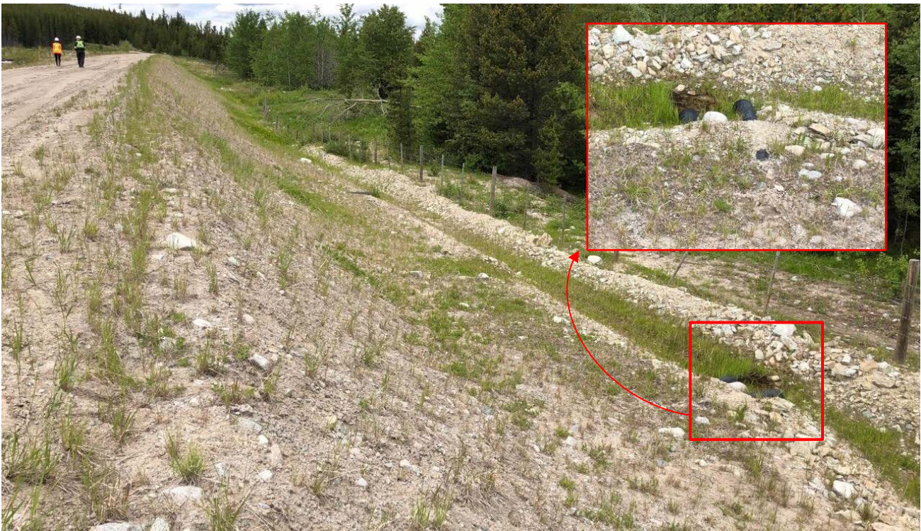
Photo II-B-30 S5 Pond: Overview of downstream slope and blocked outlet pipe daylighting at toe, looking north (HGH-2019-35)
