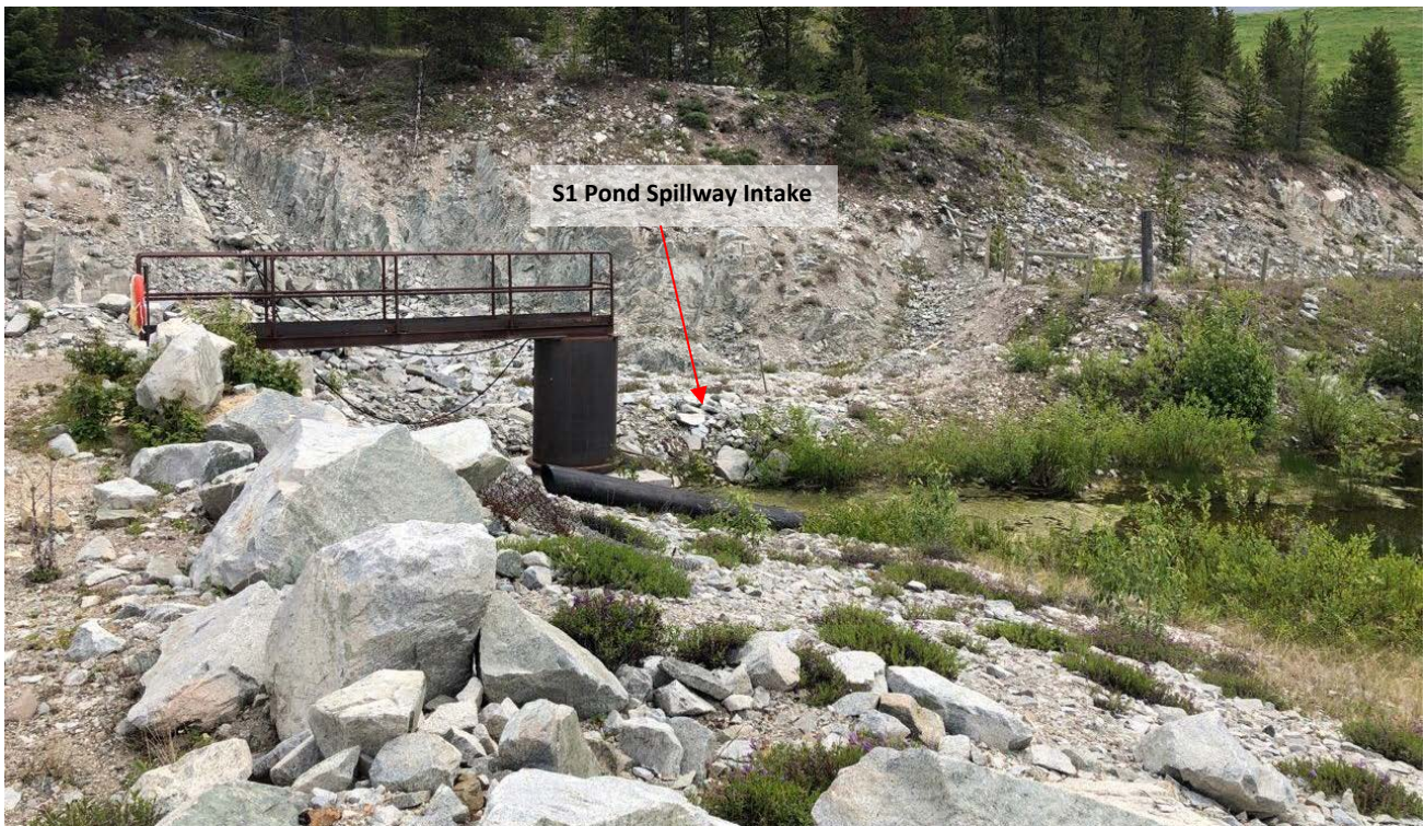
Photo II-B-5 S1 Pond: Overview of upstream slope and S1 Pond Spillway intake. (HGH-2019-23)
