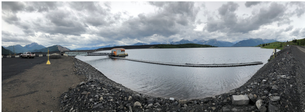
Photograph 3: Main Tailings Dam – Reclaim Barge; looking Southwest, 17 July 2019
