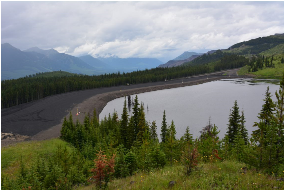
Photograph 23: West Tailings Dam – Crest and South and North Abutments; looking North, 17 July 2019
