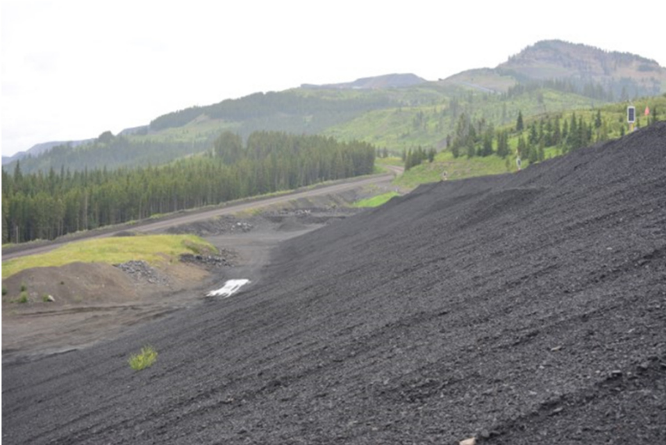
Photograph 22: West Tailings Dam – Downstream Slope and Toe Area; looking North, 17 July 2019
