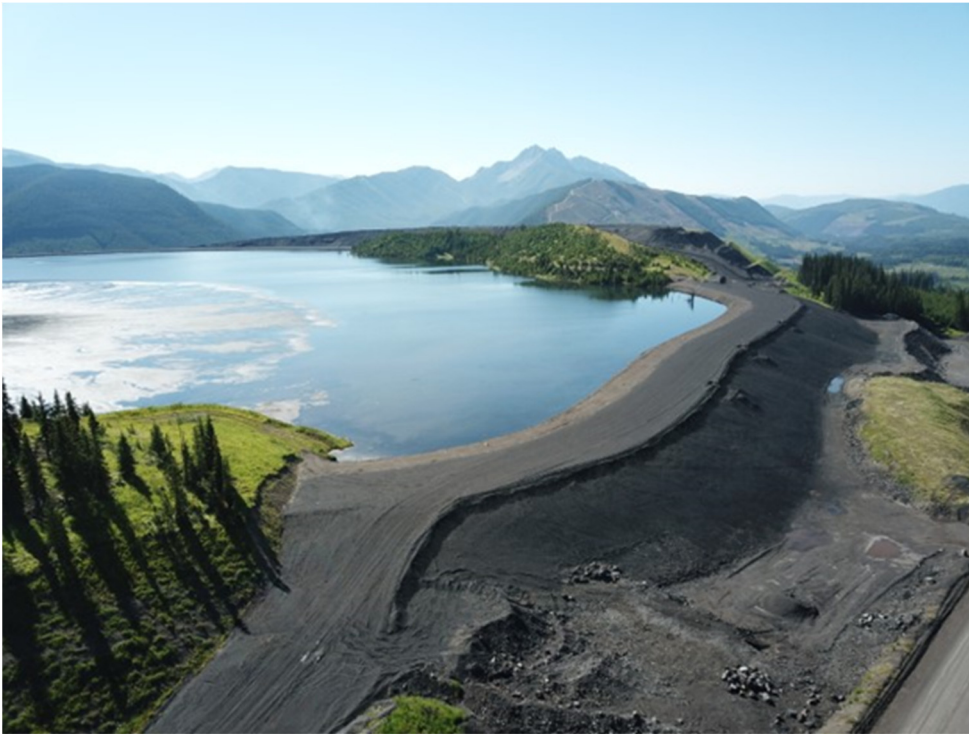
Photograph 19: West Tailings Dam – looking Southeast, 26 September 2019
