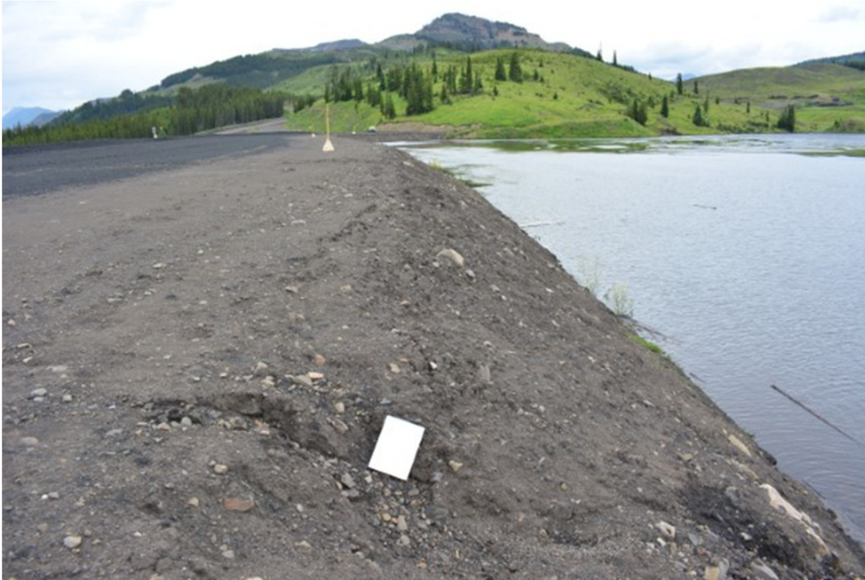
Photograph 21: West Tailings Dam – crest and Upstream Slope, Minor Erosion Rill on Upstream Slope; looking North, 17 July 2019
