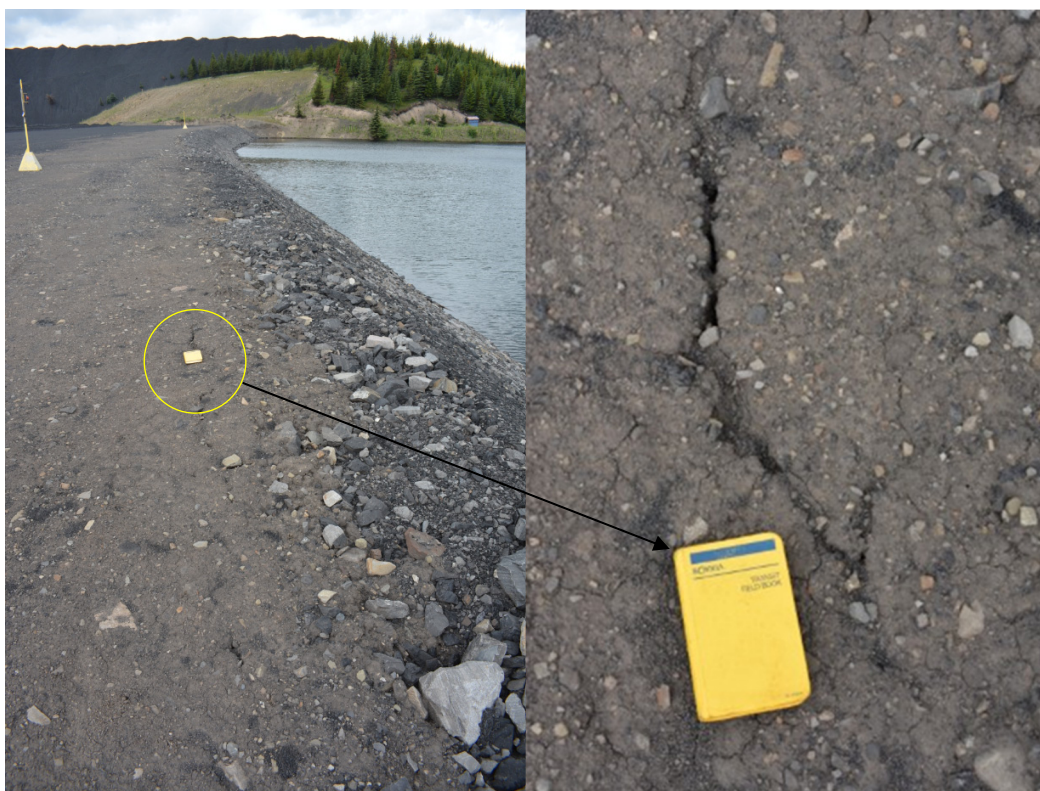
Photograph 6a (left) and 6b (right): Main Tailings Dam – Minor Longitudinal Cracks on Crest Adjacent to Riprap on Upstream Slope; looking Southwest, 17 July 2019
