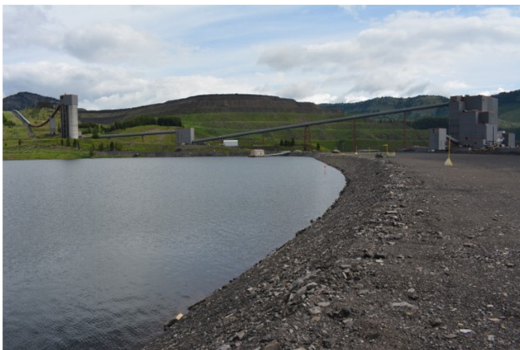
Photograph 4: Main Tailings Dam – Upstream Slope, Crest and East Abutment; looking Northeast, 17 July 2019
