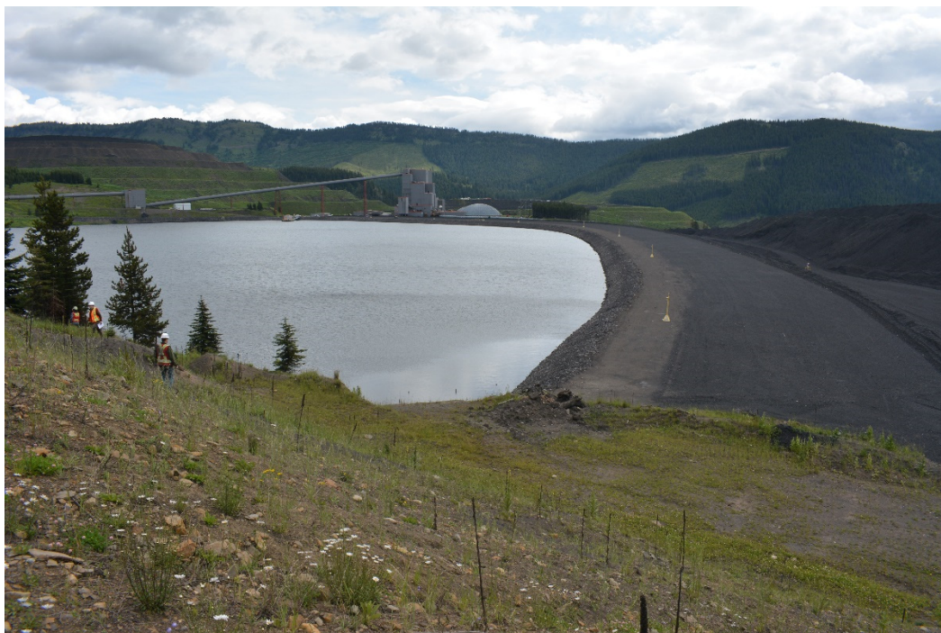
Photograph 8: Main Tailings Dam – Crest and West Abutment; looking East, 17 July 2019
