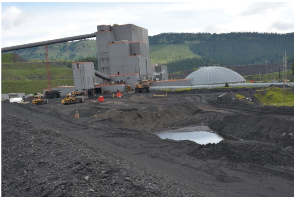
Photograph 9: Main Tailings Dam – East Abutment, Poned Surface Water; looking Northeast, 17 July 2019
