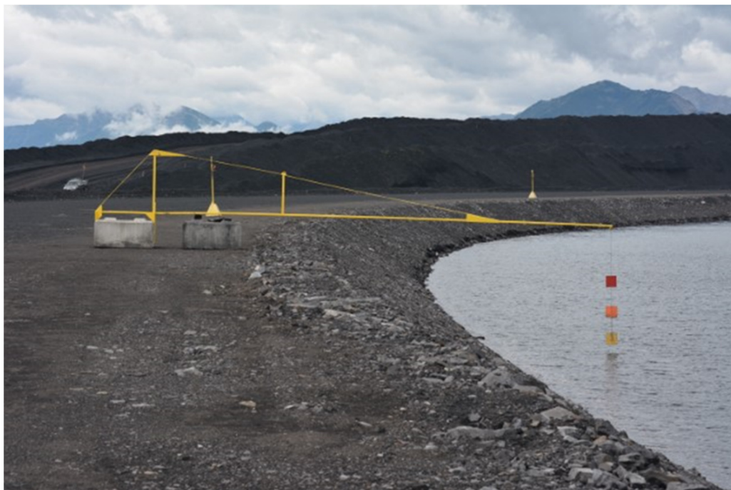
Photograph 5: Main Tailings Dam –Freeboard Indicator; looking Southwest, 17 July 2019
