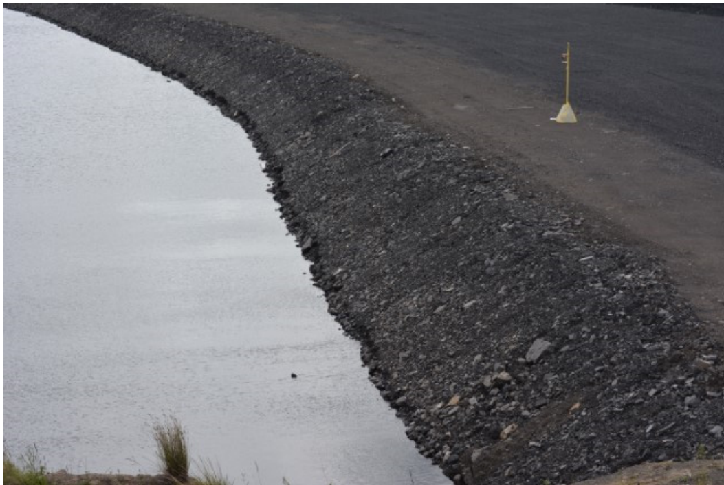
Photograph 7: Main Tailings Dam – Upstream Slope and Crest; looking Southeast, 17 July 2019
