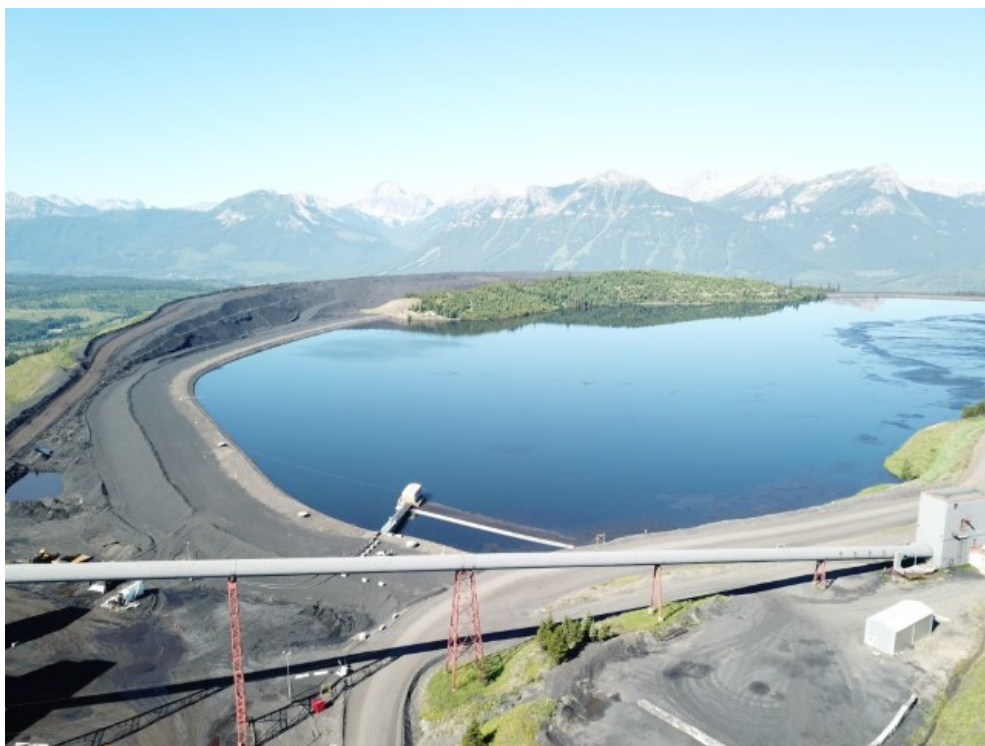
Photograph 2: Main Tailings Dam – looking West, 26 September 2019
