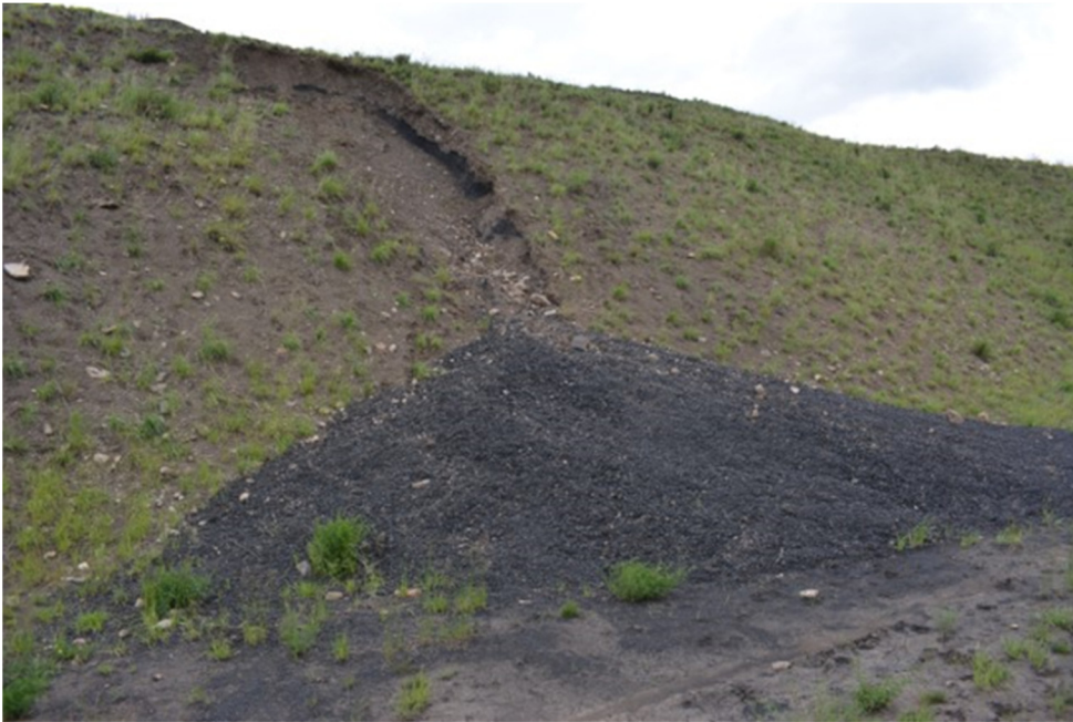
Photograph 17: Site C Coarse Coal Refuse Spoil – Slump First Observed 18 April 2019; 17 July 2019
