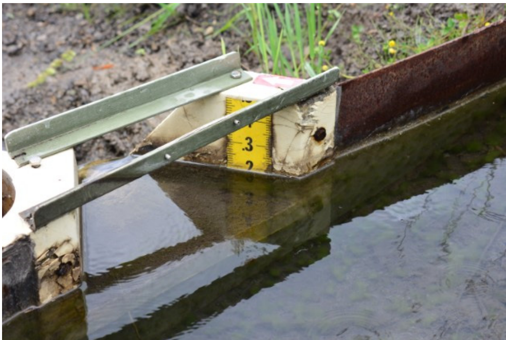
Photograph 24: West Tailings Seepage Weir - Measurement Gauge; 17 July 2019
