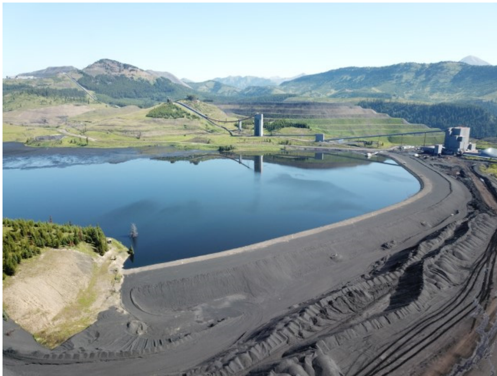
Photograph 1: Main Tailings Dam – looking Northeast, 26 September 2019
