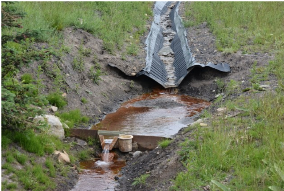
Photograph 15: Site C Seepage Weir - looking Northeast, 17 July 2019
