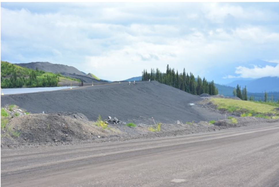
Photograph 20: West Tailings Dam – Downstream Slope and Toe Area; looking Southeast, 17 July 2019
