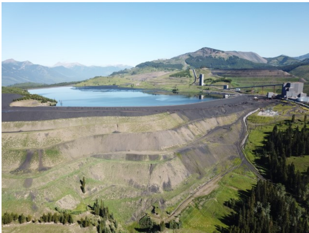
Photograph 13: Site C Coarse Coal Refuse Spoil and Main Dam – looking North, 26 September 2019
