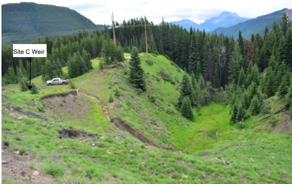
Photograph 14: Site C Weir and Downstream Creek; looking South, 17 July 2019
