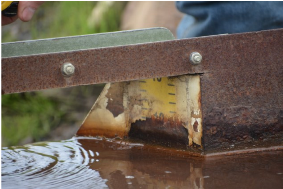
Photograph 16: Site C Seepage Weir – Measurement Gauge; looking West, 17 July 2019
