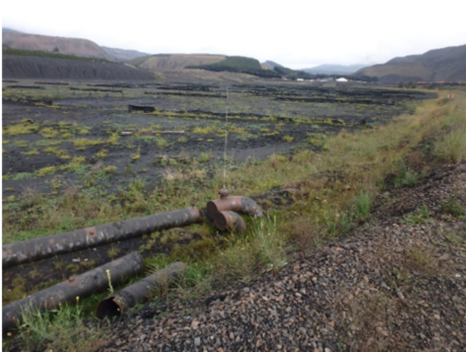
Photograph A-35: On NTP Upstream Slope, Unused Reclaim Pipelines (capped pipeline that go into dam section and cross under dam crest), looking North, 11 September 2019
