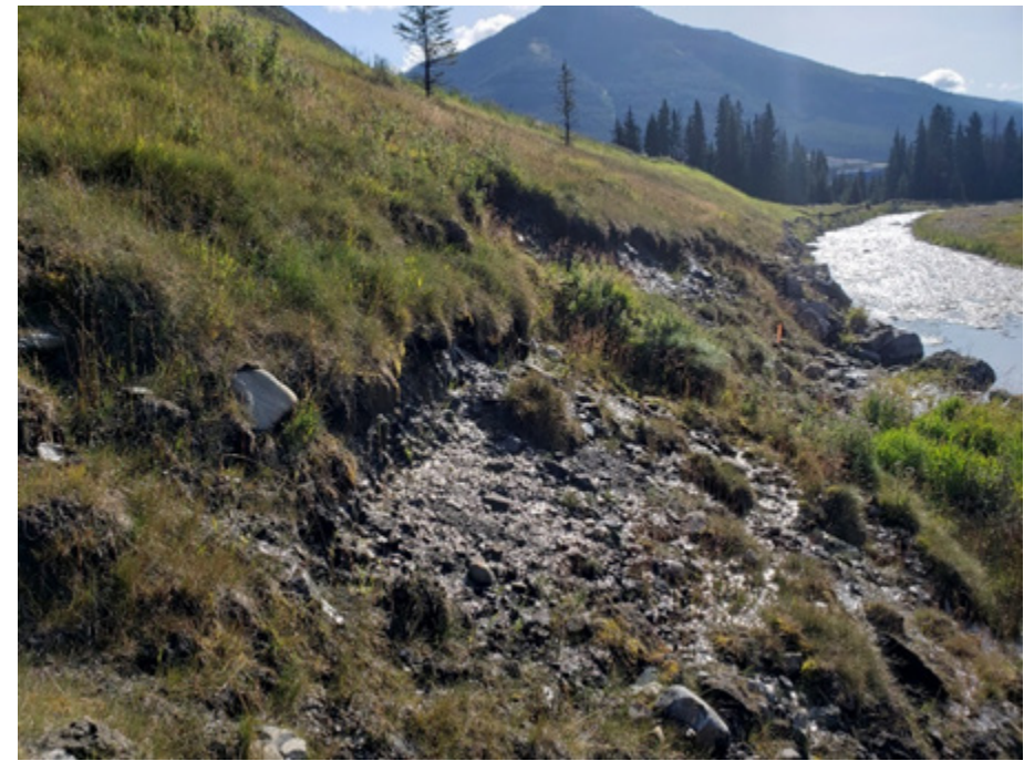
Photograph A-9: STP West Dam, looking South at the Toe of the Cut Slope Above Fording River Diversion, Seepage was Observed to be Coming out of the Slope Adjacent to the West Seepage Pipes, 10 September 2019
