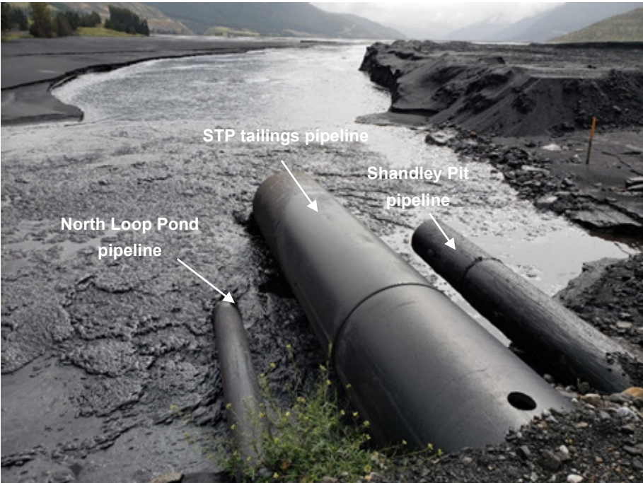
Photograph A-3: STP, North single point discharge, make up water pipelines, and channel to main pond, looking South, 10 September 2019
