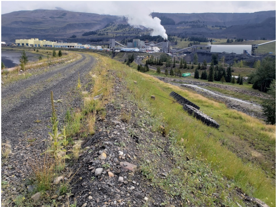
Photograph A-35: On NTP Upstream Slope, Unused Reclaim Pipelines (capped pipeline that go into dam section and cross under dam crest), looking North, 11 September 2019
