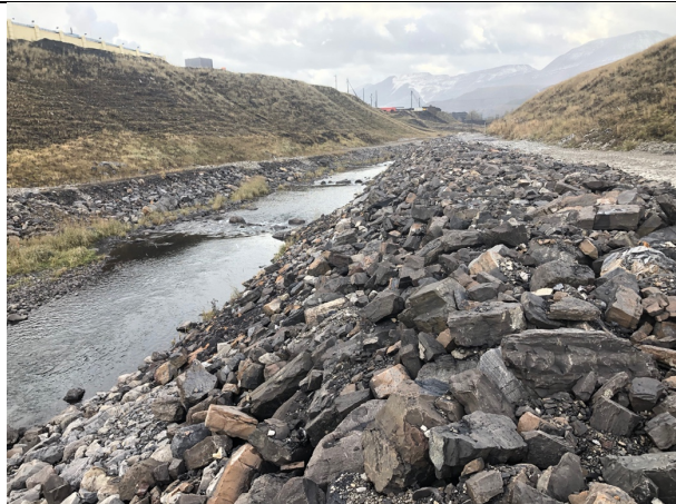
Photo 3: Looking downstream at NTP riprap (approx. Sta. 0+450)
