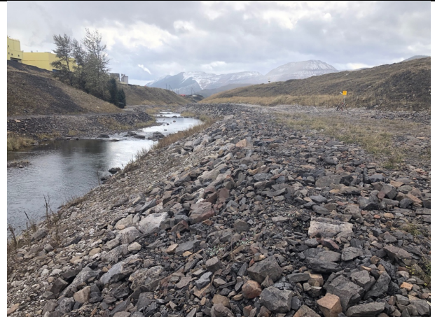
Photo 2: Looking downstream at NTP riprap covered by gravel (approx. Sta. 0+180)
