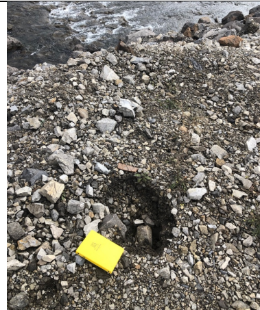
Photo 4: Small sinkhole about 1.5 m from top of bank on running surface of riprap along the NTP riprap (approx. Sta. 0+710)
