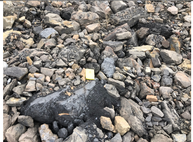
Photo 6: Riprap degradation due to weathering on a surface of a piece of riprap (approx. Sta. 0+900)
