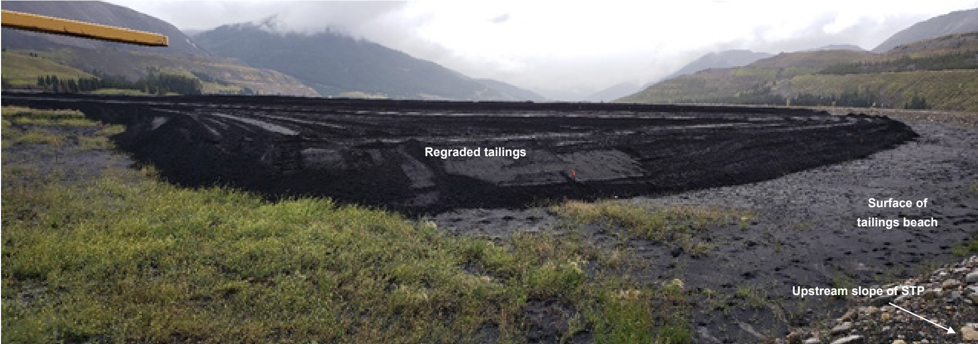
Photograph A-6: STP West Dam near Station 0+000, Regraded tailings to 0.2 m below STP dam crest and minimum 10 m Wide Channel was Maintained between Regarded Tailings and Upstream Slope of Dam during Tailings Regrading Work, looking South, 10 September 2019
