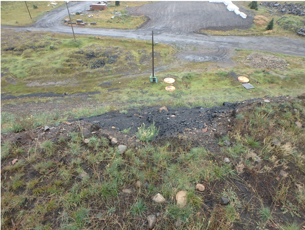
Photograph A-13: STP Main Dam, Looking Southeast At Erosion Channel Along Downstream Slope At Station 1+450, 10 September 2019
