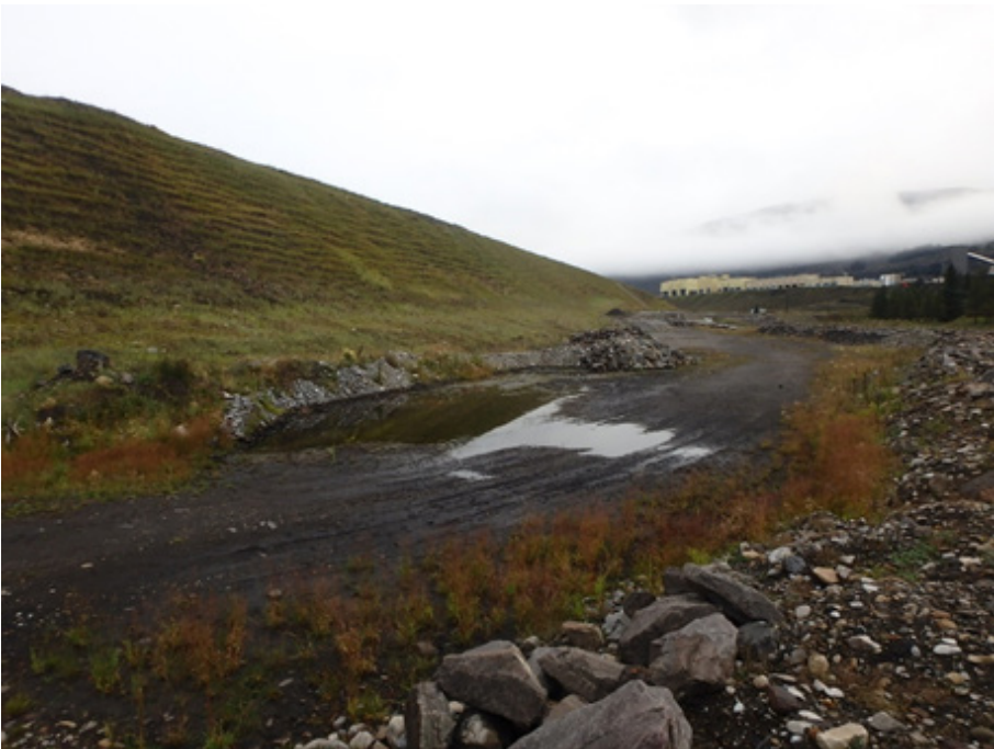
Photograph A-32: NTP Dam Downstream Slope and Toe and Stepped Erosion and Area of Ponding Water, at Station 1+200, 11 September 2019
