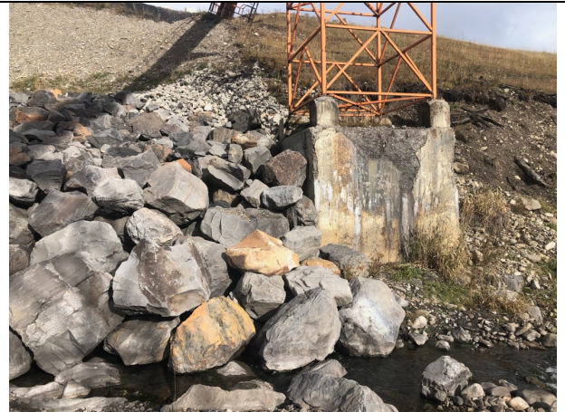
Photo 12: STP riprap tie-in to pipe bridge abutment (approx. Sta. 0+685)
