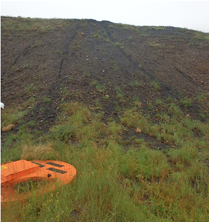
Photograph A-14: STP Main Dam, Looking Up At Downstream Slope From Dam Toe At Erosion Gullies From Photo A-13, 10 September 2019
