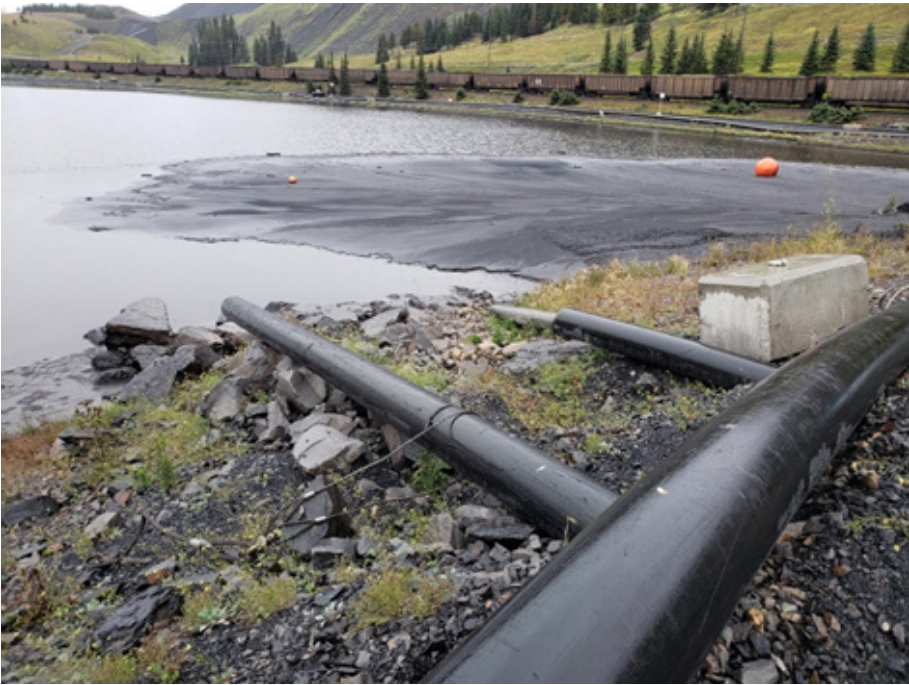
Photograph A-21: STP South Abutment Till Blanket Area, Makeup Water Pipelines from Kilmarnock Ponds with Rip Rap Protection on Blanket, Looking Northeast, 10 September 2019
