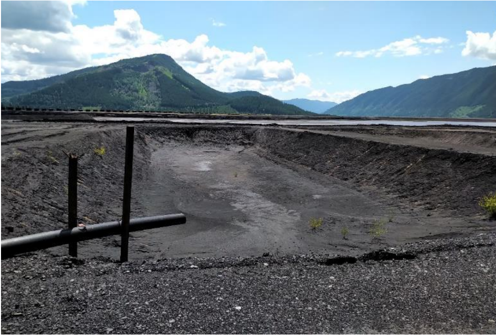
Photo ID-11 Typical internal cell on crest. (looking south)
