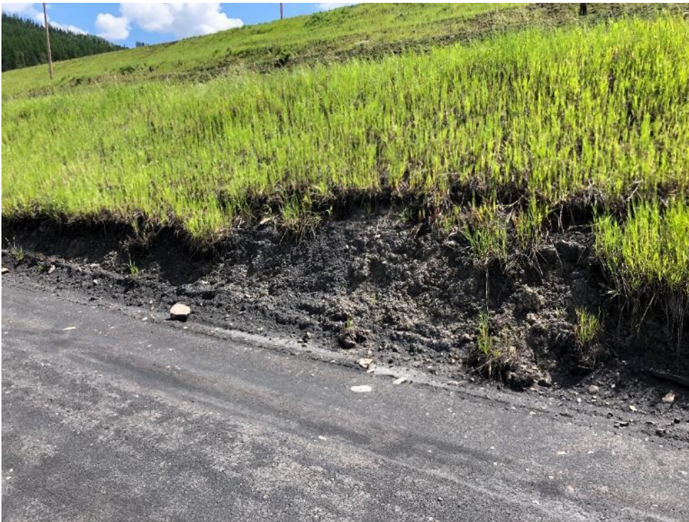
Photo ID-10 Minor bench erosion. (looking south)
