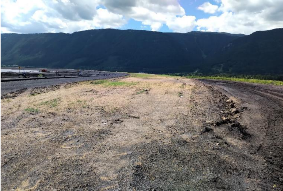
Photo ID-5 Typical crest conditions. (looking west)
