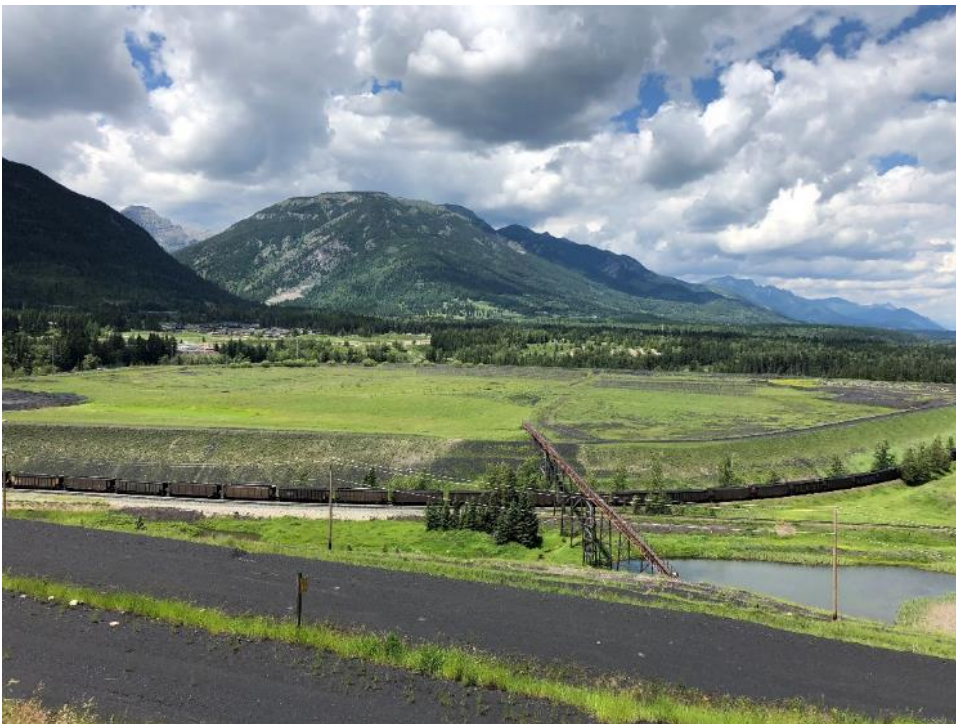
Photo ID-16 Transfer pipeline from Lagoon D to Lagoon C. (looking north)
