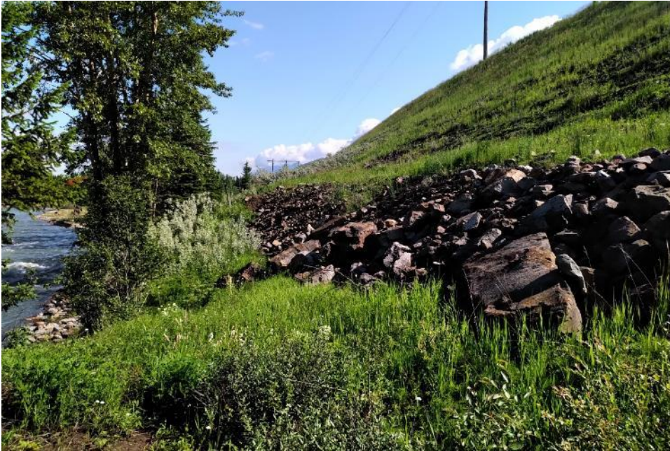
Photo IC-11 Riprap on at the toe of Lagoon C, adjacent to the Elk River. (looking North)
