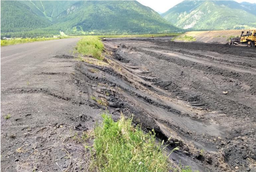
Photo ID-9 Upstream crest erosion 2. (looking west)
