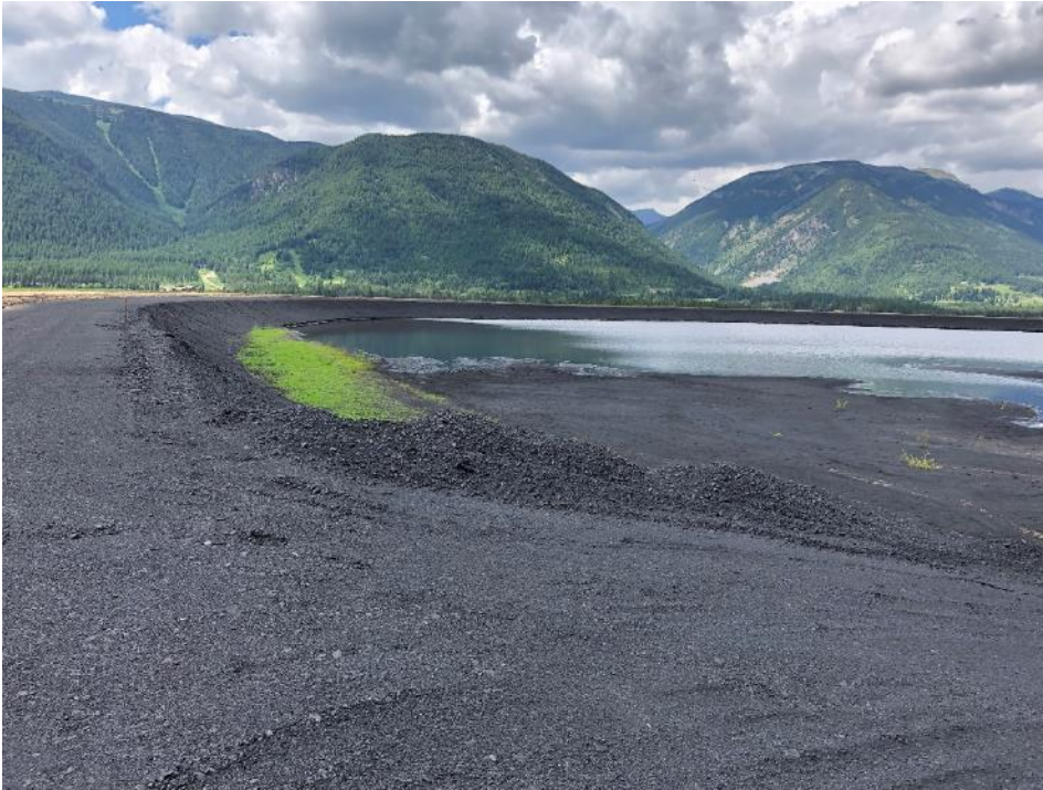
Photo ID-17 Decant Pond and upstream slope conditions. (looking west)
