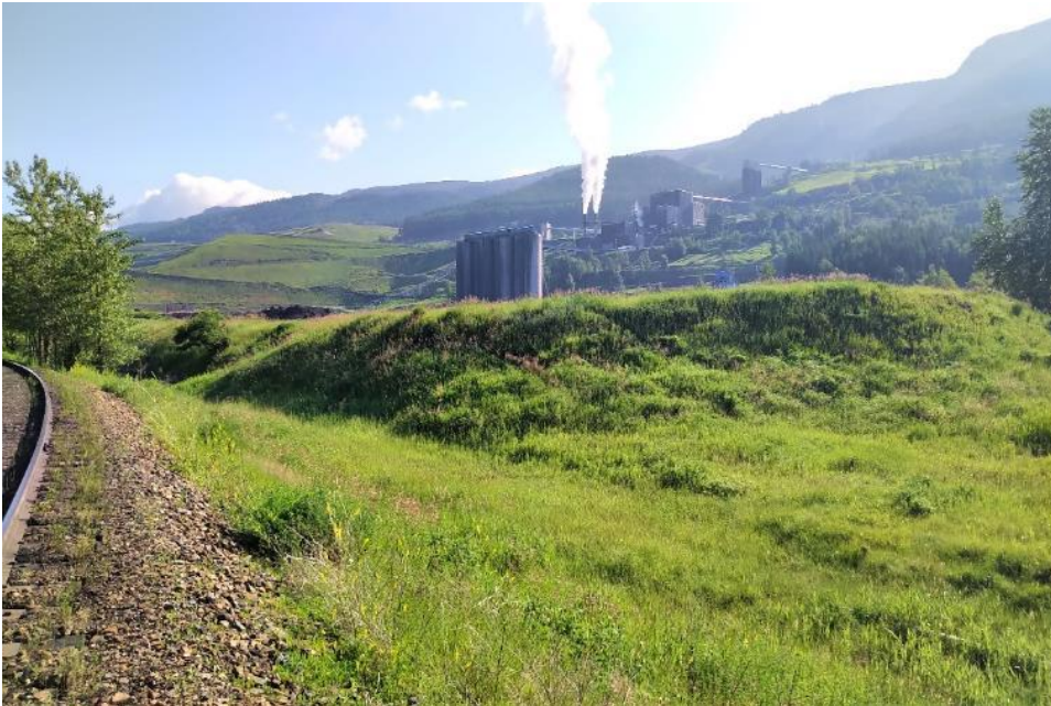
Photo IB-4 Minor slumping of Lagoon B. (looking northeast)
