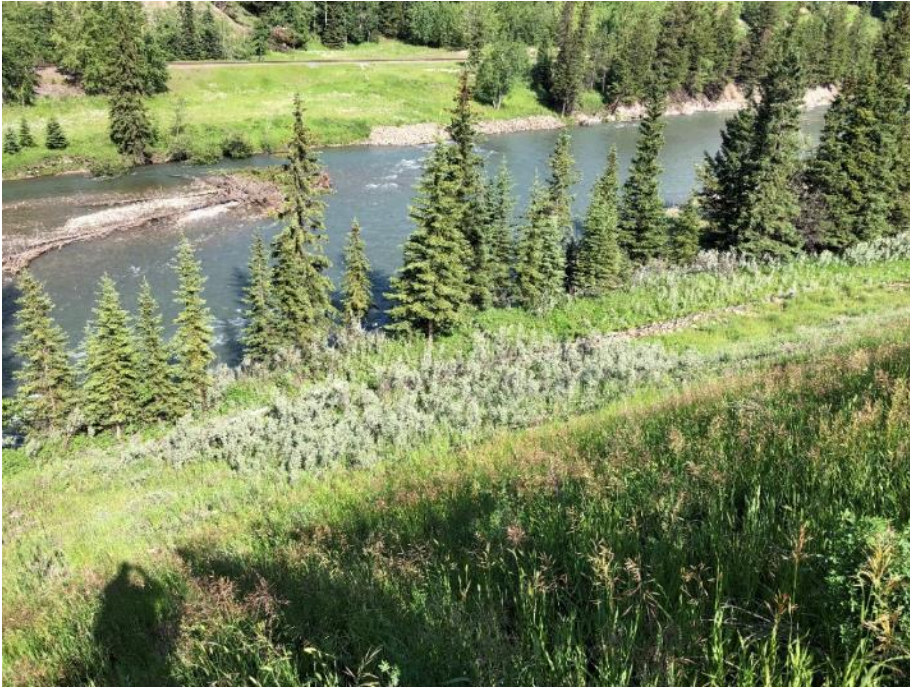
Photo IC-7 Changes in vegetation potentially indicating seepage or wet spots. (looking west)
