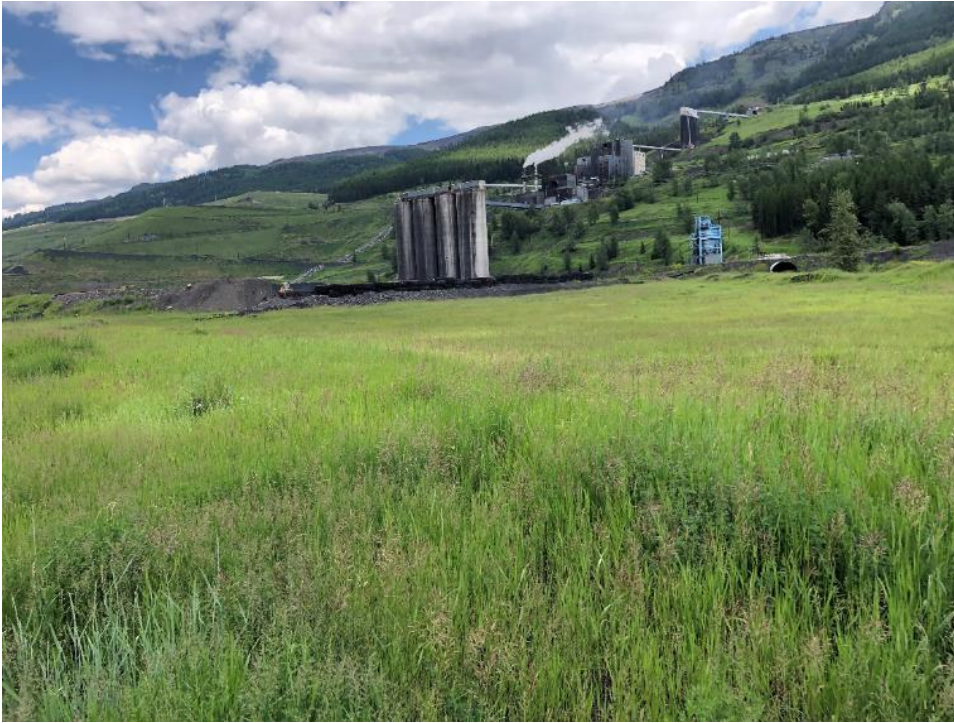
Photo IB-3 Typical surface conditions. (looking northeast)
