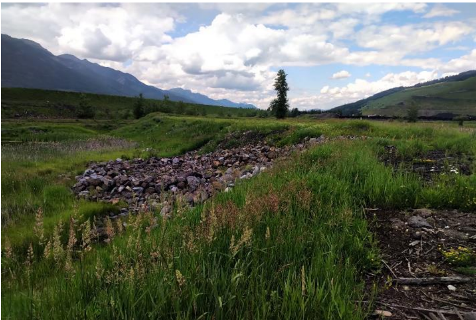
Photo IA-4 Rockfill armoured spillway. (looking north)
