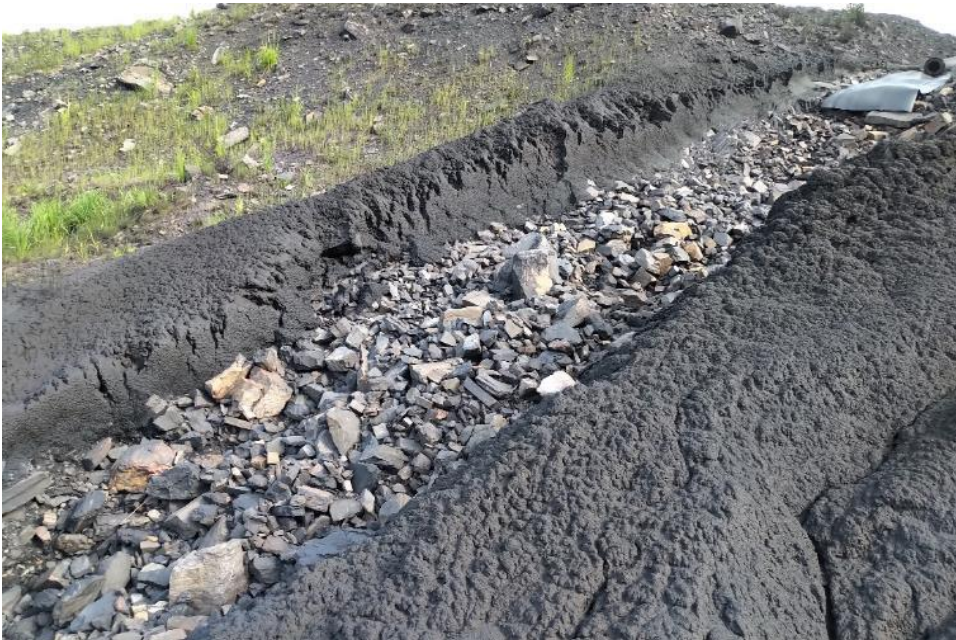
Photo IW-6 Upstream slope erosion protection at spigot 2. (looking south)
