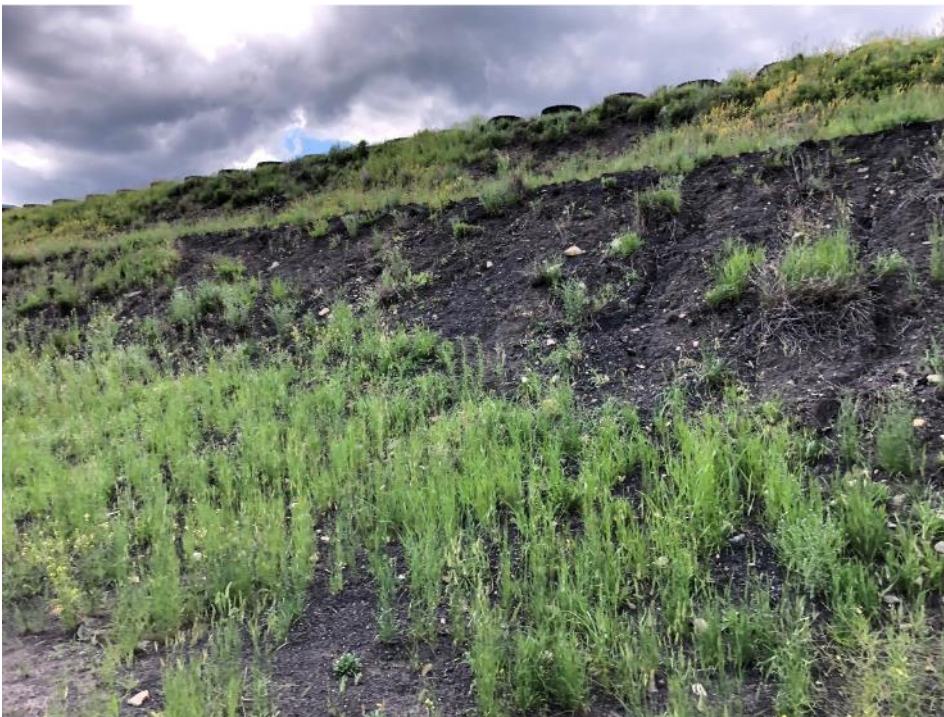
Photo ID-18 Downstream erosion and sparse vegetation. (looking west)
