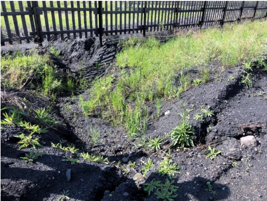
Photo IC-8 Erosion on the upstream side near the pumphouse. (looking south)
