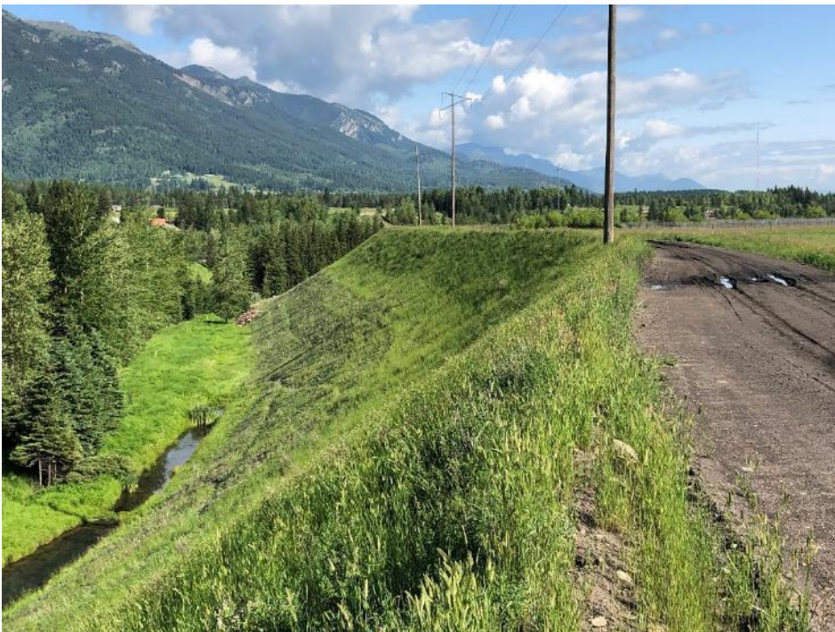
Photo IC-4 Typical downstream slope condition. (looking north)
