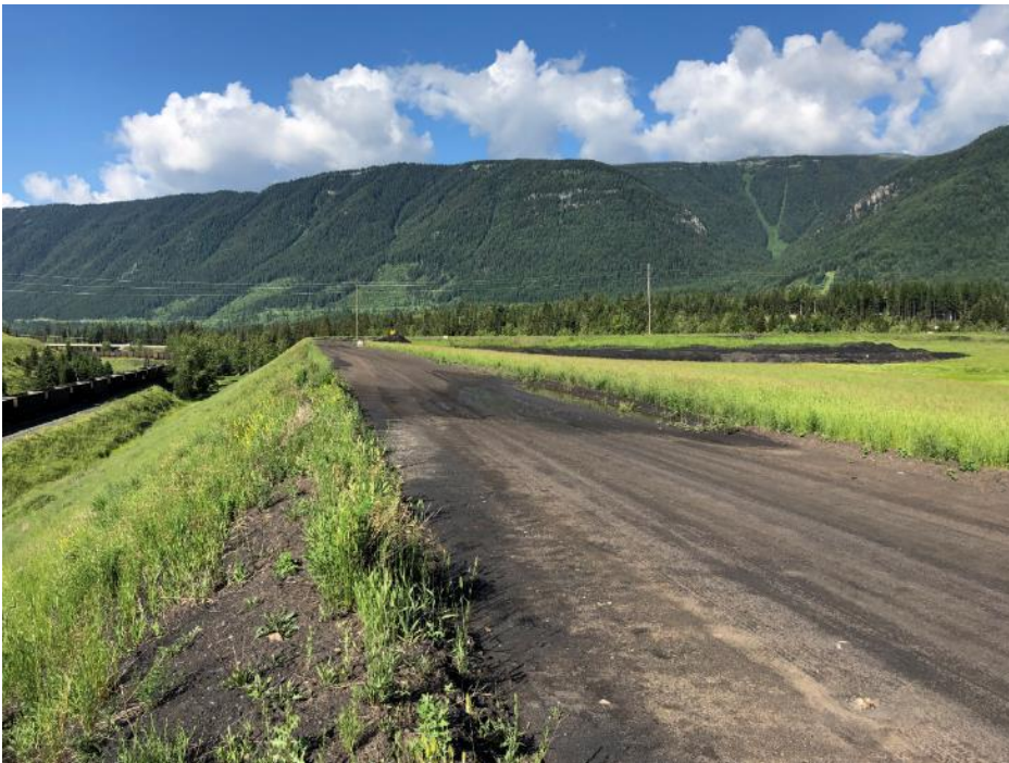
Photo IC-6 Local low spot on crest. (looking east)
