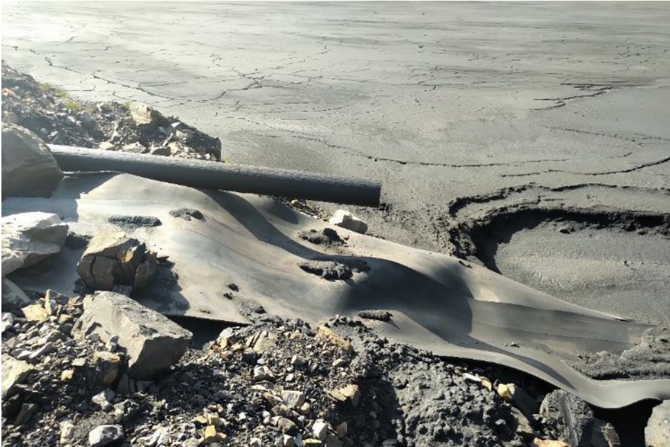
Photo IW-5 Upstream slope erosion protection at spigot 1. (looking northwest)
