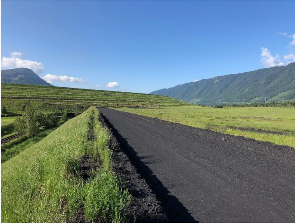
Photo IC-3 Typical crest and surface conditions. (looking southwest)
