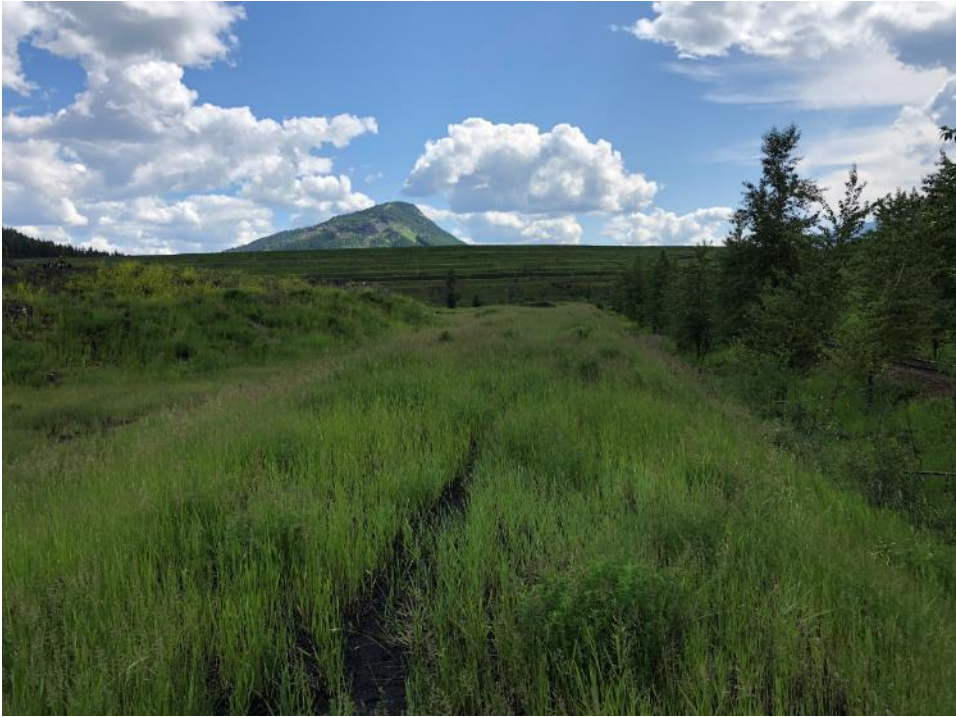
Photo IB-5 Typical downstream slope condition. (looking southwest)
