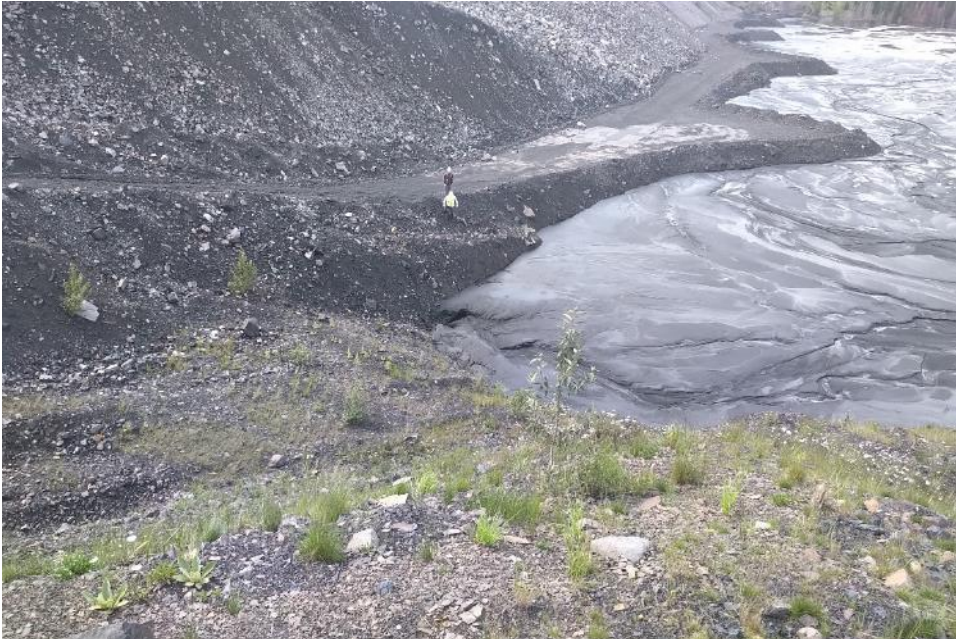
Photo IW-3 Adit Toe Berm and tailings infiltration into west abutment. (looking north)
