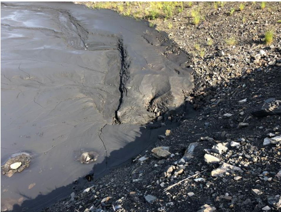
Photo IW-4 Tailings infiltration into east abutment. (looking north)
