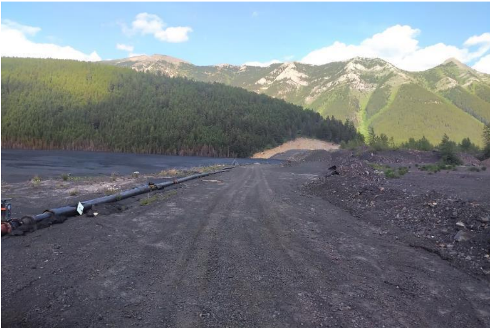
Photo IW-8 Crest typical conditions 2. (looking east)
