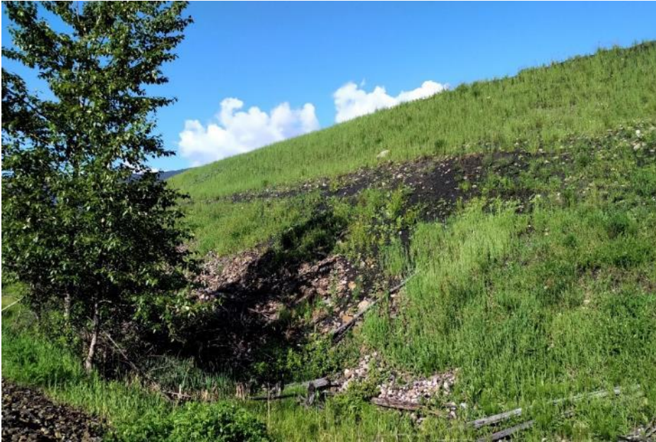
Photo IC-5 Local erosion and sparse vegetation. (looking southwest)
