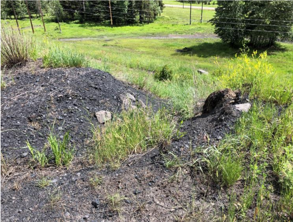
Photo ID-19 Minor gully erosion on the southern portion of the lagoon. (looking south)
