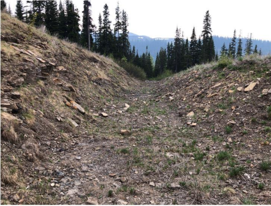
Photo II-24 BTD Spillway Outlet. Riprap D_{50} of approximately 300 mm – looking downstream (BTD-2019-17)
