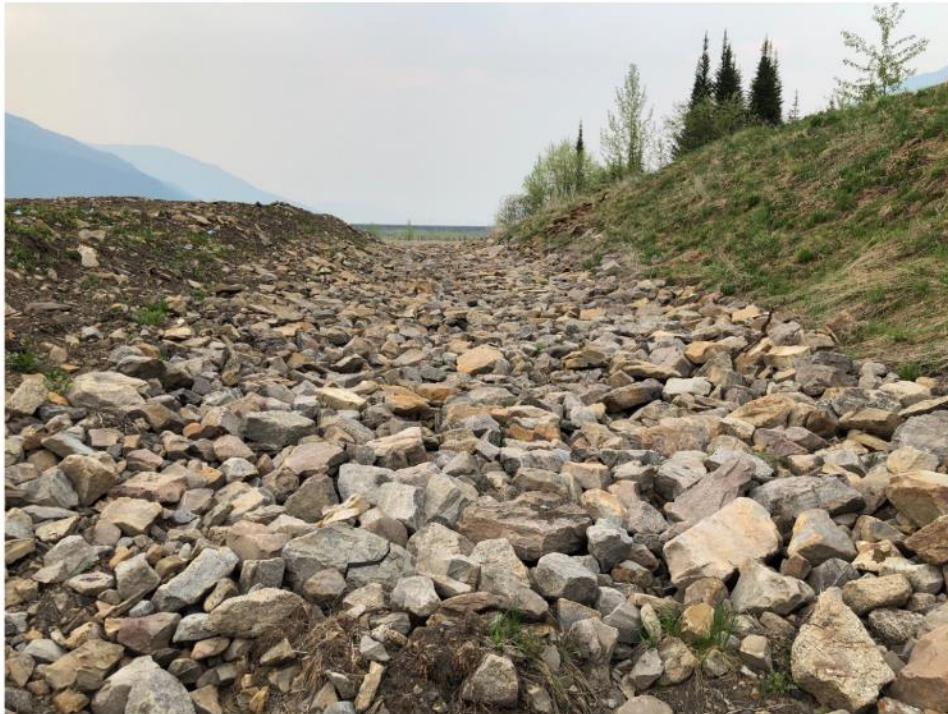
Photo II-21 BTD Spillway. Riprap armoured portion of the spillway – looking upstream (BTD-2019-16)
