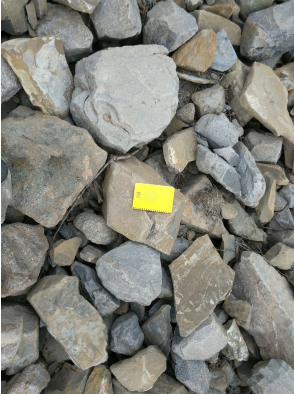
Photo II-22 BTD Spillway Riprap. D 50 of approximately 300 mm – looking upstream (BTD-2019-16)
