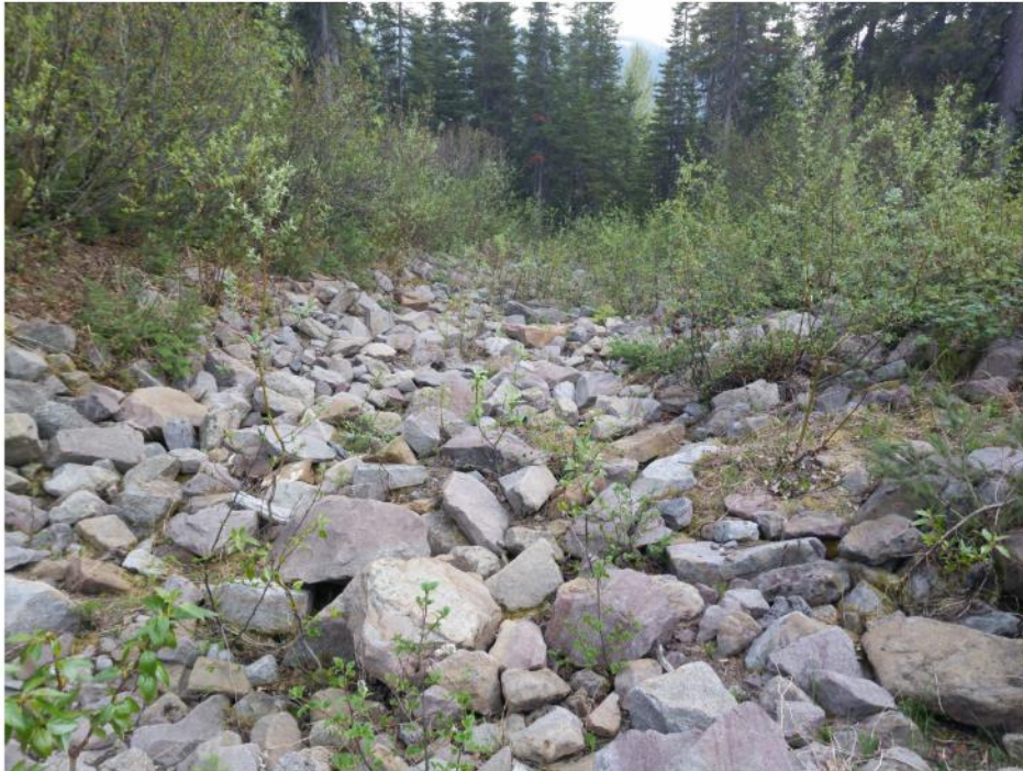
Photo II-24 BTD Spillway Outlet. Riprap D_{50} of approximately 300 mm – looking downstream (BTD-2019-17)
