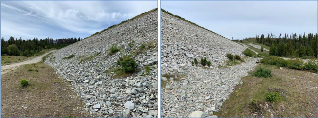
Photo II-B-6 Pile of sand (not tailings) on upper part of starter dam slope. Appears to have been dumped there rather than resulting from seepage. Well above water level and no sign of flow in the area (BTH-2019-09)
