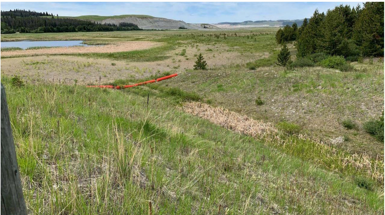
Photo II-B-11 Spillway inlet and approach channel. Vegetation to be cleared from flow channel as part of routine maintenance including approach channel and initial segment of riprap channel (BTH-2019-11)
