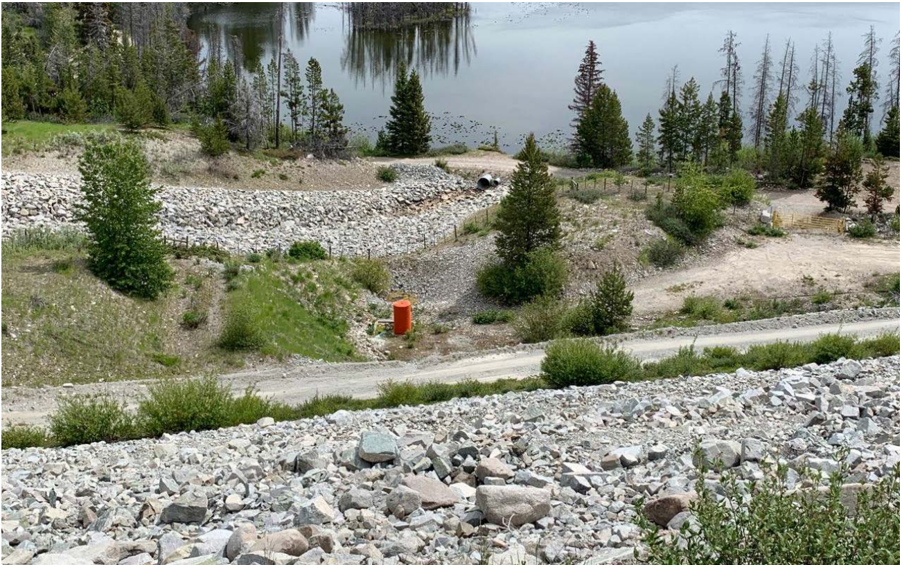
Photo II-B-18 Spillway road culverts – not significantly obstructed (BTH-2019-14)
