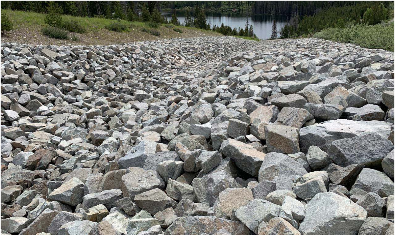
Photo II-B-15 Spillway channel, looking southeast (downstream) towards Bose Lake (BTH-2019-12)
