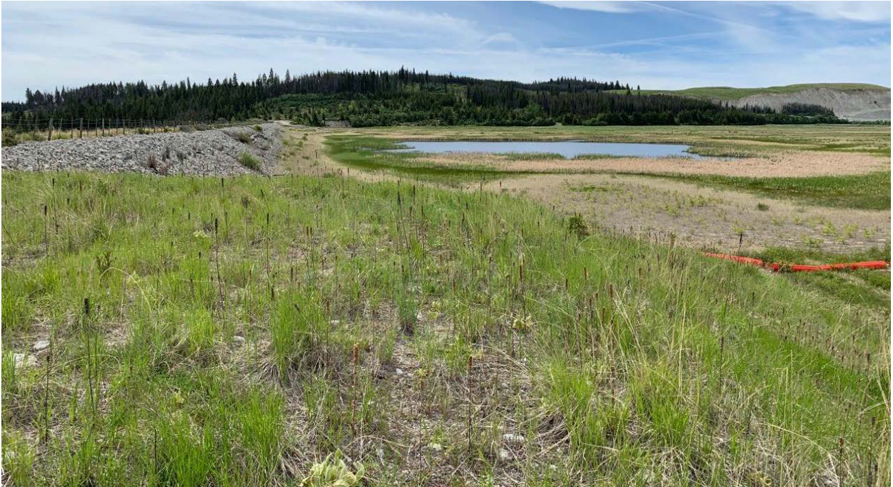
Photo II-B-11 Spillway inlet and approach channel. Vegetation to be cleared from flow channel as part of routine maintenance including approach channel and initial segment of riprap channel (BTH-2019-11)
