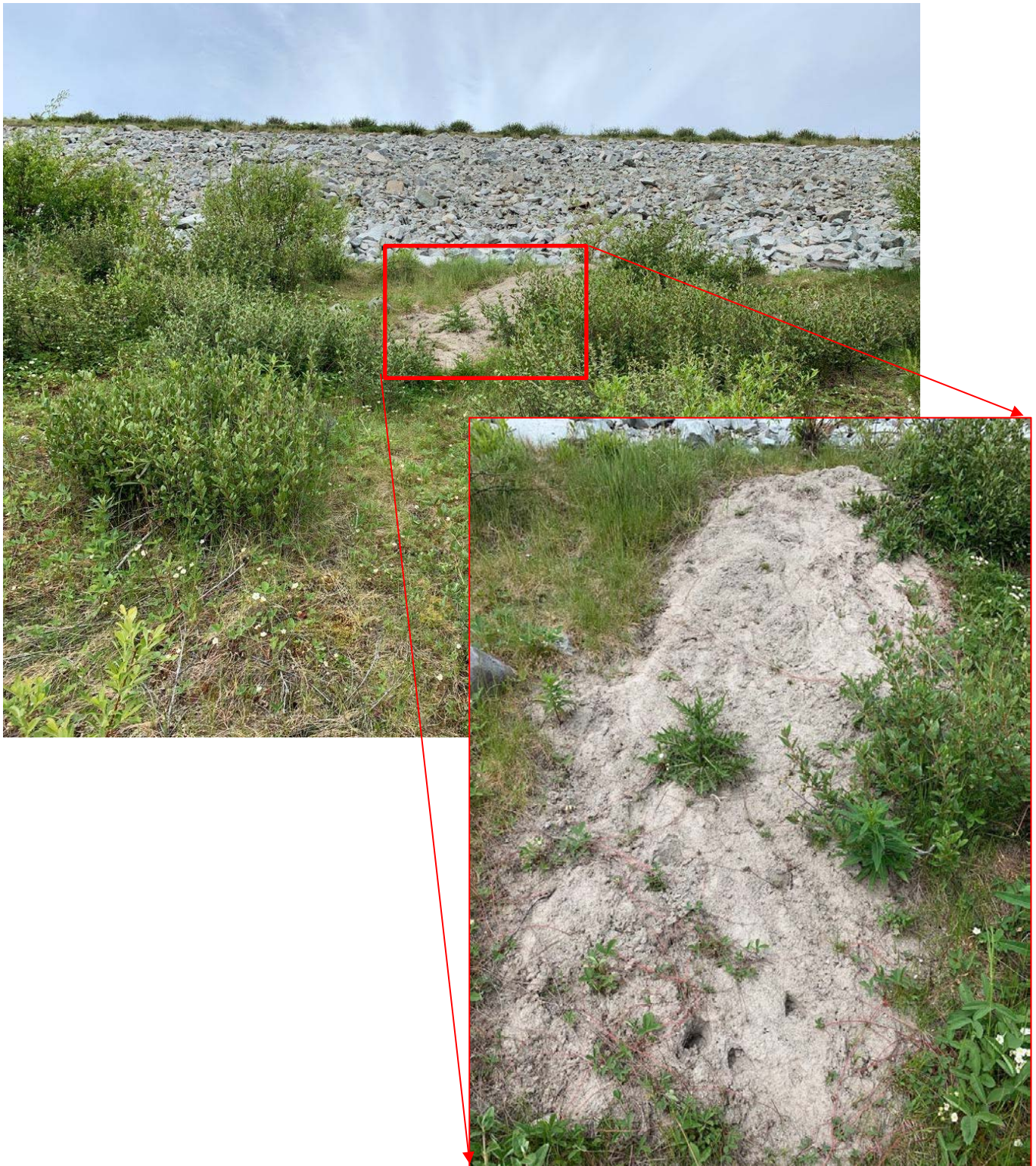
Photo II-B-7 Sand pile similar to the one observed in Photo II-B-6 and at a similar elevation (BTH-2019-10)
