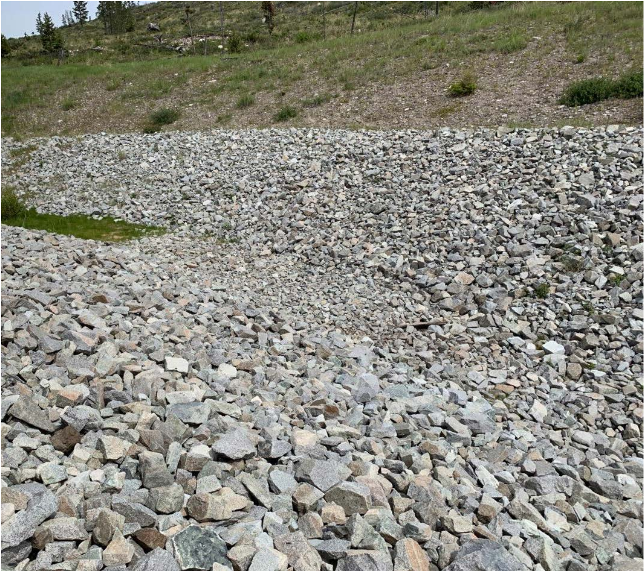
Photo II-B-14 Overview of spillway channel – No vegetation around spillway bend. Riprap not degrading (BTH-2019-12)
