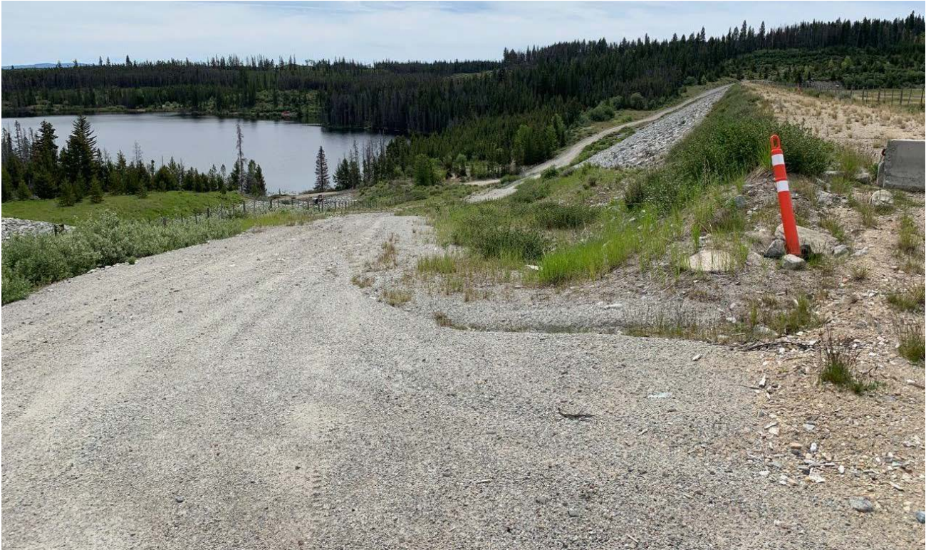
Photo II-B-2 Overview of downstream toe from left abutment (BTH-2019-06)
