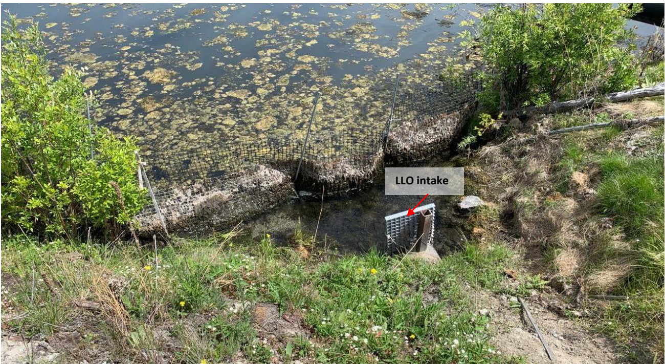
Photo II-C-4 Pond and trash rack for Low-Level Outlet (LLO) (BTH-2019-18)
