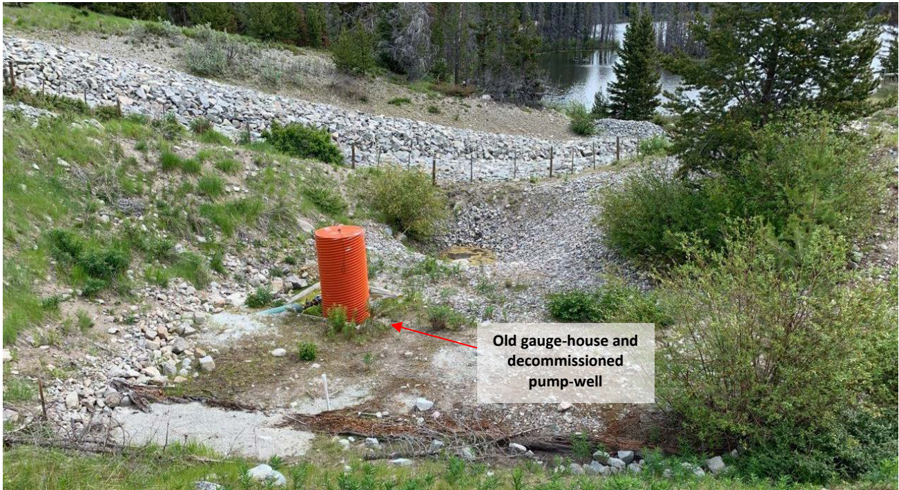
Photo II-B-16 Overview spillway channel (BTH-2019-13)
