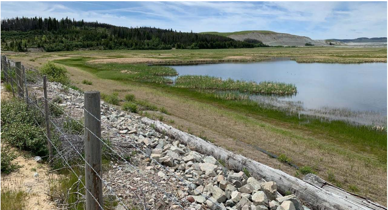
Photo II-B-9 Upstream riprap, tailings beach and Pond No. 2, looking towards right abutment (BTH-2019-05)
