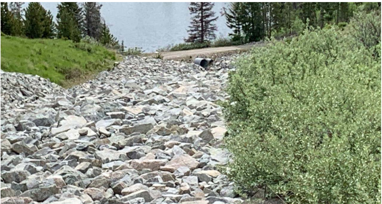
Photo II-B-18 Spillway road culverts – not significantly obstructed (BTH-2019-14)
