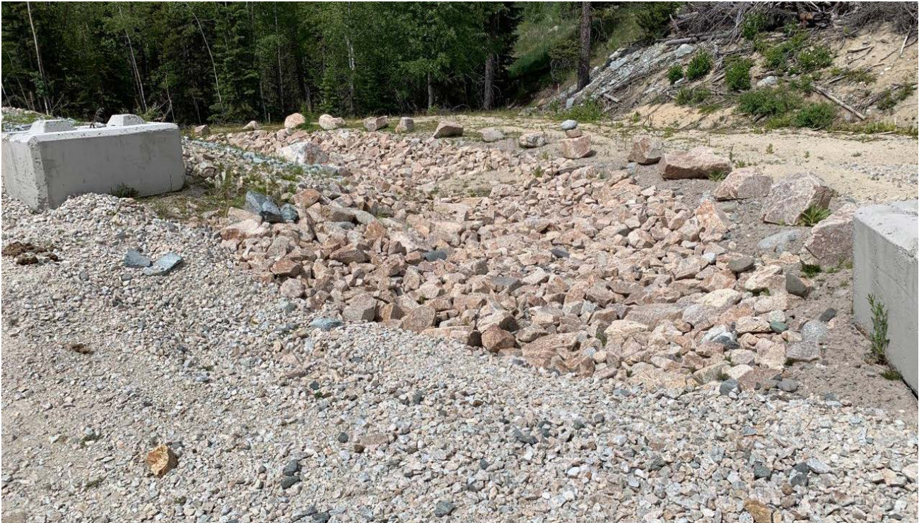
Photo II-C-4 Pond and trash rack for Low-Level Outlet (LLO) (BTH-2019-18)
