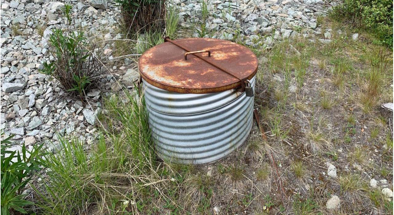
Photo II-B-19 Seepage relief well at downstream toe, looking west (upstream) – Well was locked but low flow inside could be heard (BTH-2019-15)
