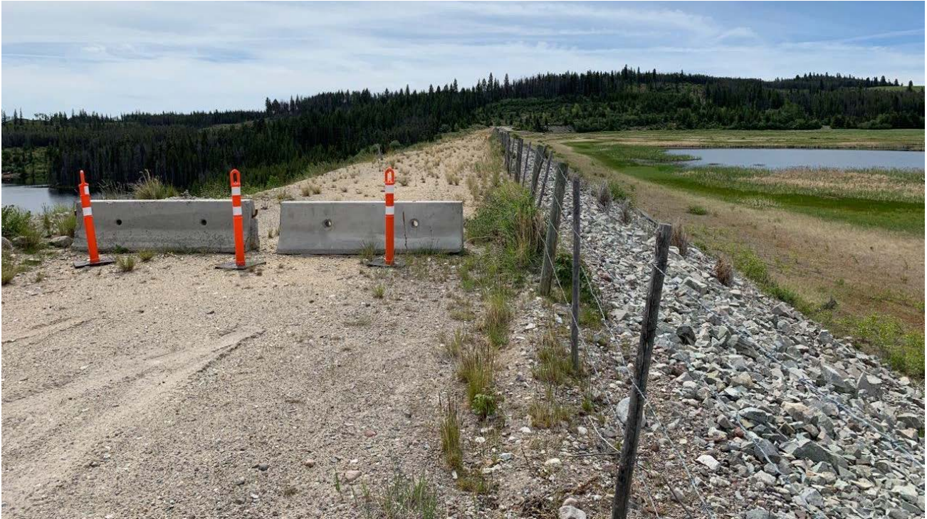
Photo II-B-9 Upstream riprap, tailings beach and Pond No. 2, looking towards right abutment (BTH-2019-05)
