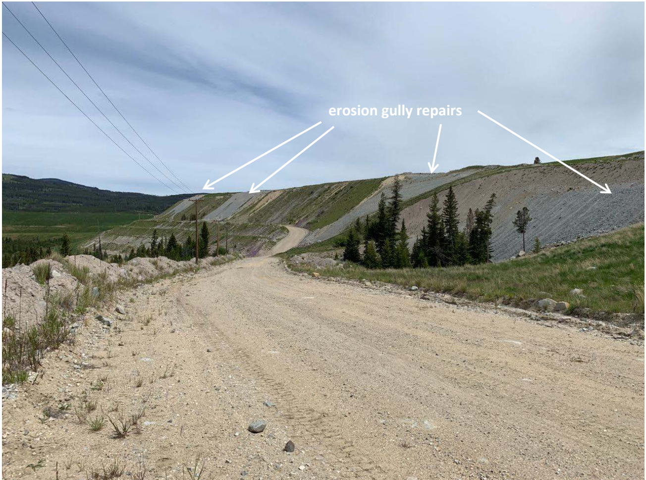
Photo II-A-5 Overview of downstream slope and toe from left abutment (BTH-2019-04)
