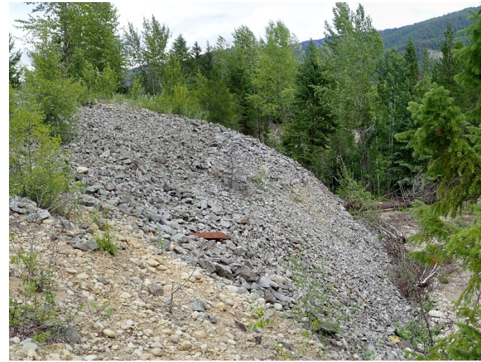
Photograph 10: South TSF, Cell 4, downstream slope, looking northeast. 10 July 2019.
