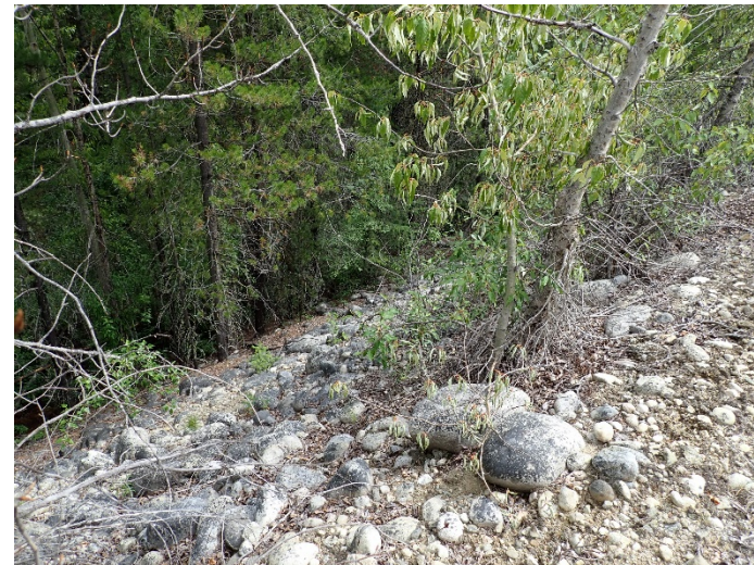
Photograph 32: North TSF, Cell 7, downstream slope of south embankment, looking southwest. 10 July 2019.
