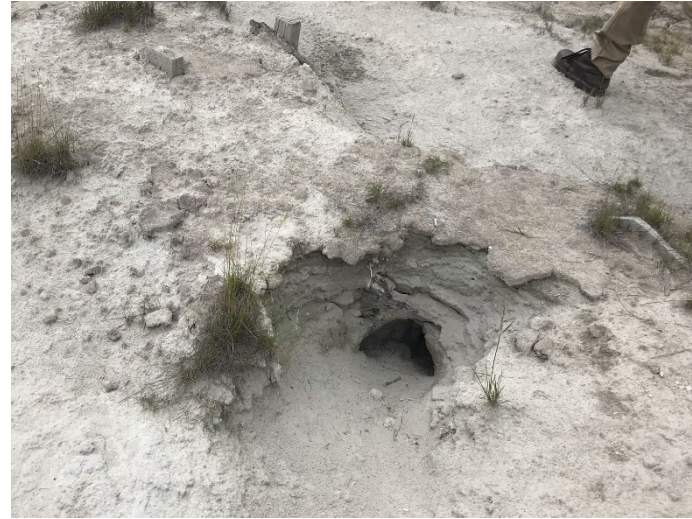
Photograph 38: North TSF, Cell 7, animal burrow in tailings surface, looking east. 10 July 2019.
