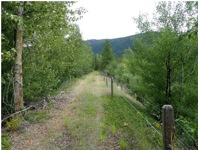
Photograph 31: North TSF, Cell 7, crest of south embankment, looking east. 10 July 2019.
