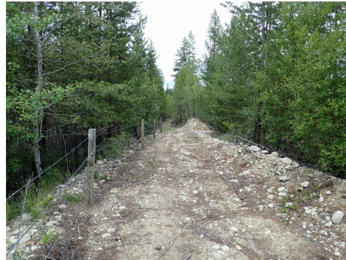
Photograph 2: South TSF, Cell 1, crest of west embankment looking northeast. 10 July 2019.
