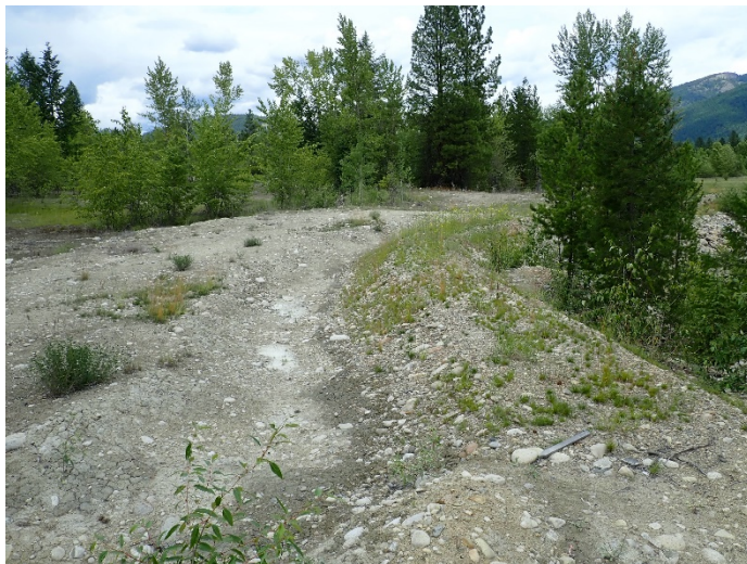
Photograph 3: South TSF, Cell 1, crest and upstream ditch at southeast embankment, looking northeast. 10 July 2019.
