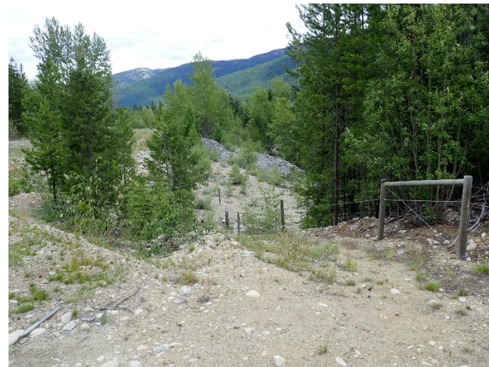
Photograph 4: South TSF, Cell 1, southeast embankment, looking northeast. 10 July 2019.
