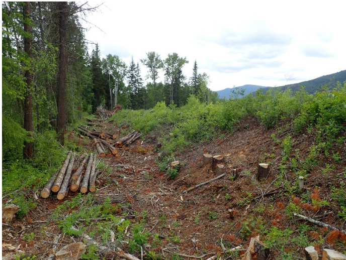
Photograph 23: South TSF, Cell 3, felled trees on crest and downstream slope, looking south. 10 July 2019.
