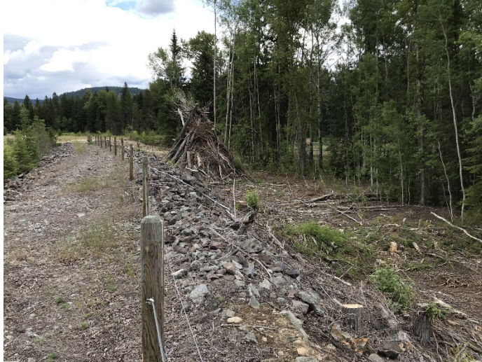
Photograph 21: South TSF, Cell 3, crest and downstream slope with felled trees, looking northeast. 10 July 2019.
