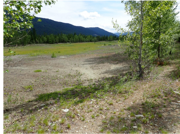
Photograph 30: North TSF, Cell 6, tailings surface from division between Cell 6 (left) and Cell 7 (right), looking southeast. 10 July 2019.
