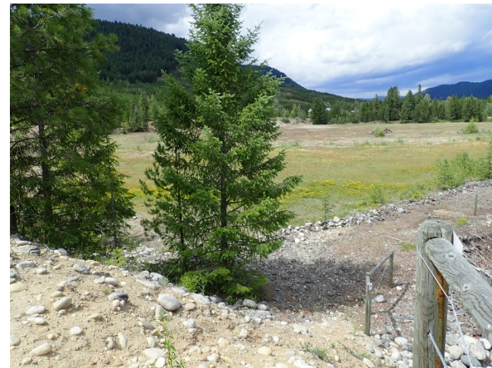
Photograph 16: South TSF, Cell 3, tailings surface and embankment crest, looking northwest. 10 July 2019.
