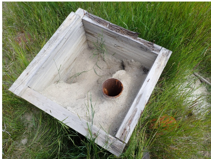
Photograph 11: South TSF, Cell 5, backfilled decant tower, 10 July 2019.
