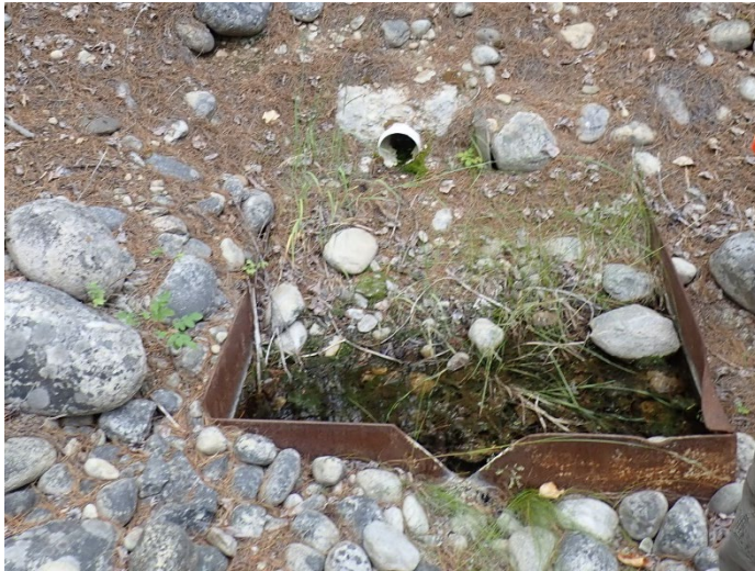
Photograph 29: North TSF, Cell 6, decant outlet at toe of south embankment, looking north. 10 July 2019.
