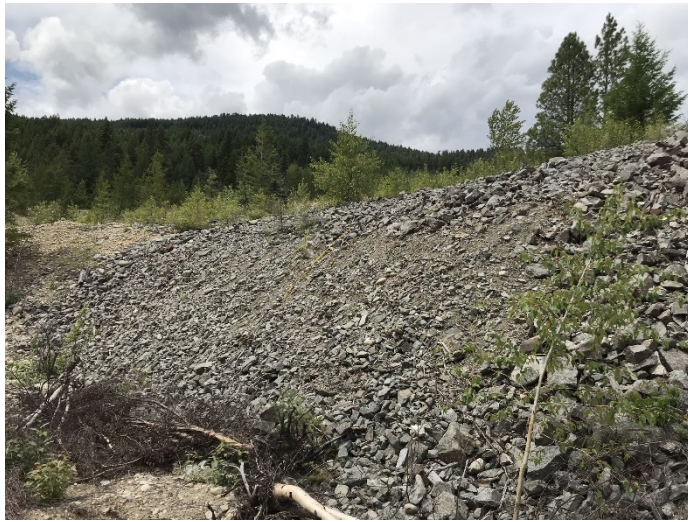
Photograph 5: South TSF, Cell 1/5, downstream slope waste rock, looking west. 10 July 2019.
