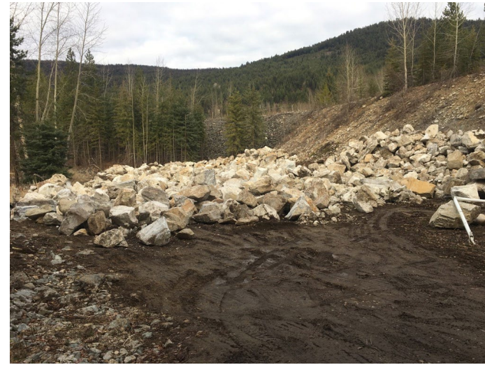
Photograph 42: Riprap stockpile at the toe of Cells 4 and 5, looking southwest. 12 April 2019.
