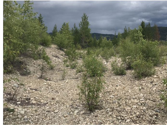
Photograph 34: North TSF, Cell 7, spillway at southwest corner, looking north. 10 July 2019.
