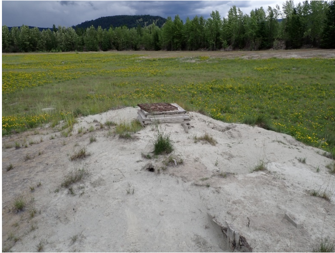
Photograph 37: North TSF, Cell 7, tailings surface and decant tower, looking east. 10 July 2019.
