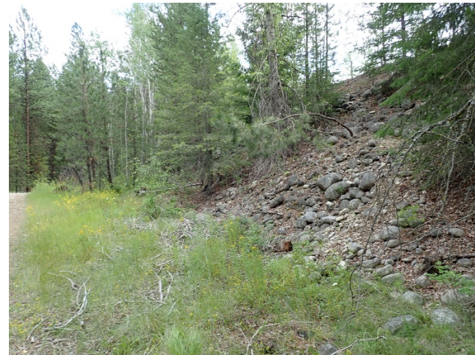
Photograph 28: North TSF, Cell 6, east embankment downstream slope, looking south. 10 July 2019.
