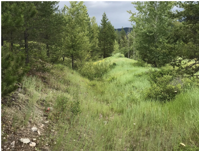
Photograph 39: North TSF, Cell 7, diversion channel reach 1, west of TSF, looking north. 10 July 2019.
