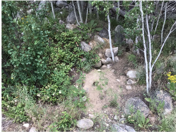
Photograph 33: North TSF, Cell 7, animal burrow in downstream slope of south embankment, looking north. 10 July 2019.
