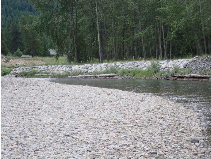
Photograph 41: Armouring of neighbouring land on left bank of West Kettle River, looking southeast. 10 July 2019.
