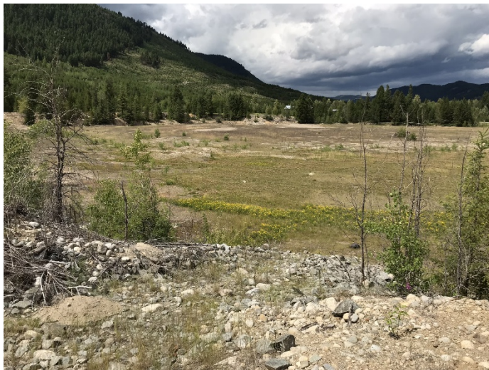
Photograph 15: South TSF, spillway between Cell 4 and Cell 3, looking northwest. 10 July 2019.
