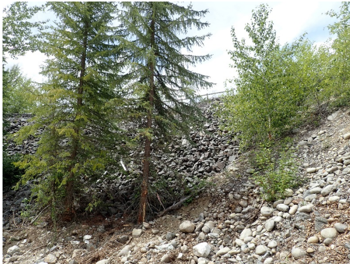
Photograph 13: South TSF, Cell 4, downstream slope, looking northwest. 10 July 2019.
