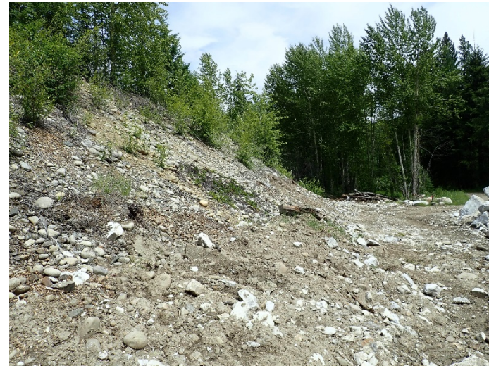
Photograph 14: South TSF, Cell 4, downstream slope, looking northeast. 10 July 2019.
