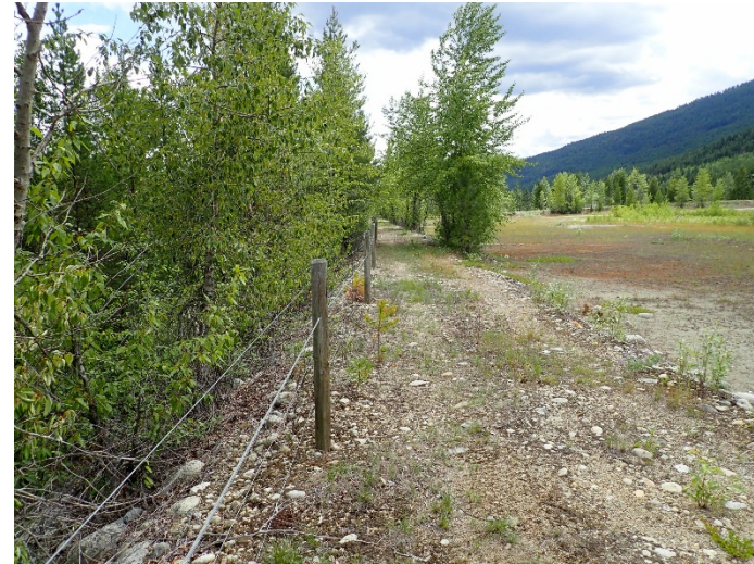
Photograph 26: North TSF, Cell 6, east embankment crest, looking southwest. 10 July 2019.
