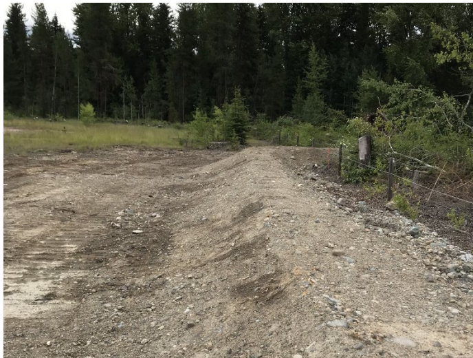
Photograph 19: South TSF, Cell 3, crest and berm, looking northeast. 10 July 2019.
