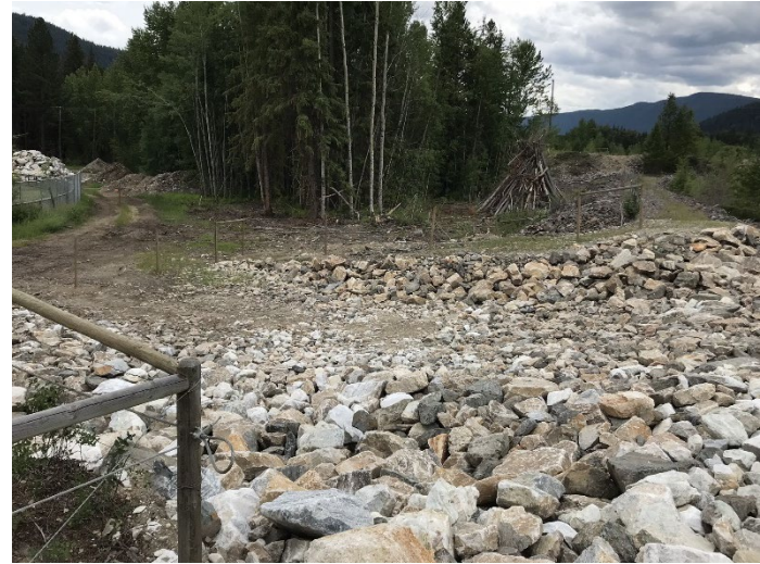
Photograph 18: South TSF, Cell 3, remediated spillway downstream, looking southeast. 10 July 2019.
