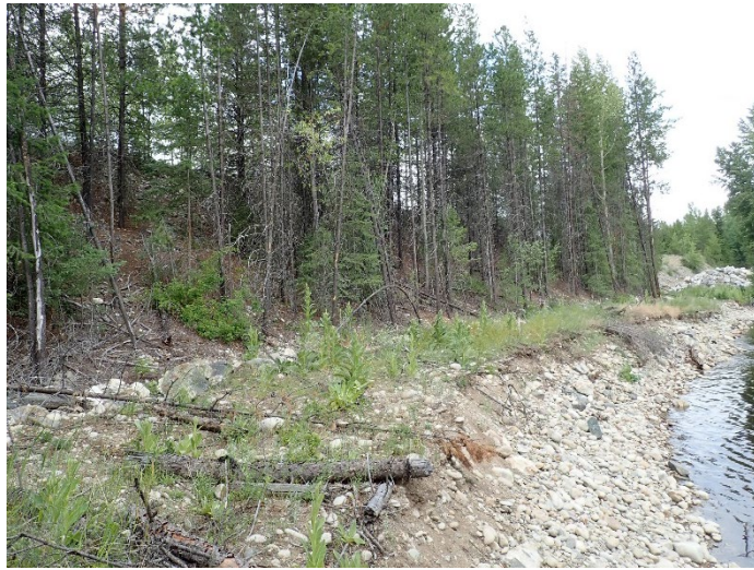
Photograph 9: South TSF, Cell 5, toe and downstream slope, looking northeast. 10 July 2019.
