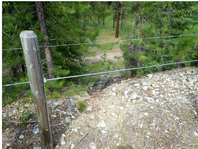
Photograph 27: North TSF, Cell 6, erosion on north embankment downstream slope, looking northeast. 10 July 2019.
