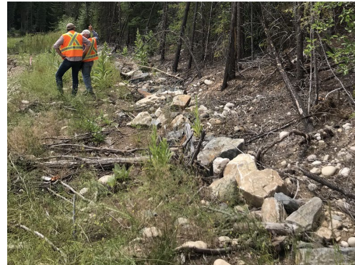
Photograph 8: South TSF, Cell 5, downstream dam slope riprap at toe, looking southwest. 10 July 2019.
