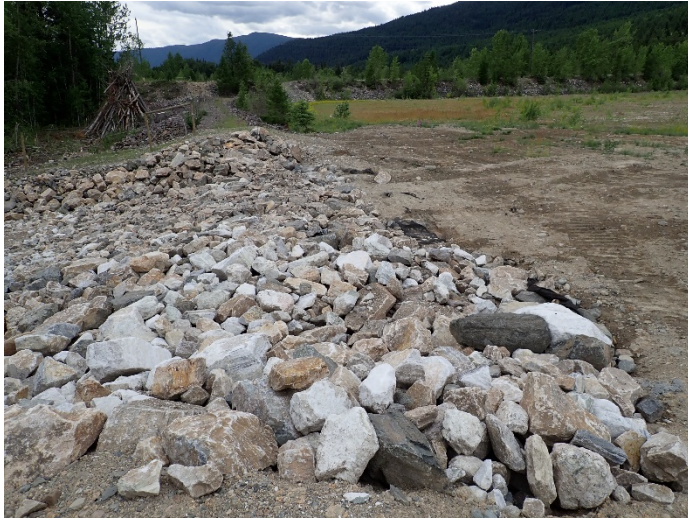
Photograph 17: South TSF, Cell 3, remediated spillway crest, looking southwest. 10 July 2019.
