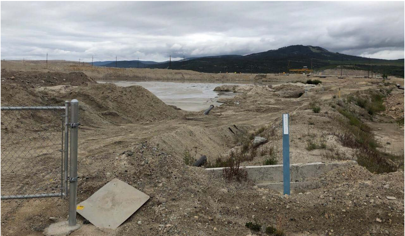
Photo II-4 Overview of pond and upstream slope of west and north perimeter access roads – good freeboard is maintained (SDP-2019-15)
