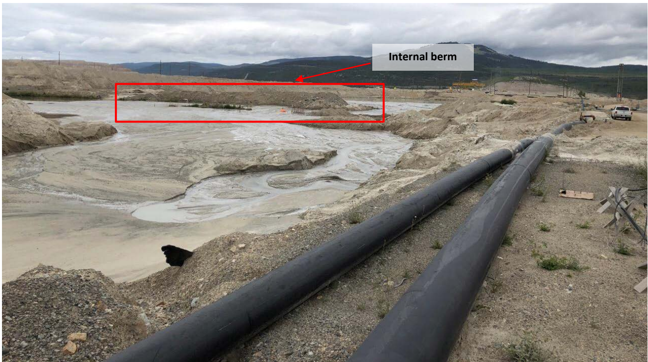
Photo II-10 Overview of the internal berm within the impoundment (SDP-2019-05)
