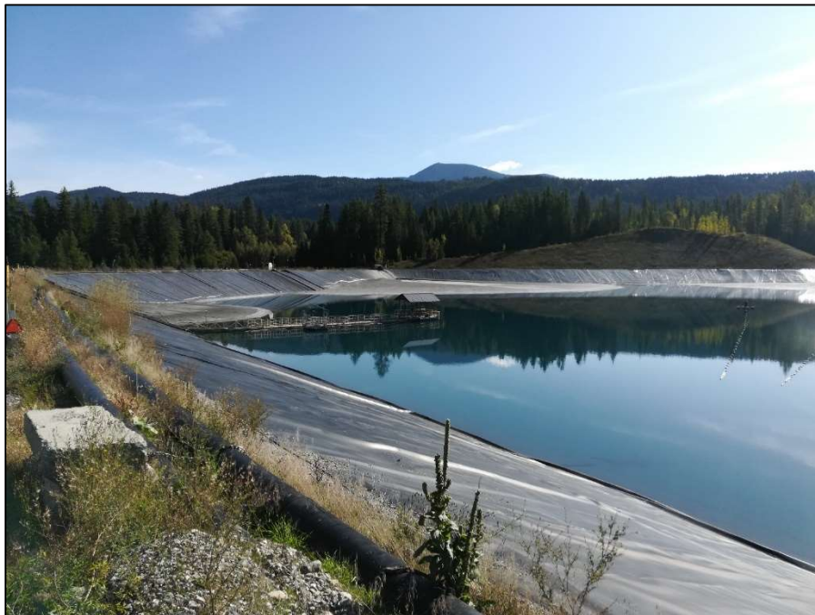
PHOTO 6 – Reclaim barge and upstream northwest embankment.
