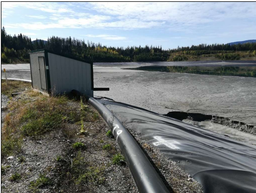
PHOTO 18 – E2 tailings discharge spigot looking south.
