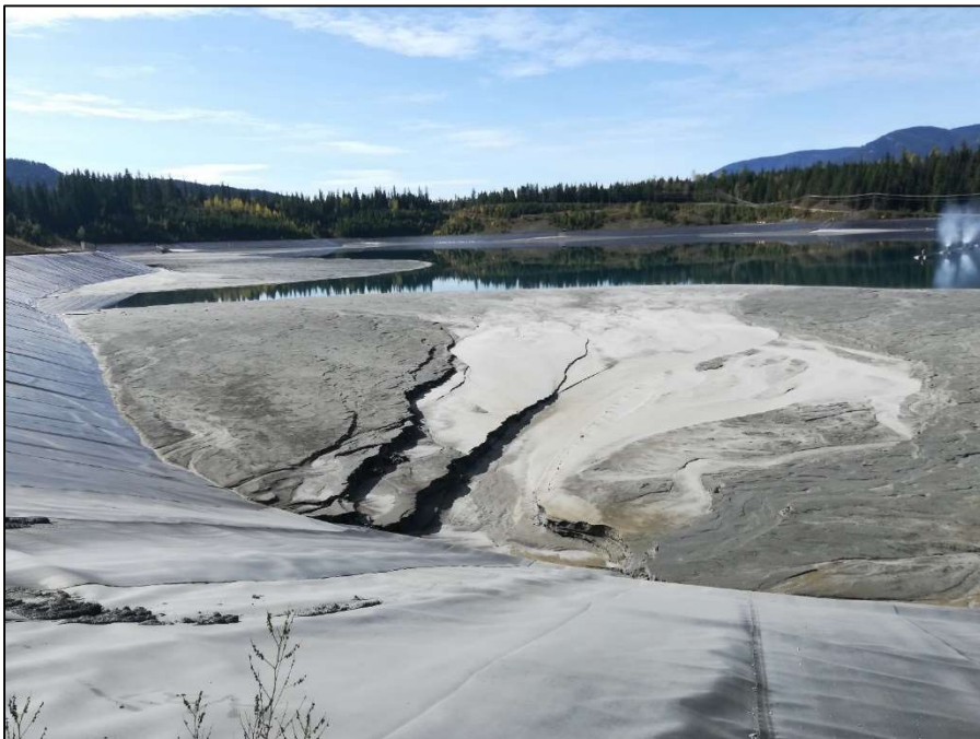
PHOTO 14 – Tailings beach at northwest end of facility
