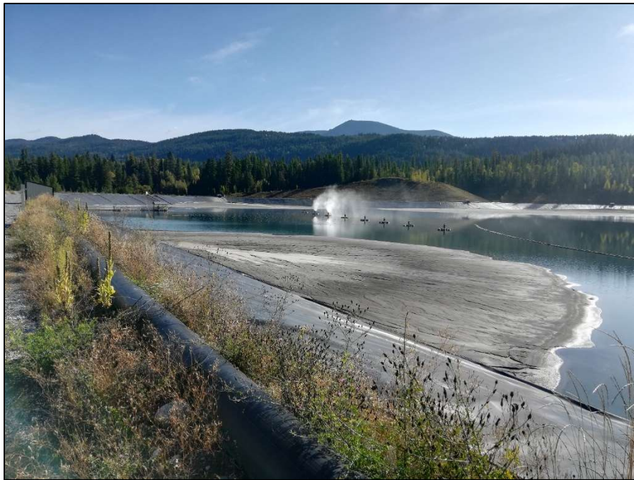
PHOTO 5 – Evaporators from the northwest. Two operational at time of inspection.
