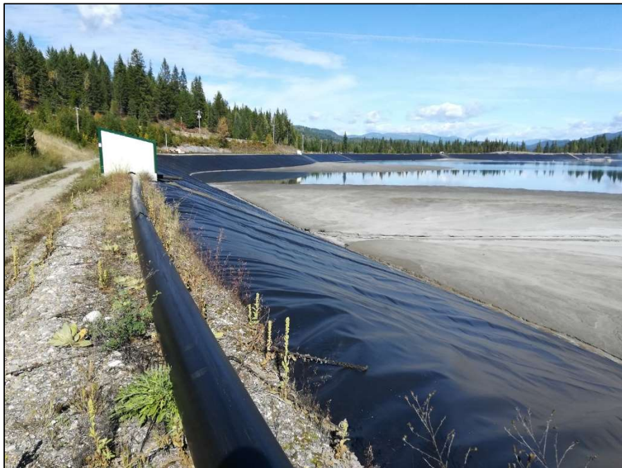
PHOTO 24 – Western portion of facility and W3 tailings discharge spigot looking north.
