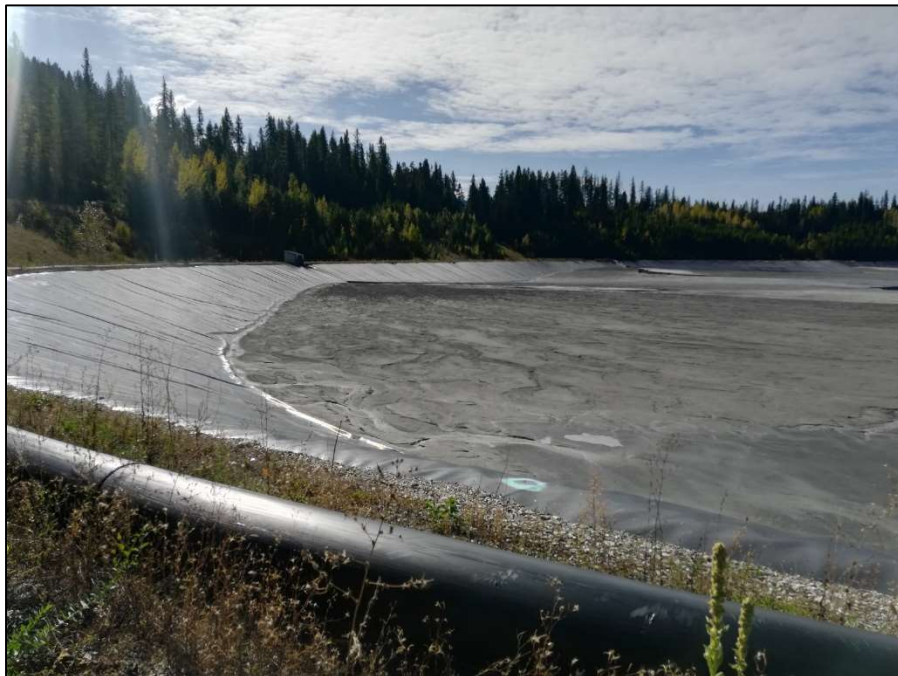
PHOTO 20 – Eastern facility slopes and tailings deposition.
