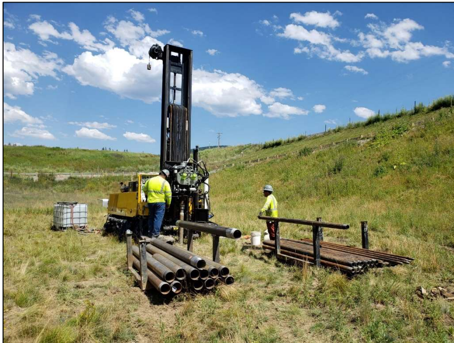
PHOTO 26 – Yellow Jacket Rig – Performing sonic drilling at northwest dam.
