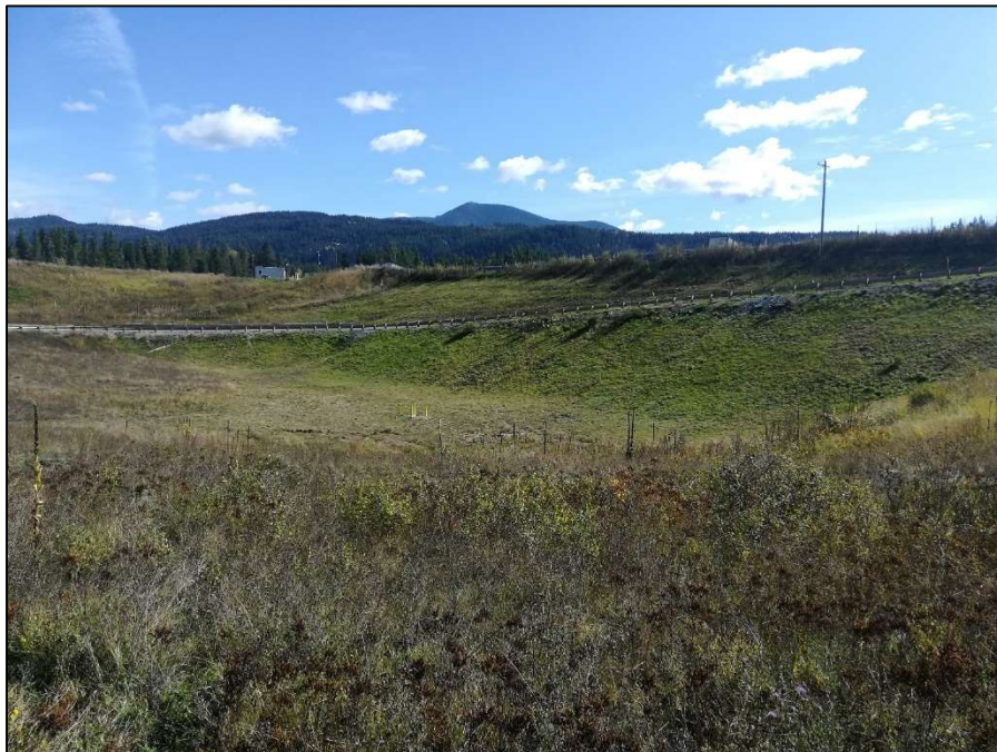
PHOTO 8 – Downstream face of northwest dam from toe.
