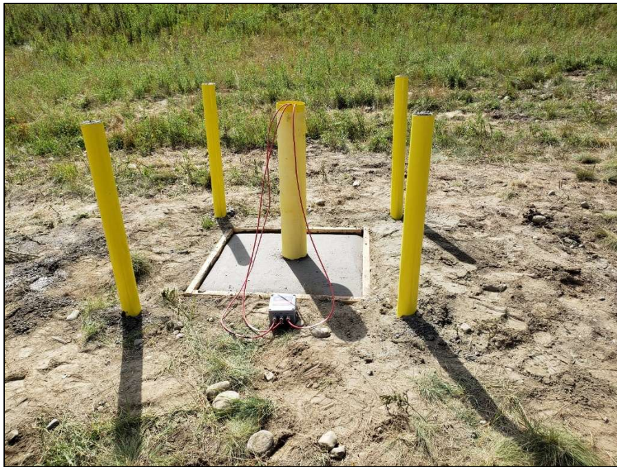
PHOTO 27 – Vibrating wire piezometer installation in standpipe at northwest dam.
