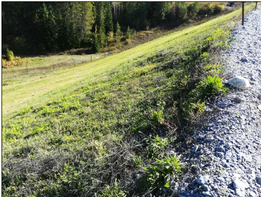
PHOTO 10 – Downstream face of northeast dam from crest.
