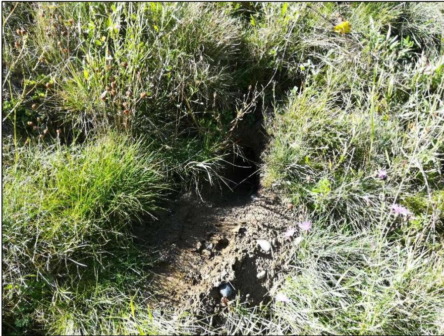
PHOTO 13 – Animal burrow at downstream toe of northeast dam.
