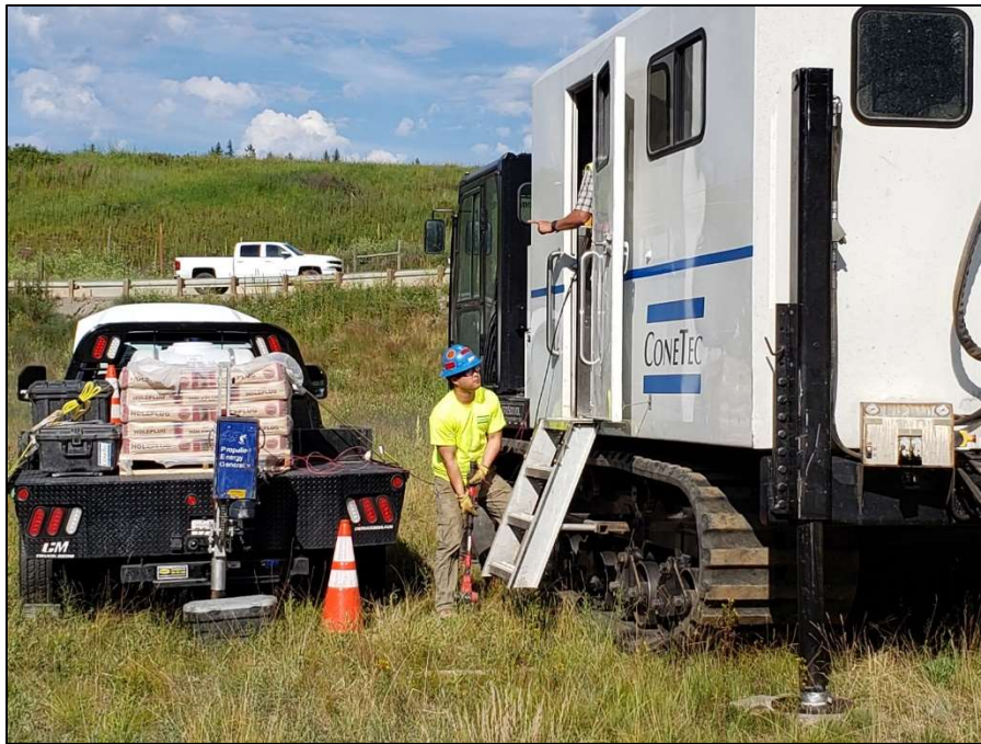
PHOTO 25 – Conetec CPT rig – Performing CPT at the northwest dam.
