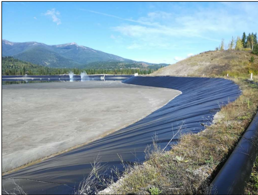
PHOTO 21 – Eastern portion of facility looking north.
