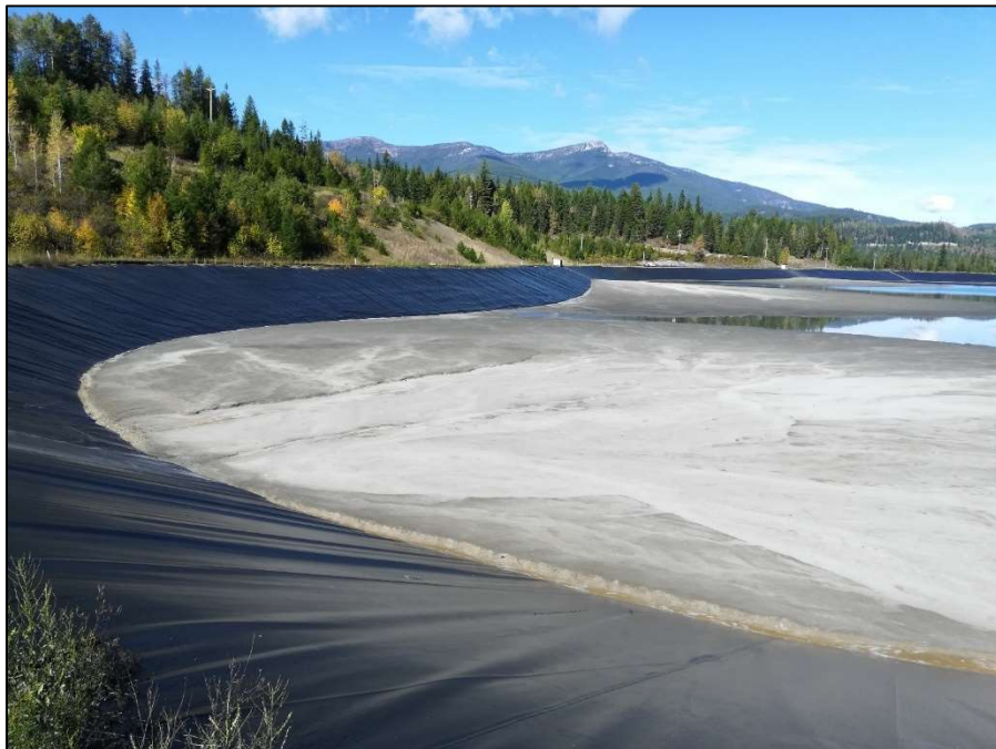
PHOTO 22 – Western portion of facility looking north.
