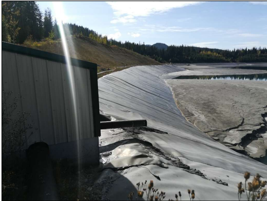
PHOTO 15 – E1 tailings discharge spigot looking south.
