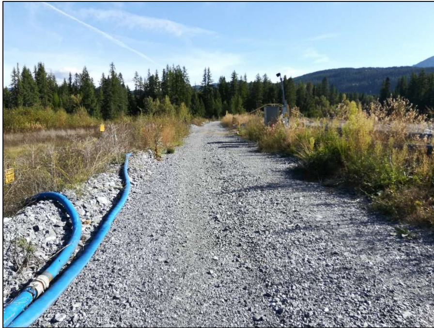
PHOTO 9 – TDF #3 perimeter road connecting northeast and northwest Dams.
