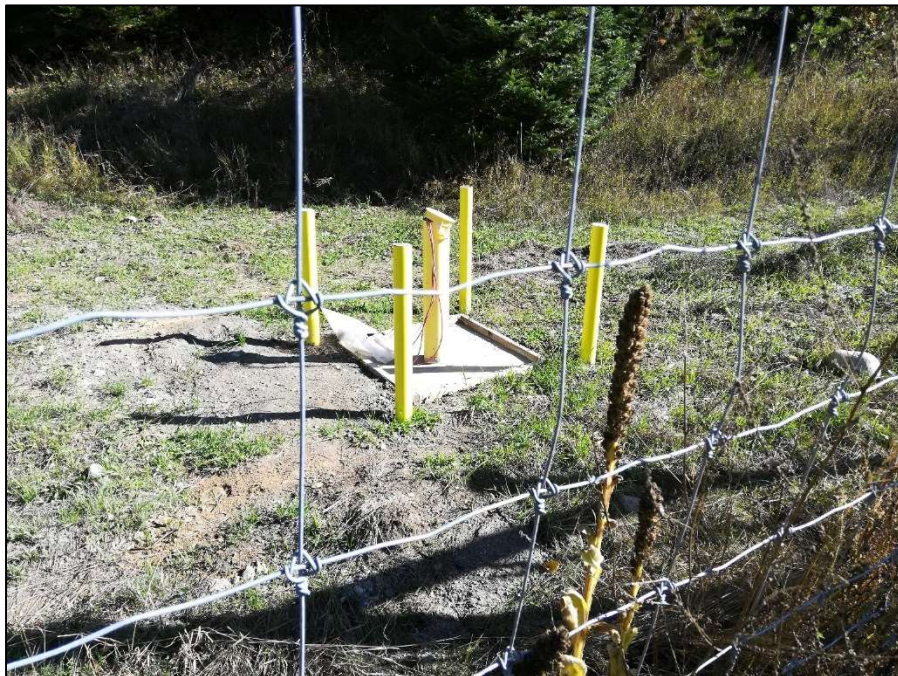
PHOTO 12 – Piezometer installed at northeast dam toe.
