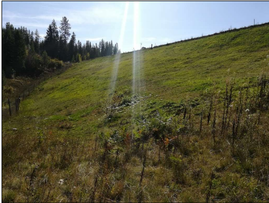
PHOTO 11 – Downstream face of northeast dam from toe.
