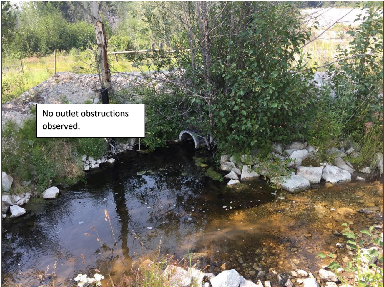
Photo II-C-7 Low-level outlet discharge pipe (TRJ-2018-34)
