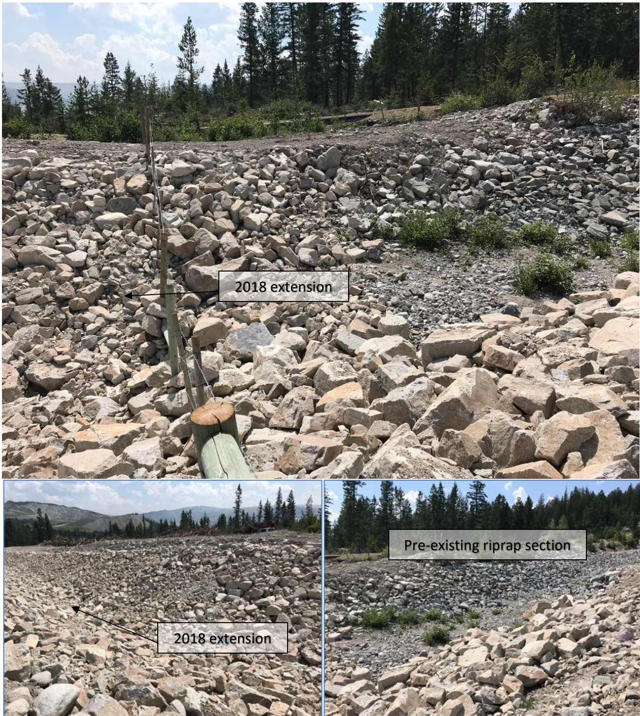
Photo II-A- 19 Spillway extension transition zone (TRJ-2018-22)
