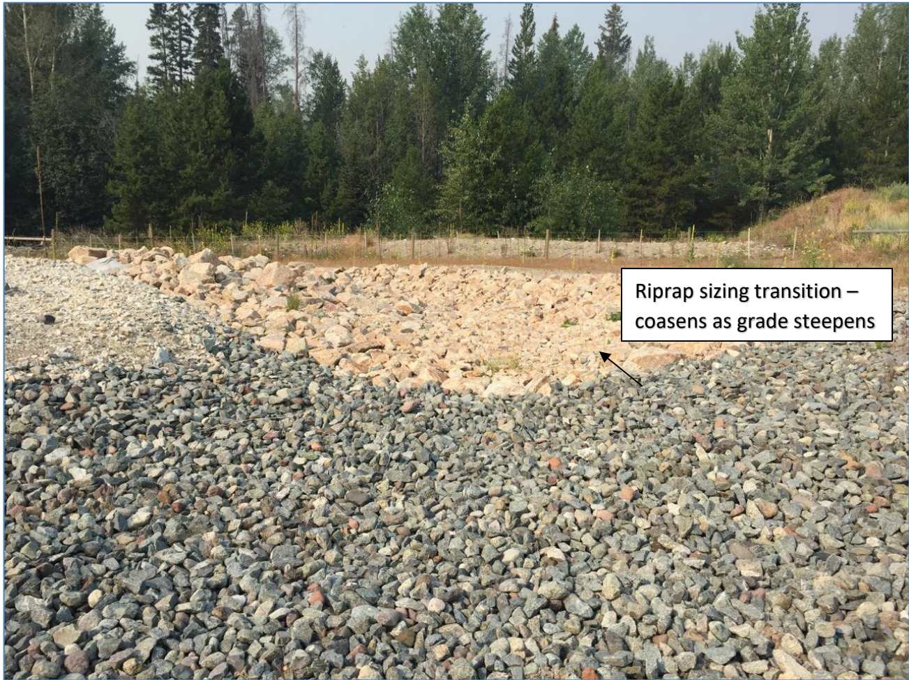
Photo II-B- 8 Spillway channel (TRJ-2018-28)
