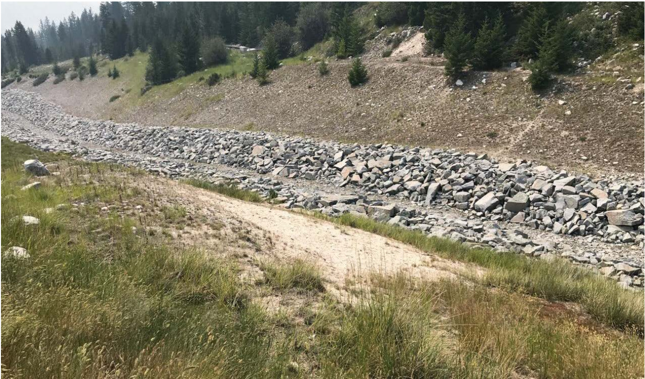
Photo II-A- 17 Spillway channel – extension of riprap section (TRJ-2018-20)
