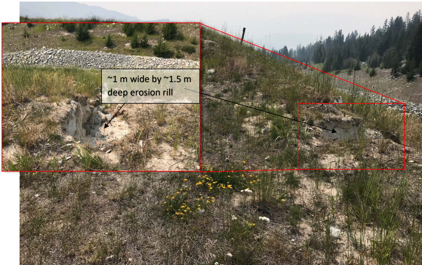
Photo II-A- 15 Spillway channel – left bank dam slope erosion feature (TRJ-2018-17)
