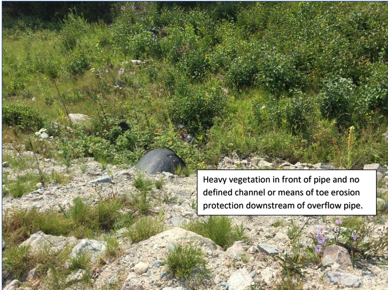
Photo II-C-2 Downstream slope near right abutment with overflow pipe (TRJ-2018-31)
