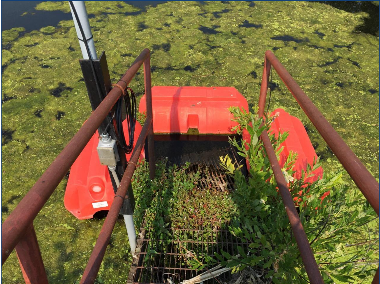
Photo II-C-6 Low-level outlet intake and secured debris booms (TRJ-2018-33)
