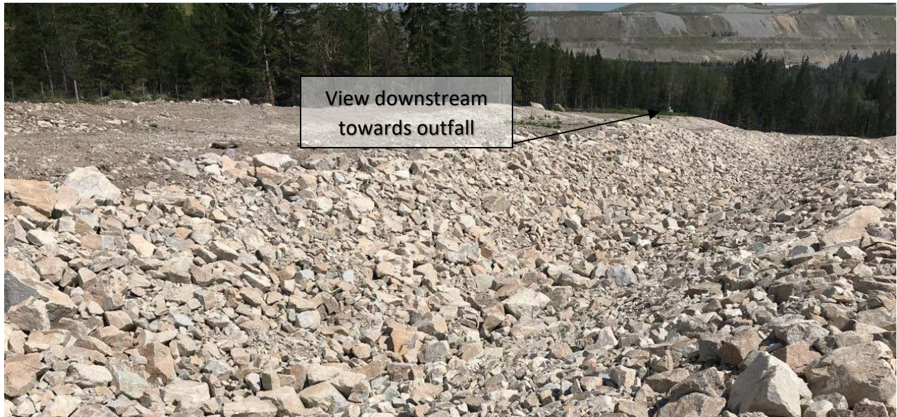
Photo II-A- 18 Spillway channel – extension of riprap section (TRJ-2018-21)
