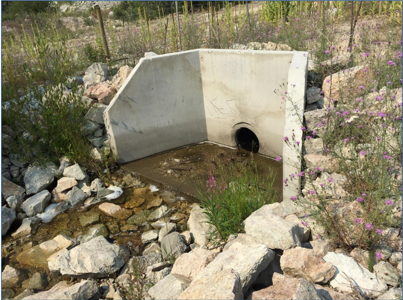
Photo II-C-8 Inflow culvert from Trojan Diversion Ditch (TRJ-2018-34)
