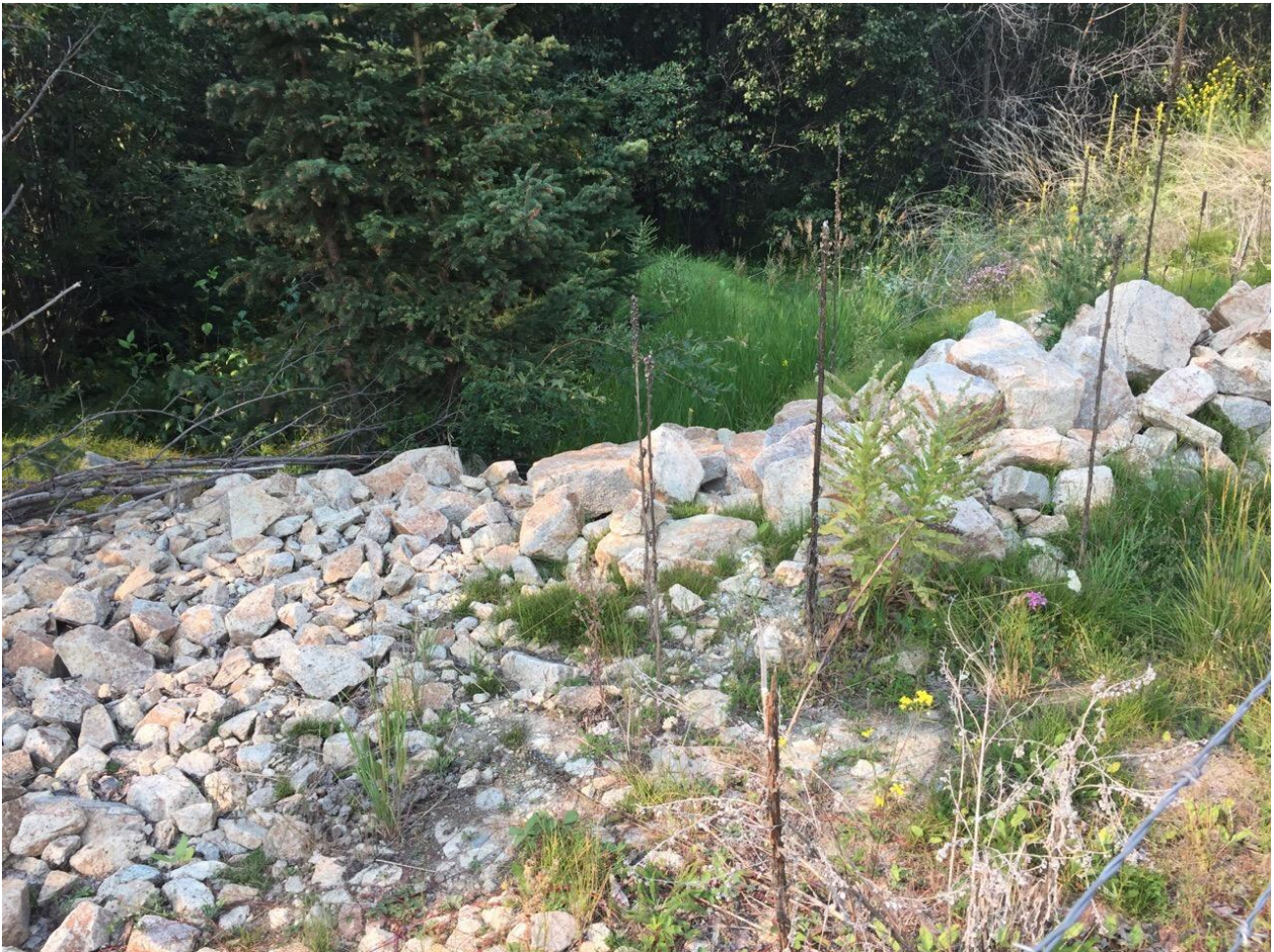
Photo II-B- 9 Spillway channel – transition to grass-lined channel (TRJ-2018-29)
