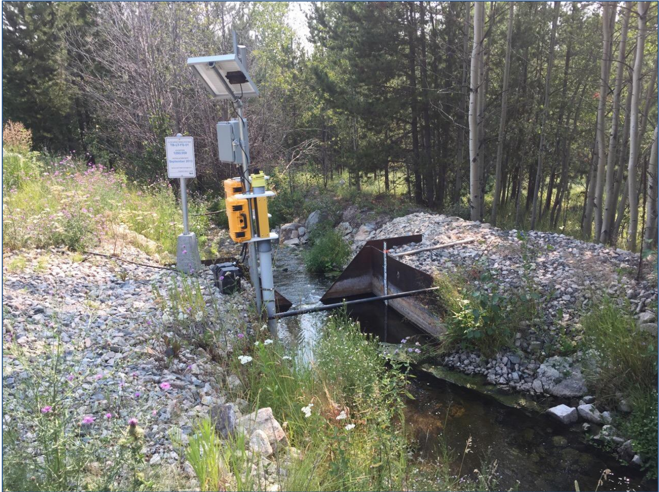
Photo II-C-9 Discharge channel to weir TB-LT-FS-01 (TRJ-2018-34)
