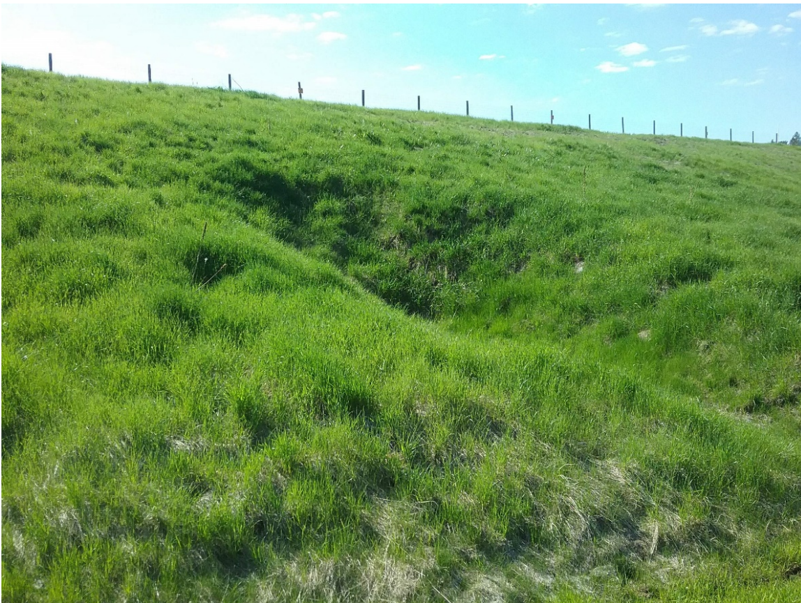
Photo A.6 Localized Depressions on Downstream Face of ARD Pond North Dam
