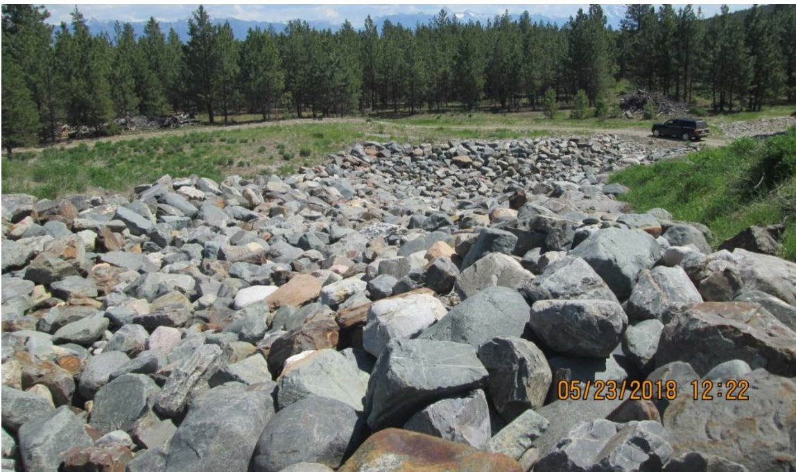
Photo B.6 Downstream End of the Emergency Spillway
