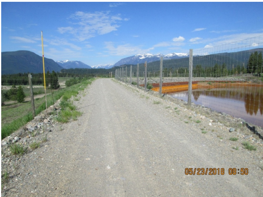
Photo A.2 Crest and Upstream Slope of ARD Pond South Dam
