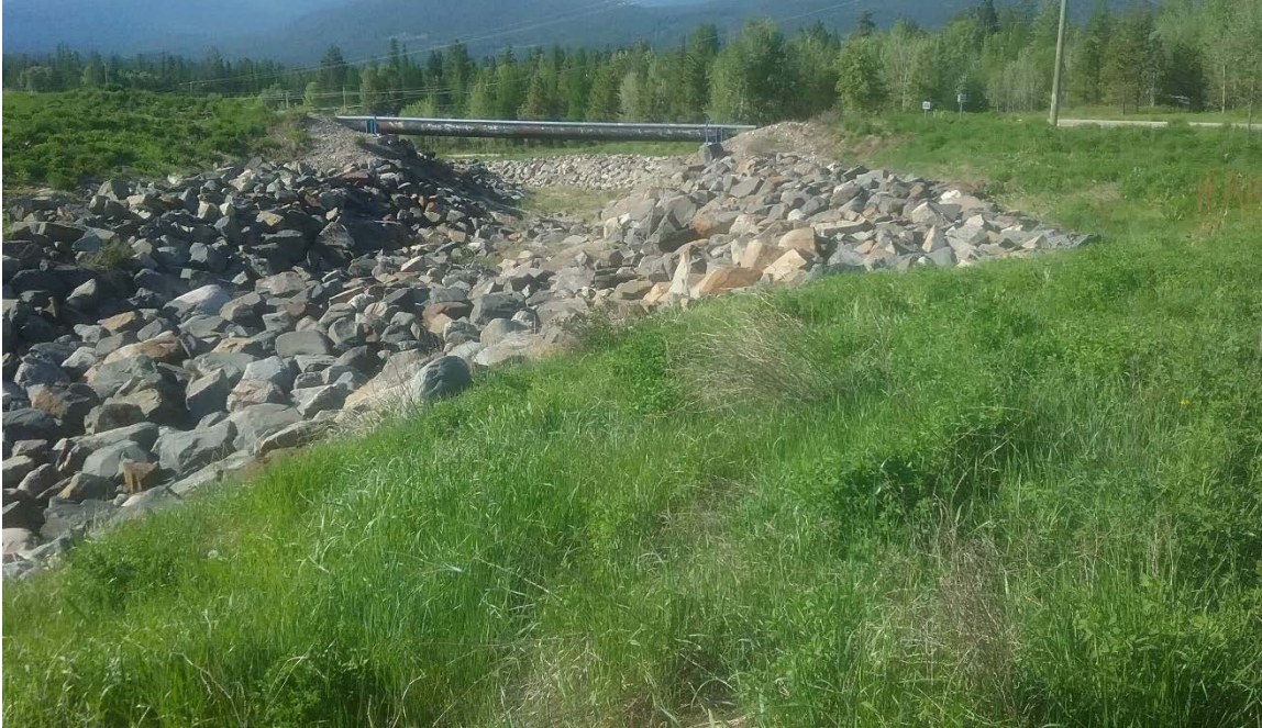
Photo B.6 Downstream End of the Emergency Spillway
