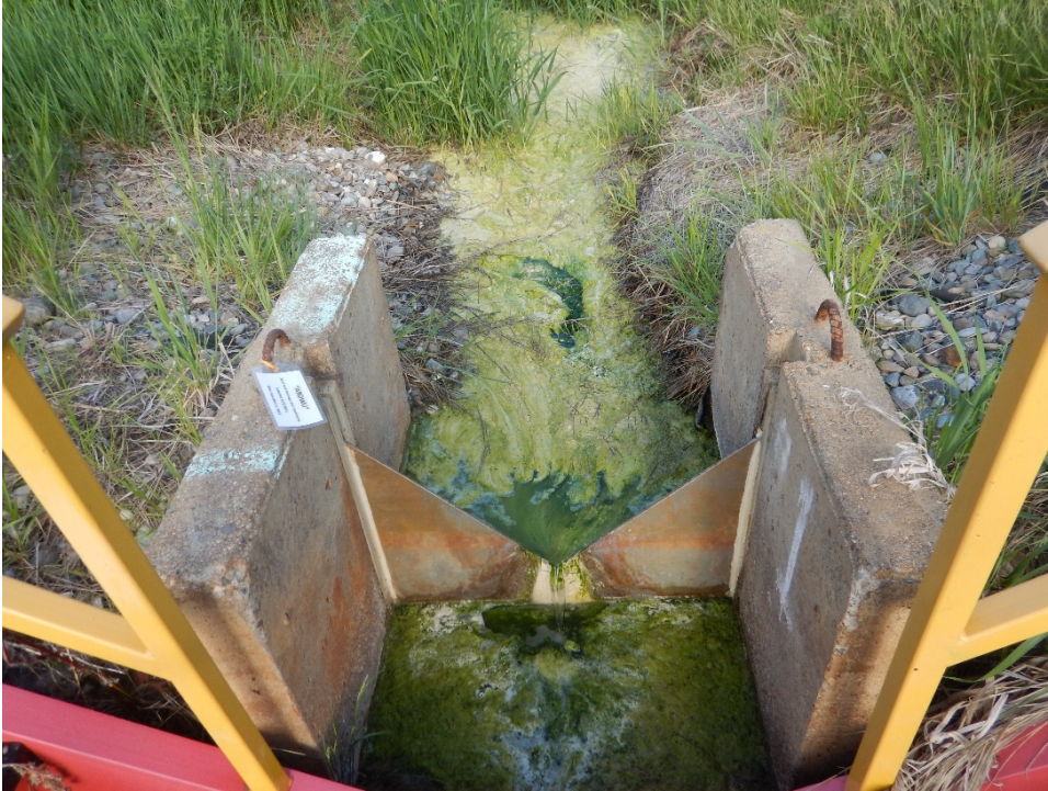
Photo A.12 Weir #1 Downstream of ARD Pond. Channel requires cleaning
