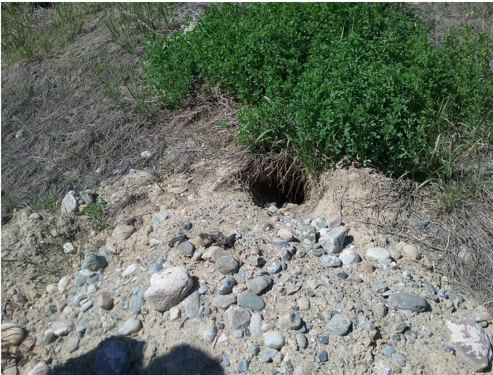
Photo F.8 Animal Burrow in West Gypsum Dike
