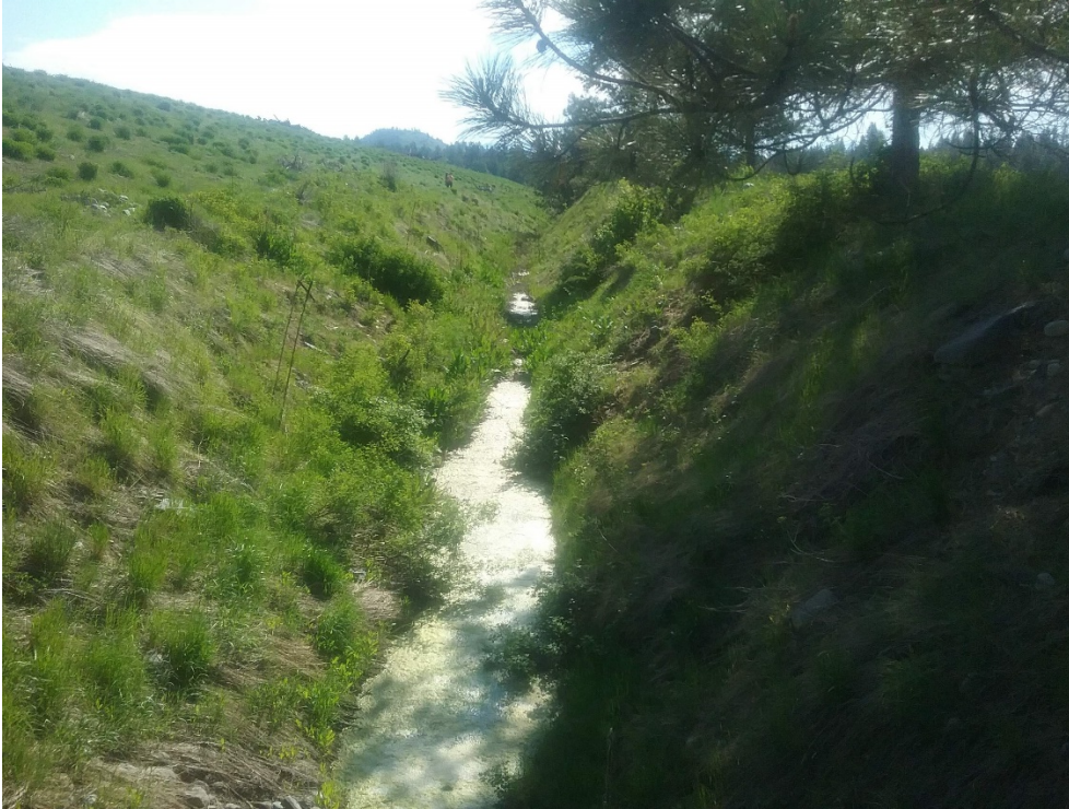
Photo F.6 Seepage Collection Ditch Downstream of Gypsum Dikes
