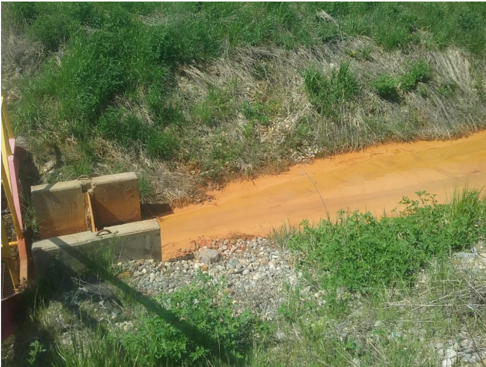
Photo G.9 Silting of Channel upstream of Weir #4
