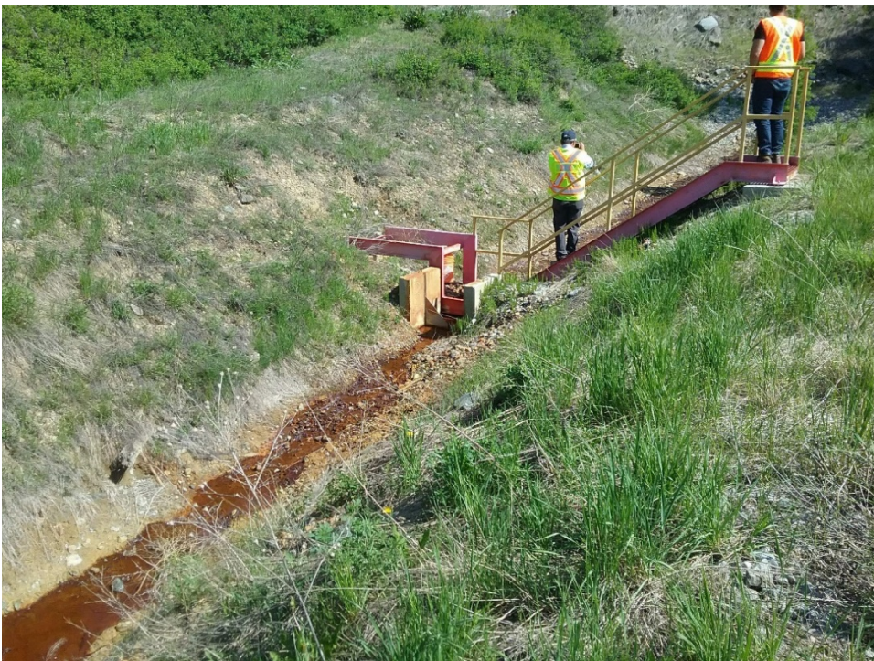
Photo G.2 Seepage Collection Ditch at Toe of Iron Dike
