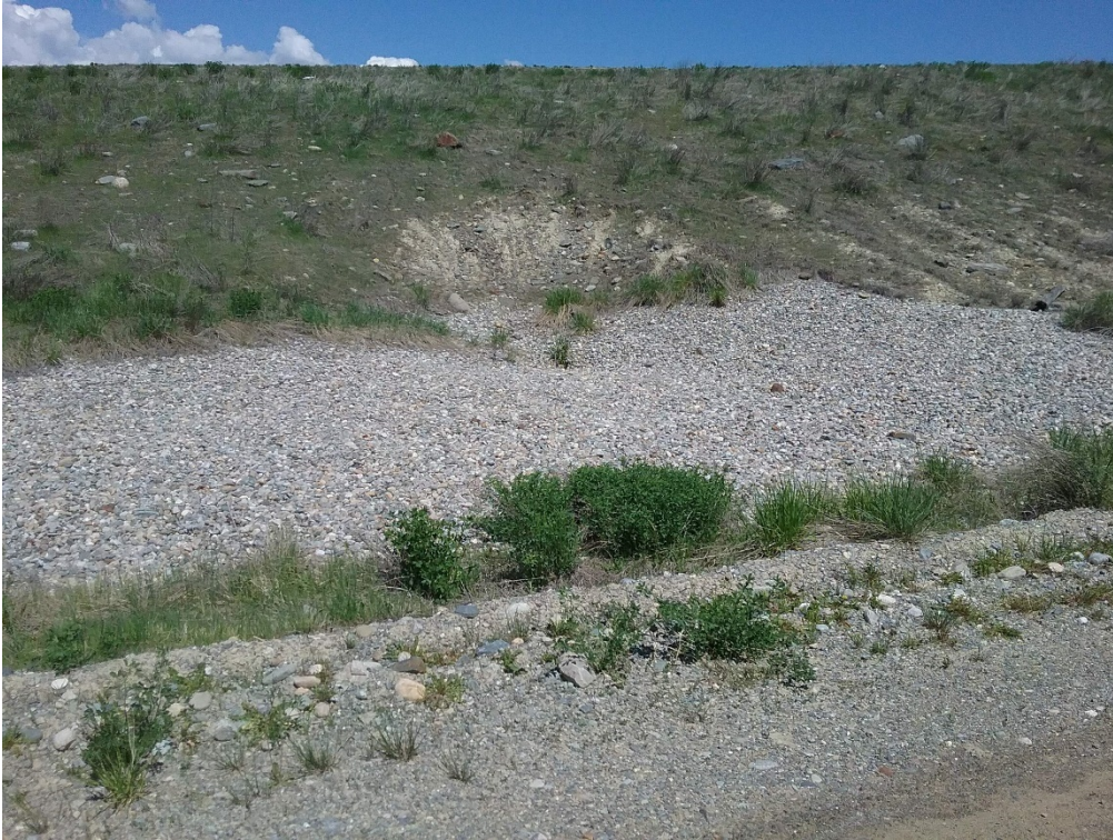
Photo G.8 Seepage Collection Ditch downstream from Iron TSF (Weir #4)
