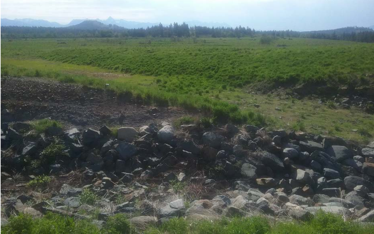
Photo F.2 Animal Burrows at Toe of West Gypsum Dike
