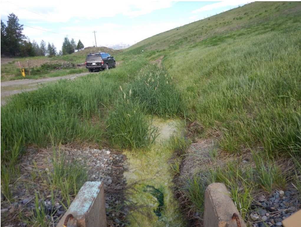
Photo A.12 Weir #1 Downstream of ARD Pond. Channel requires cleaning
