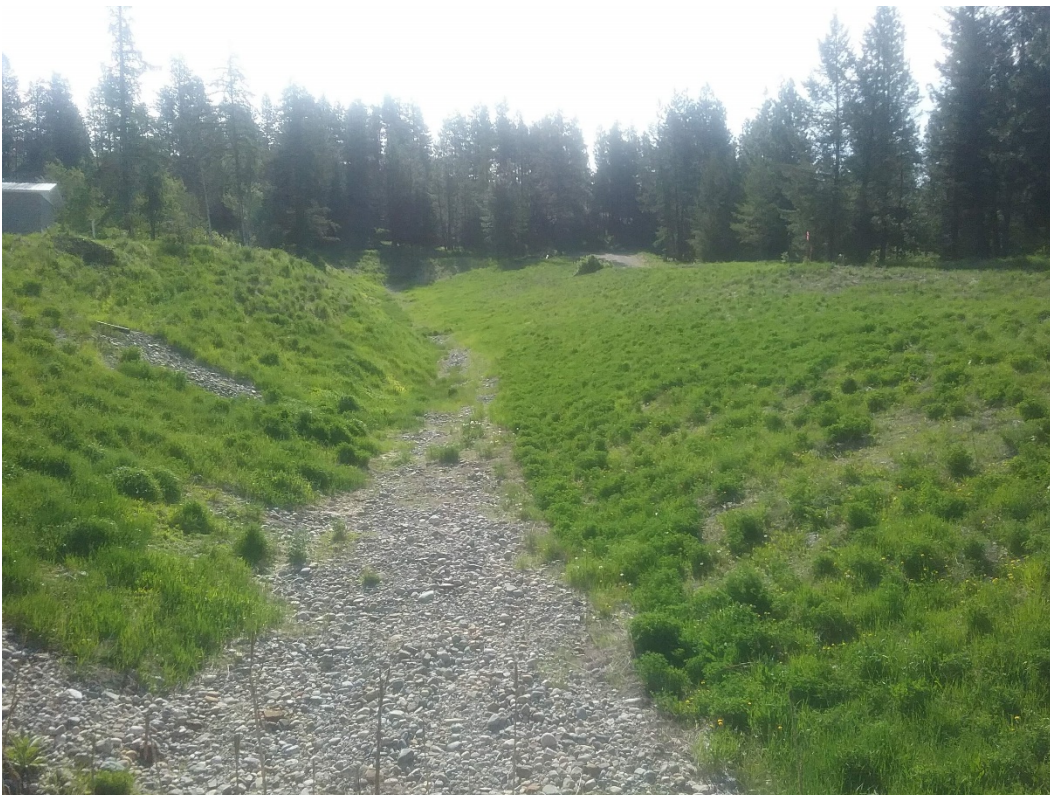
Photo F.6 Seepage Collection Ditch Downstream of Gypsum Dikes
