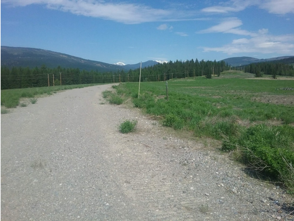
Photo H.3 Crest and Downstream Slope of Old Iron Dike
