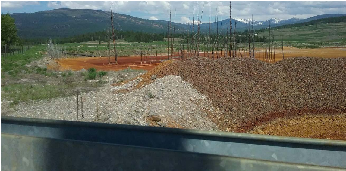
Photo I.3 Overview of tailings area and Iron Pond
