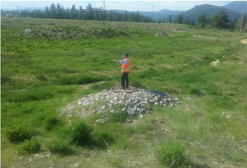
Photo F.4 Decommissioned Decant Pipe downstream of East Gypsum Dike
