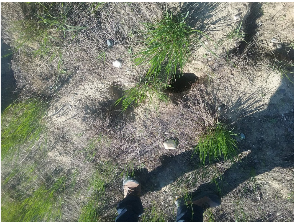
Photo F.2 Animal Burrows at Toe of West Gypsum Dike
