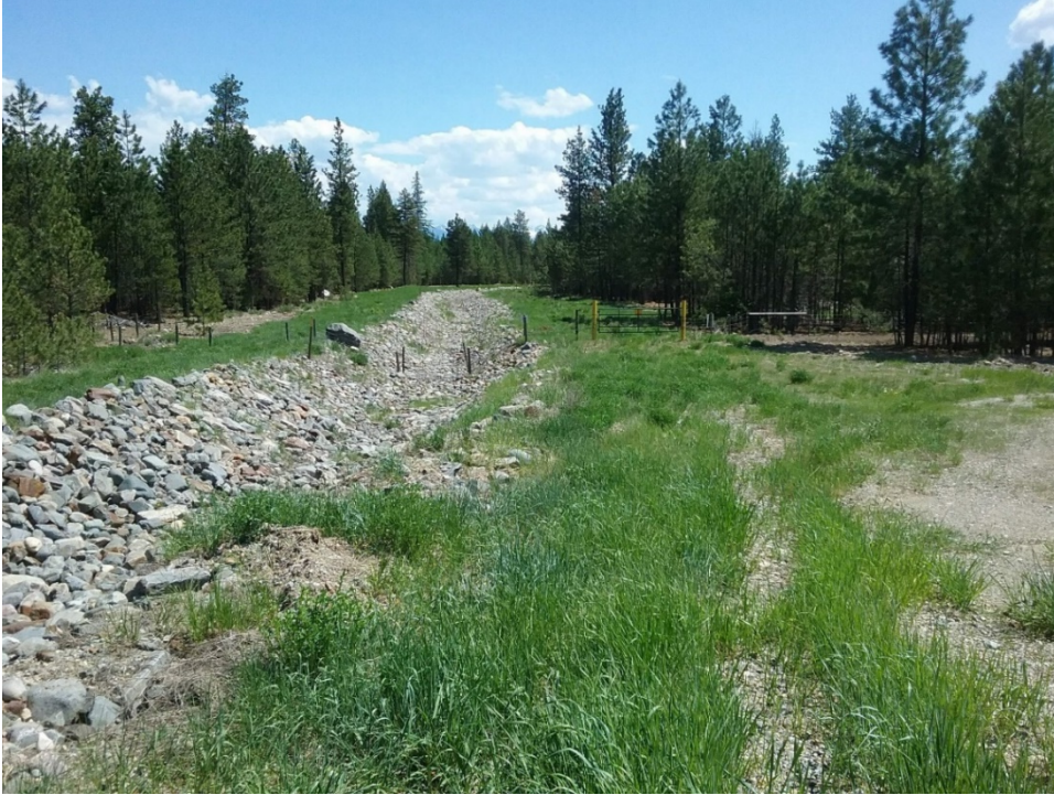
Photo C.2 Downstream Slope of Siliceous Dike
