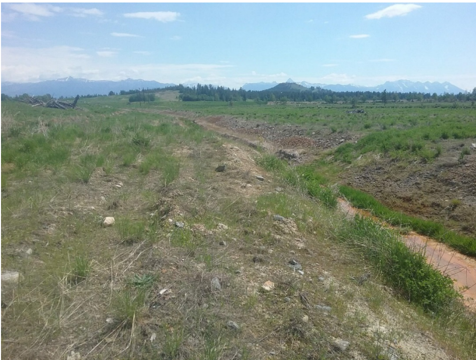
Photo G.8 Seepage Collection Ditch downstream from Iron TSF (Weir #4)
