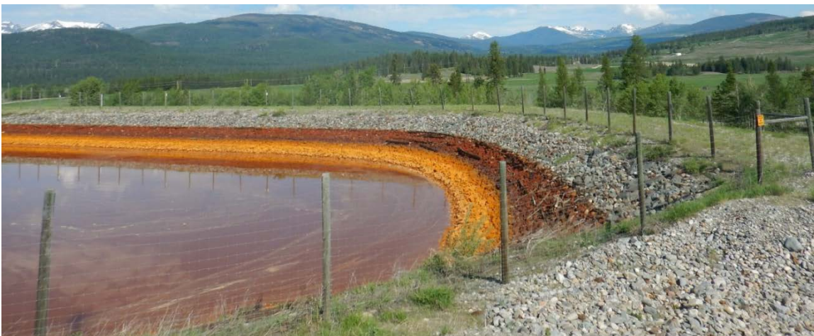
Photo A.4 Upstream Face of ARD Pond North Dam
