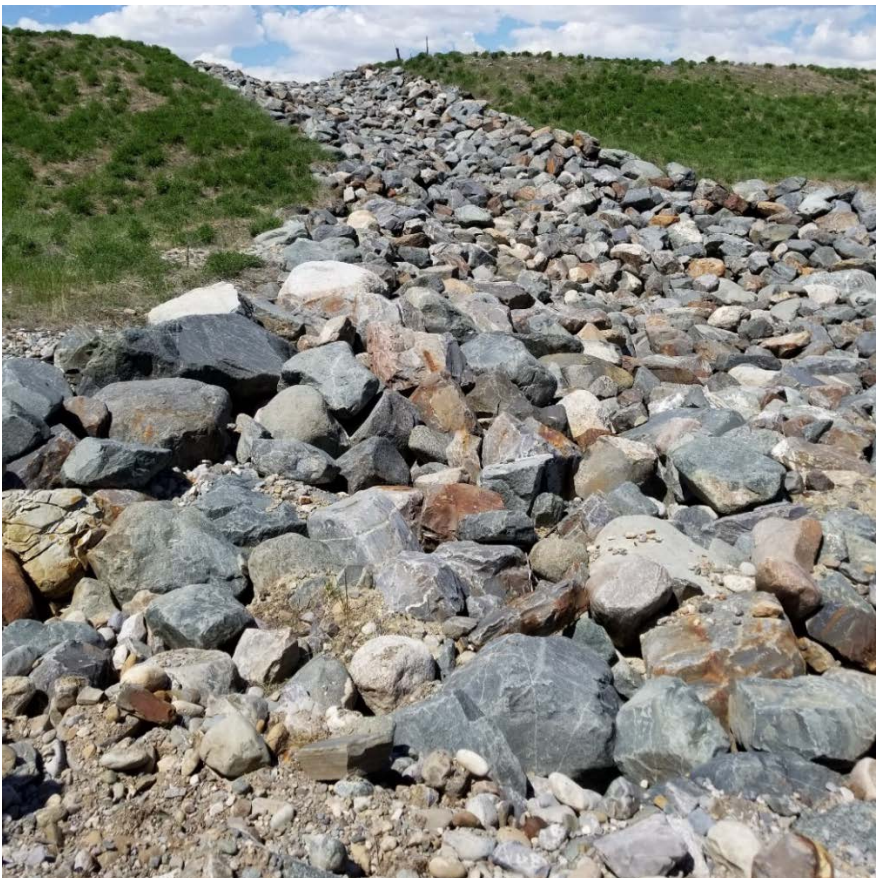
Photo C.4 Siliceous TSF Emergency Spillway
