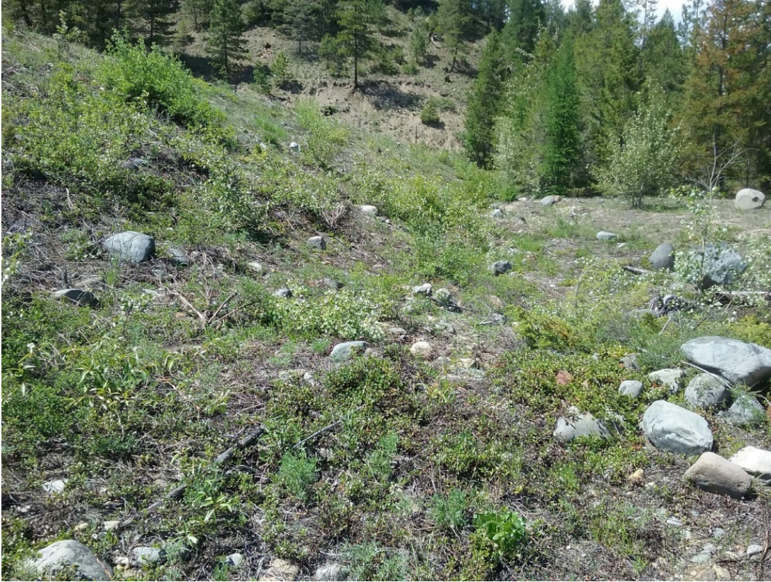
Photo D.5 Sludge Impoundment North Dike Downstream Slope
