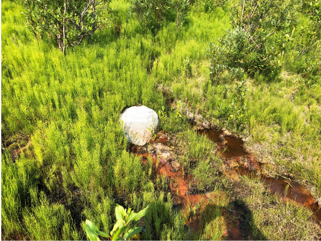
Photo 7: Seepage at toe of North Dam, mainly due to hillside seepage from the west
