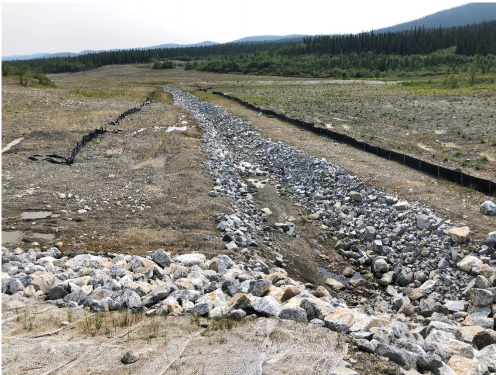
Photo 20: View of the south channel looking south from the SRS Dyke
