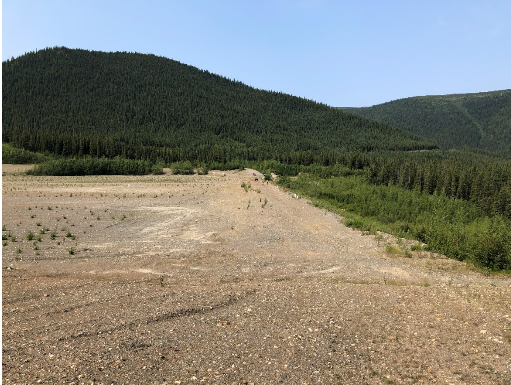
Photo 1: North Dam Crest looking west
