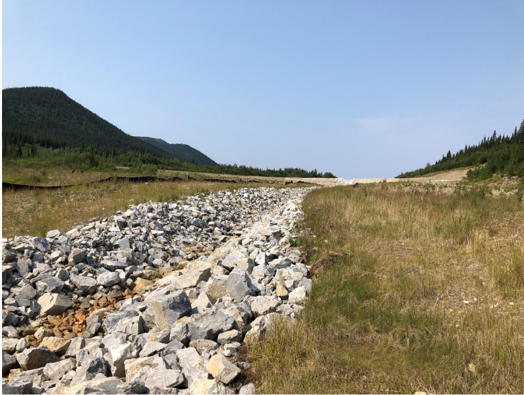
Photo 23: View north along the South Diversion drainage channel
