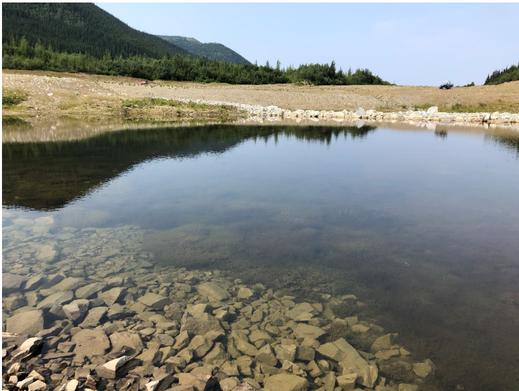
Photo 18: Sediment collection pond upstream of SRS
