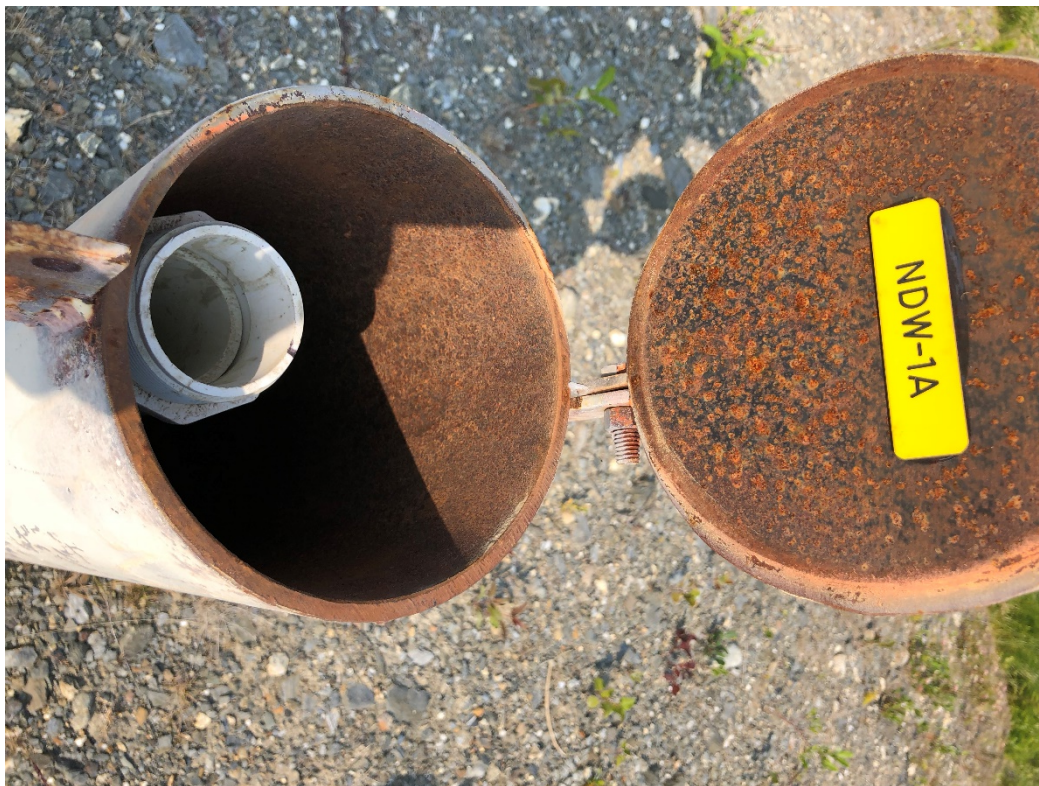
Photo 4: Missing cap on Piezo NDW 1A.
