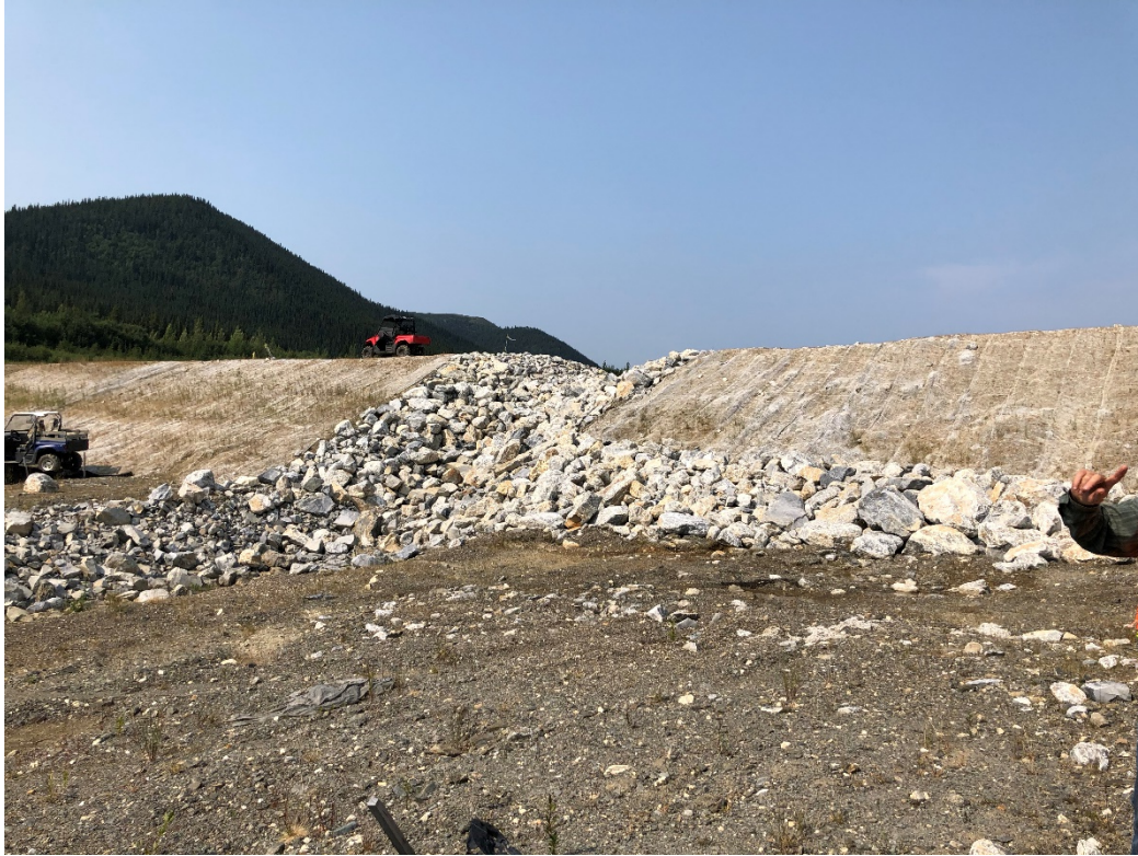
Photo 17: View looking north of the spillway at the SRS
