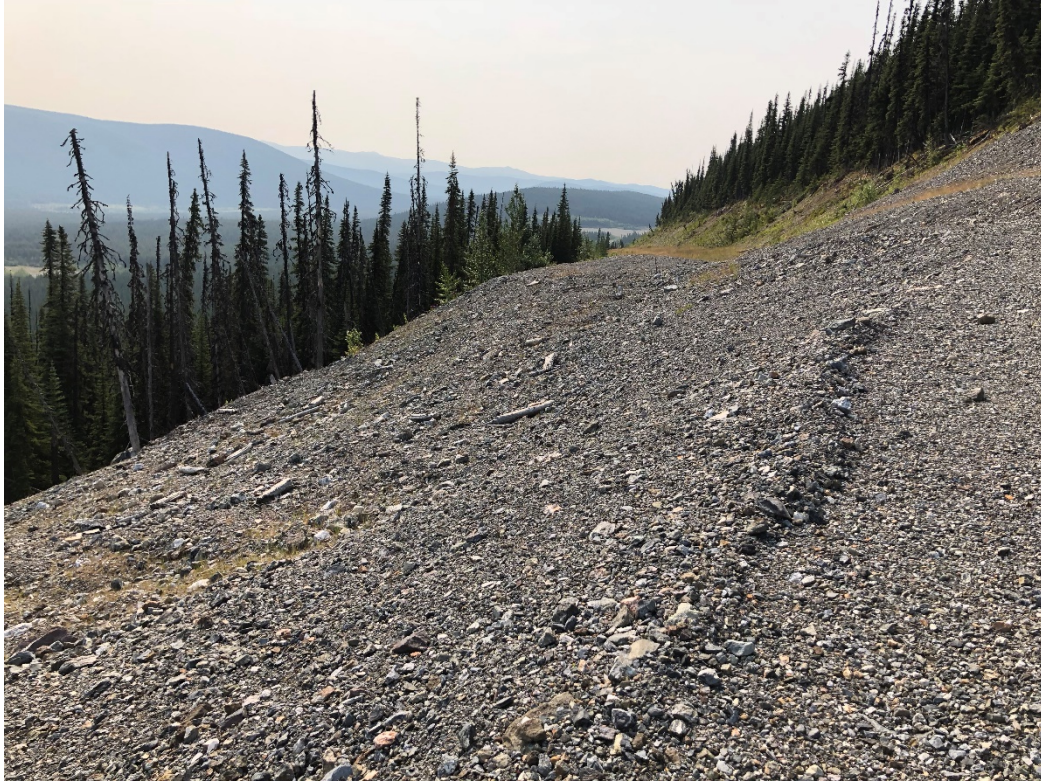
Photo 27 minor subsidence on the slope of the backfill at Portal 1200 on Burnick
