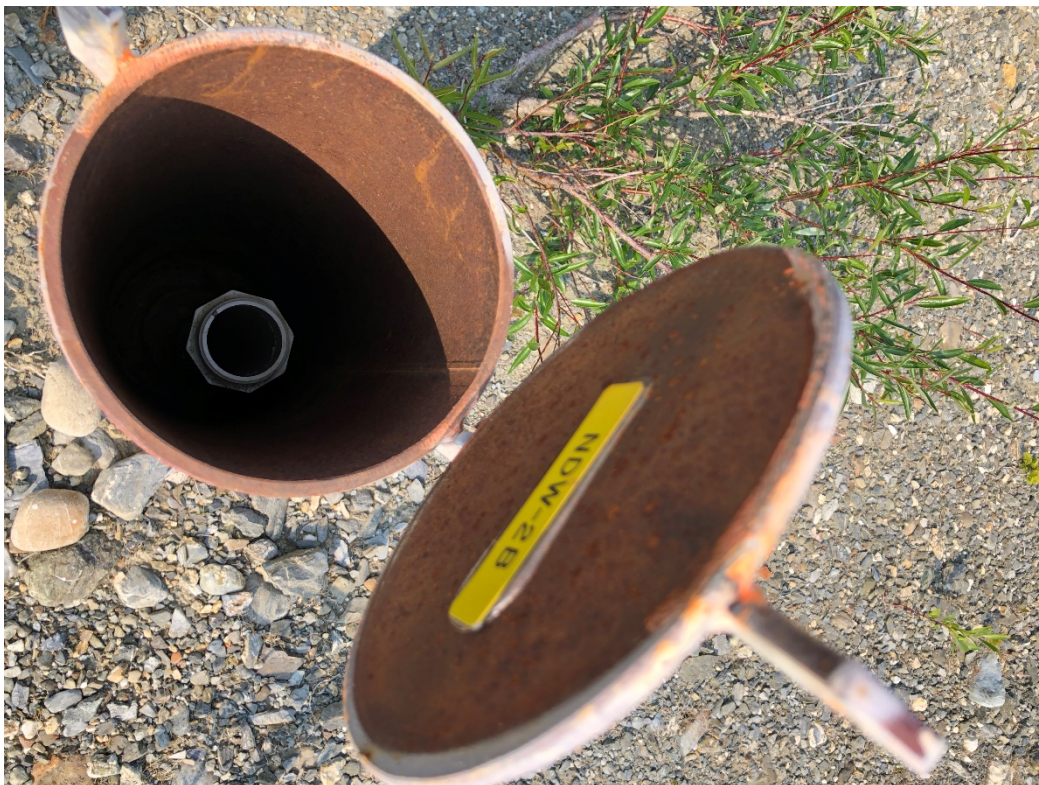
Photo 6: Missing cap on Piezometer NDW-2B
