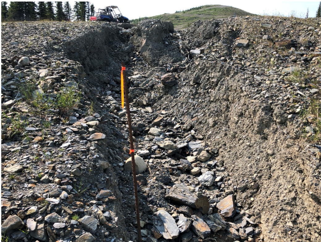
Photo 26: erosion gully at toe of Jewelbox waste rock dump with monitoring pin
