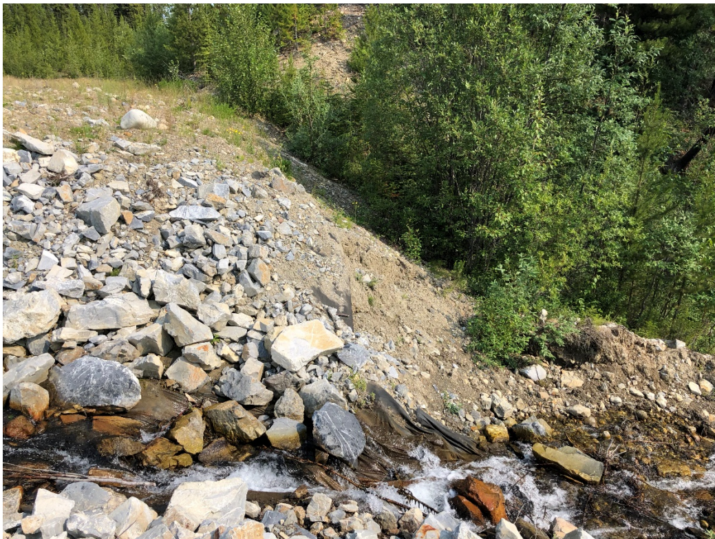
Photo 14: Outlet of North Creek crossing
