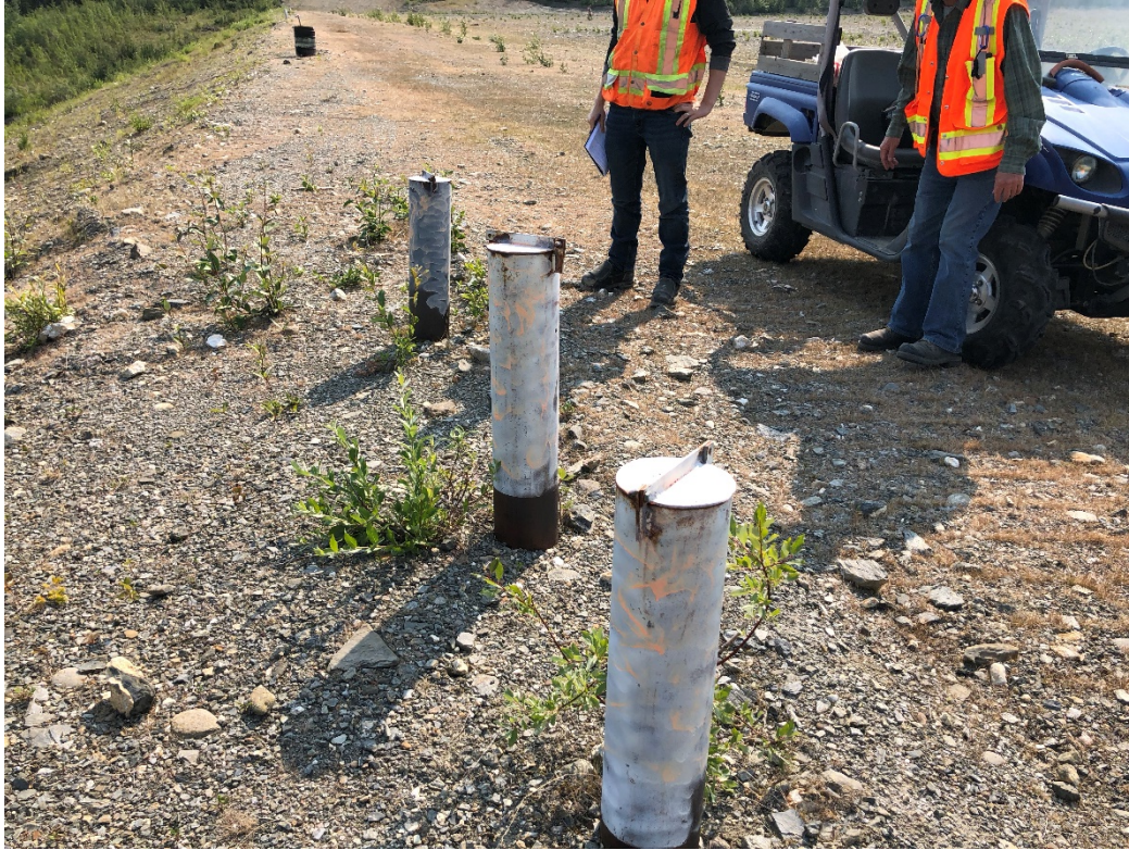
Photo 3: North Dam Piezometers NDW-3A and 3B, NDS-3
