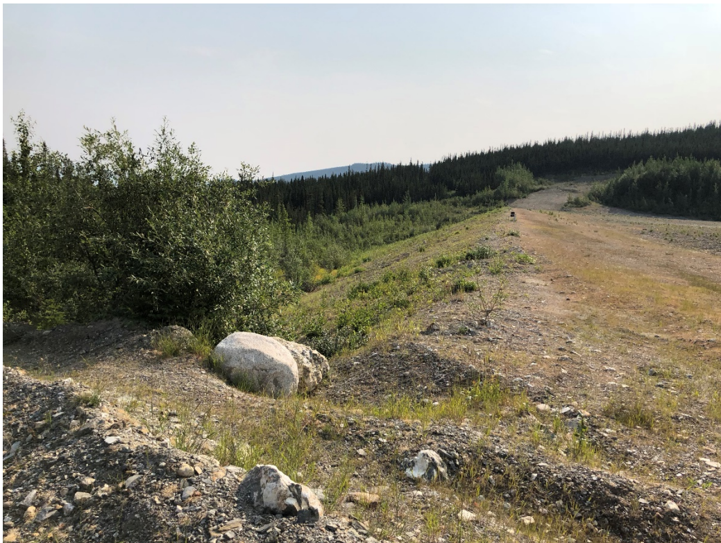
Photo 2: Downstream slope of the North Dam looking east
