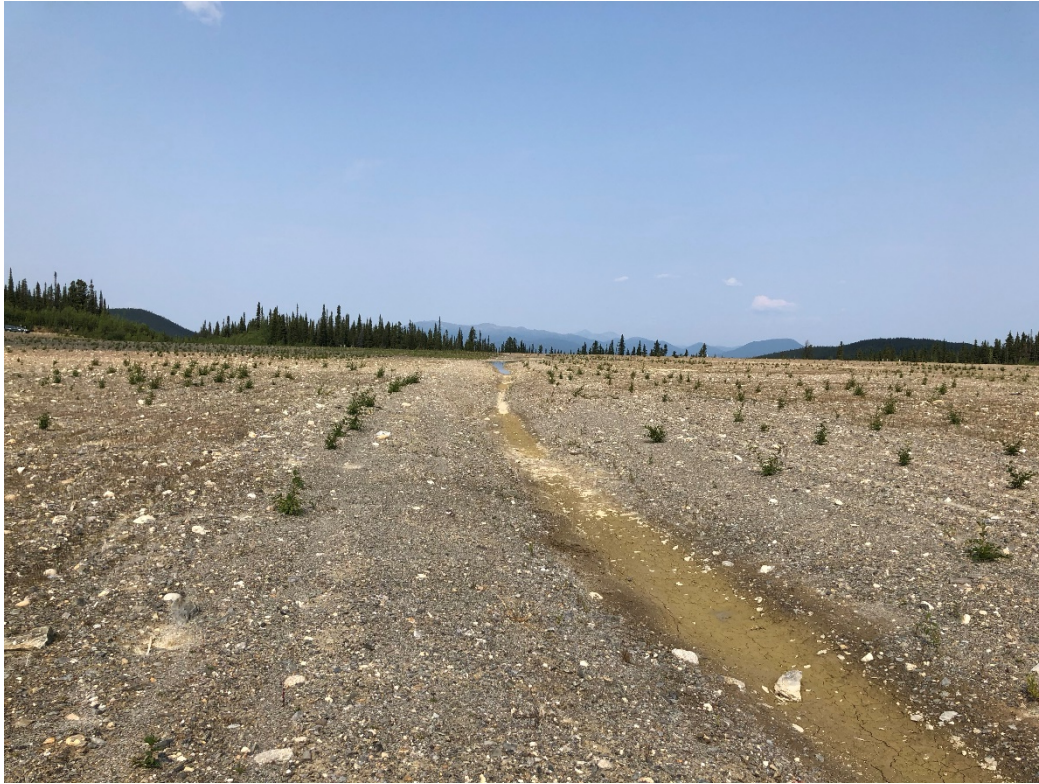
Photo 9: View looking north of drainage swale on tailings till cover
