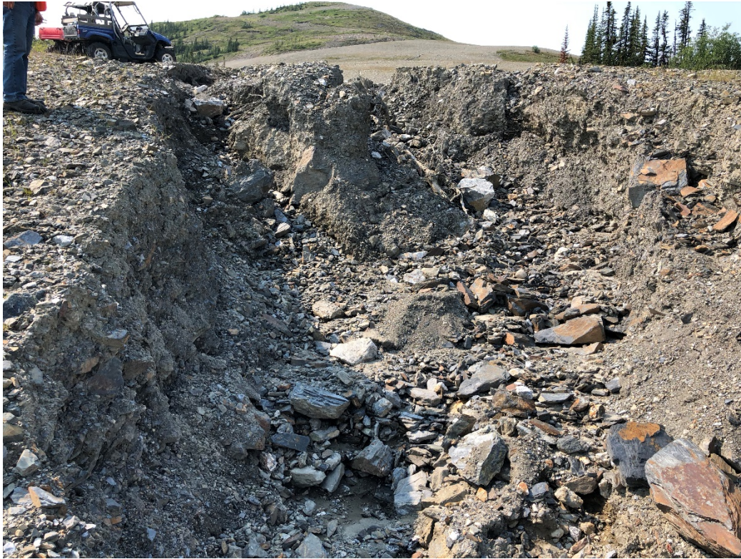
Photo 25: Erosion gully at toe of Jewelbox Waste rock dump
