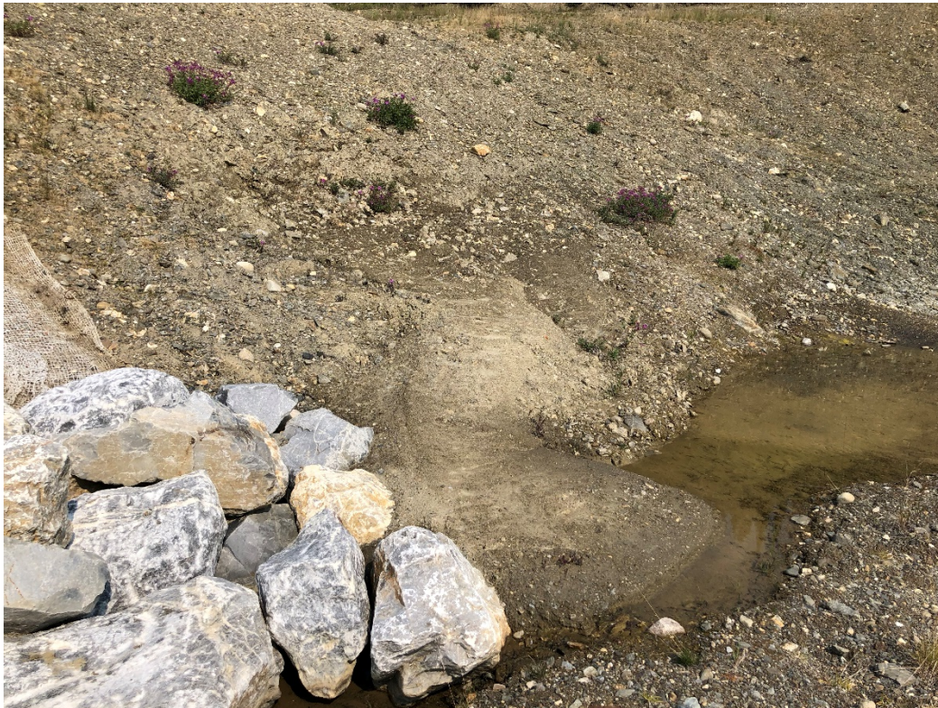
Photo 19: View of the eastern end of the riprap buttress along the D/S toe of the SRS dyke
