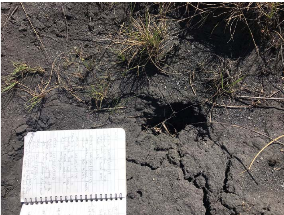
Photo I-19 Sinkhole 5 – first observed in 2017. Approximately 0.2 m x 0.1 m x 0.2 m deep (SNTD-SINKHOLE-05)
