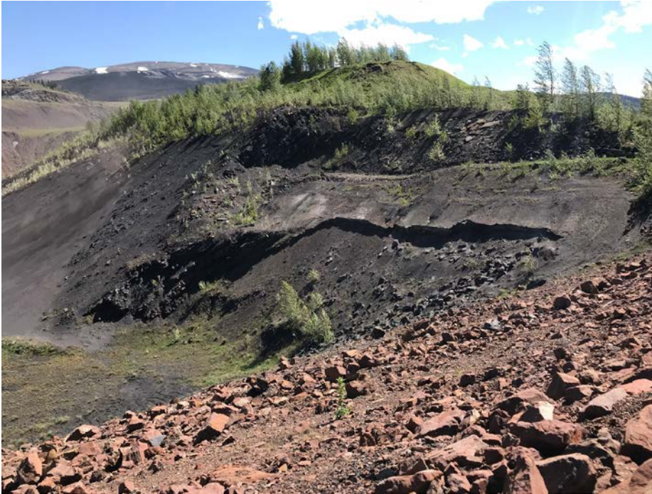
Photo I-6 West abutment, continued ravelling of shale slope upstream of abutment. No significant changes from 2017 condition (SNTD-2018-03)
