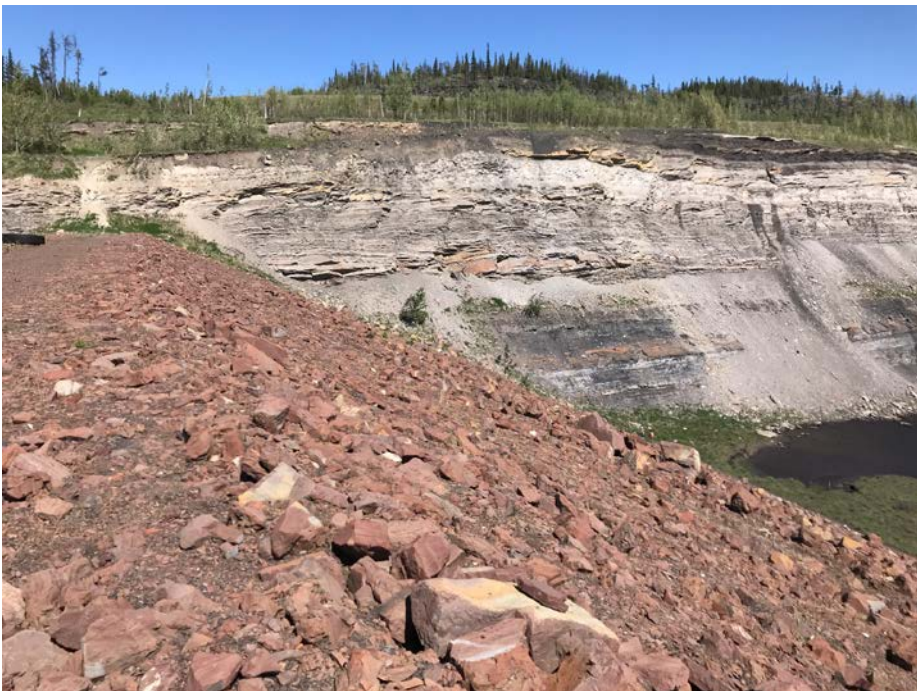
Photo I-7 Upstream slope taken from mid-length of the crest – looking north. Slope appears to be in good condition (SNTD-2018-03)
