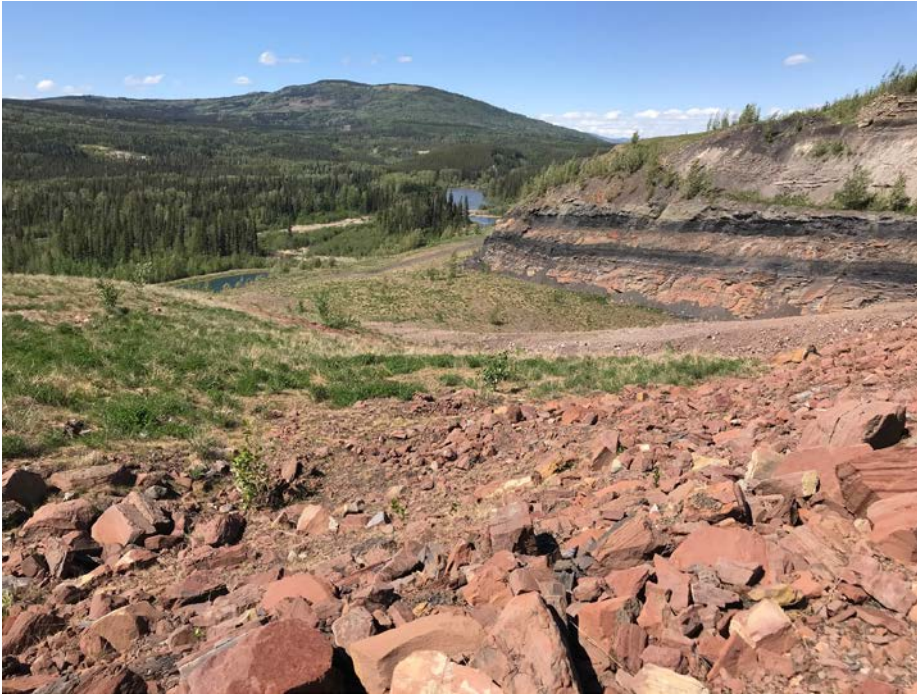
Photo I-4 Downstream slope taken from west abutment – looking northwest. Slope appears to be in good condition (SNTD-2018-02)
