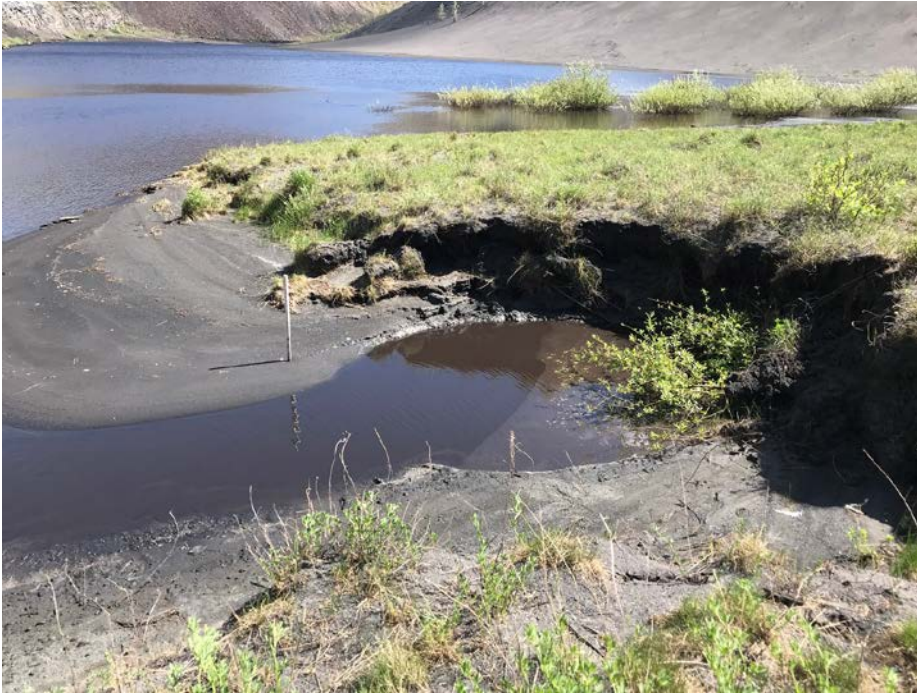
Photo I-13 Drainage channel inside the impoundment (SNTD-2018-06)
