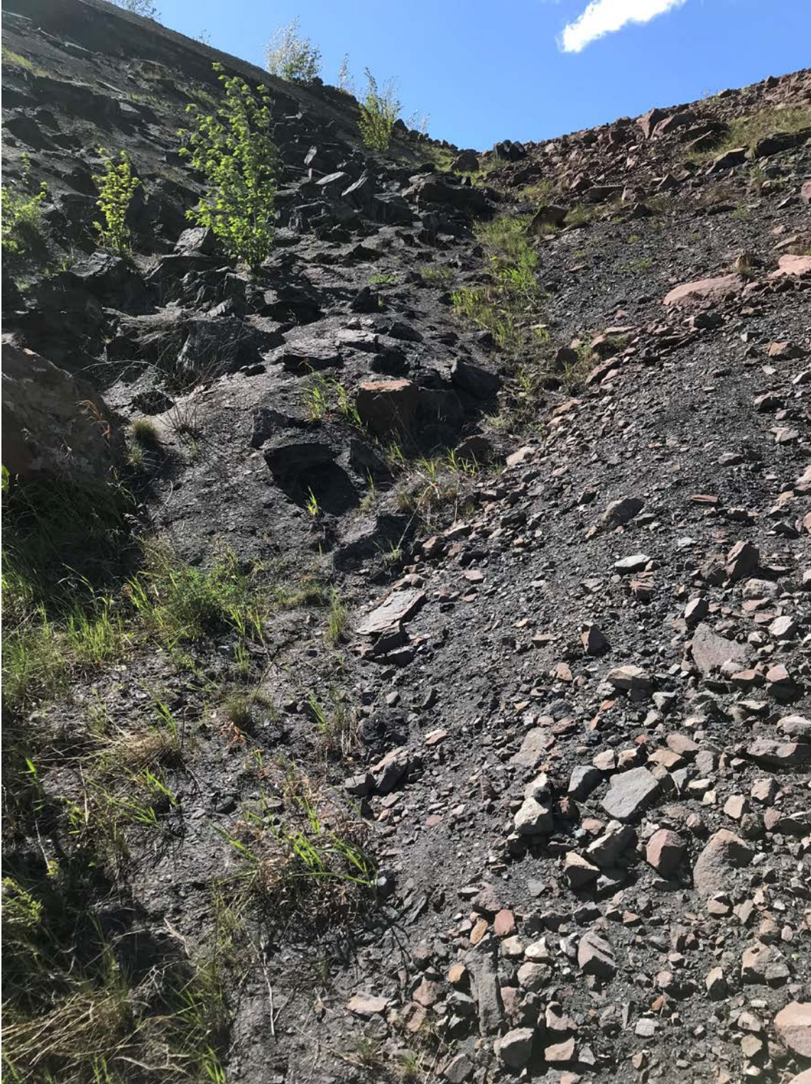
Photo I-23 SNTD west abutment - upstream contact with the Shikano pit west wall – small erosion gully noted but appears to be unchanged from 2017 condition (SNTD-2018-09)
