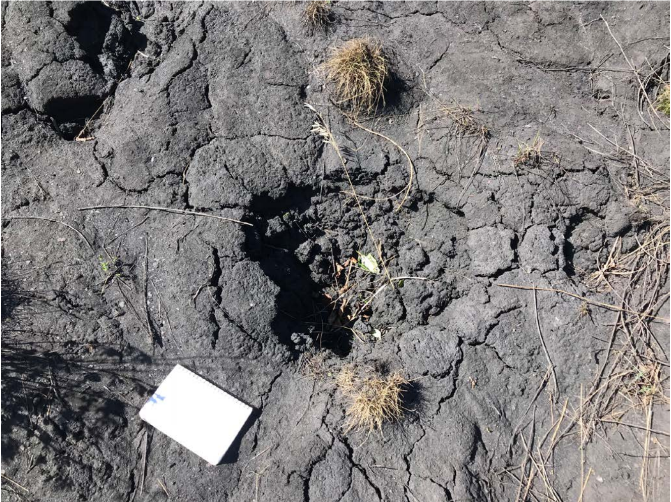
Photo I-22 Sinkholes 7 to 10 - typical smaller sinkholes noted along the southern half of the tailings beach (between SNTD-2018-07 and SNTD-2018-08)
