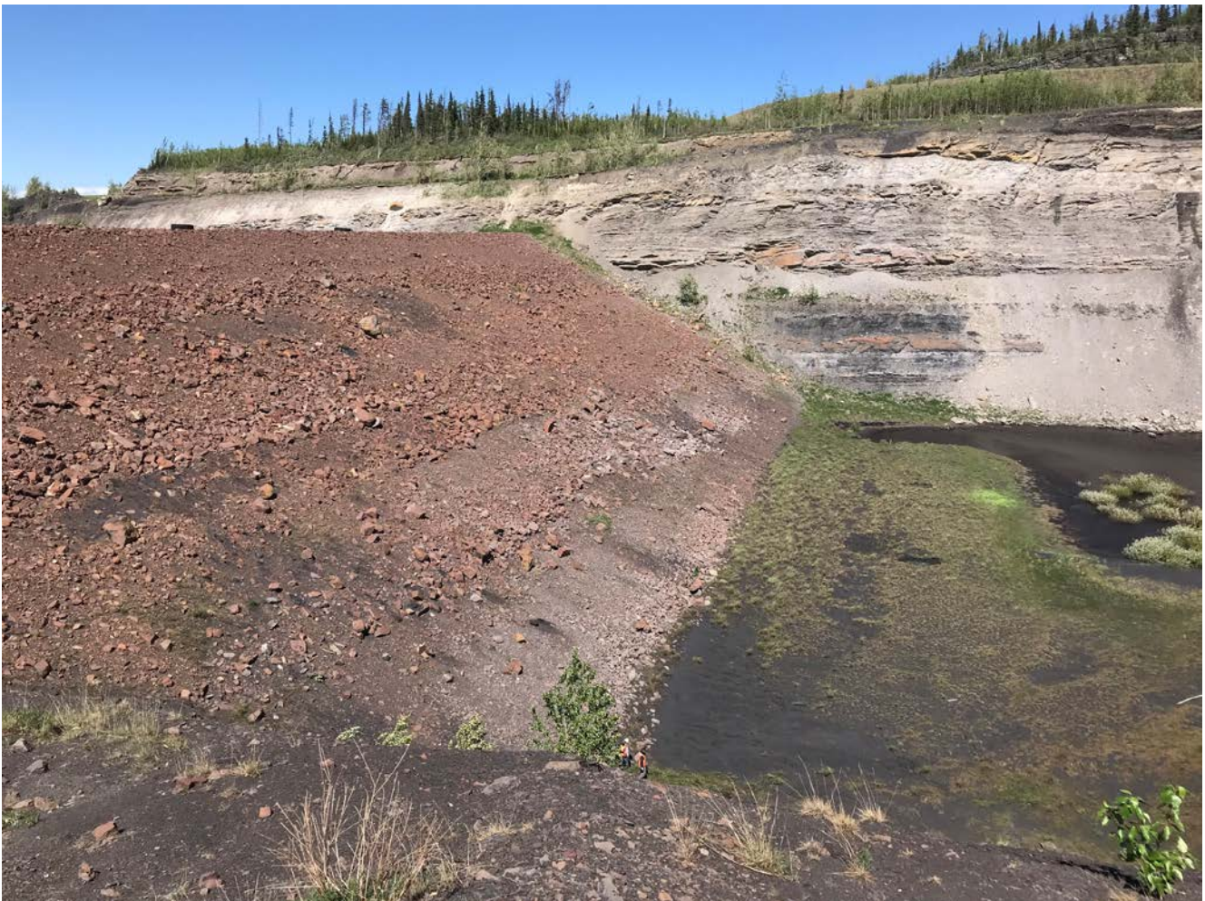
Photo I-1 Upstream slope taken from the west abutment – looking northeast. Slope appears to be in good condition with no signs of erosion or movement (SNTD-2018-01)
