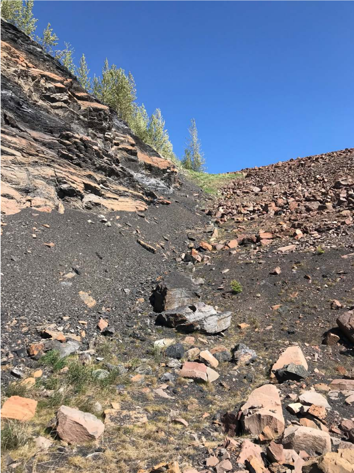
Photo I-26 Downstream contact with east abutment – looking east. No changes in condition from previous year (SNTD-2018-12)
