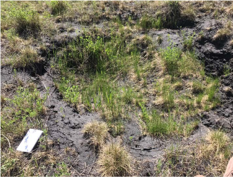
Photo I-15 Sinkhole 2 – approximately 3.2 m x 3.0 m x 0.6 m deep (SNTD-SINKHOLE-02)
