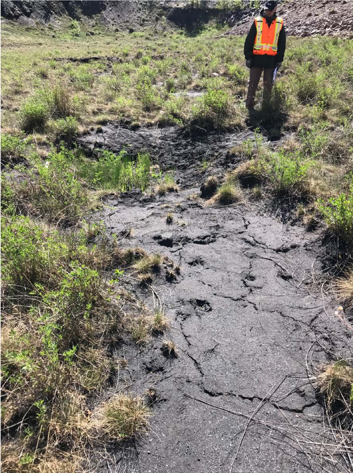
Photo I-17 Sinkhole 3 – settled tailings surface immediately adjacent to Sinkhole 3, indicating Sinkhole 3 may be increasing in size (SNTD-SINKHOLE-03)
