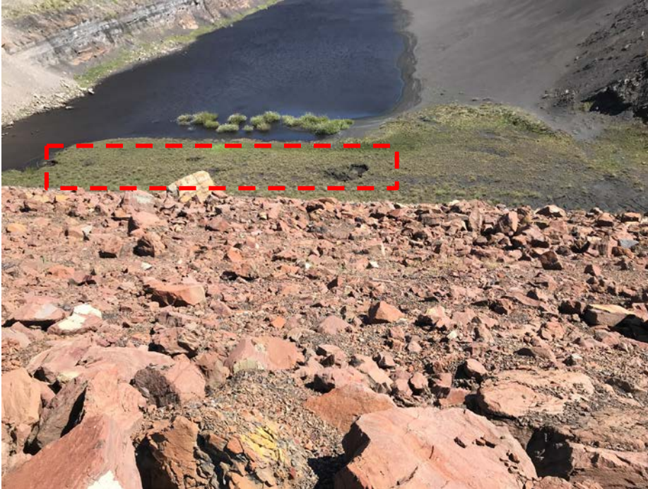
Photo I-8 Upstream slope taken from mid-length of the crest – slope appears to be in good condition. General area where sinkholes are observed is shown in red box (SNTD-2018-03)
