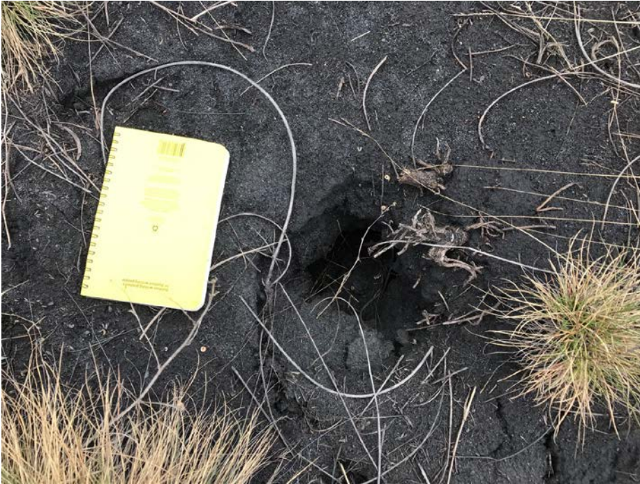
Photo I-18 Sinkhole 4 – first observed in 2017. Approximately 0.2 m x 0.1 m x 0.3 m deep (SNTD-SINKHOLE-04)
