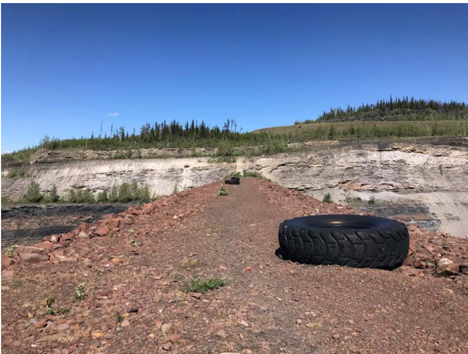
Photo I-3 Dam crest from east abutment – looking northwest. No signs of dam safety issues (e.g., sinkholes, cracks, settlement, etc.) (SNTD-2018-02)
