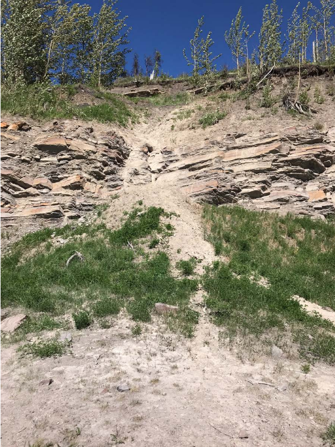
Photo I-10 East abutment – minor ravelling of material from slope above onto the crest – appears to be in similar condition as previous year’s (SNTD-2018-05)
