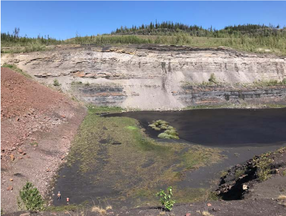
Photo I-2 North abutment – looking northeast. Pit wall erosion appears unchanged from 2017 condition (SNTD-2018-01)
