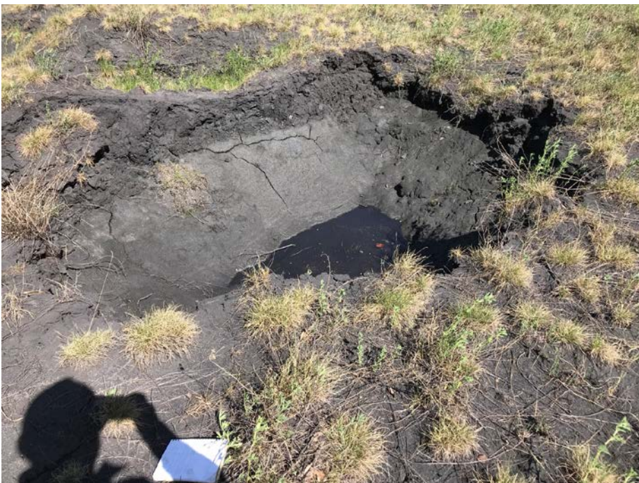
Photo I-21 Sinkhole 6 – water noted at the bottom of one of the sinkholes (SNTD-SINKHOLE-06)
