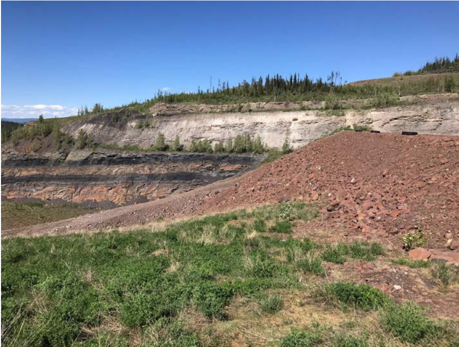
Photo I-24 Downstream slope taken from west abutment – looking north; no signs of erosion or movement (SNTD-2018-10)
