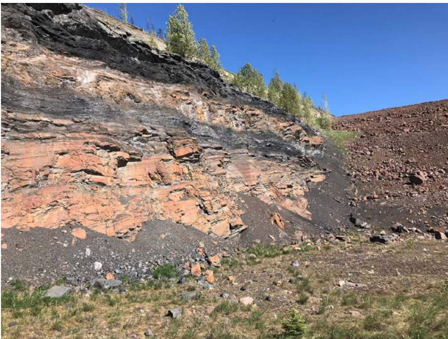
Photo I-25 Downstream east abutment – looking east. No changes in condition when compared to 2017 observation (SNTD-2018-11)
