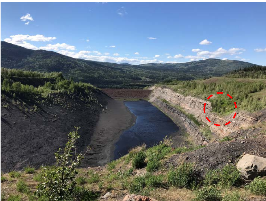
Photo I-30 Shikano North Tailings Dam – looking northwest. Historic slumping failure circled with red dash line. No significant changes since 2012 (SNTD-2018-16)
