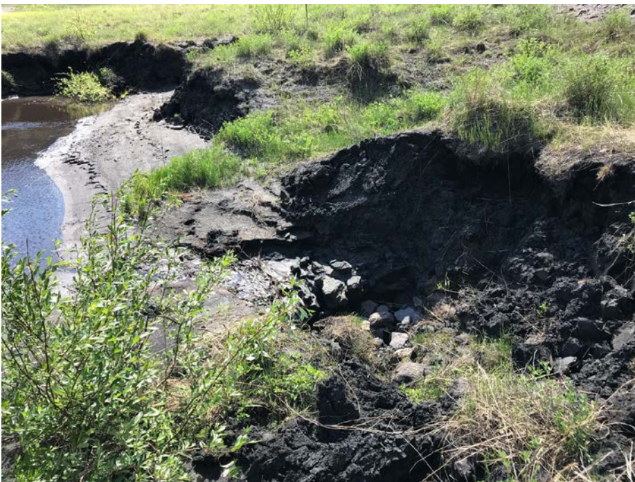
Photo I-12 Sinkhole 11 – first observed in 2018. Approximately 5.0 m x 3.0 m x 1.0 m deep. Flow of water into the underlying rockfill was observed – not a dam safety concern (SNTD-SINKHOLE-11)
