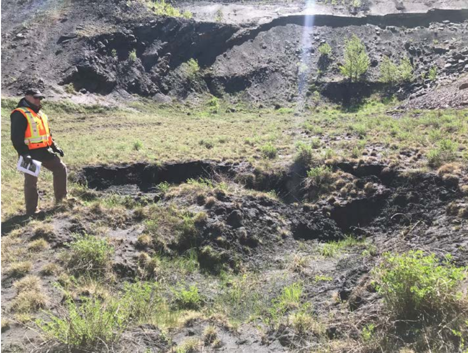
Photo I-20 Sinkhole 6 used to be a cluster of three sinkholes up to 2017. In 2018, all three sinkholes have developed into one large sinkhole approximately 9.4 m x 7.4 m x 0.5 m deep (SNTD-SINKHOLE-06)
