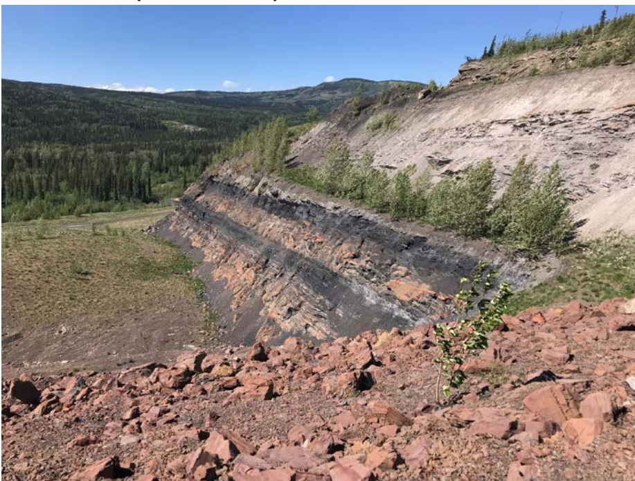
Photo I-9 Downstream slope taken from the east abutment – looking northwest. Slope appears to be in good condition with no signs of erosion or movement (SNTD-2018-04)
