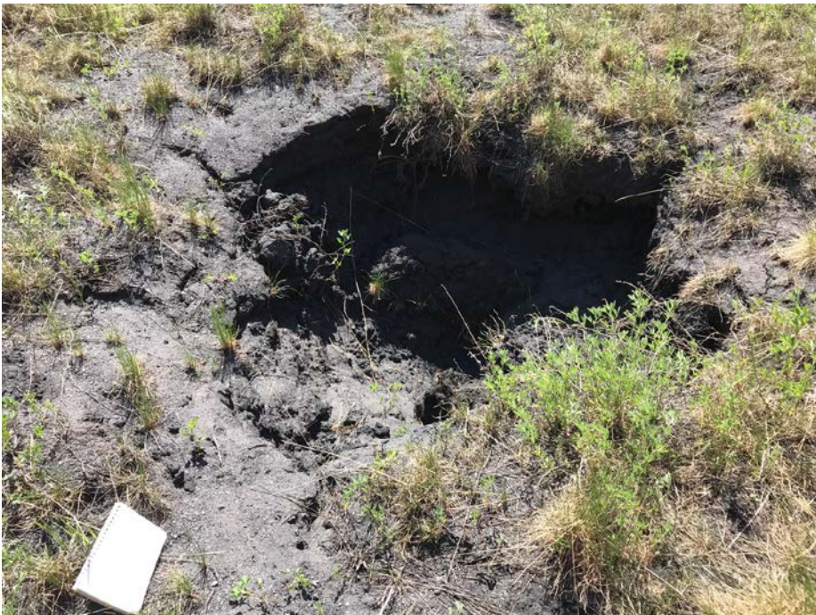
Photo I-14 Sinkhole 1 – first observed in 2016. Approximately 1.9 m x 1.7 m x 1.0 m deep (SNTD-SINKHOLE-01)
