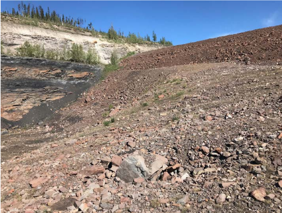
Photo I-27 Downstream, access ramp and downstream slope – looking north. No significant signs of erosion or movement (SNTD-2018-13)
