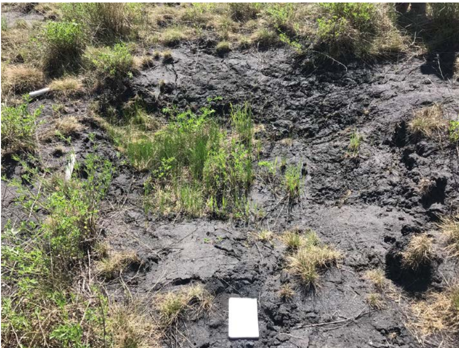
Photo I-16 Sinkhole 3 – approximately 3.0 m x 2.5 m x 0.6 m deep (SNTD-SINKHOLE-03)
