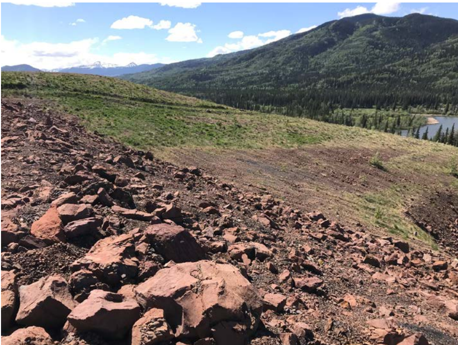
Photo I-5 Downstream slope and west abutment contact – looking west. No signs of erosion or movement (SNTD-2018-03)
