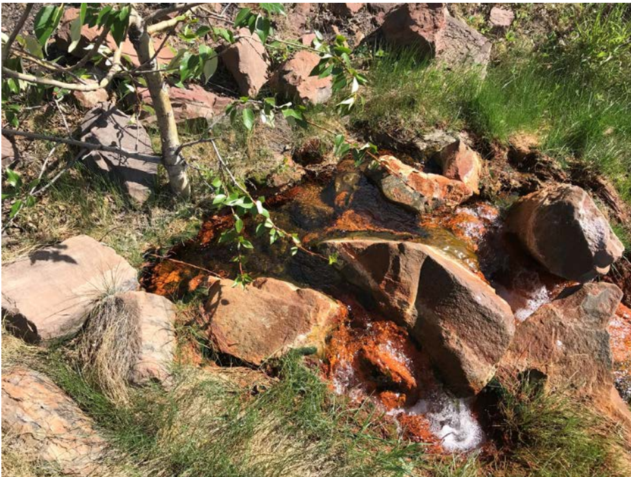
Photo I-28 Seepage from low level outlet downstream of the dam (SNTD-2018-14)
