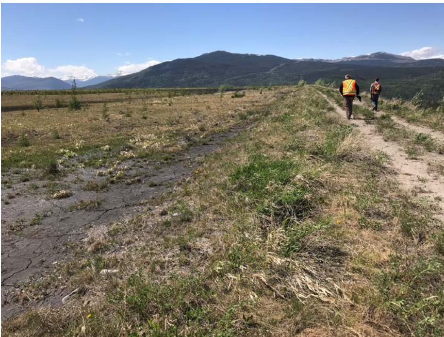
Photo I-34 Upstream slope and tailings beach – no sinkholes or signs of distress. Tailings surface is less than 1 m below the crest; not a dam safety concern (PTD-2018-23)
