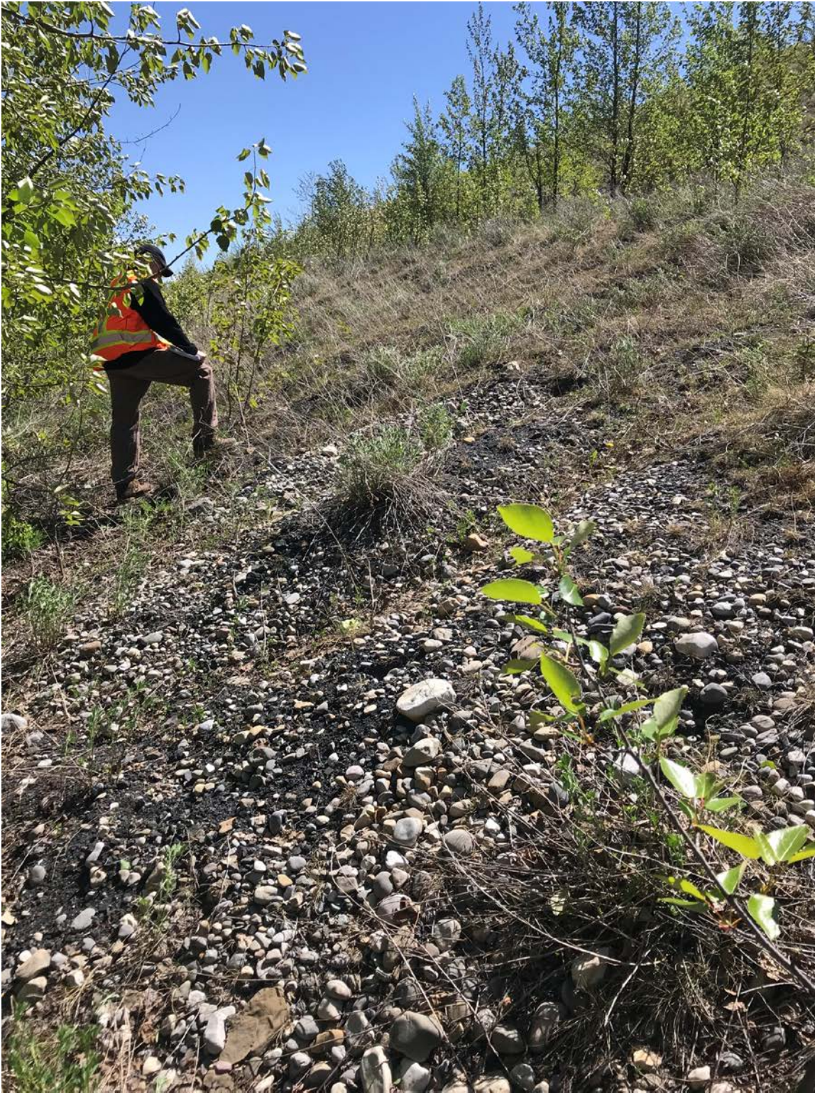
Photo I-24 Typical dry finger drain along the north embankment (PTD-DRAIN-23)
