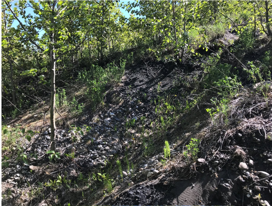
Photo I-10 Finger drain at PTD toe; area downstream of the finger drain is boggy and well vegetated (PTD-DRAIN-08/09)
