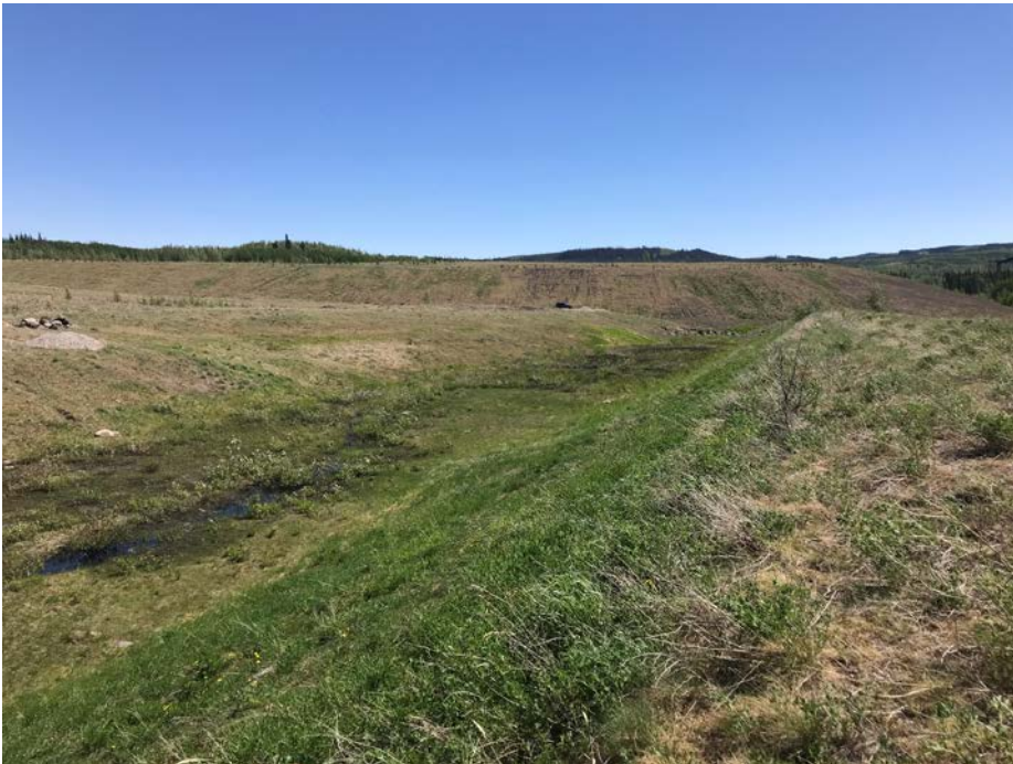
Photo I-48 Spillway channel - viewed from the embankment looking east along the channel – channel is well vegetated but no obstruction observed (PTD-2018-35)
