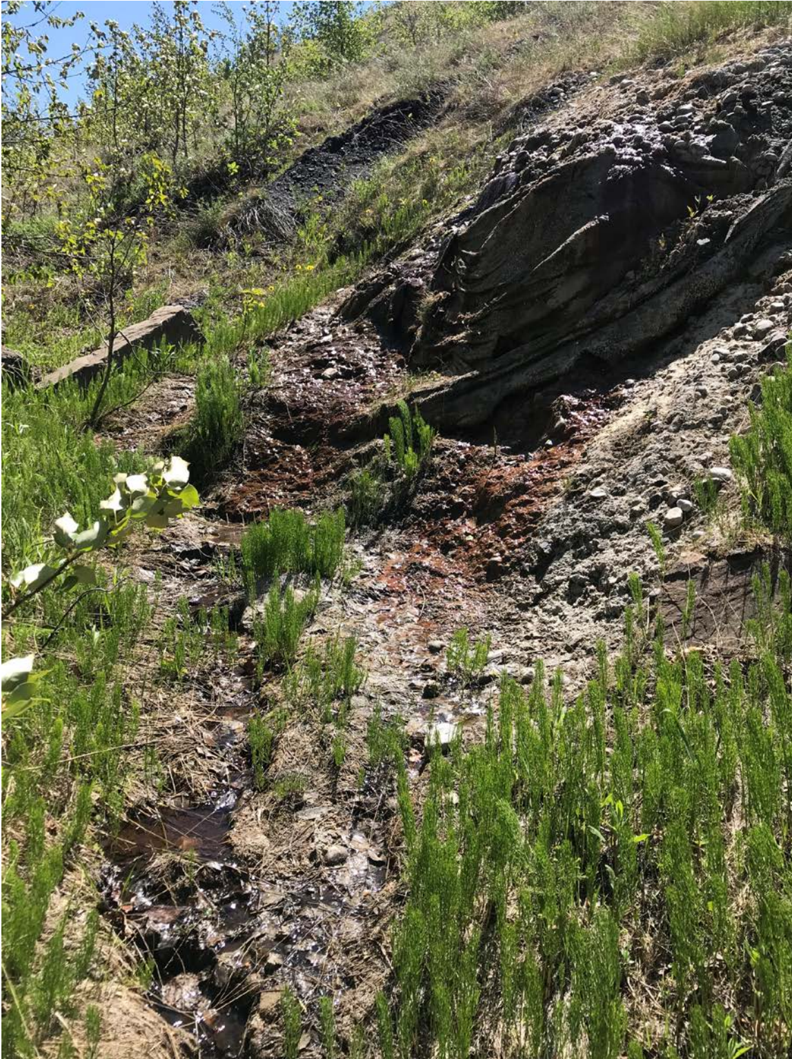
Photo I-23 Finger drain with geotextile – red (oxidized iron) precipitate observed (PTD-DRAIN-22)
