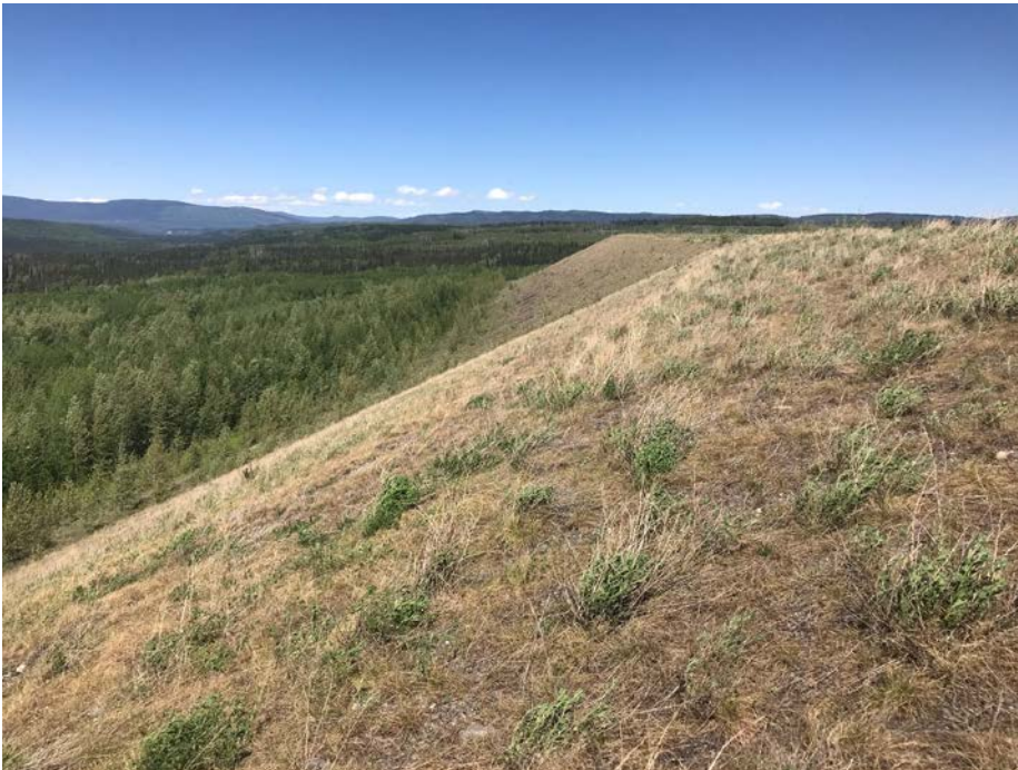
Photo I-42 Overview of the downstream slope from the dam crest near Sta. 0+900 – looking north. No signs of distress, significant movement (PTD-2018-29)
