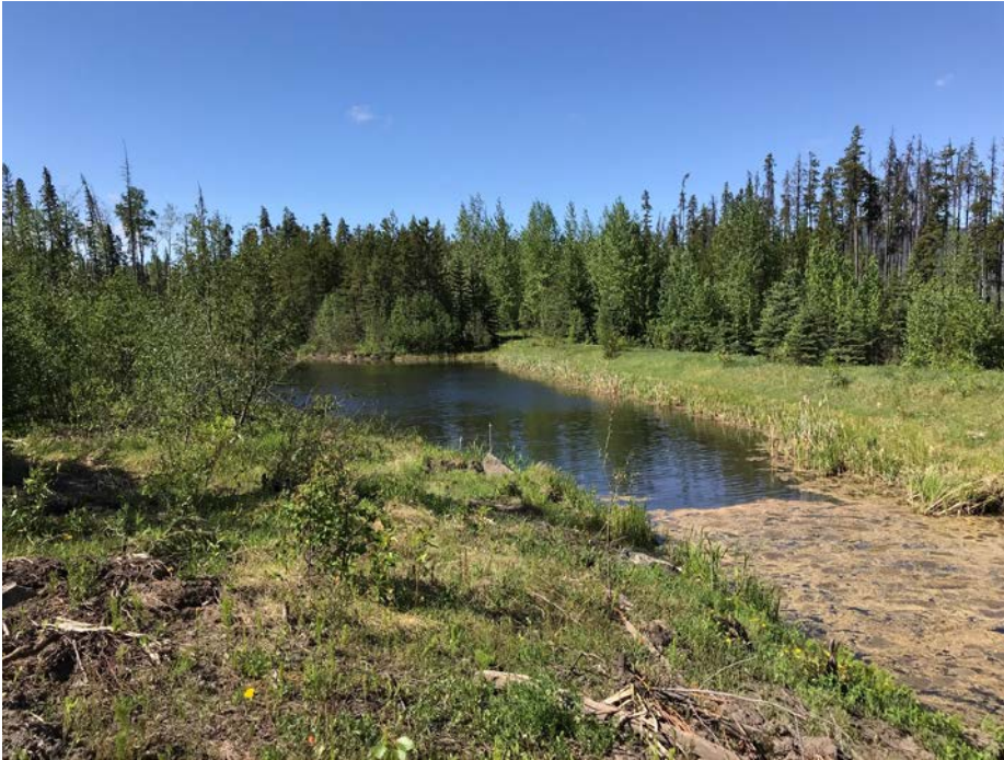
Photo I-12 PTD Seepage Collection Pond – looking west. Beaver dam noted obstructing the outlet area of the pond (PTD-2018-09)
