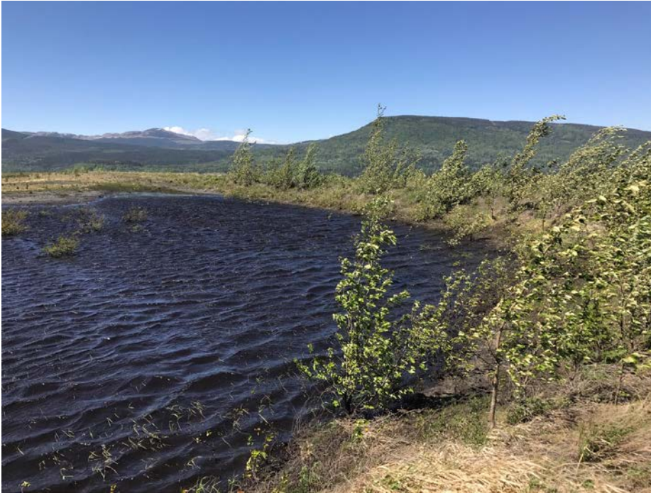
Photo I-32 Upstream slope and tailings beach – looking west. No sinkholes or signs of distress – looking west (PTD-2018-22)
