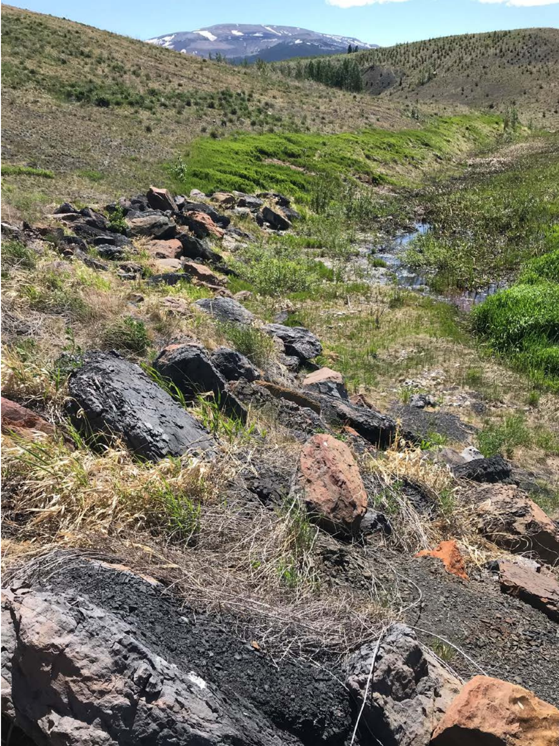
Photo I-51 Standing on the spillway channel slope looking south at deteriorating riprap and ponded area inside local depressions inside the channel (PTD-2018-38)
