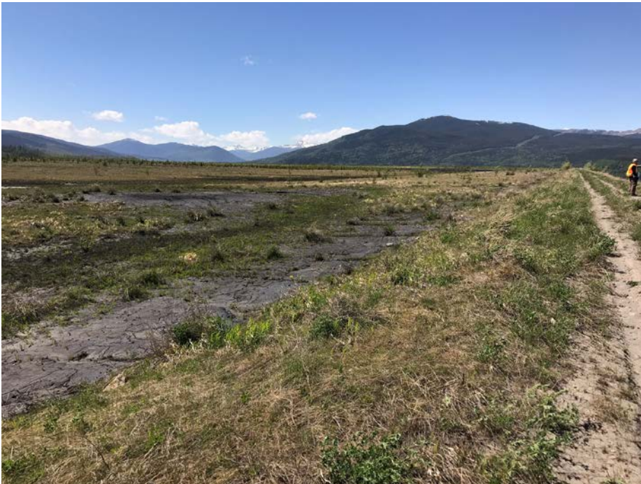
Photo I-32 Upstream slope and tailings beach – looking west. No sinkholes or signs of distress – looking west (PTD-2018-22)
