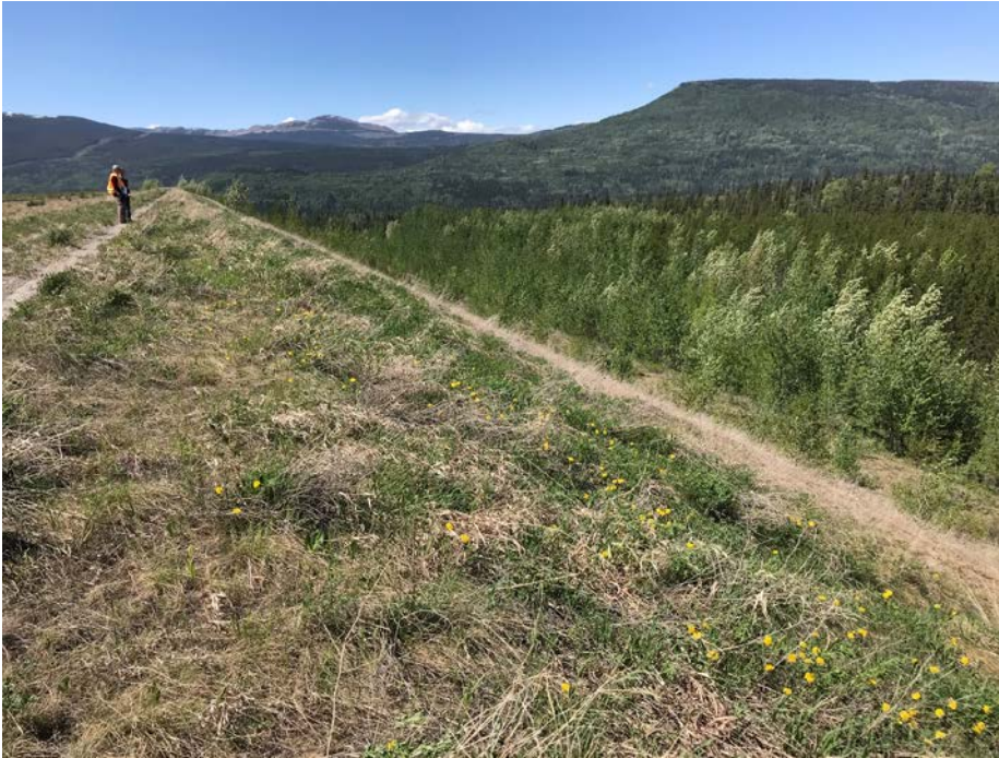
Photo I-33 Downstream slope of the PTD - looking west at approximately Sta. 2+100. No signs of displacement or deformation (PTD-2018-22)
