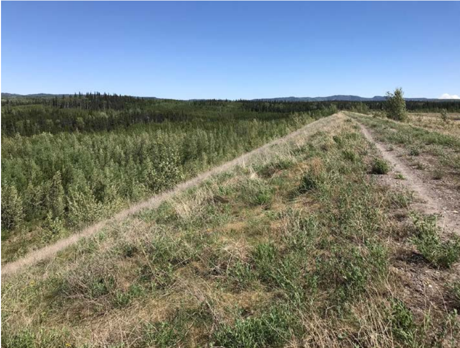
Photo I-39 Overview of the downstream slope from the dam crest near Sta. 1+640 – looking east. No signs of distress, significant movement or erosion (PTD-2018-26)
