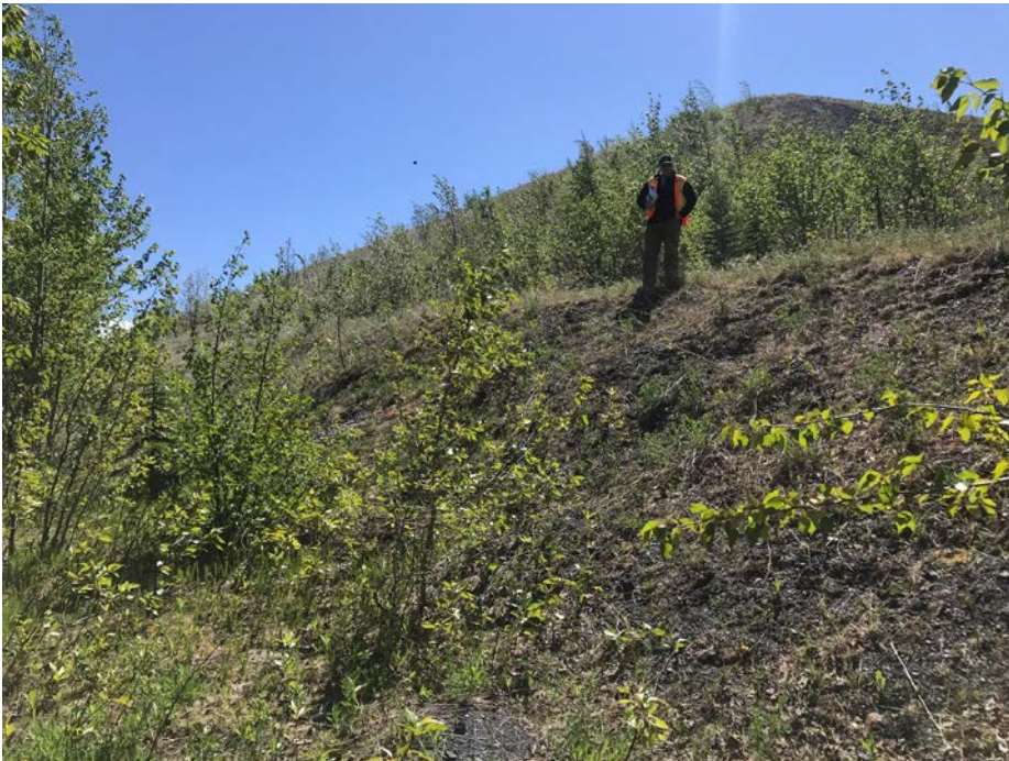
Photo I-22 Overview of PTD northwest corner - steep scarp near downstream slope ramp – inactive due to the amount of vegetation growth on scarp (PTD-2018-16)
