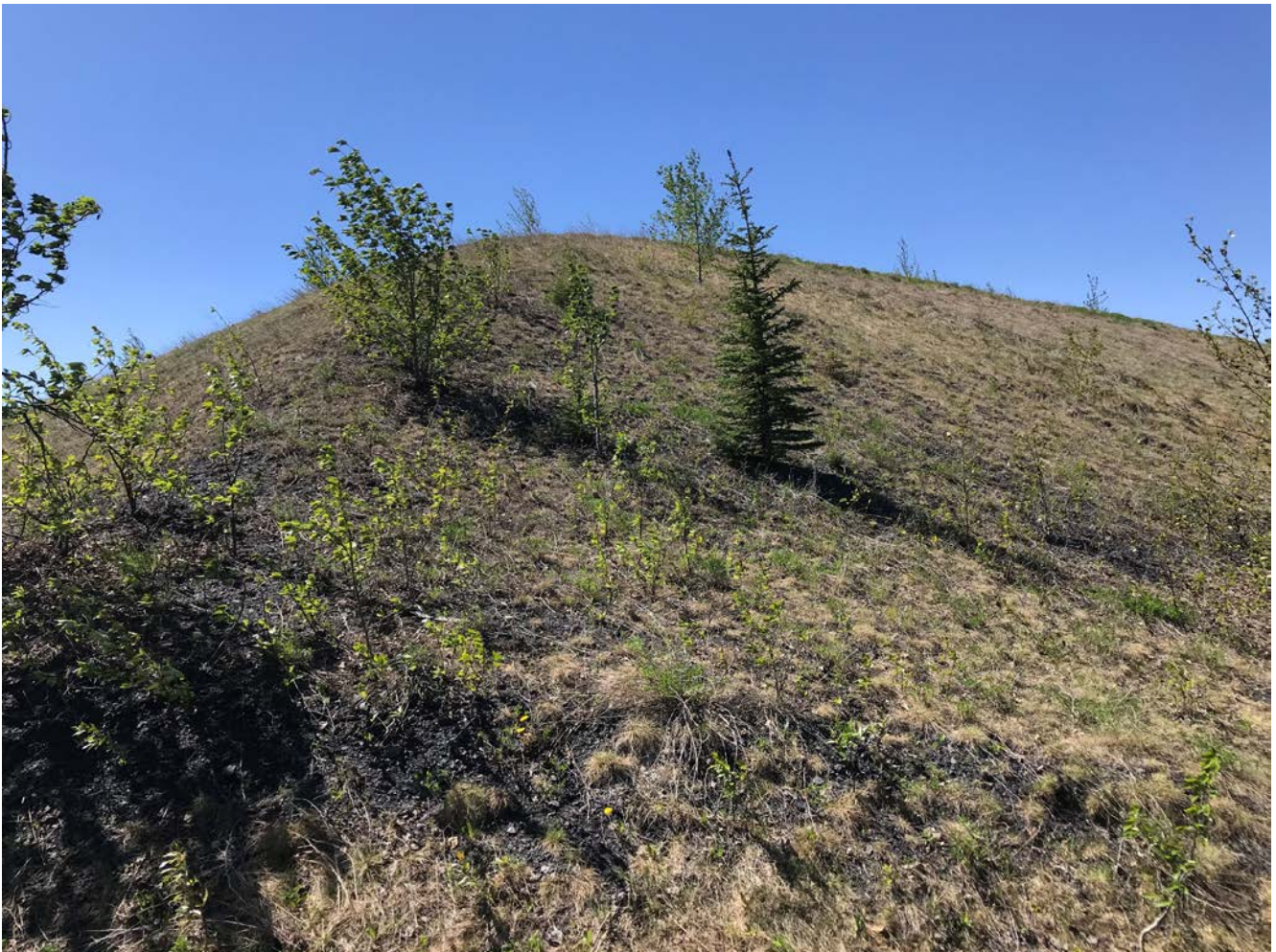
Photo I-25 PTD northeast corner's downstream slope – no signs of distress (PTD-2018-17)
