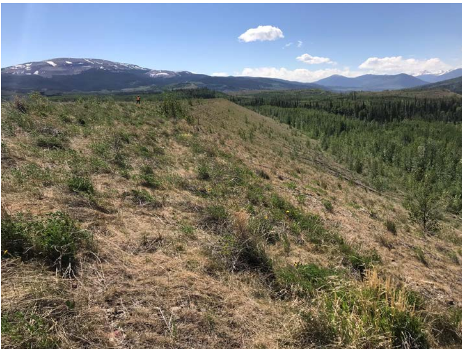
Photo I-40 Overview of the downstream slope from the dam crest near Sta. 1+230 – looking south. No signs of distress, significant movement or erosion (PTD-2018-27)
