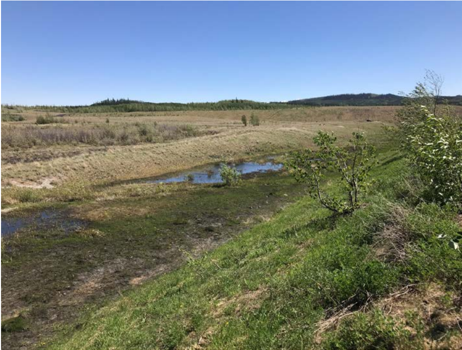
Photo I-48 Spillway channel - viewed from the embankment looking east along the channel – channel is well vegetated but no obstruction observed (PTD-2018-35)
