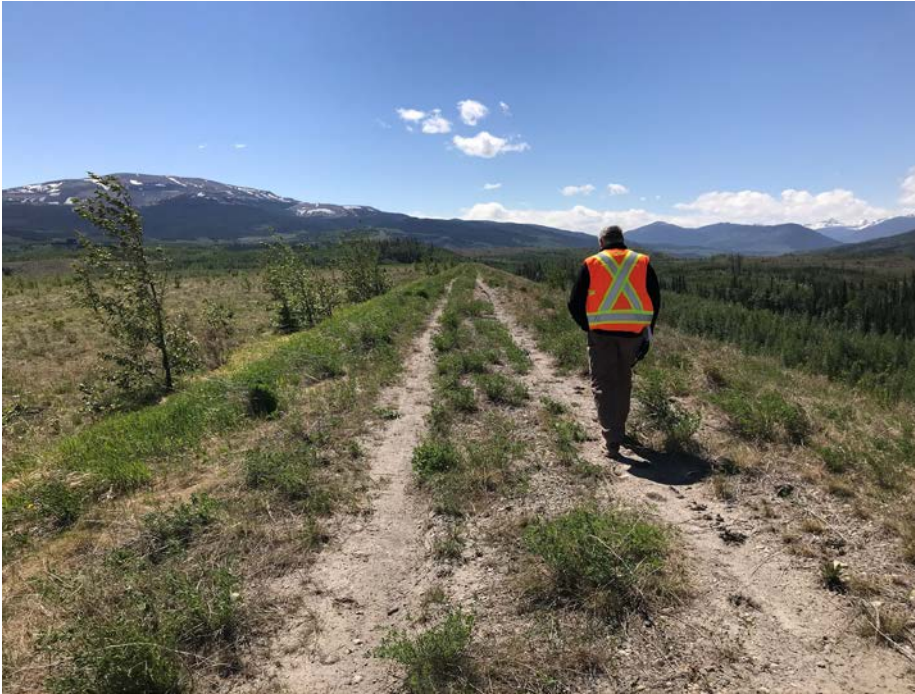
Photo I-42 Overview of the downstream slope from the dam crest near Sta. 0+900 – looking north. No signs of distress, significant movement (PTD-2018-29)
