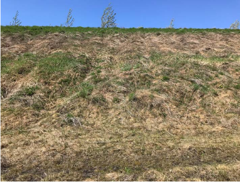
Photo I-28 Small sloughed area on the dam's downstream slope – looking south. The feature is likely caused by animal activity (PTD-2018-19)
