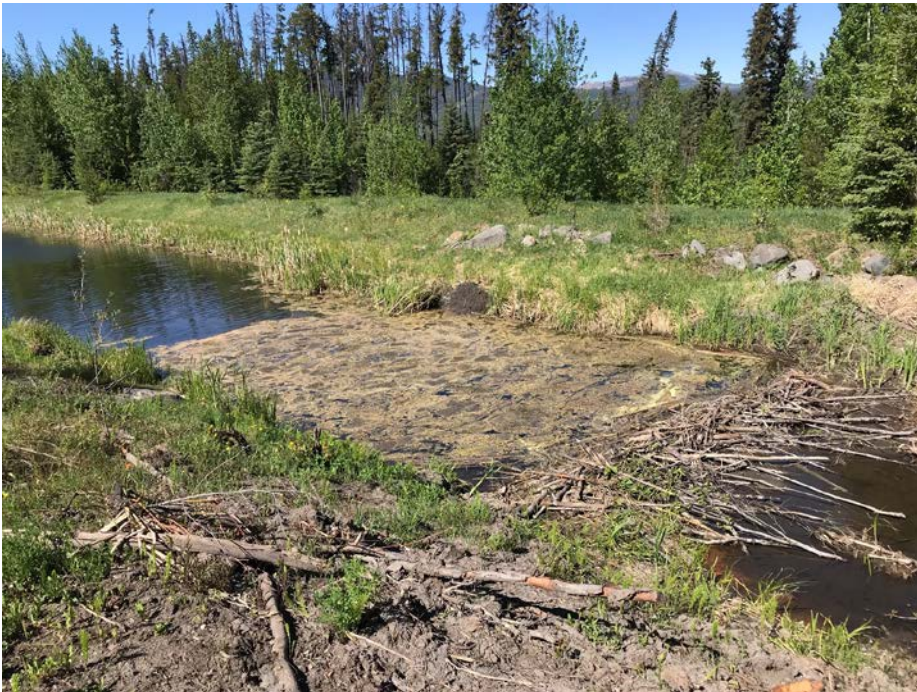
Photo I-12 PTD Seepage Collection Pond – looking west. Beaver dam noted obstructing the outlet area of the pond (PTD-2018-09)
