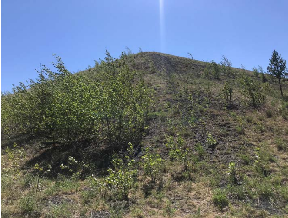
Photo I-22 Overview of PTD northwest corner - steep scarp near downstream slope ramp – inactive due to the amount of vegetation growth on scarp (PTD-2018-16)
