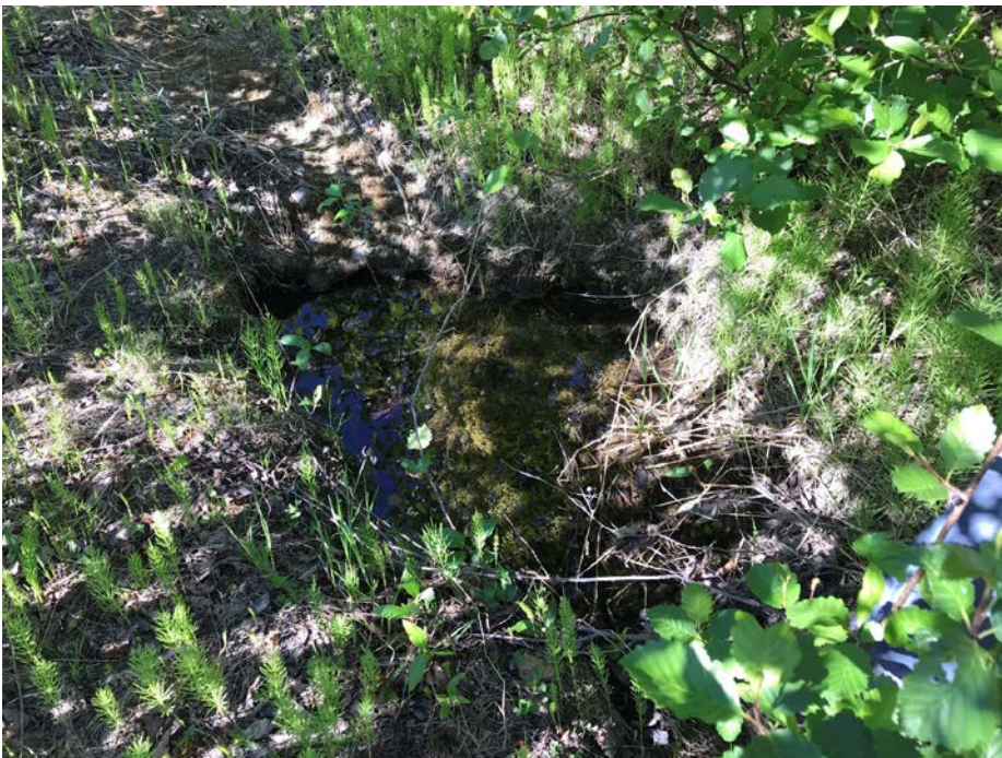
Photo I-9 Small sinkhole located downstream of the dam's toe – suspected to be collapsed animal burrow (PTD-2018-08)
