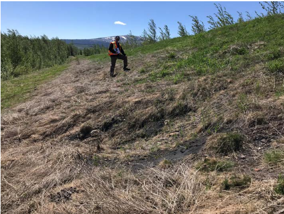
Photo I-28 Small sloughed area on the dam's downstream slope – looking south. The feature is likely caused by animal activity (PTD-2018-19)
