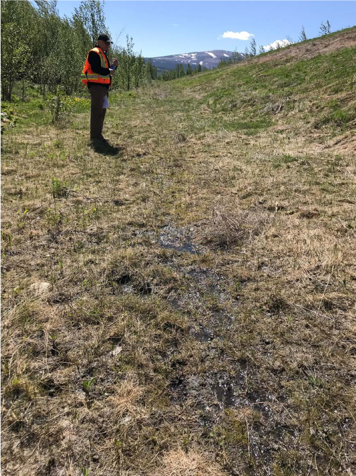
Photo I-26 PTD east embankment downstream toe area – looking south. Wet ground noted and likely due to seepage (PTD-2018-18)
