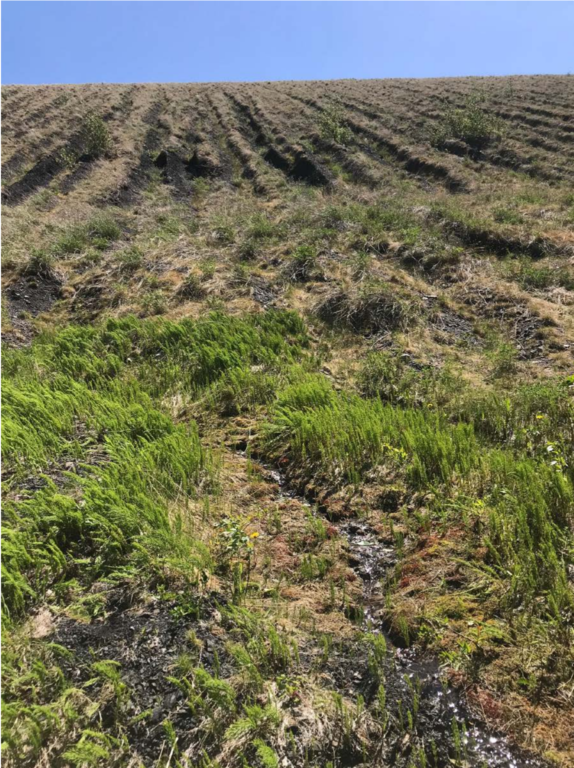
Photo I-20 Flow noted coming from a finger drain (Chanel 2) – flow was estimated 1 L/min (PTD-DRAIN-19)
