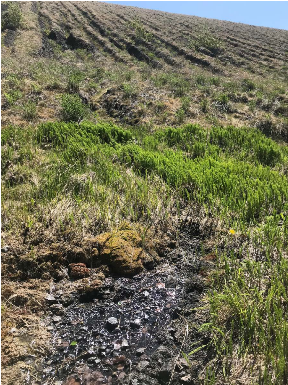
Photo I-19 Flow noted coming from downstream toe adjacent to a finger drain (Chanel 1) - flow was estimated 1 L/min (PTD-DRAIN-19)
