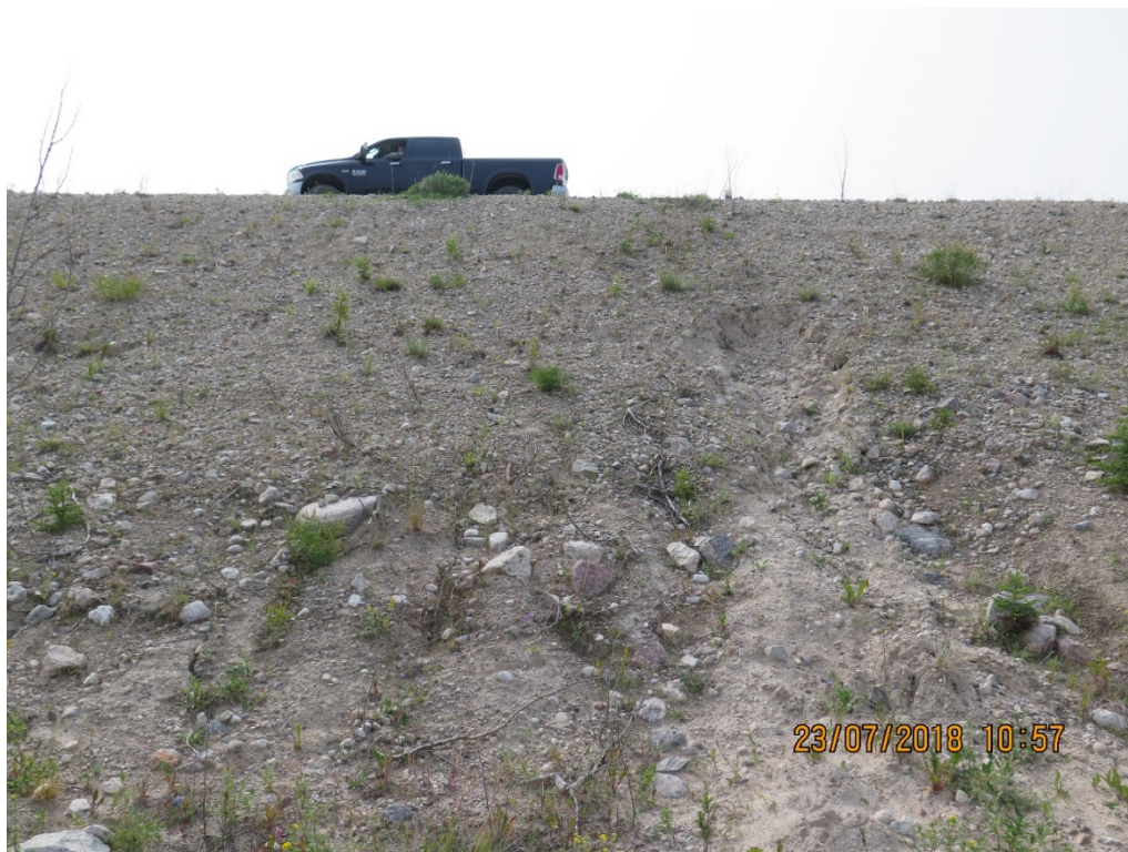
Photograph 9: North Dyke – Erosion Feature on Downstream Slope Near West End, Looking South. 23 July 2018
