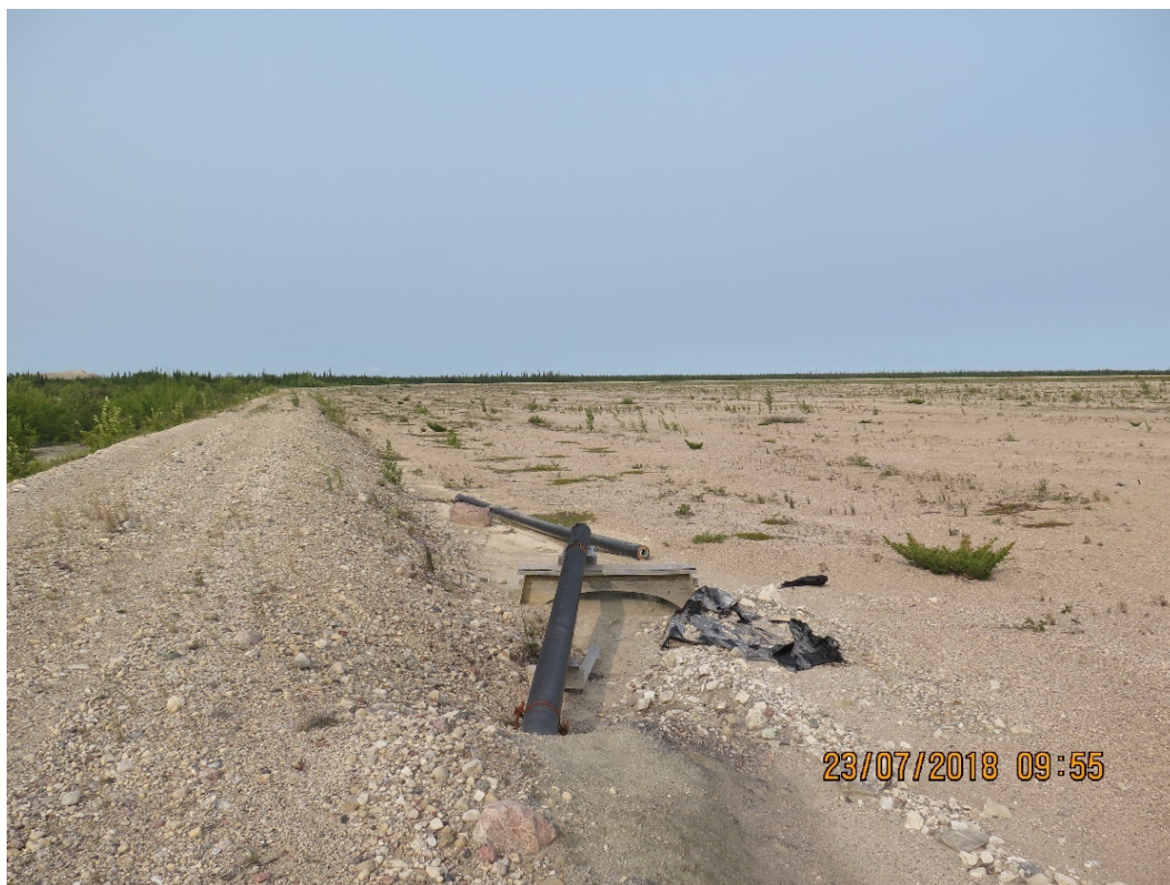
Photograph 2: South Dyke – Upstream Face of Central Portion, Looking West. 23 July 2018
