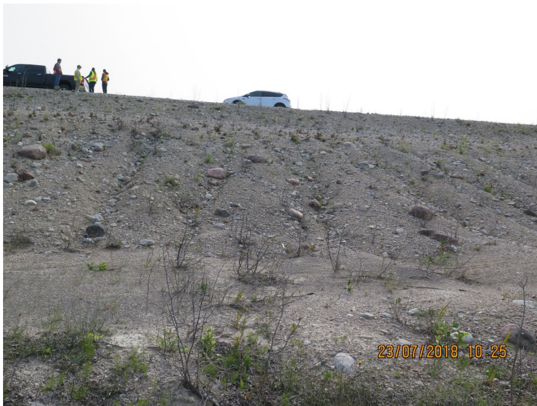
Photograph 7: West Dyke – Downstream Toe and Slope Near North End, Looking East, Minor Erosion Features. 23 July 2018
