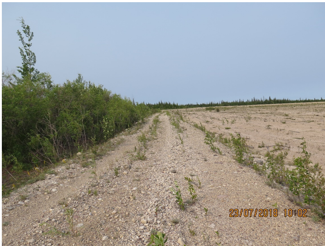
Photograph 3: South Dyke – Crest at West End with Vegetation on Downstream Face, Looking West. 23 July 2018
