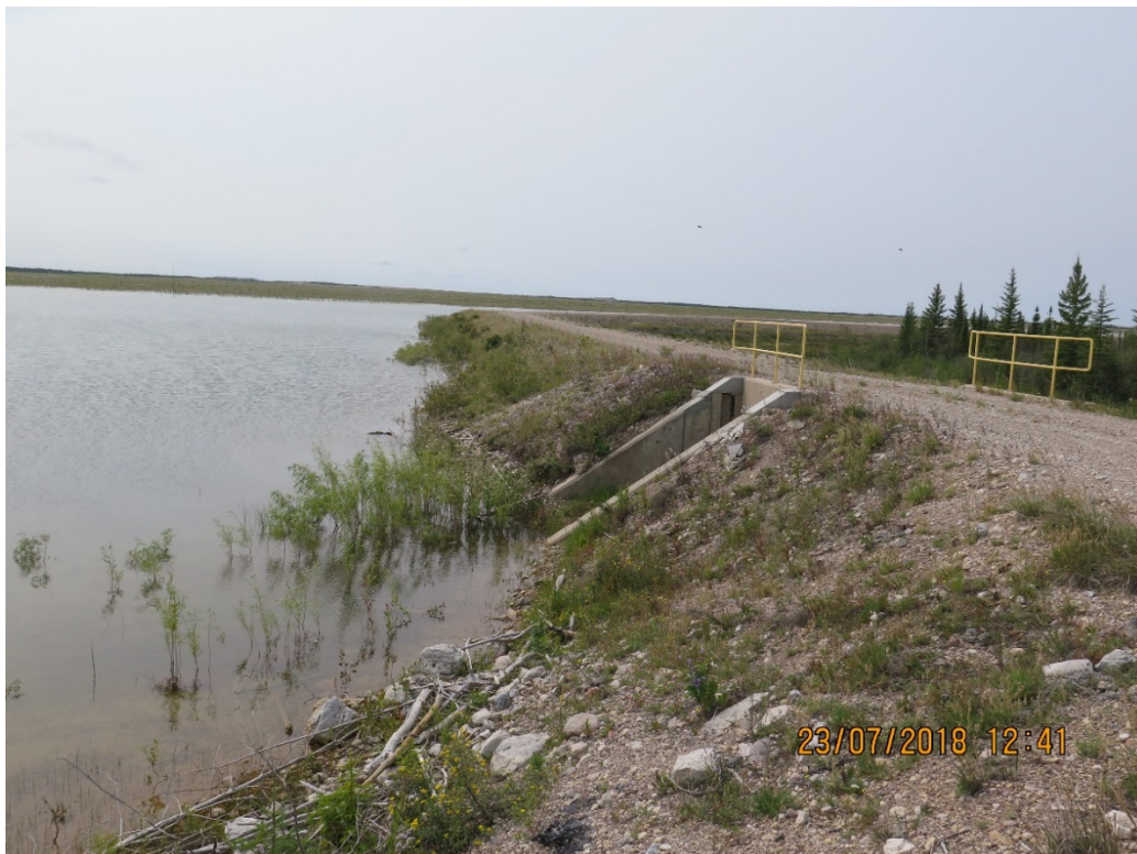
Photograph 14: Main Pond Spillway – Upstream Entry (Spillway No. 1), Looking South. 23 July 2018
