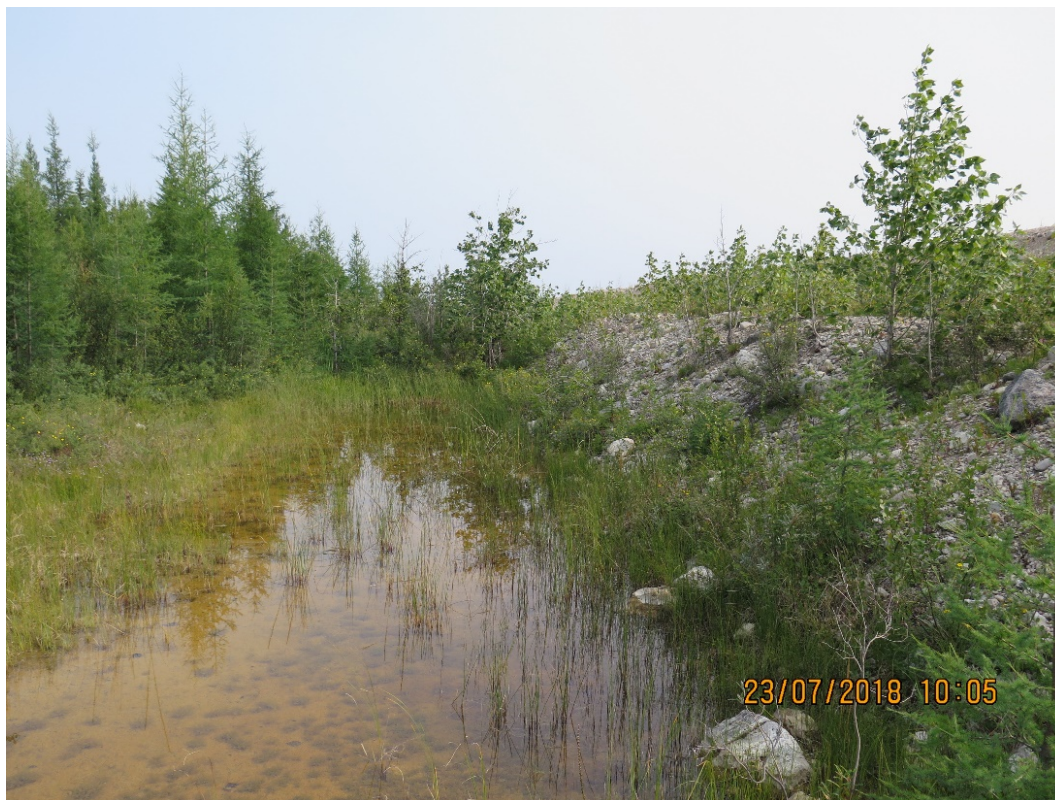
Photograph 5: West Dyke – Downstream Toe at South End, Looking North. 23 July 2018
