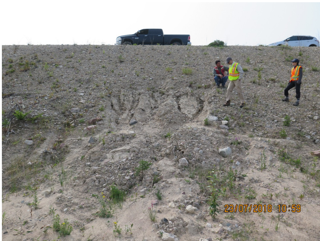
Photograph 10: North Dyke – Erosion Feature on Downstream Slope Near West End, Looking South. 23 July 2018
