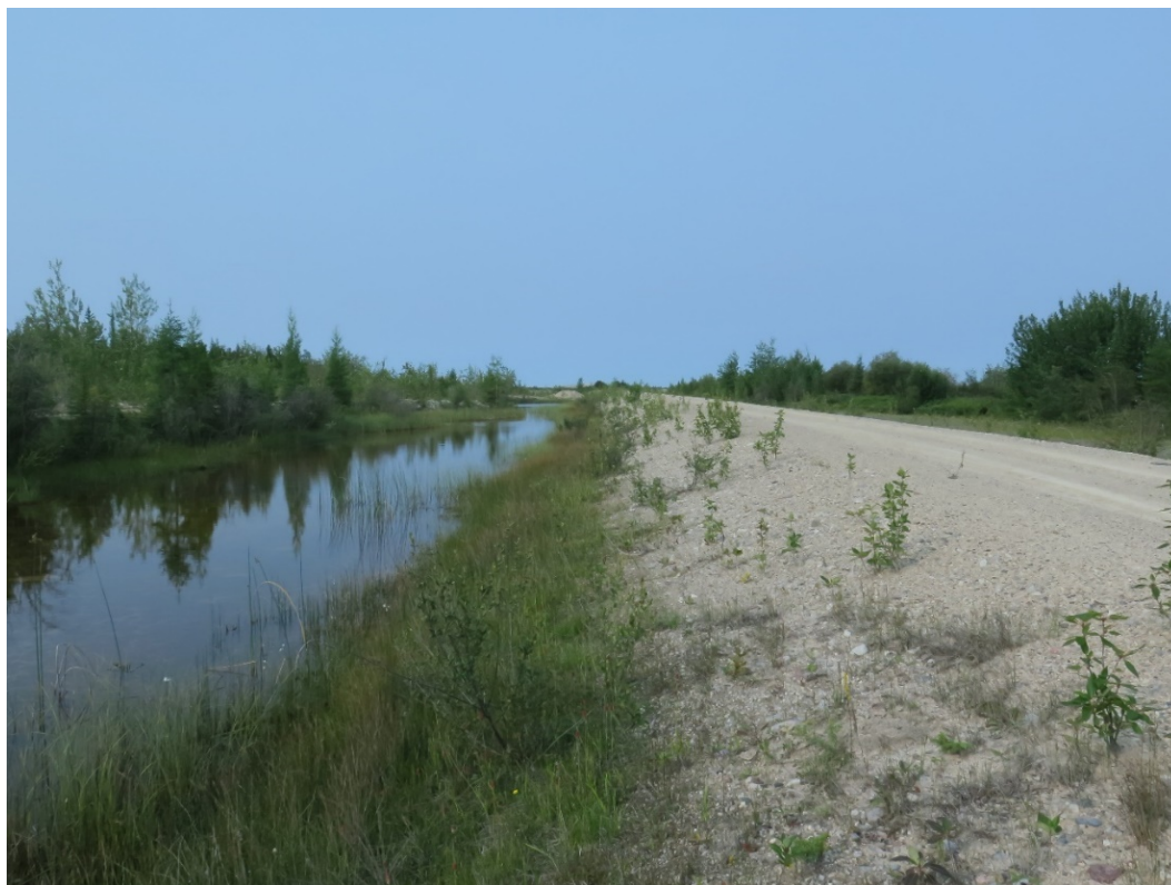
Photograph 1: South Dyke – Downstream Face at East End, Looking Southwest. 23 July 2018
