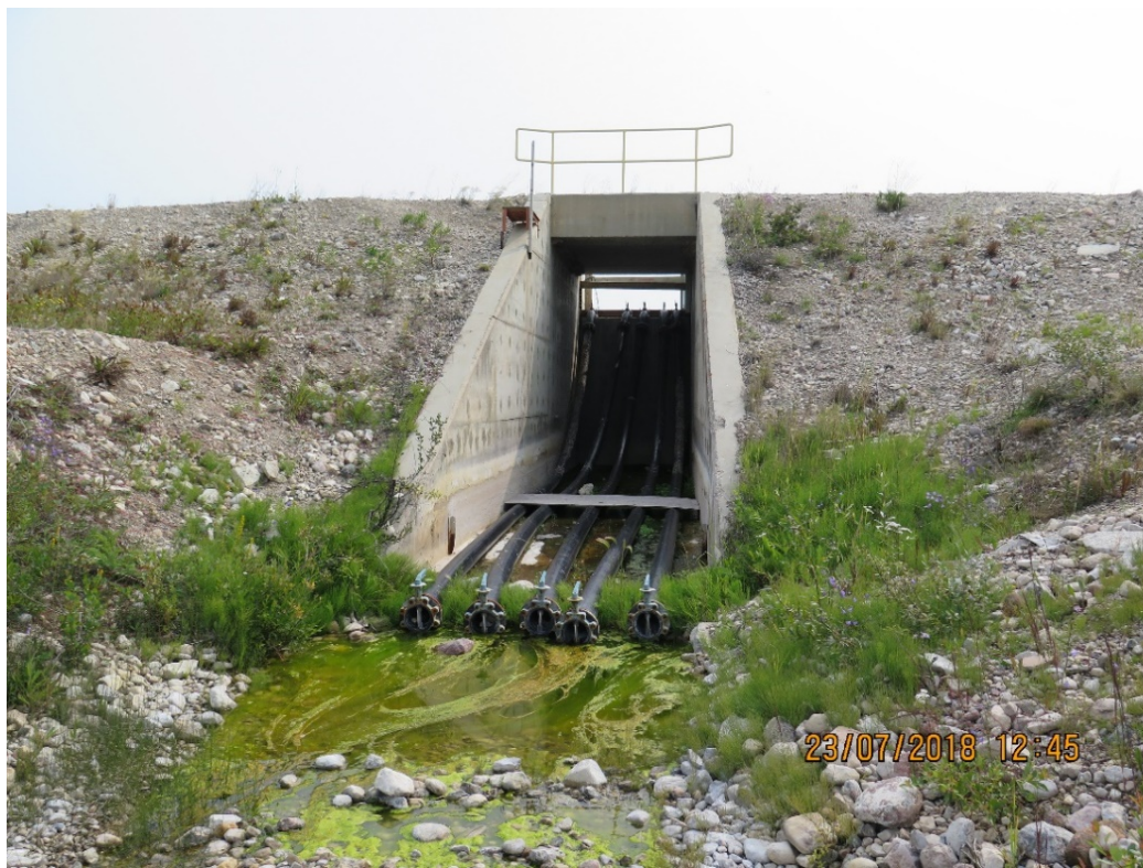
Photograph 15: Polishing Pond Spillway (Spillway No.2) Outlet, Looking East. 23 July 2018
