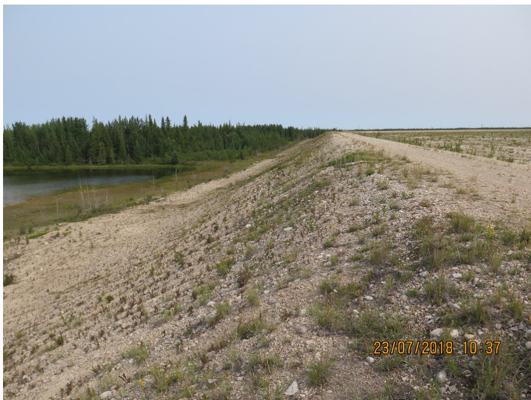
Photograph 8: North Dyke – Downstream Slope (left side of photo) Near West End, Looking East. 23 July 2018
