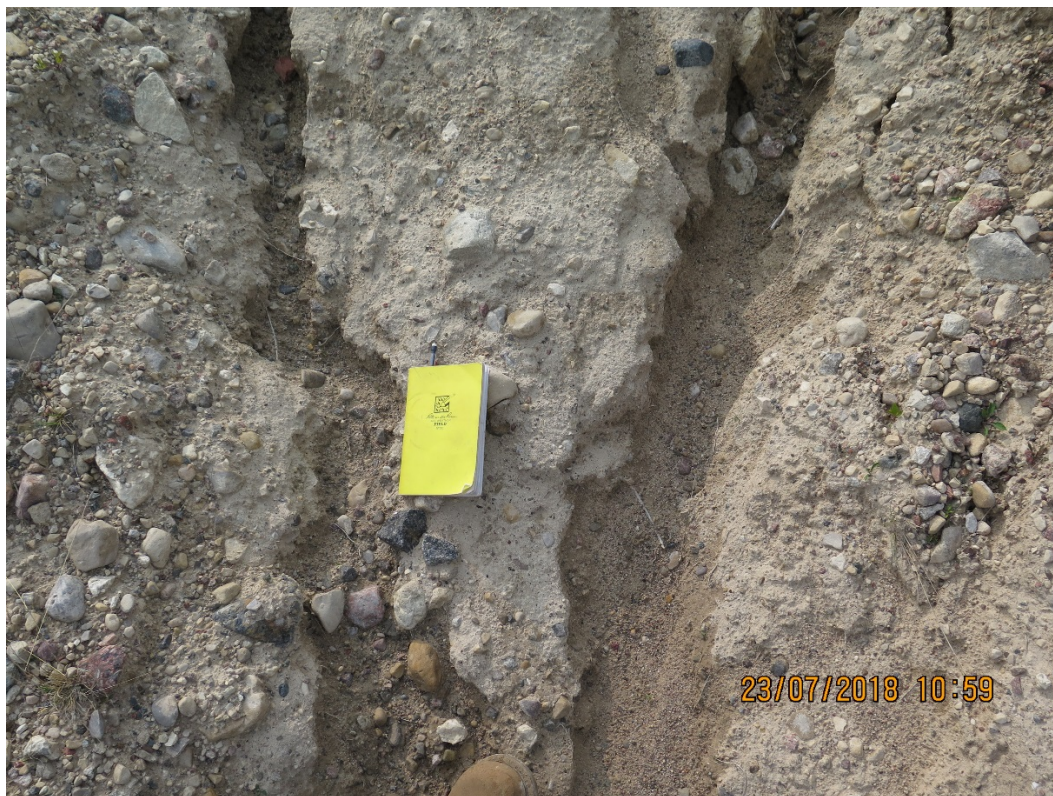
Photograph 11: North Dyke - Close Up of Erosion Feature on Downstream Slope Near West End, Looking South. 23 July 2018
