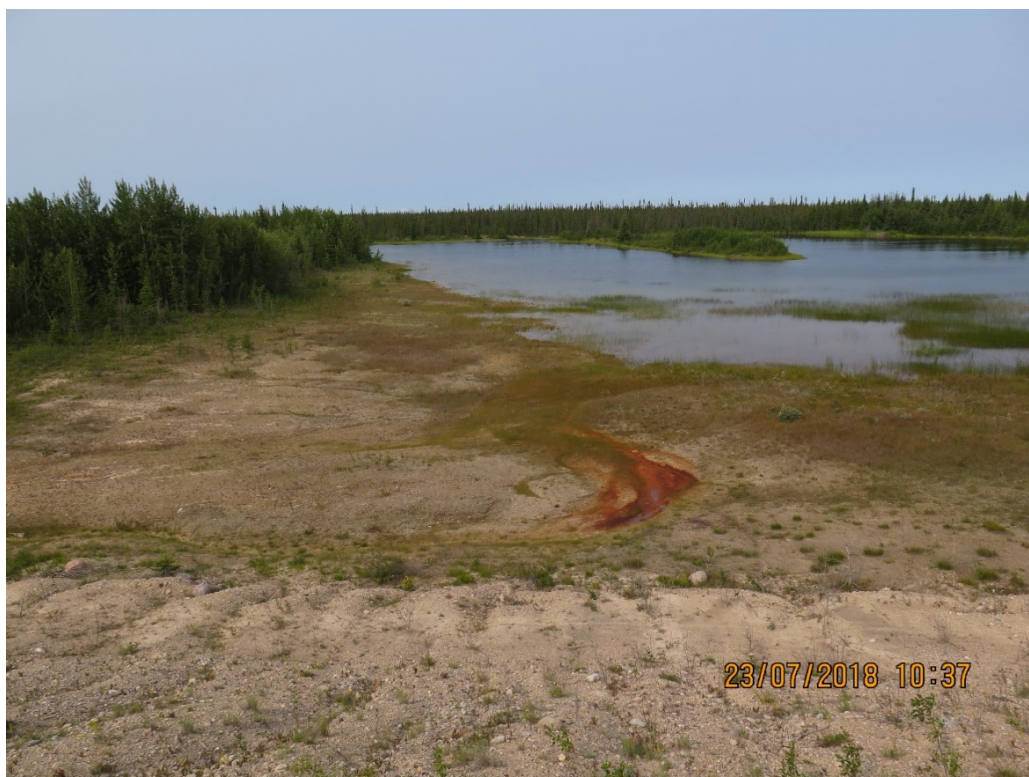
Photograph 6: West Dyke – Downstream Drainage Course near North End, Looking West, Staining Noted Near Seep. 23 July 2018
