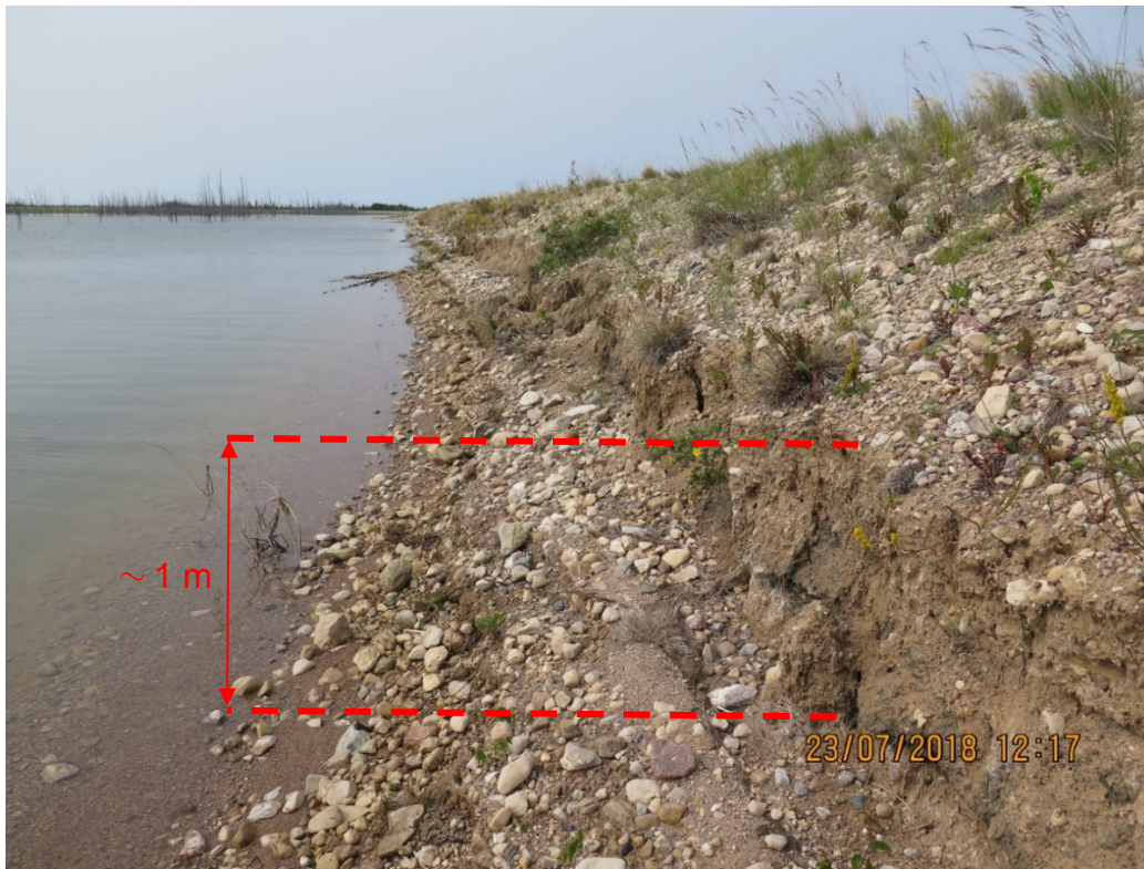
Photograph 13: North Dyke – Repair at Waterline on Upstream Face West of Dogleg, Erosion Approximately 1 m scarp, Looking West. 23 July 2018
