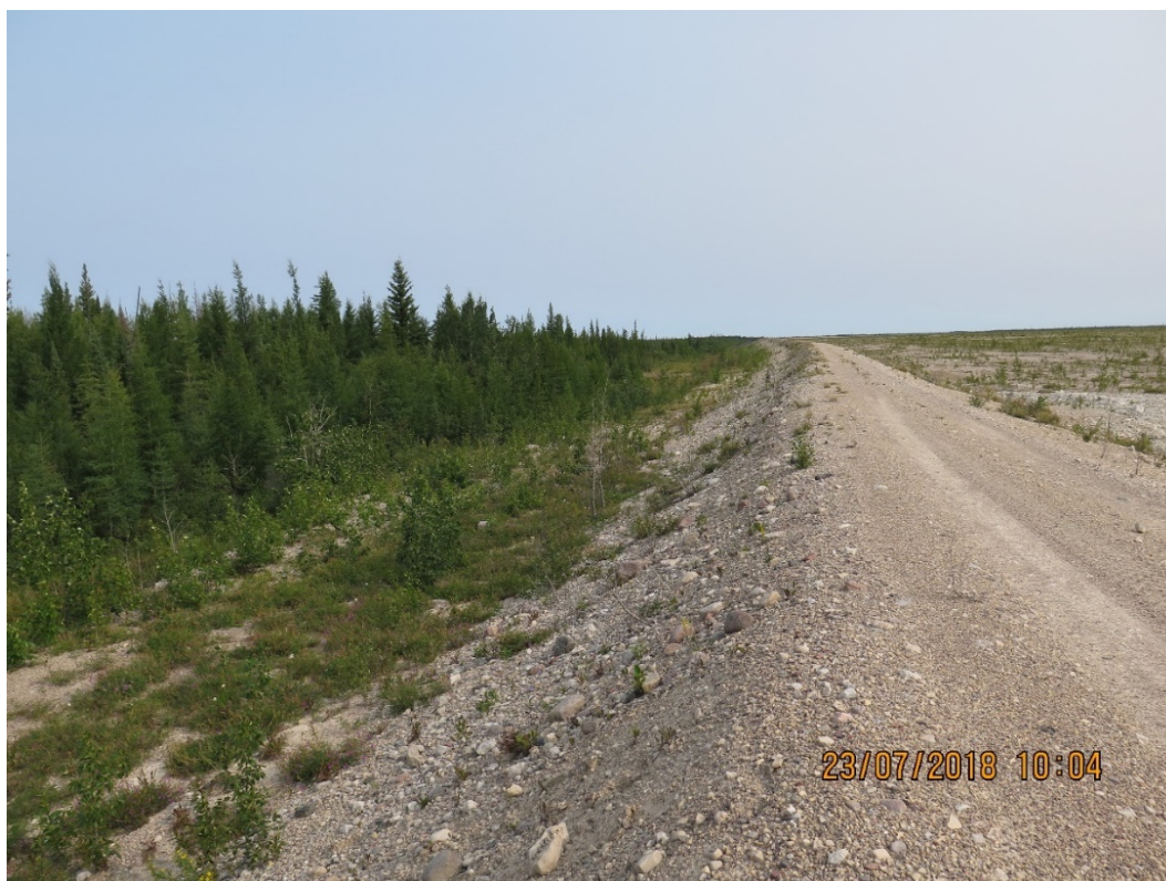
Photograph 4: West Dyke – Downstream Face Near South End, Looking North. 23 July 2018
