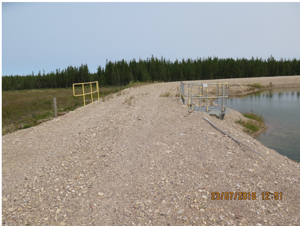
Photograph 16: North Dyke – Crest at Polishing Pond Spillway (Spillway No.2), Polishing Pond on Right, Looking North. 23 July 2018
