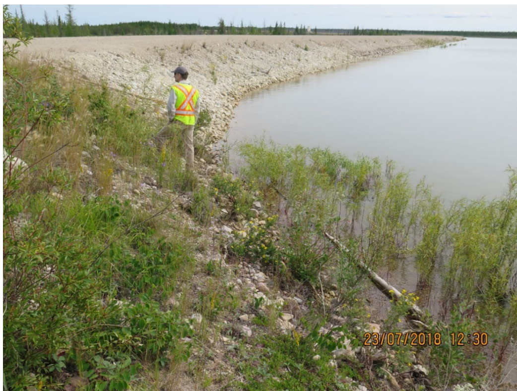
Photograph 12: North Dyke - Upstream Face, Gravel and Cobbles at Pond Waterline, at Dogleg Looking East. 23 July 2018
