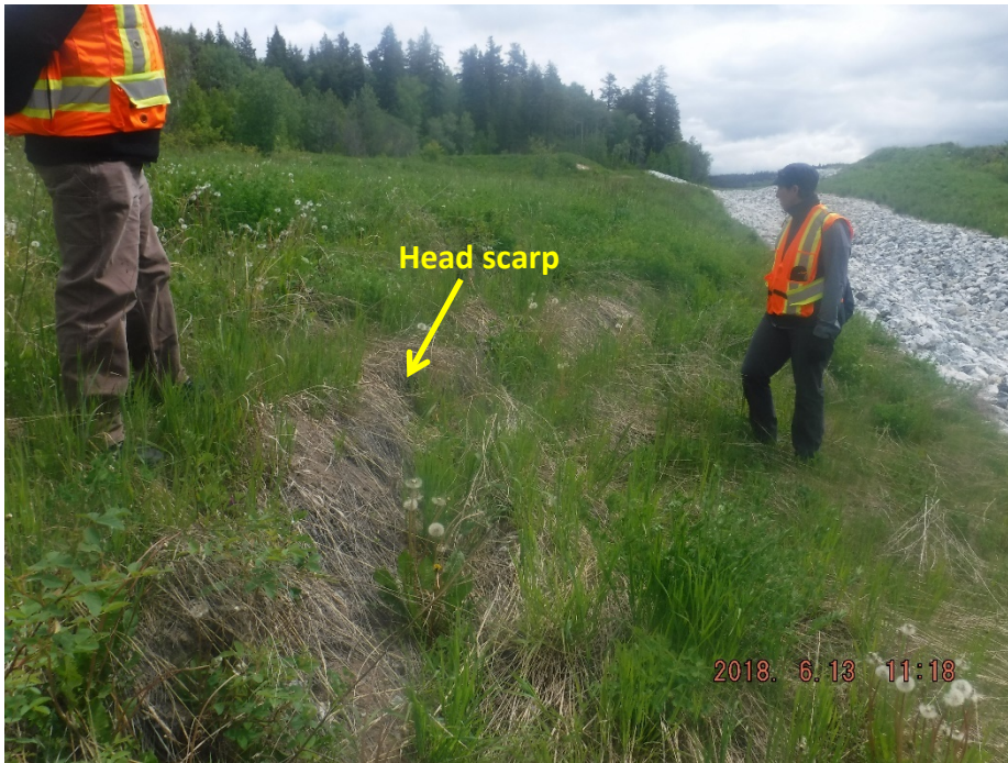
Photo II-35 Closure Spillway – head scarp of slump above right bank, 90 m downstream of centreline
