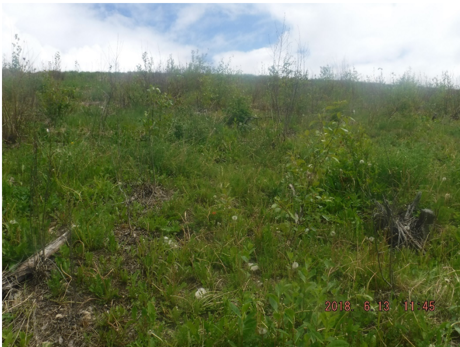
Photo II-22 Tailings Dam – southwest leg, looking upstream from dam toe.
