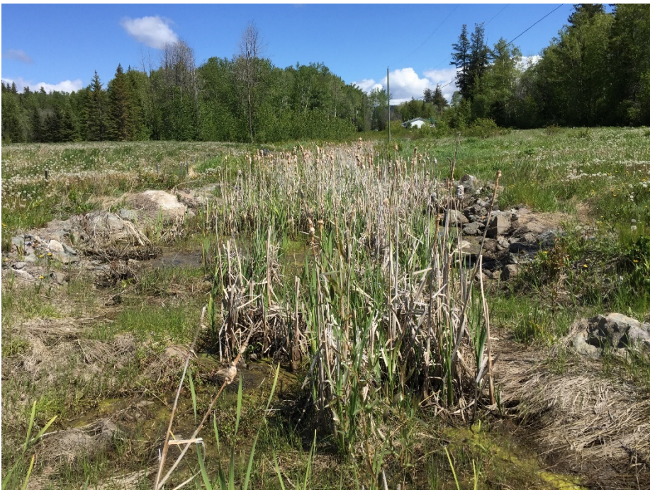
Photo II-40 Spillway Downstream Channel – Middle Reach, looking upstream from culvert beneath road to former caretaker’s house.
