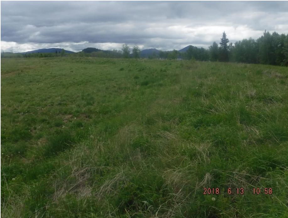
Photo II-25 Tailings Dam – west leg, looking south along upstream slope. Covered tailings surface is on the left.
