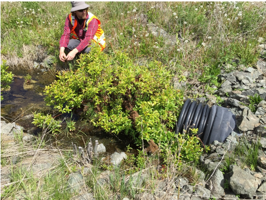
Photo II-62 Inlet of 460 mm culvert on north bank of Ed Creek Diversion Channel. There is vegetation upstream of the inlet that could block the channel during flood conditions.
