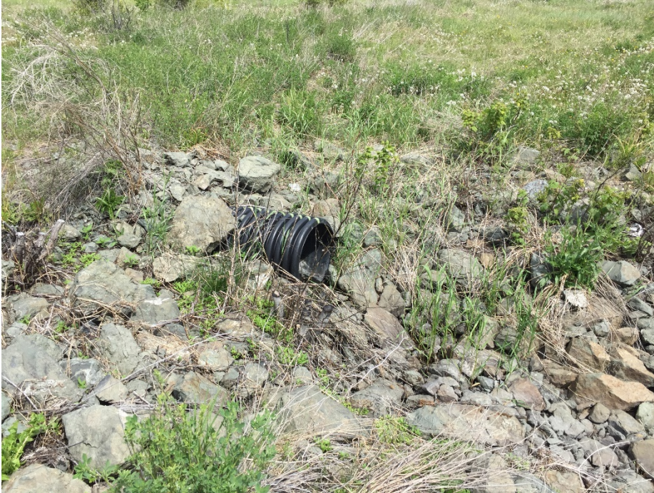
Photo II-61 Outlet of 460 mm culvert on north bank of Ed Creek Diversion Channel.
