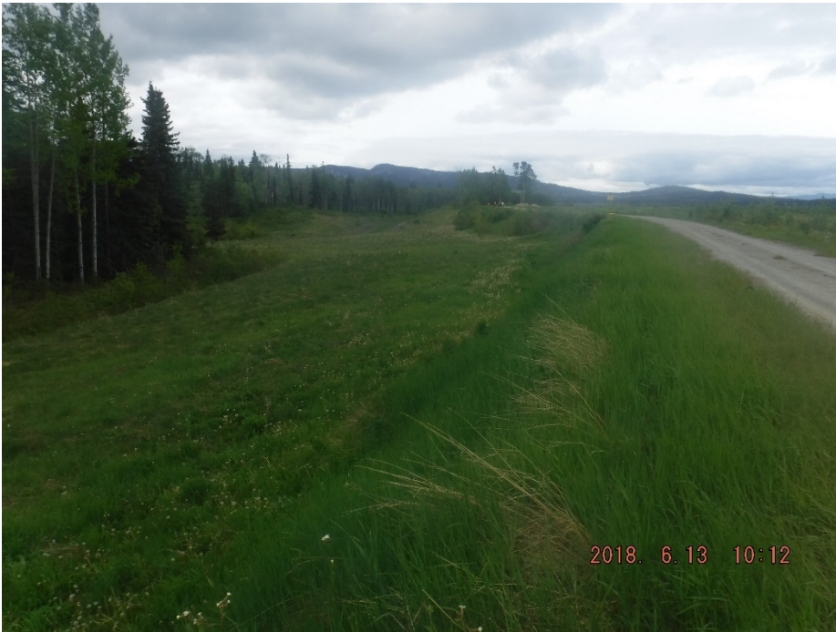
Photo II-7 Tailings Dam – east leg, looking north.
