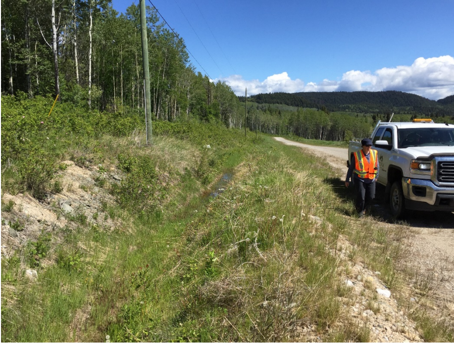
Photo II-49 Road ditch above tailings impoundment, looking east.
