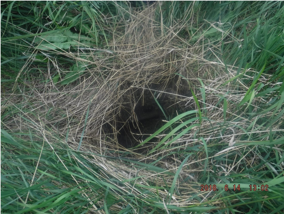
Photo II-13 Tailings Dam – hole at former survey monument location 1018 on upstream side of crest at south leg.
