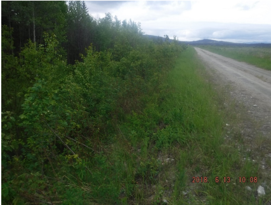
Photo II-1 Tailings Dam – east leg, looking south. Note vegetation on dam slope.
