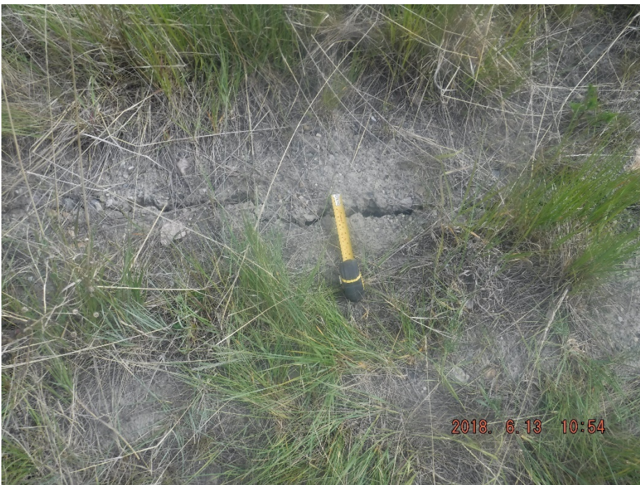
Photo II-18 Tailings Dam – southwest leg, crack on dam crest in tire track.
