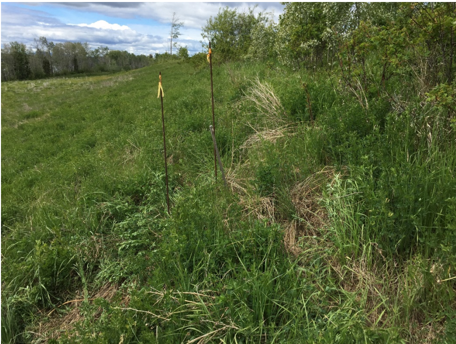
Photo II-44 Borrow Area A – tension crack monitoring rod location 103.
