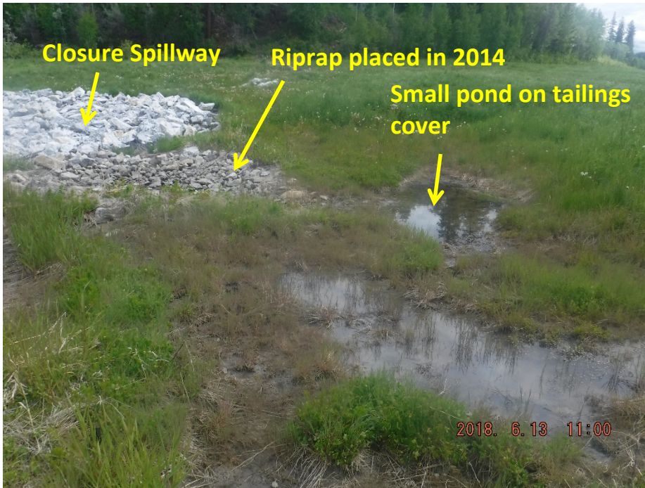
Photo II-29 Downstream end of surface runoff channel where it discharges to the Closure Spillway, showing riprap which was placed in 2014.
