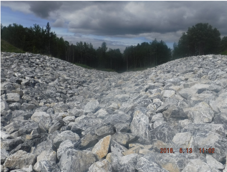
Photo II-31 Closure Spillway – looking downstream from inlet.
