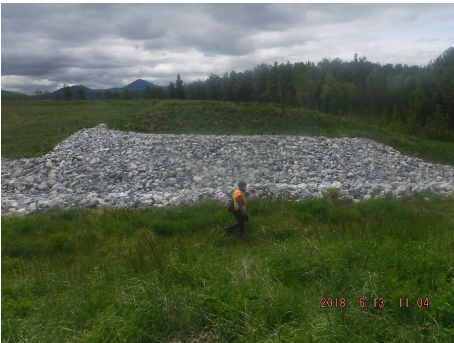
Photo II-32 Closure Spillway – looking south from dam crest
