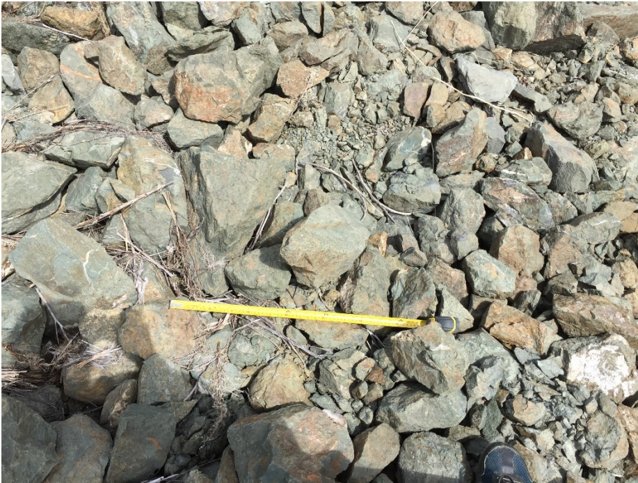
Photo II-53 Ed Creek Diversion Channel – Riprap on right bank, showing weathering and breakage.
