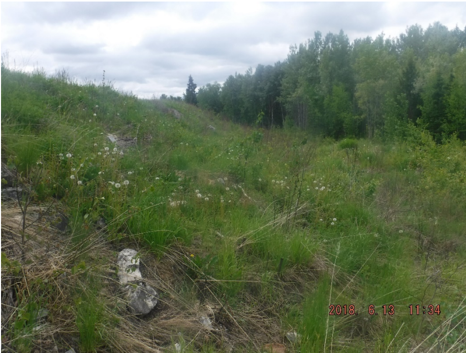
Photo II-27 Tailings Dam – west leg, looking south along dam slope.
