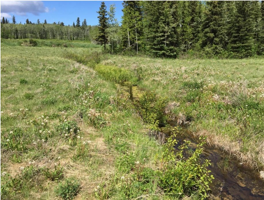
Photo II-63 Drainage ditch between pond area at the toe of the east leg of the Tailings Dam and Ed Creek Diversion Channel. Looking upstream from culvert shown in Photo II-62.
