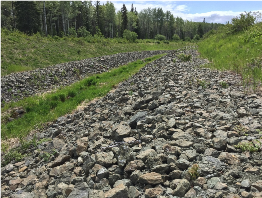
Photo II-57 Ed Creek Diversion Channel – looking downstream from between first and second bends.
