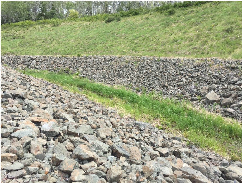
Photo II-52 Ed Creek Diversion Channel – looking upstream from near outlet.
