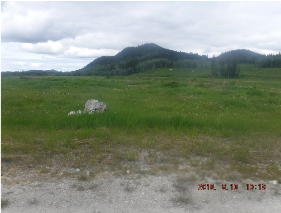
Photo II-9 Tailings Dam – east leg, looking west at the covered tailings surface.
