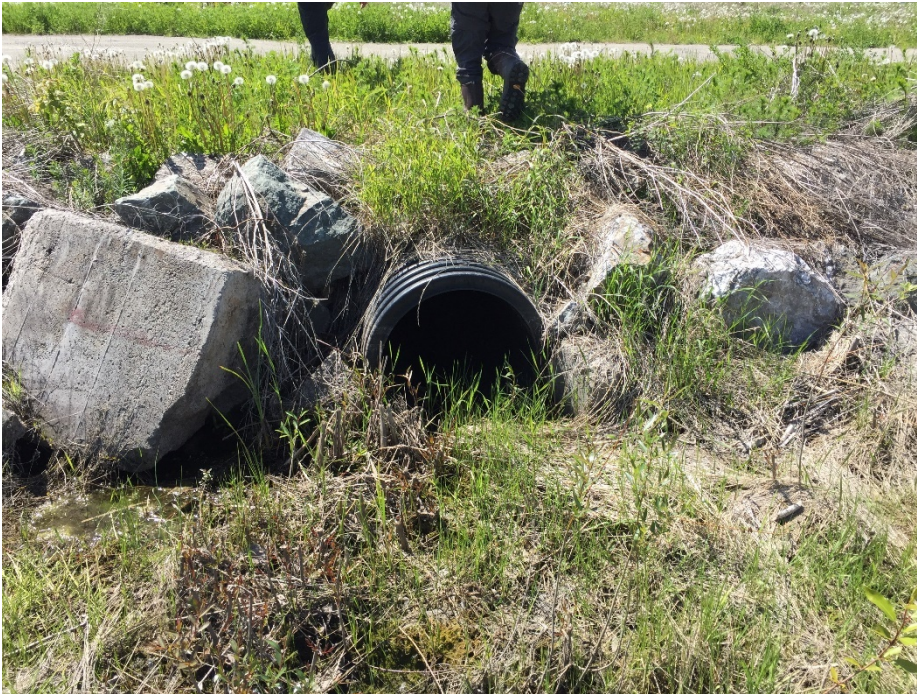
Photo II-39 Spillway Downstream Channel – inlet to culvert beneath road to former caretaker’s house.
