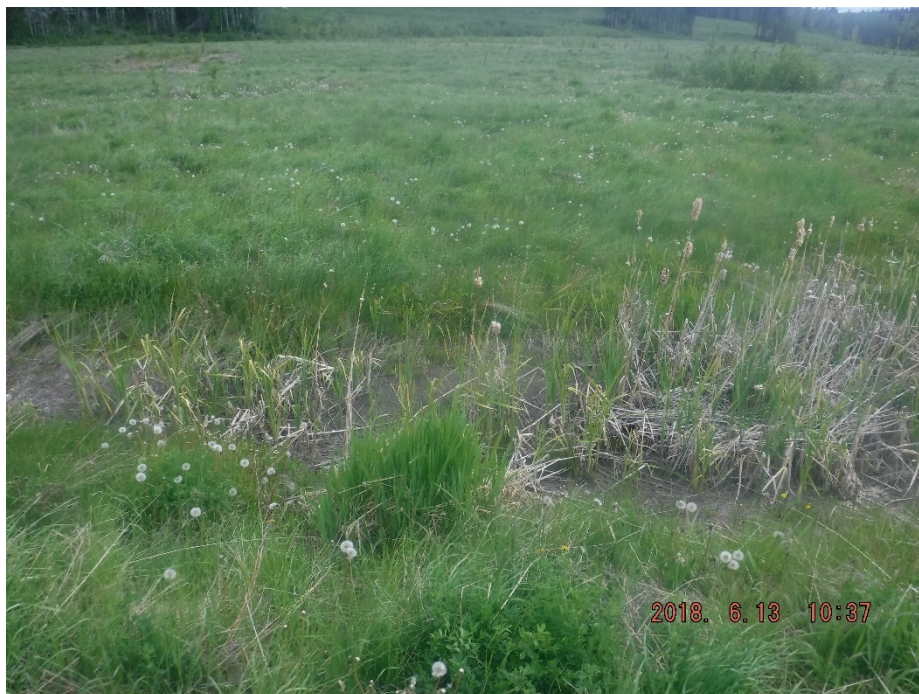
Photo II-20 Tailings Dam – southwest leg, surface runoff channel in tailings cover upstream of dam.
