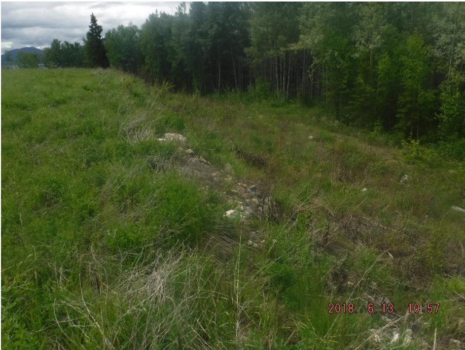
Photo II-24 Tailings Dam – west leg, looking south along downstream slope.
