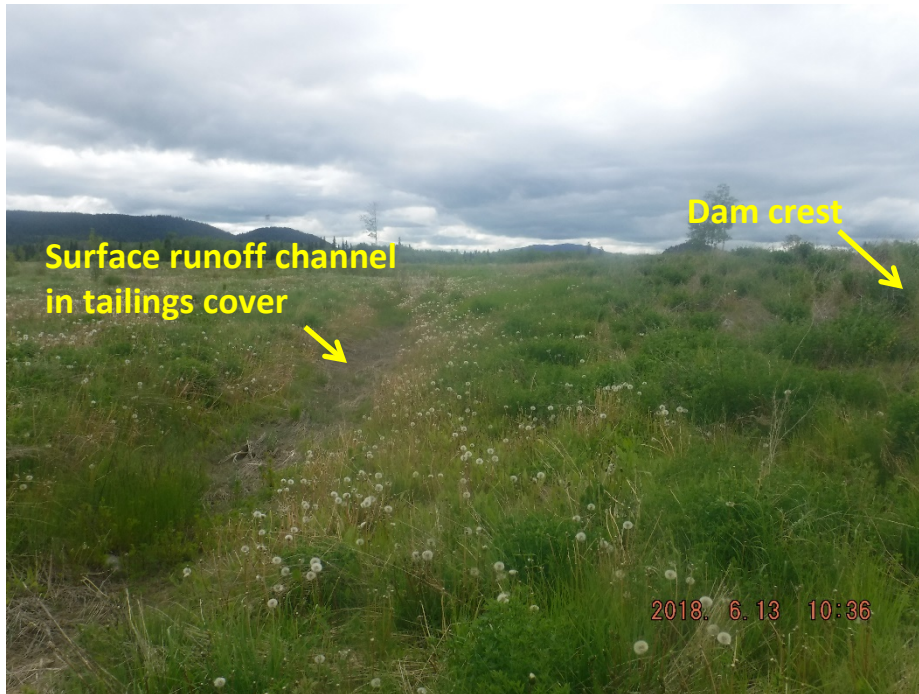
Photo II-19 Tailings Dam – southwest leg, surface runoff channel in tailings cover upstream of dam.
