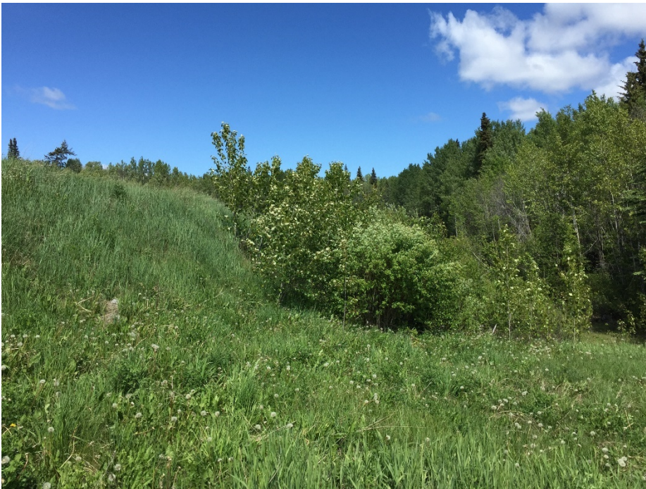
Photo II-6 Tailings Dam – east leg, looking north. Note vegetation on dam slope.
