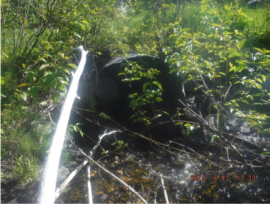
Photo II-65 Inlet of east culvert under Pinchi Lake Road.
