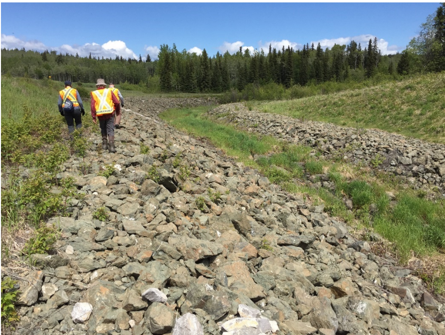
Photo II-58 Ed Creek Diversion Channel – looking upstream from between first and second bends.
