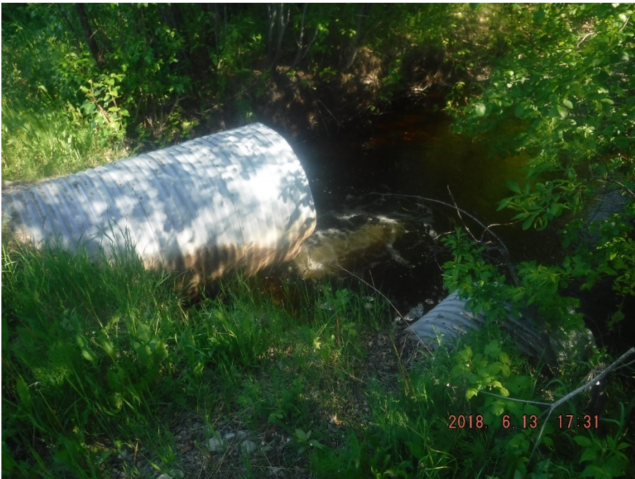
Photo II-66 Outlets of Ed Creek culverts under Pinchi Lake Road.
