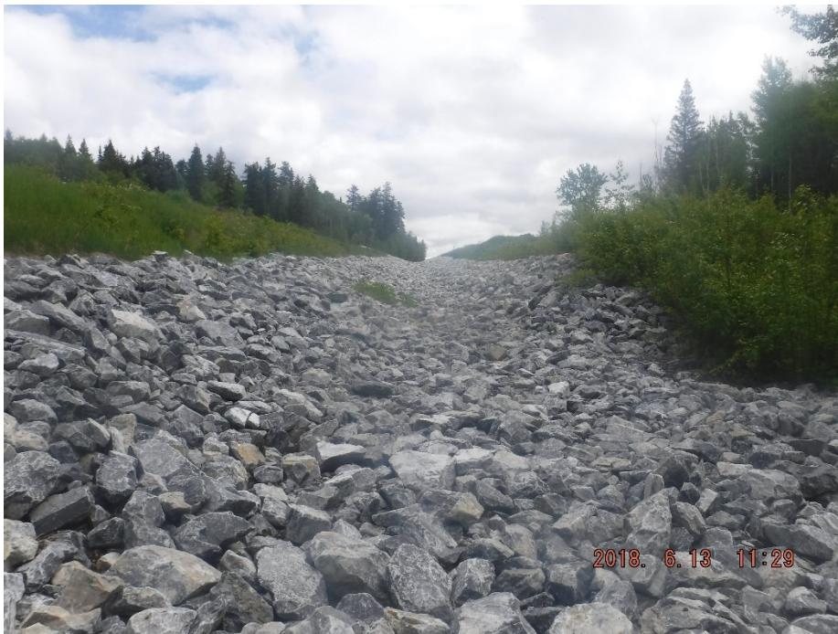
Photo II-36 Closure Spillway – looking upstream from downstream end of riprap.
