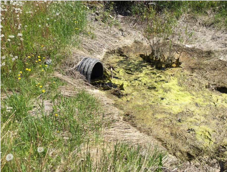
Photo II-41 Spillway Downstream Channel – outlet of culvert beneath road to former caretaker’s house.
