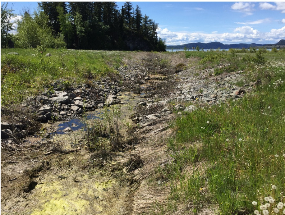
Photo II-42 Spillway Downstream Channel – Lower Reach, looking downstream from culvert beneath road to former caretaker’s house.
