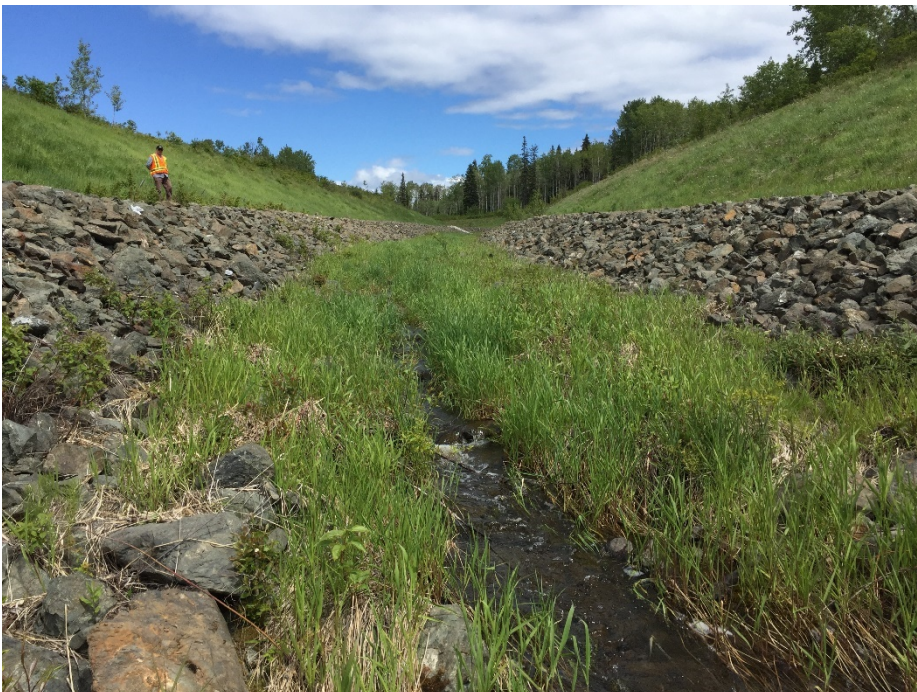
Photo II-54 Ed Creek Diversion Channel – looking upstream from near third bend. Flow depth in channel is 20 cm.
