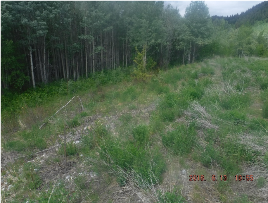
Photo II-23 Tailings Dam – southwest leg, looking northwest along dam slope towards corner with west leg.
