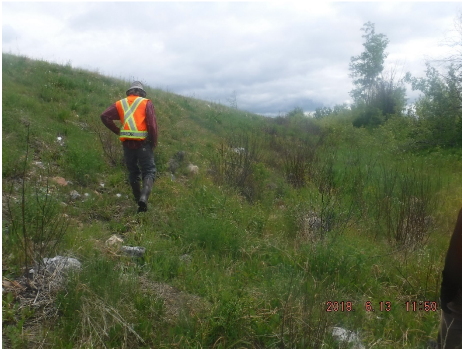
Photo II-21 Tailings Dam – southwest leg, looking southeast along dam toe.
