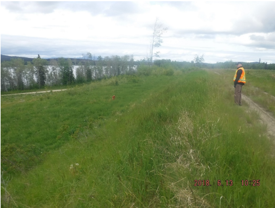
Photo II-12 Tailings Dam – south leg, looking west along downstream slope.
