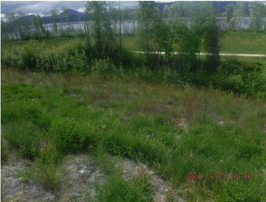
Photo II-17 Tailings Dam – southwest leg, looking downstream from the crest.
