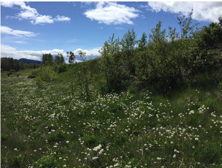
Photo II-8 Tailings Dam – east leg, looking south. Note vegetation on dam slope.
