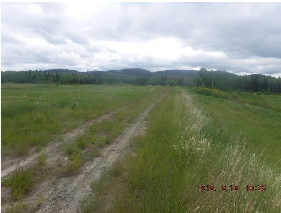
Photo II-10 Tailings Dam – south leg, looking east from mid-point towards Ed Creek.
