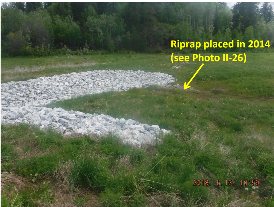
Photo II-28 Closure Spillway – inlet apron.
