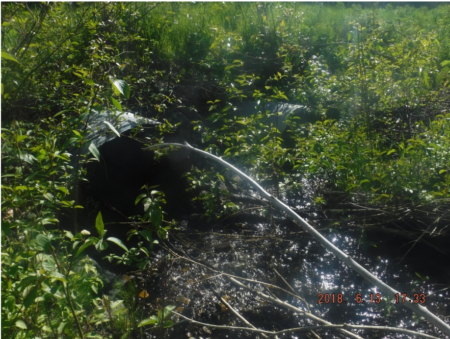
Photo II-64 Inlets of Ed Creek culverts under Pinchi Lake Road.
