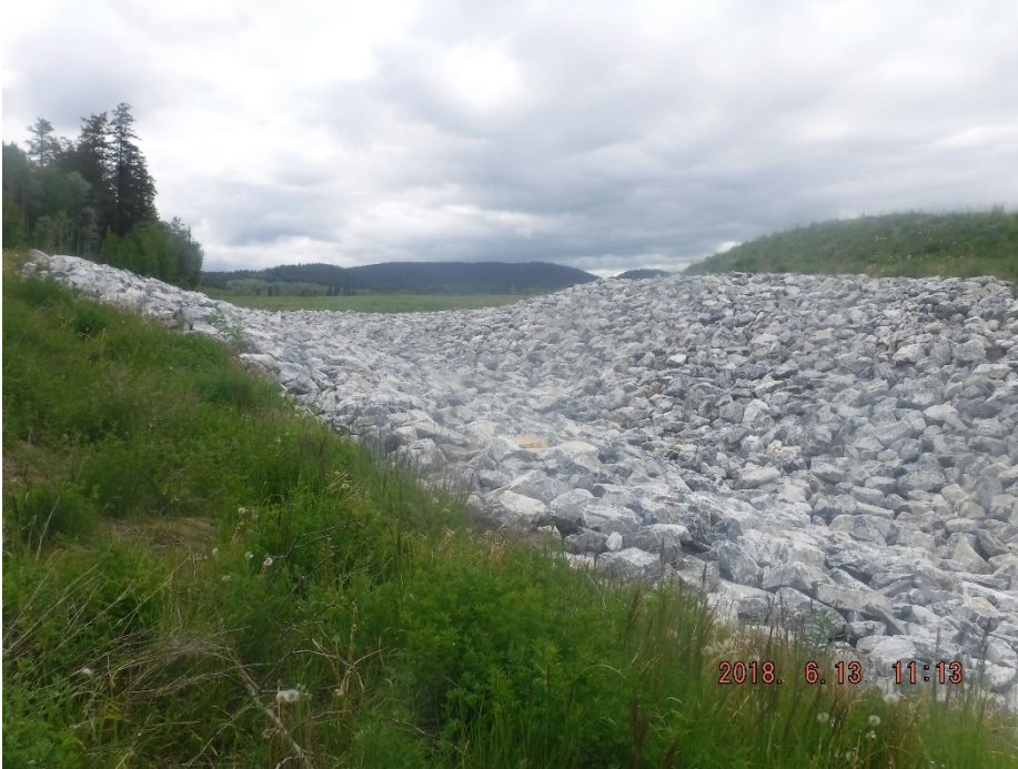
Photo II-33 Closure Spillway – looking upstream from dam toe area.
