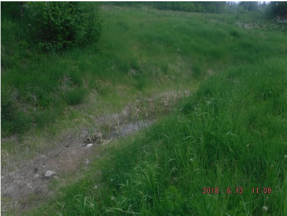
Photo II-38 West Ditch – looking northeast. Note small pond in base of ditch.
