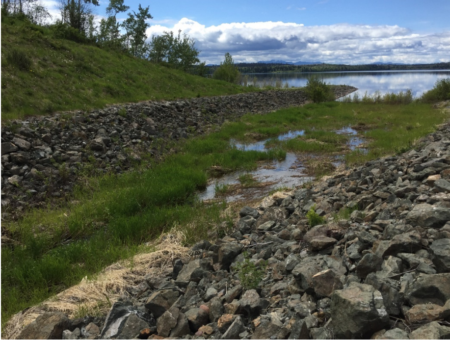
Photo II-51 Ed Creek Diversion Channel – outlet at Pinchi Lake.
