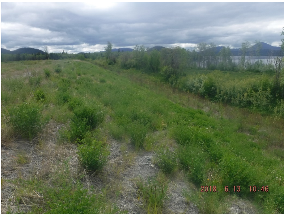
Photo II-16 Tailings Dam – southwest leg, looking southeast along the downstream slope.
