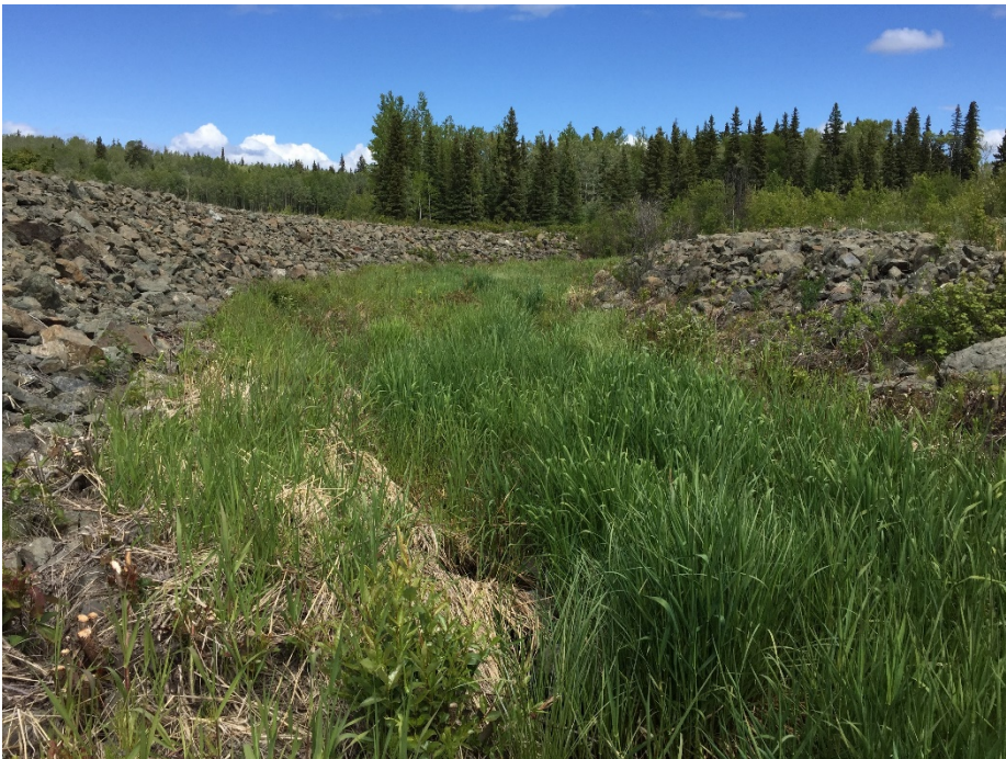
Photo II-60 Ed Creek Diversion Channel – looking upstream towards first bend.
