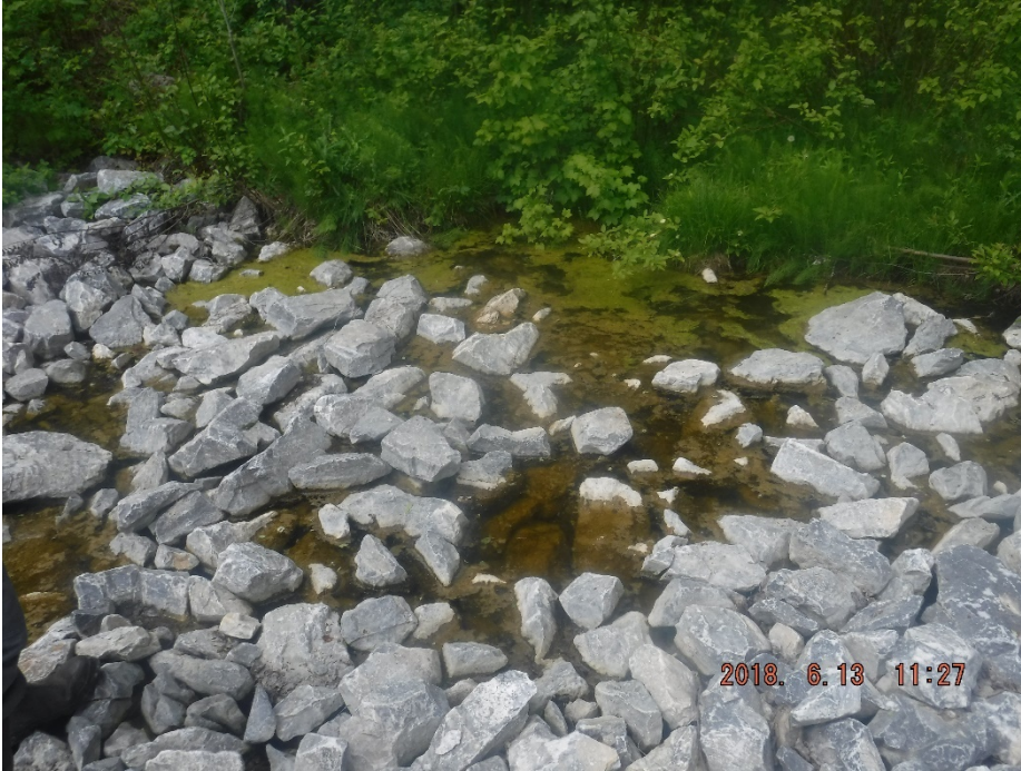
Photo II-37 Closure Spillway – pond at downstream end of riprap.
