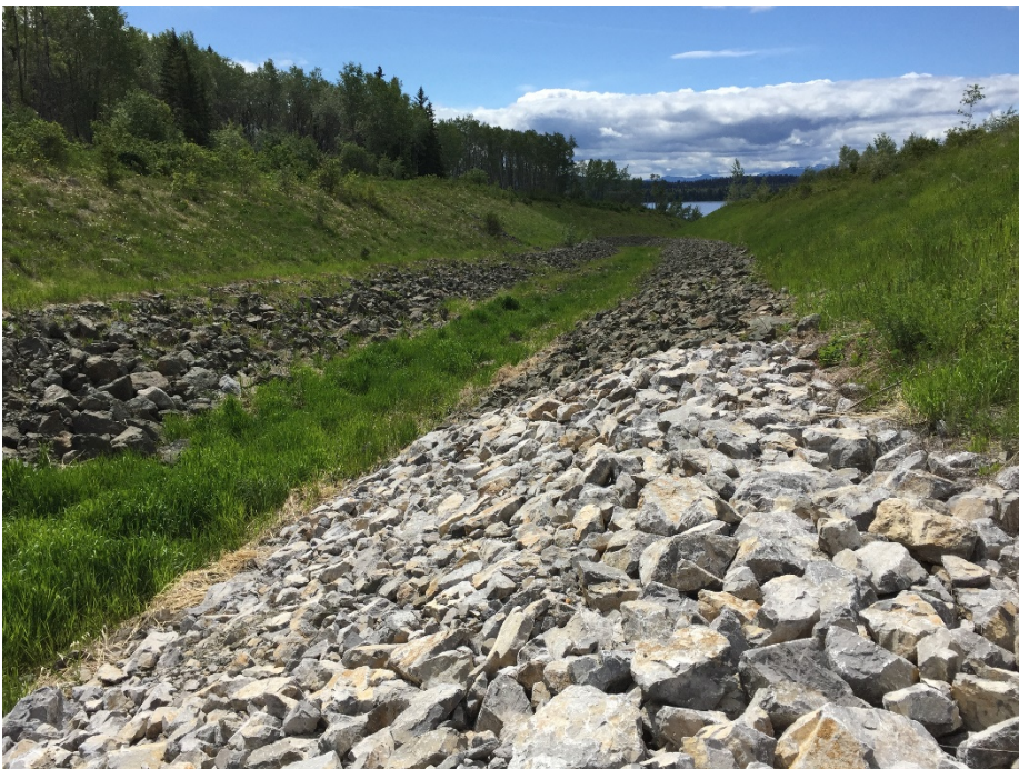
Photo II-56 Ed Creek Diversion Channel – looking downstream from near second bend. Light-coloured area of riprap was replaced in 2014, and is in good condition.
