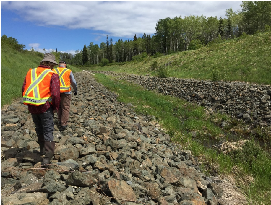
Photo II-55 Ed Creek Diversion Channel – looking upstream from between second and third bends.
