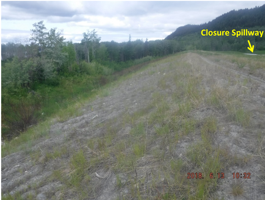
Photo II-15 Tailings Dam – southwest leg, looking northwest along the downstream slope.
