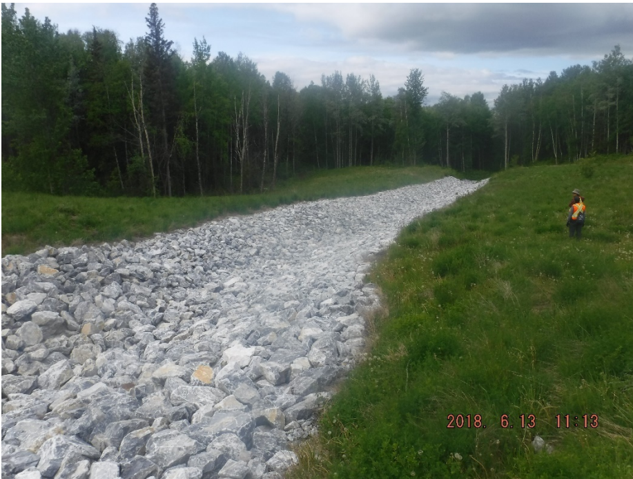
Photo II-34 Closure Spillway – looking downstream.
