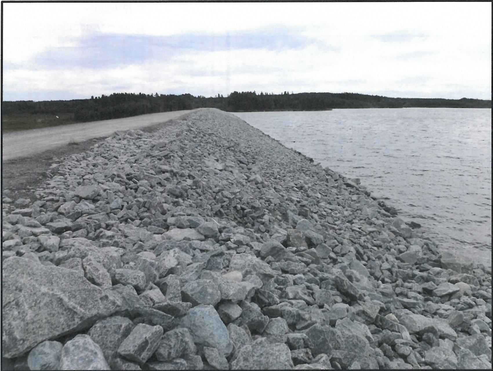
Photograph 6: Dam 1D, upstream slope
