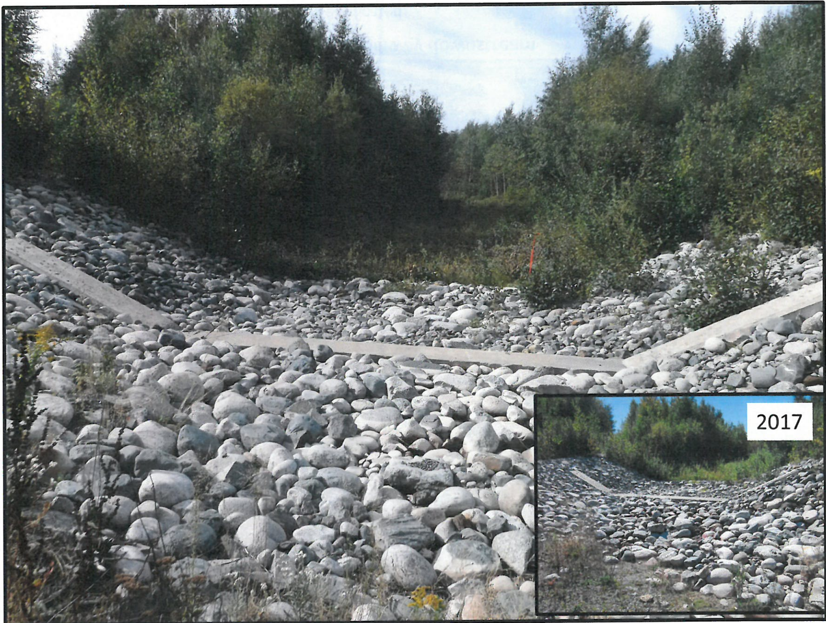
Photograph 8: Dam 1E, emergency spillway upstream
