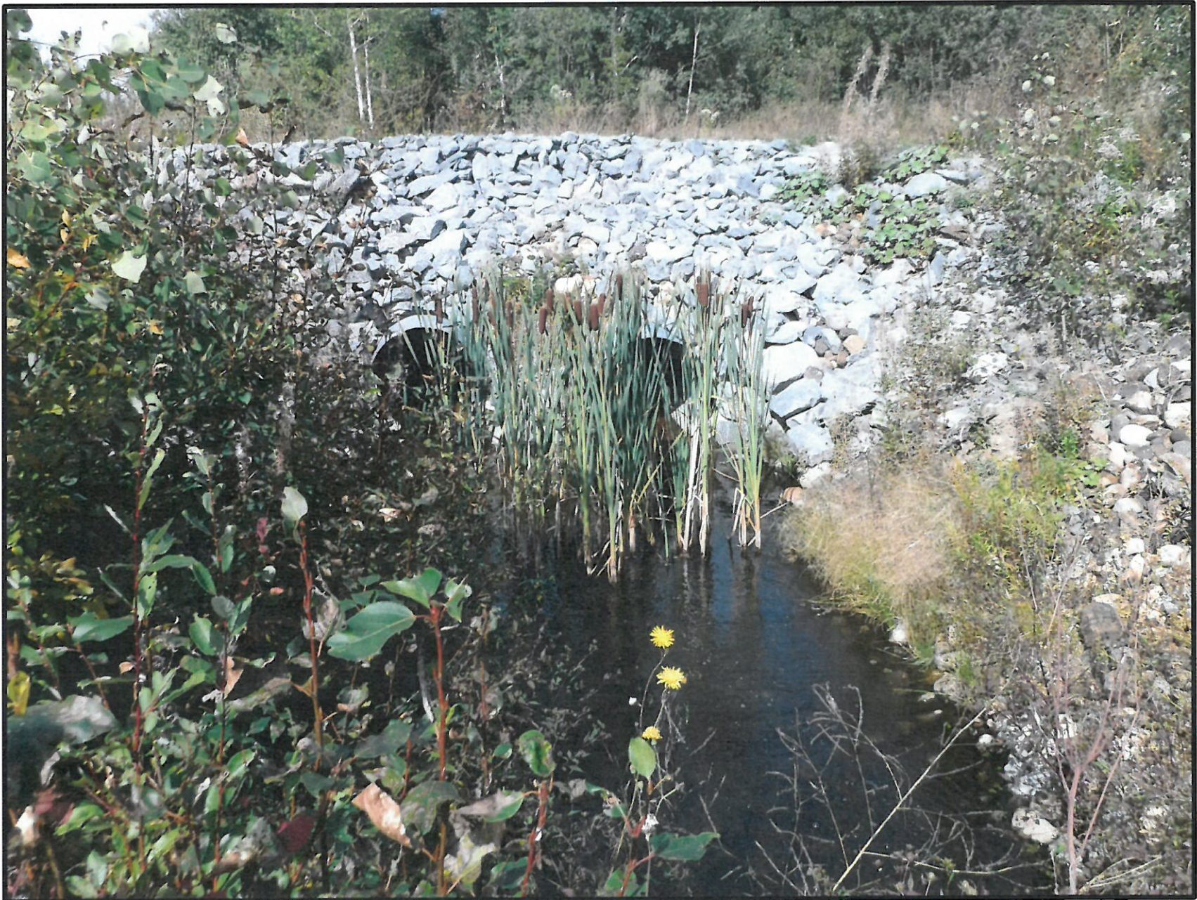
Photograph 2: Dam 4B, final effluent
