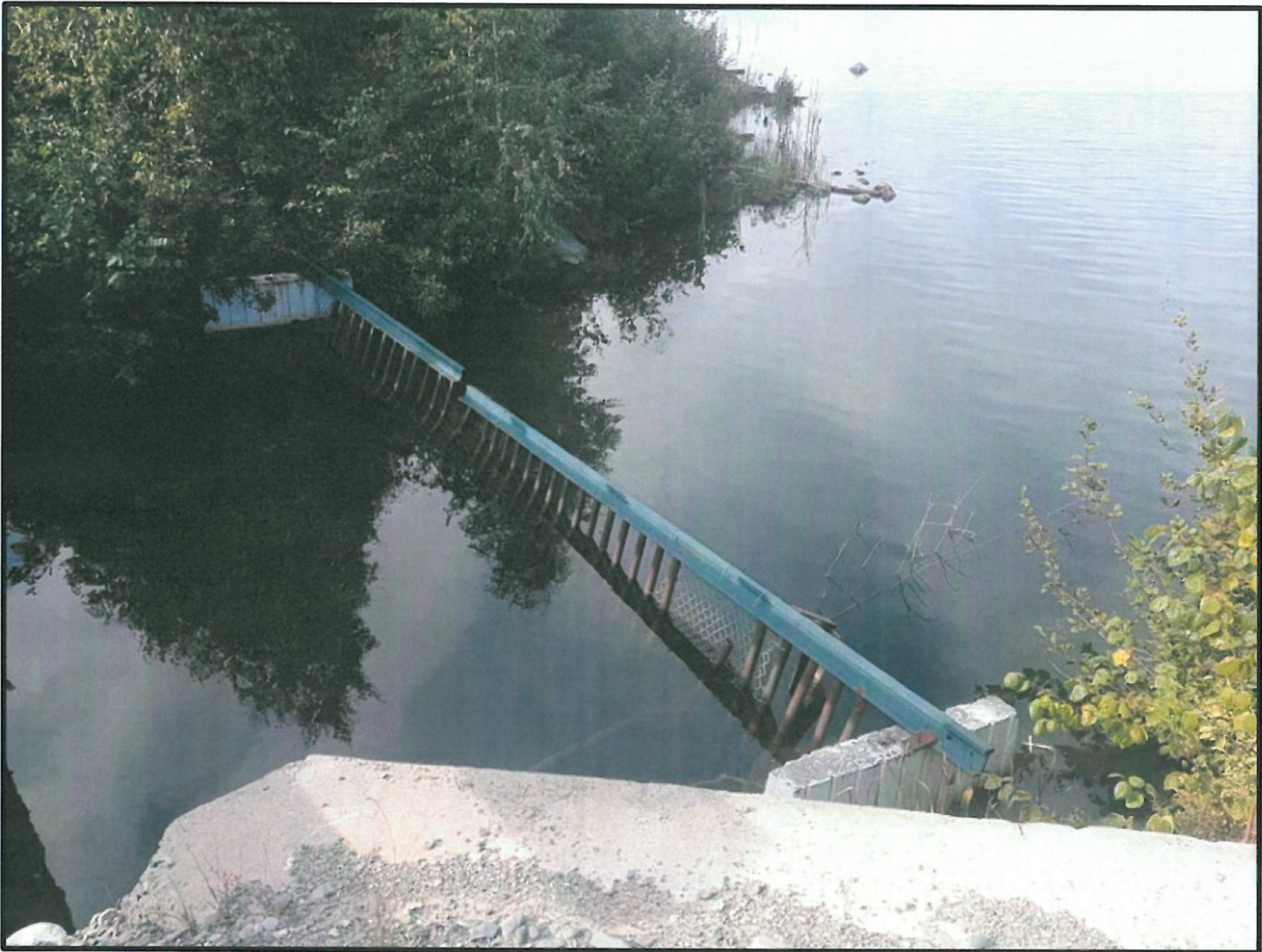
Photograph 7: Dam 1E Spillway
