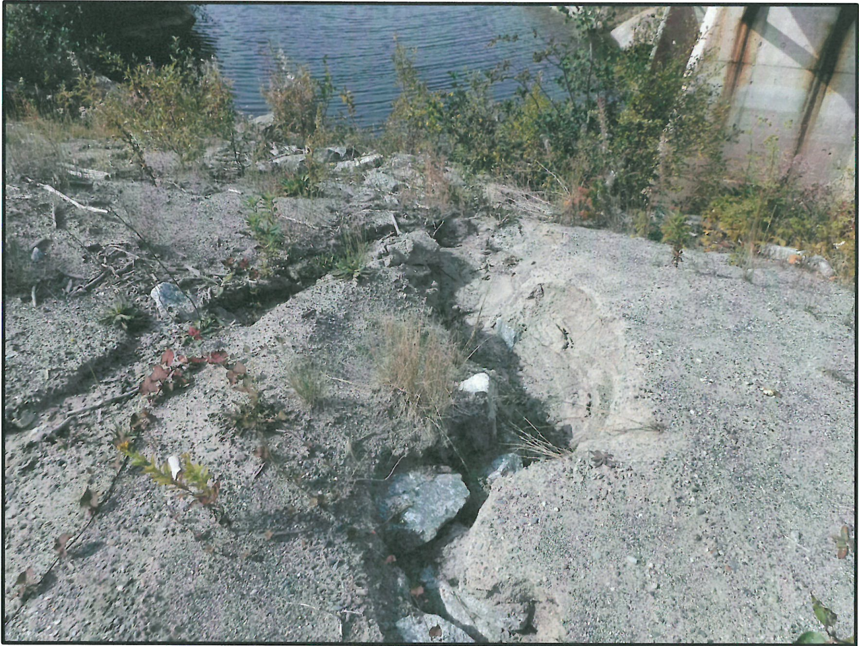
Photograph 5: Dam 4B, spillway
