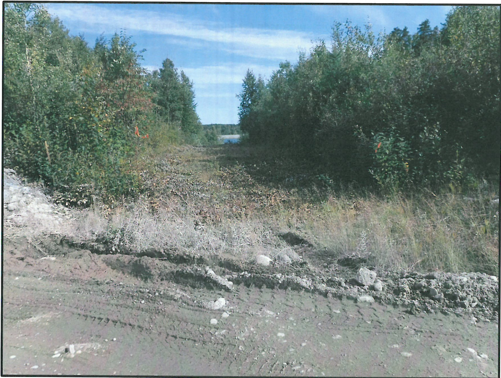
Photograph 9: Dam 1E, emergency spillway downstream
