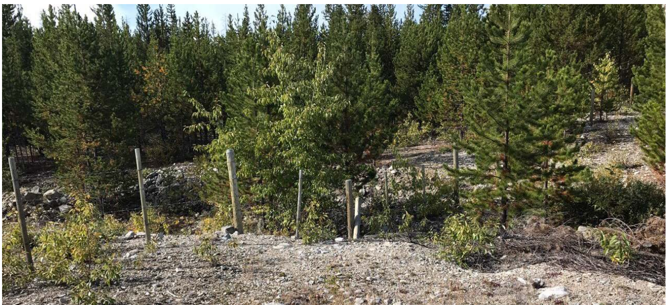
Photo II-B-20 S3: spillway channel downstream of blockade. (HGH-2018-20)
