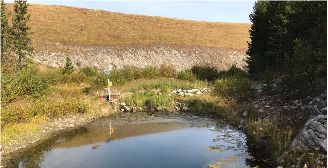
Photo II-A-7 Steepened section of downstream slope and underdrain flow channel. Underdrain discharge seems similar to 2017 DSI. There is no evidence of excessive ponding or high-water level on dam toe. (HGH-2018-5)
