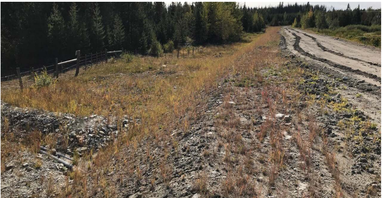
Photo II-B-23 S5: Downstream slope of central pond looking south towards right abutment. Slope is in good condition (HGH-2018-22)
