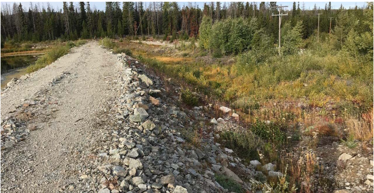
Photo II-B-7 S2: Downstream slope looking from right abutment. The slope is in good condition; no erosion was observed (HGH-2018-16)
