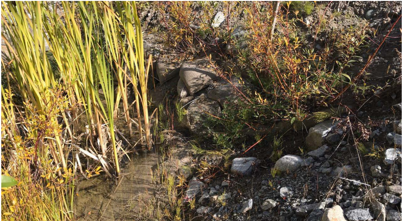
Photo II-B-30 S5: Spillway pipes (2x), inlet blocked with sand bags. (HGH-2018-25)
