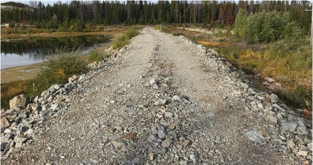
Photo II-B-7 S2: Downstream slope looking from right abutment. The slope is in good condition; no erosion was observed (HGH-2018-16)
