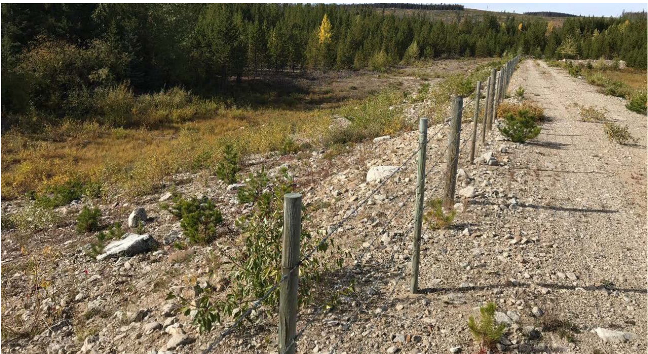
Photo II-B-15 S3: Downstream slope; no sign of erosion is observed (HGH-2018-19)
