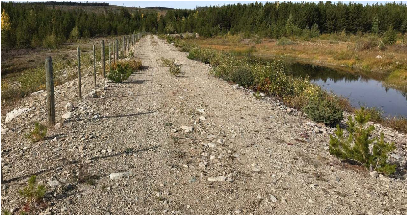
Photo II-B-15 S3: Downstream slope; no sign of erosion is observed (HGH-2018-19)
