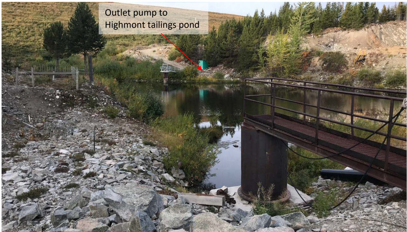
Photo II-B-5 S1: Spillway channel and pipe intake looking downstream. Pipe intake is clear with no sign of vegetation or any other obstructions. (HGH-2018-14)
