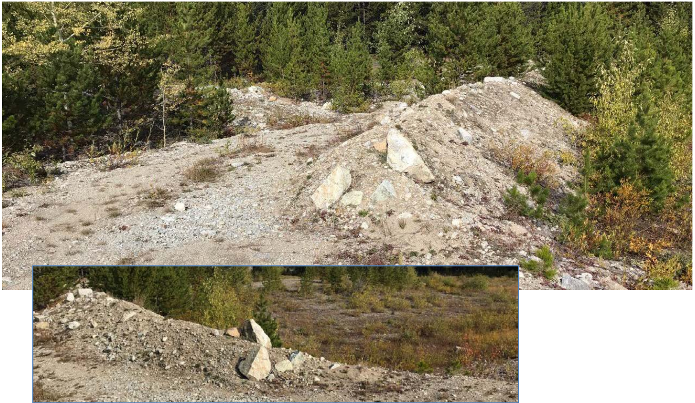
Photo II-B-19 S3: Spillway intake is blocked (HGH-2018-20)
