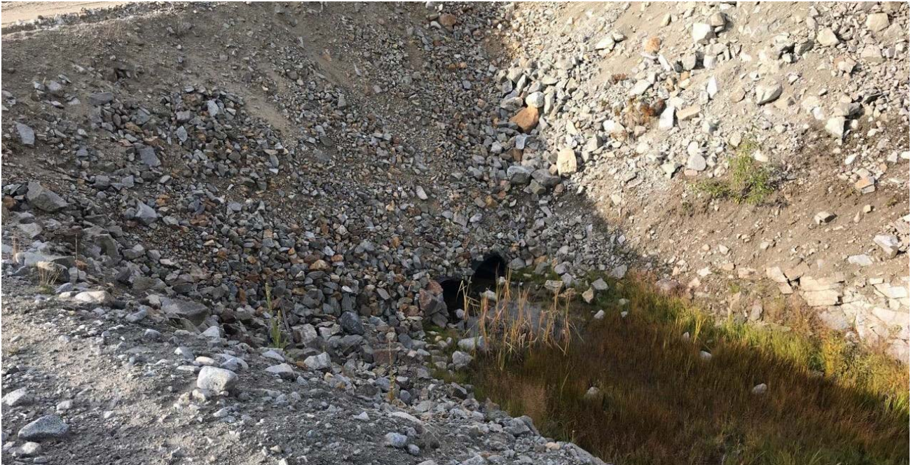
Photo II-A-20 S2: Highmont spillway; looking south. North dam toe and the road-crossing culverts are visible. There is vegetation growth which will be cleared as part of routine maintenance (HGH-2018-13).
