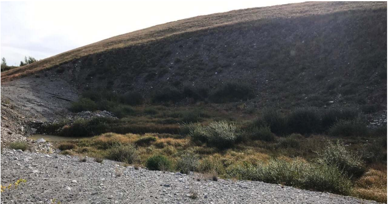
Photo II-A-7 Steepened section of downstream slope and underdrain flow channel. Underdrain discharge seems similar to 2017 DSI. There is no evidence of excessive ponding or high-water level on dam toe. (HGH-2018-5)
