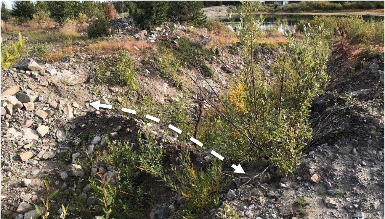
Photo II-B-13 S2: Ponded water at downstream toe, similar in size to the pond noted during the 2015, 2016, and 2017 DSI. (HGH-2018-18)
