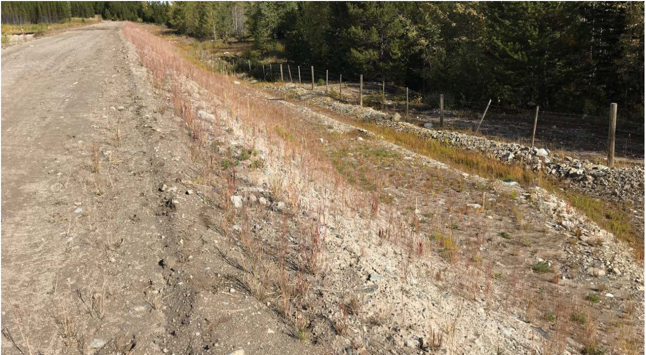
Photo II-B-23 S5: Downstream slope of central pond looking south towards right abutment. Slope is in good condition (HGH-2018-22)
