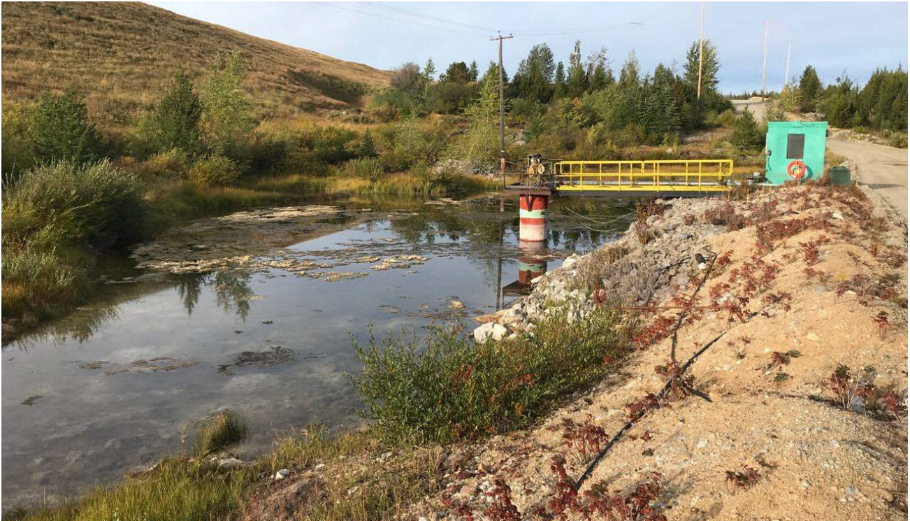
Photo II-B-35 S8: Trash rack for overflow pipe is clear of debris. (HGH-2018-27)
