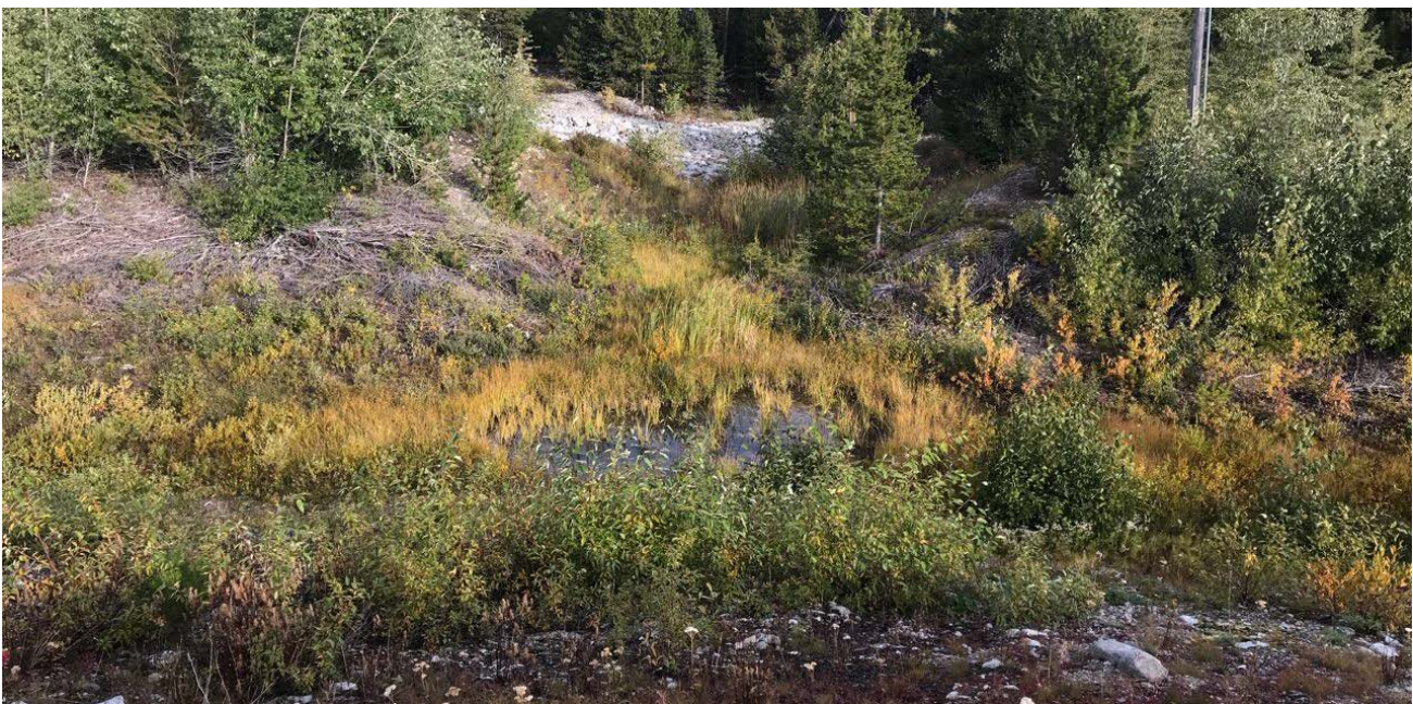
Photo II-B-13 S2: Ponded water at downstream toe, similar in size to the pond noted during the 2015, 2016, and 2017 DSI. (HGH-2018-18)
