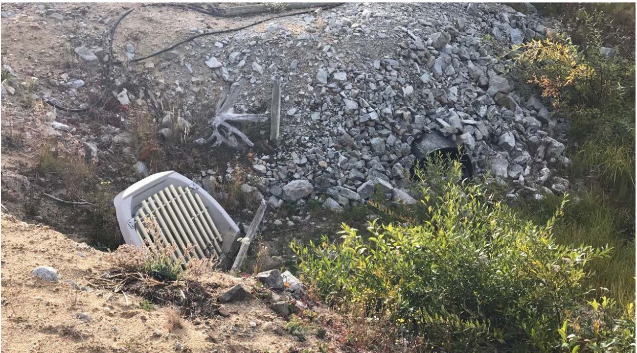
Photo II-B-35 S8: Trash rack for overflow pipe is clear of debris. (HGH-2018-27)
