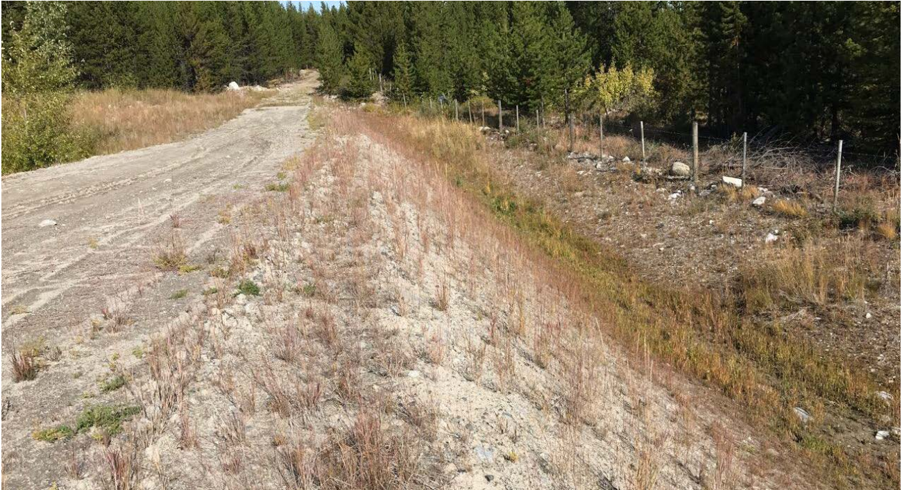
Photo II-B-25 S5: Upstream slope of central pond looking south towards right abutment. Slope is in good condition (HGH-2018-22)
