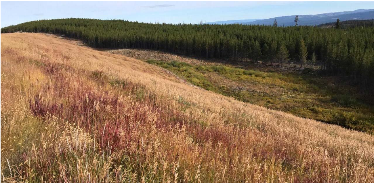
Photo II-A-3 East Dam downstream overview looking North. Slope covered by vegetation. (HGH-2018-2)
