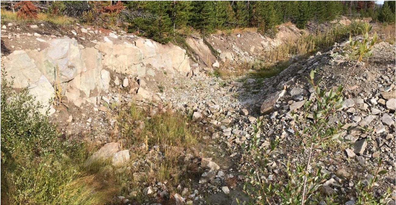
Photo II-A-21 S2: Highmont spillway; looking north. There is vegetation growth which will be cleared as part of routine maintenance (HGH-2018-13)
