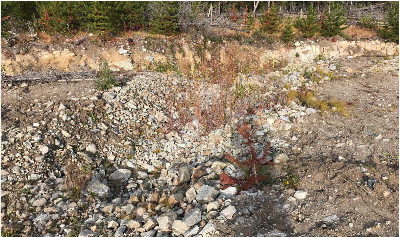
Photo II-B-10 S2: Spillway invert and channel. (HGH-2018-17)
