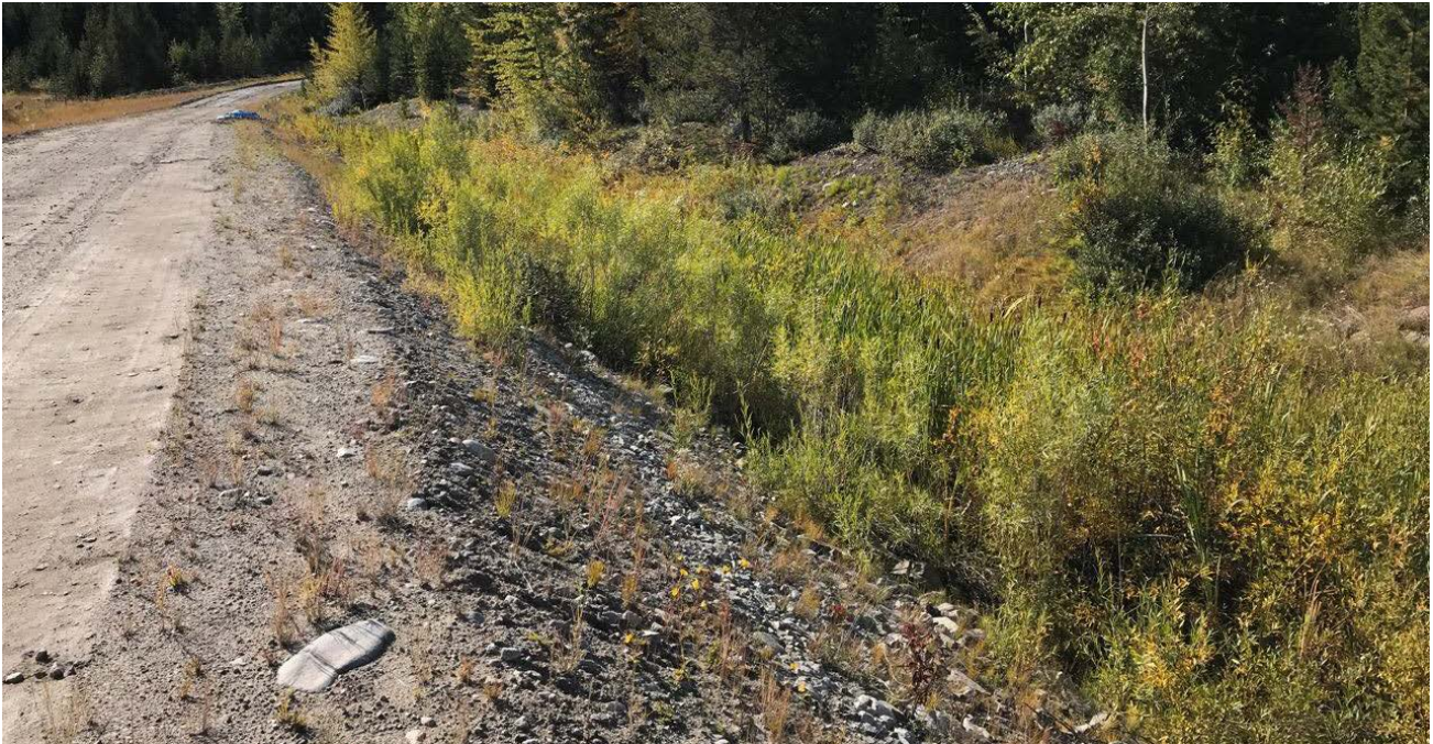
Photo II-B-26 S5: Upstream slope looking South. Slope is in good condition; no sign of erosion is observed (HGH-2018-23)
