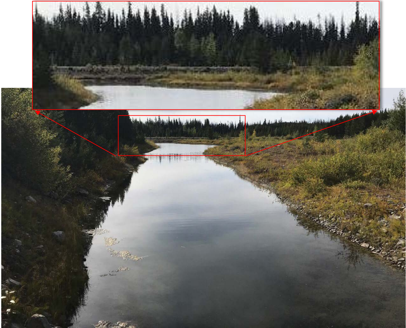
Photo II-B-16 S3: Overview of the pond and upstream slopes, looking South. Slopes are in good condition. (HGH-2018-4)
