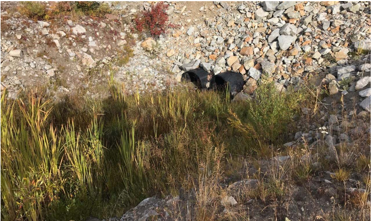
Photo II-A-18 Inlet of 33" ID spillway road culverts, showing vegetation (HGH-2018-11)
