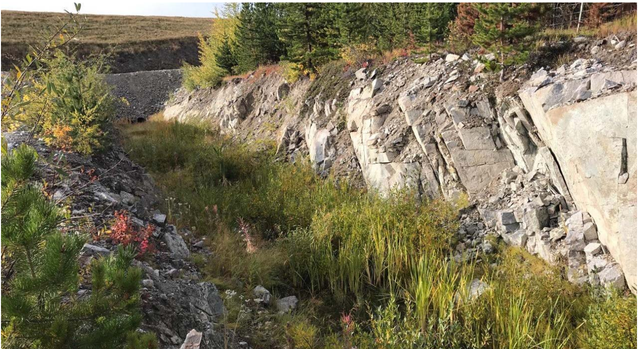
Photo II-A-20 S2: Highmont spillway; looking south. North dam toe and the road-crossing culverts are visible. There is vegetation growth which will be cleared as part of routine maintenance (HGH-2018-13).
