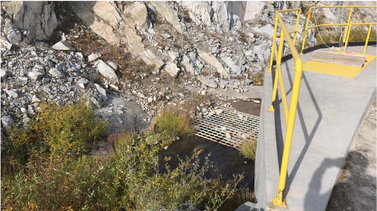
Photo II-A-14 Spillway channel looking downstream at inlet to Seepage Recovery Pond S1 pipeline division, showing trashrack on invert (HGH-2018-9)
