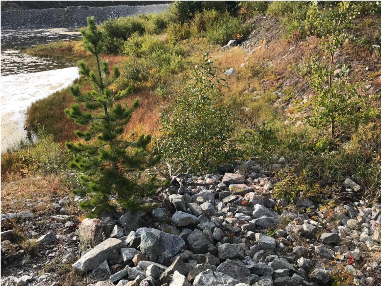
Photo II-B-11 S2: Spillway outlet. Outlet is vegetated; vegetation should be monitored and removed if reduces the outlet capacity. (HGH-2018-17)
