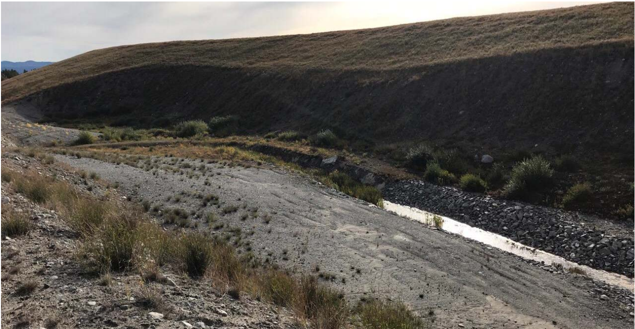
Photo II-A-18 Inlet of 33" ID spillway road culverts, showing vegetation (HGH-2018-11)
