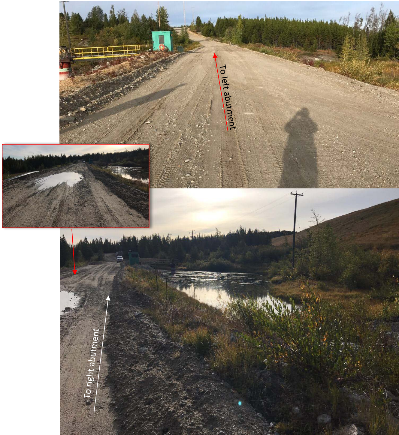
Photo II-B-31 S8: Overview of crest and upstream slope. u/s slope is in good condition. Crest has low points but there is no major distress. (HGH-2018-26)
