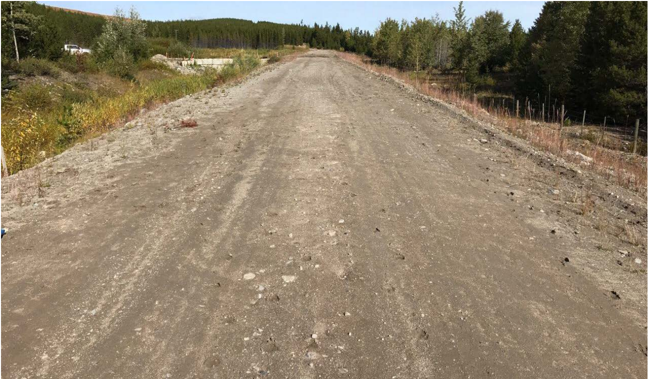
Photo II-B-21 S5: dam crest is in good condition; no evidence of erosion or distress (HGH-2018-21)
