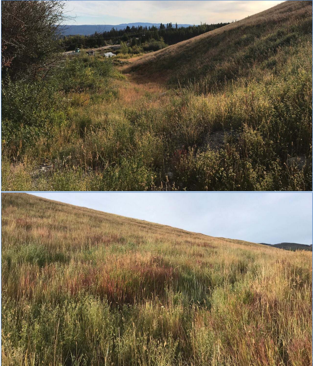
Photo II-A-8 North Dam: local excavation. Appears to be an old pipeline bench excavated at the dam toe. (HGH-2018-6)
