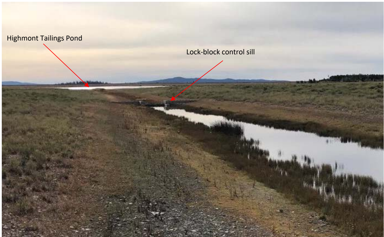
Photo II-A-9 Spillway approach channel, concrete lock-block control sill (HGH-2018-7)
