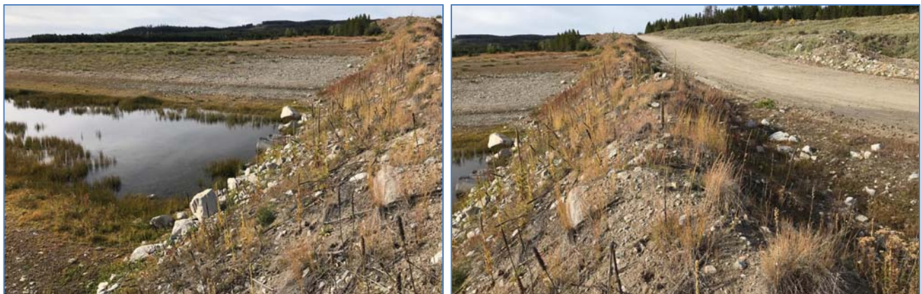
Photo II-A-10 Spillway upstream of road crest. Road is in good condition. Spillway culverts are partially submerged (HGH-2018-7)
