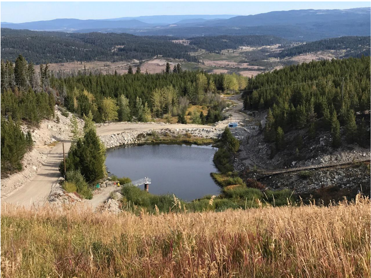
Photo II-B-1 S1: Overview of pond and upstream slope of dam from Highmont Dam crest. (HGH-2018-1)
