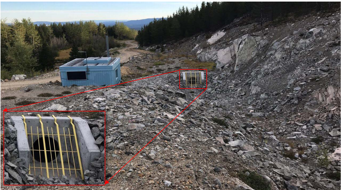
Photo II-B-5 S1: Spillway channel and pipe intake looking downstream. Pipe intake is clear with no sign of vegetation or any other obstructions. (HGH-2018-14)
