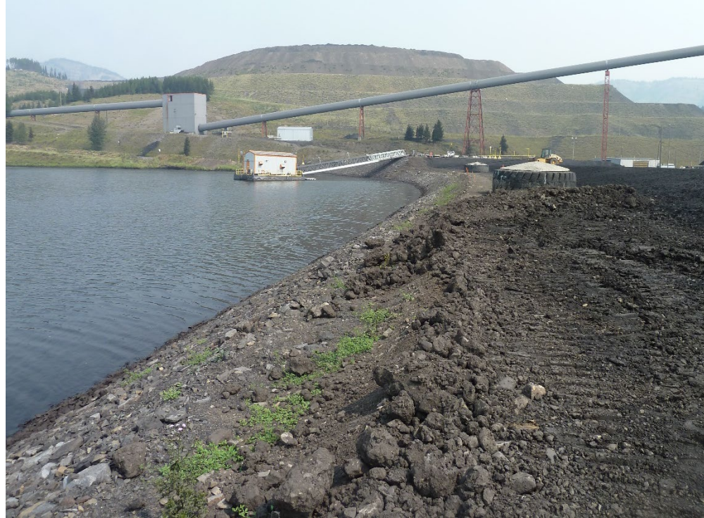
Photograph 5: Main Dam – overview of barge, east abutment, and natural ground north of GHO Tailings Pond, looking northeast. 15 August 2018.
