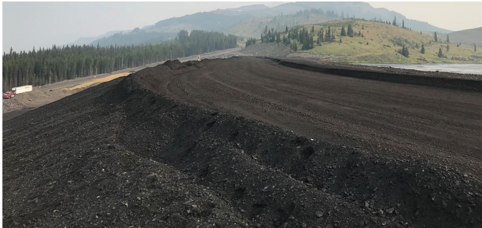
Photograph 21: West Dam – Crest and downstream slope, looking north. 15 August 2018.
