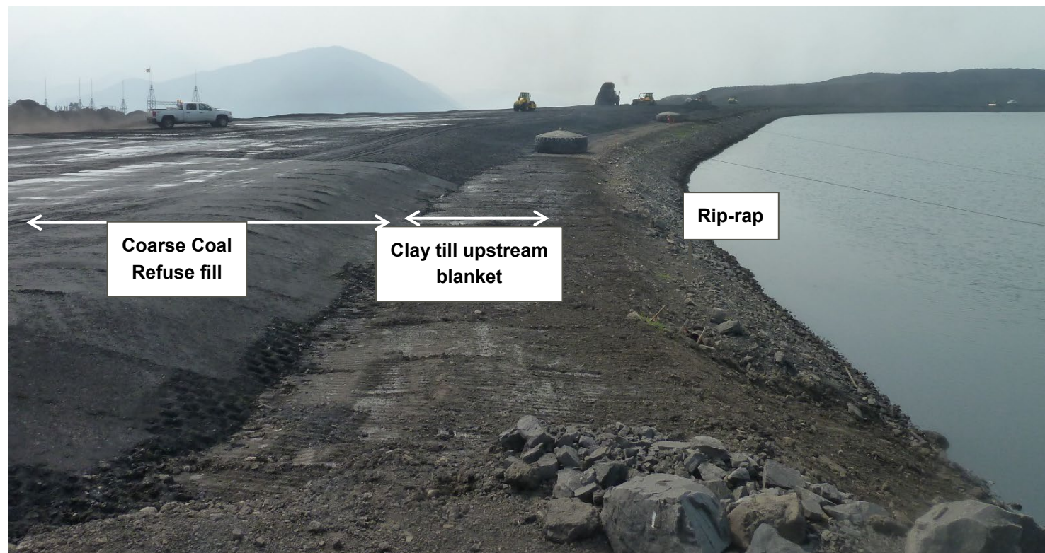
Photograph 4: Main Dam – upstream slope and crest, looking southwest. 15 August 2018.
