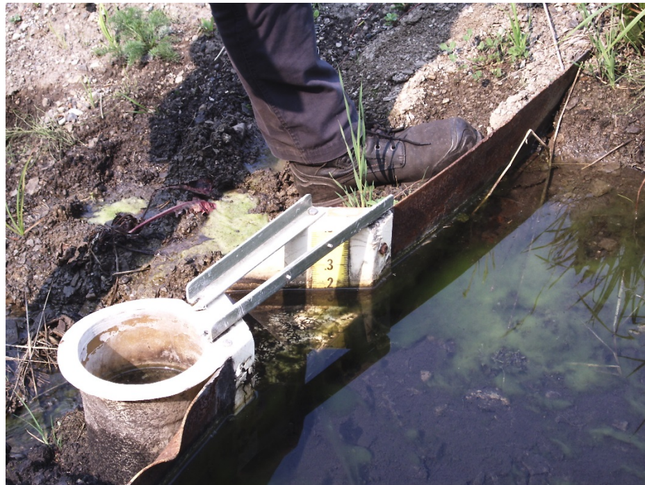
Photograph 235: West Dam – seepage weir downstream of West Dam. 15 August 2018
