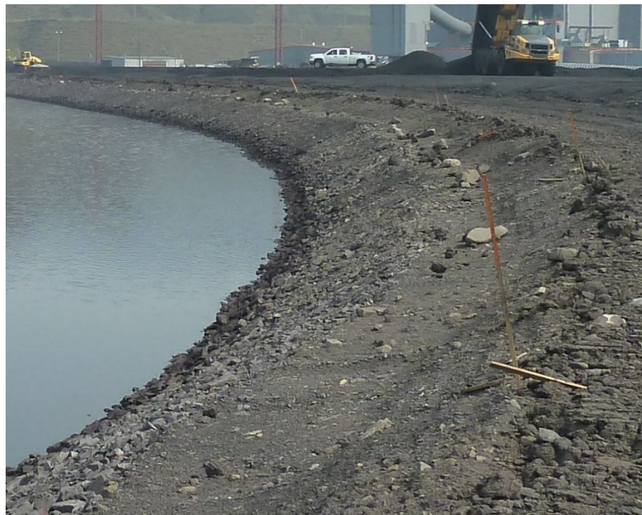
Photograph 6: Main Dam – upstream slope, looking northeast. 15 August 2018
