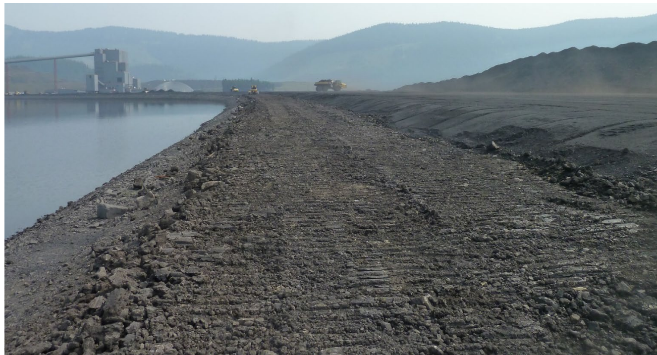
Photograph 8: Main Dam – overview from natural ground above west abutment, looking northeast. 15 August 2018.
