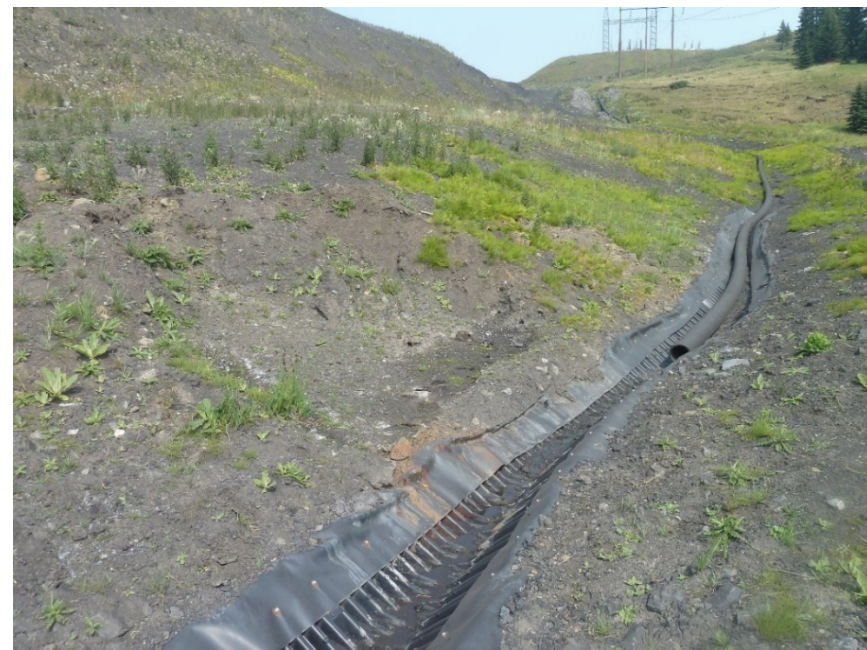
Photograph 11: Site C – view of seepage collection channel. Looking northeast. 15 August 2018.
