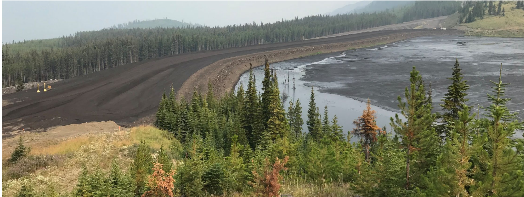
Photograph 16: West Dam – overview of upstream slope, looking northwest. 15 August 2018.
