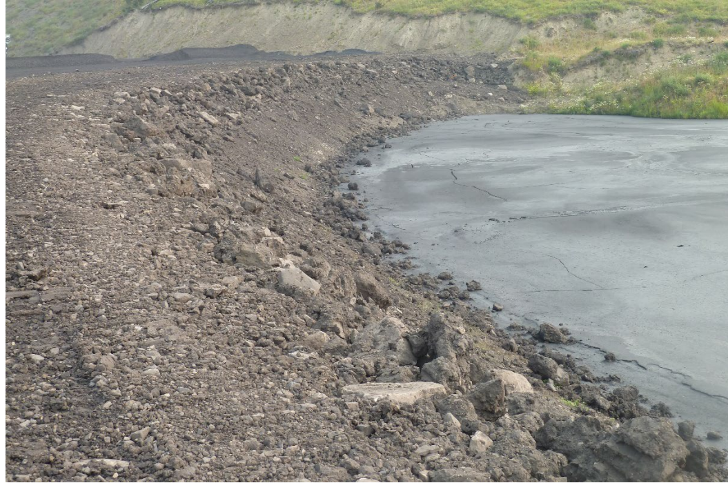
Photograph 22: West Dam – upstream slope and north abutment, looking north. 15 August 2018.
