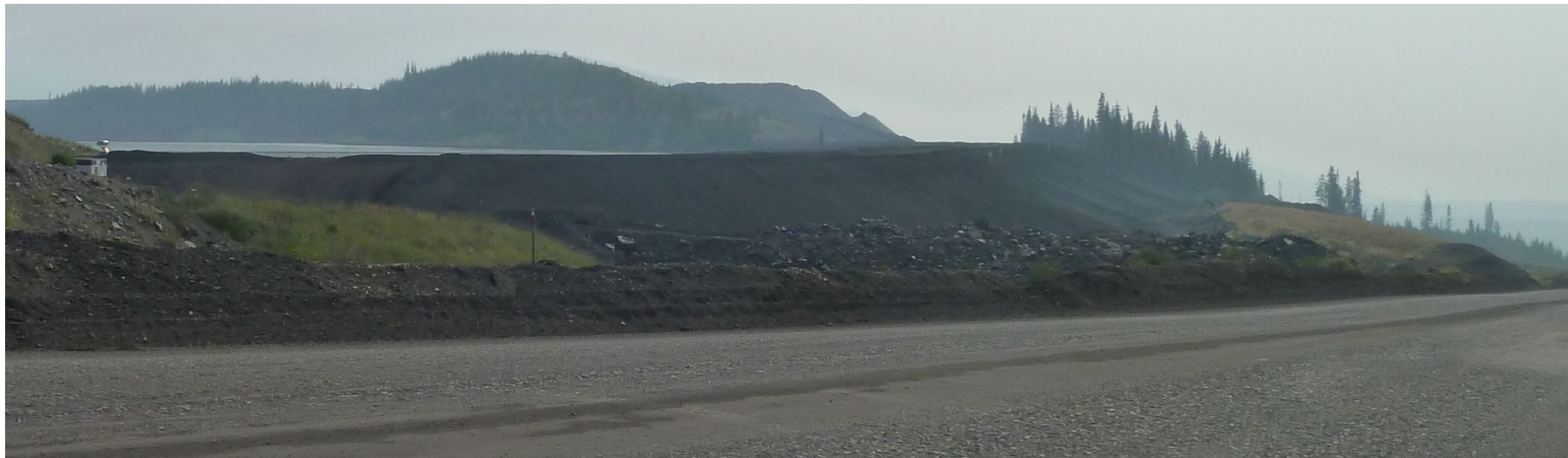
Photograph 17: West Dam – overview of downstream slope, looking south. 15 August 2018.
