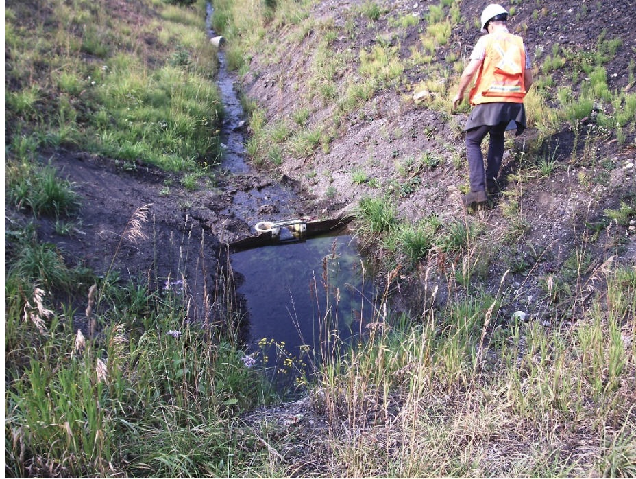
Photograph 224: West Dam – seepage weir downstream of West Dam. 15 August 2018
