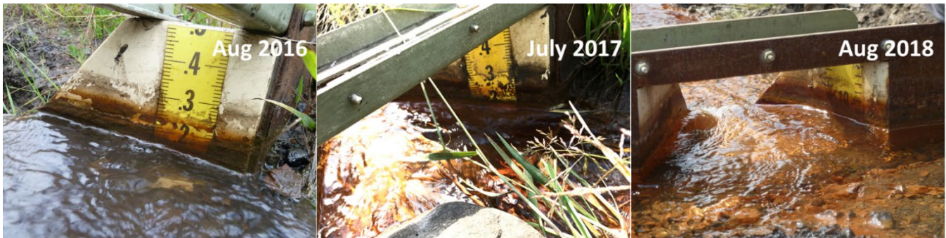
Photograph 1: Main Dam Seepage Comparison
