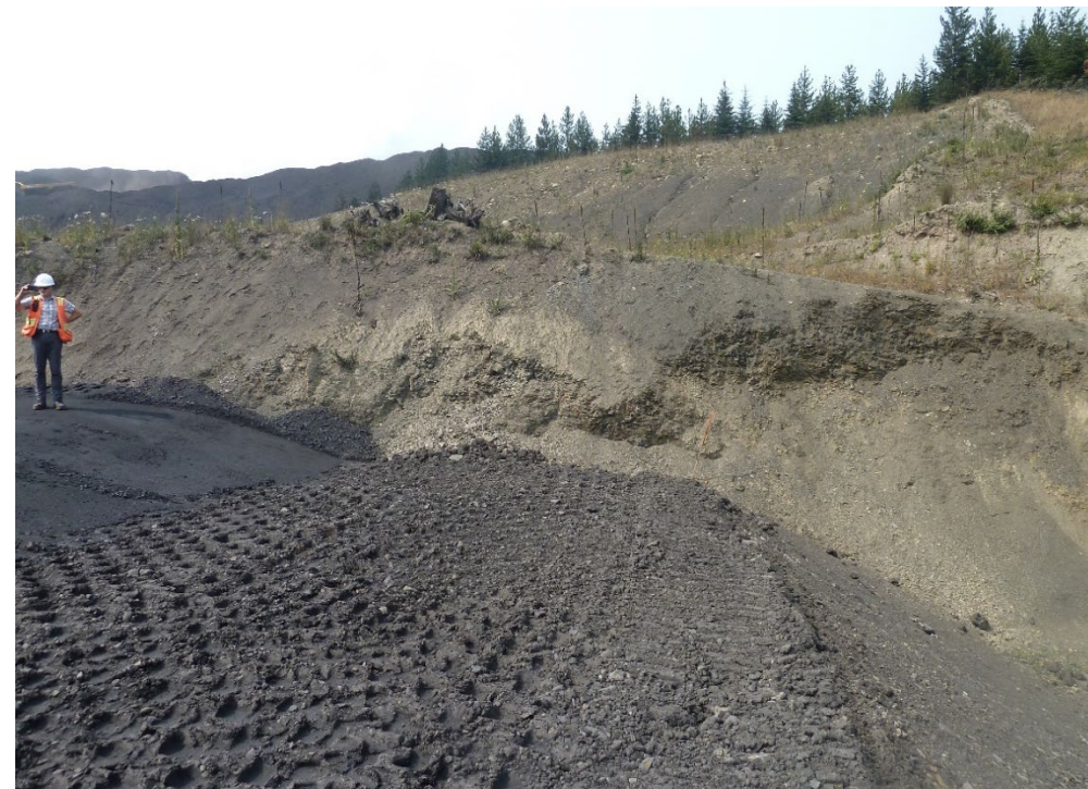
Photograph 9: Main Dam – west abutment, looking west. 15 August 2018.
