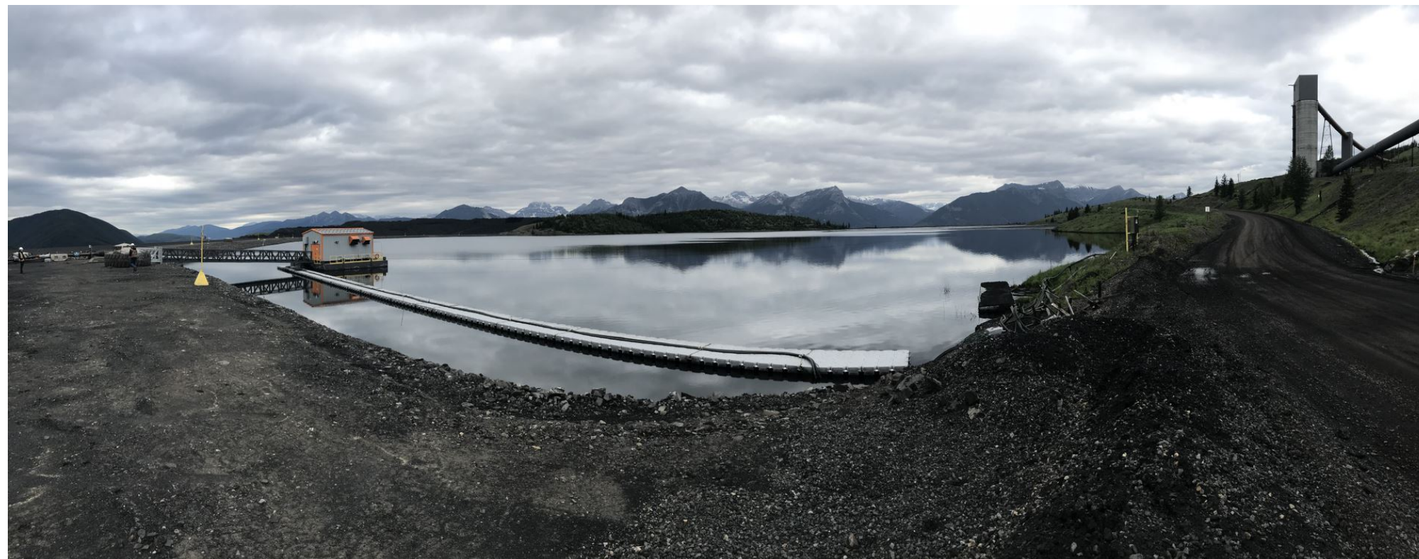
Photograph 2: Main Dam – overview of barge, looking southwest. 18 June 2018.
