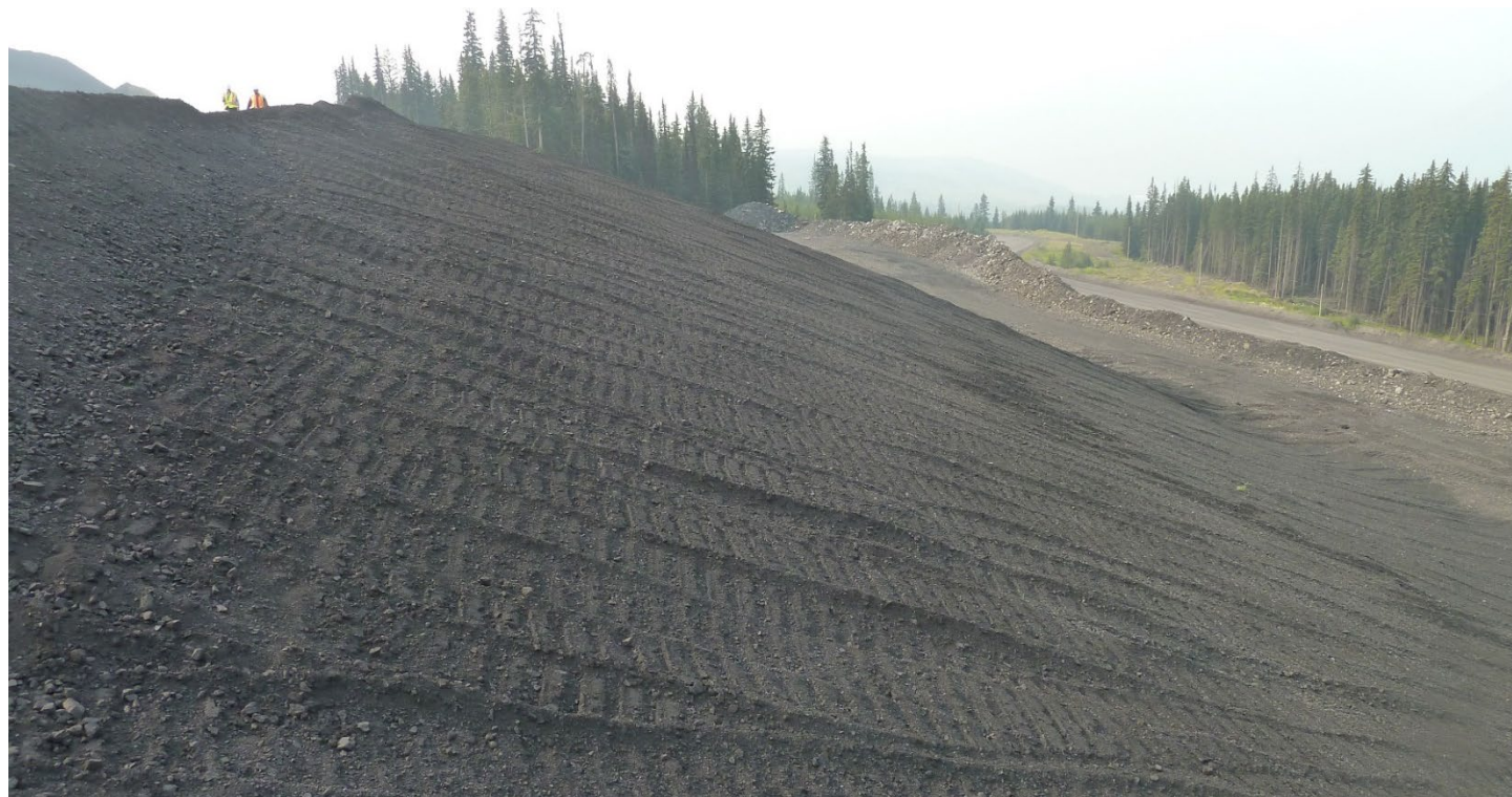
Photograph 19: West Dam – downstream slope, looking south. 15 August 2018.
