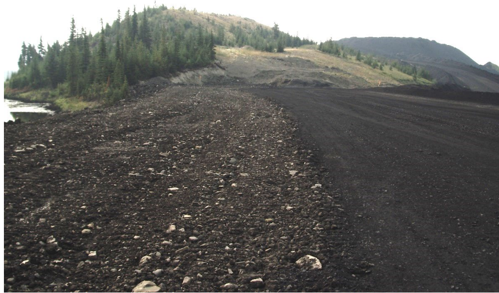
Photograph 20: West Dam – southern abutment, looking south. 15 August 2018.
