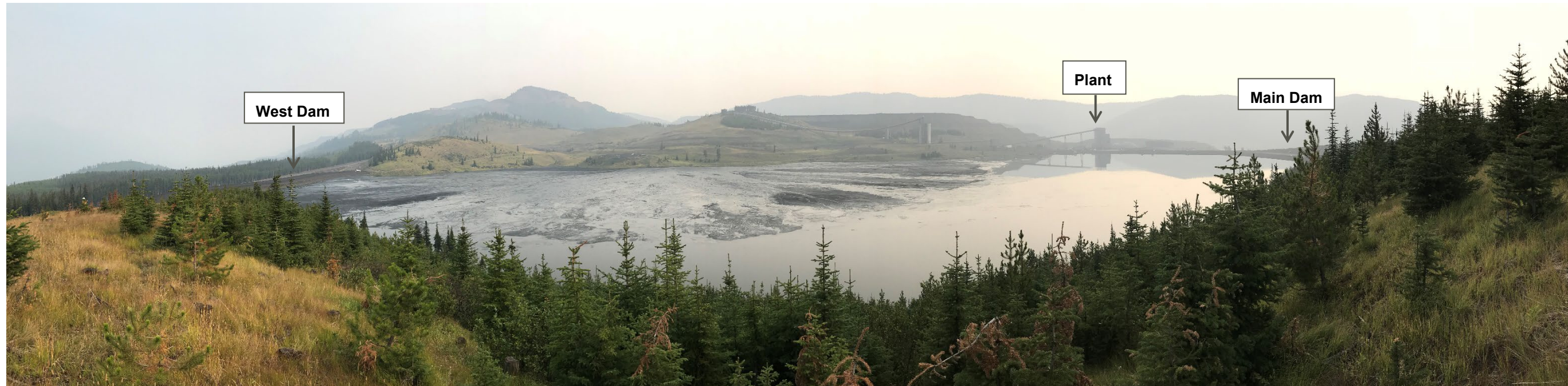
Photograph 1: Overview from rise of natural ground to the south, looking northeast. 15 August 2018.
