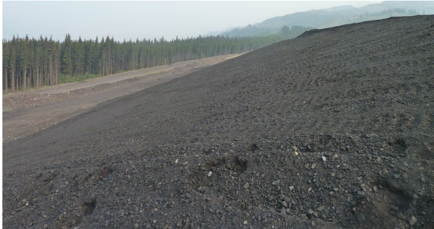
Photograph 18: West Dam – downstream slope, looking north. 15 August 2018.
