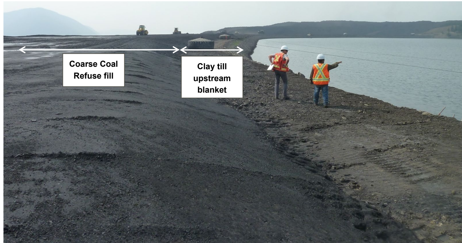
Photograph 3: Main Dam – crest, note clay till upstream blanket and coarse coal refuse fill, looking southwest. 15 August 2018.
