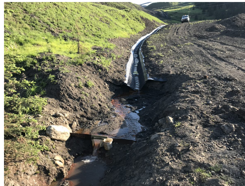
Photograph 12a: Site C – view of seepage collection channel. Looking northeast. 18 June 2018.
