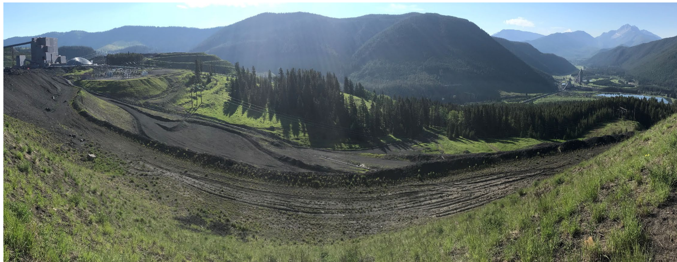
Photograph 15: Historic 2012 Site C failure scarp and toe bulge, looking east. No significant change since 2012. 18 June 2018.
