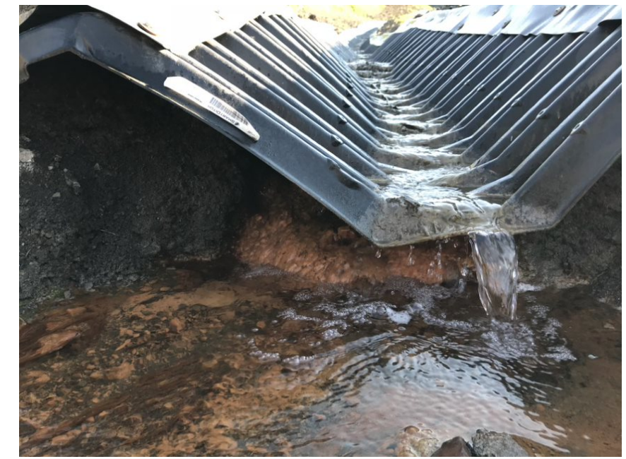
Photograph 12b: Site C –seepage under collection channel (red arrow), looking northeast. 15 August 2018.
