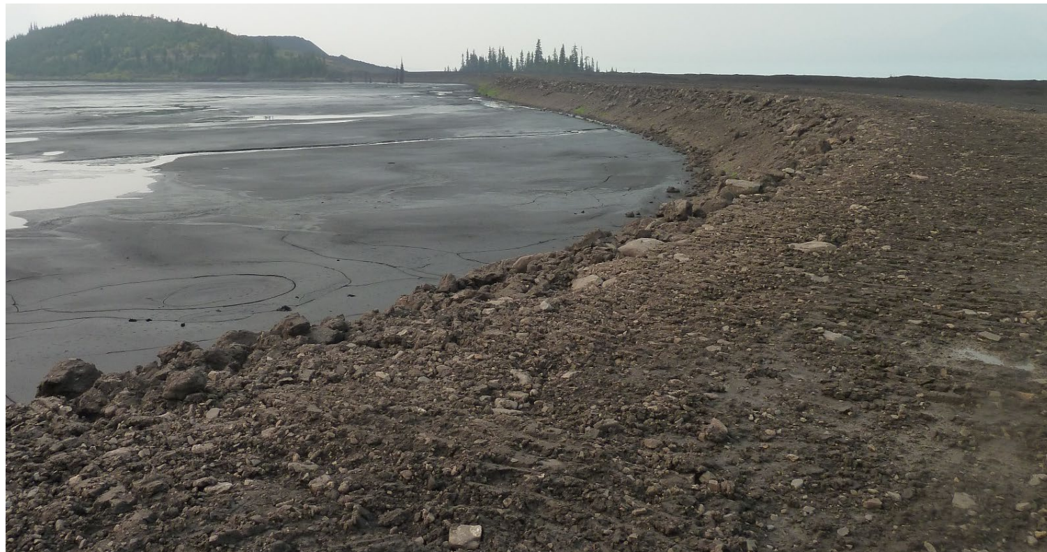
Photograph 213: West Dam – upstream slope and south abutment, looking south. 15 August 2018
