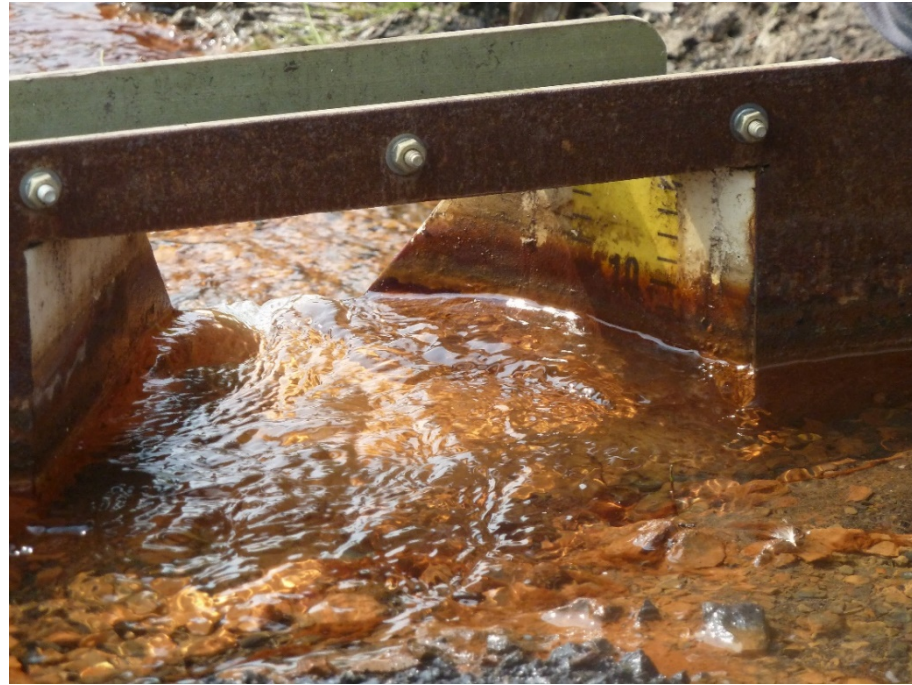
Photograph 13: Site C – weir at toe of Site C refuse spoil after trench upgrade, looking west. 15 August 2018.
