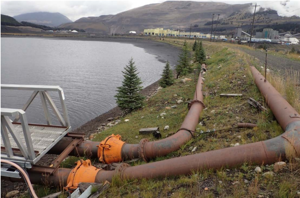
Photograph A-3: NTP dam upstream slope with small tress and vegetation growing, and unused reclaim pipes, looking northeast, 12 September 2018.
