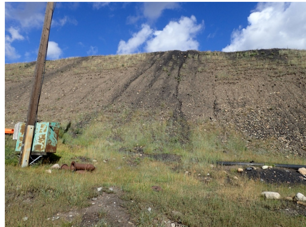
Photograph A-25: STP Main dam downstream slope from toe, showing area with on-going vertical erosion, 11 September 2018.
