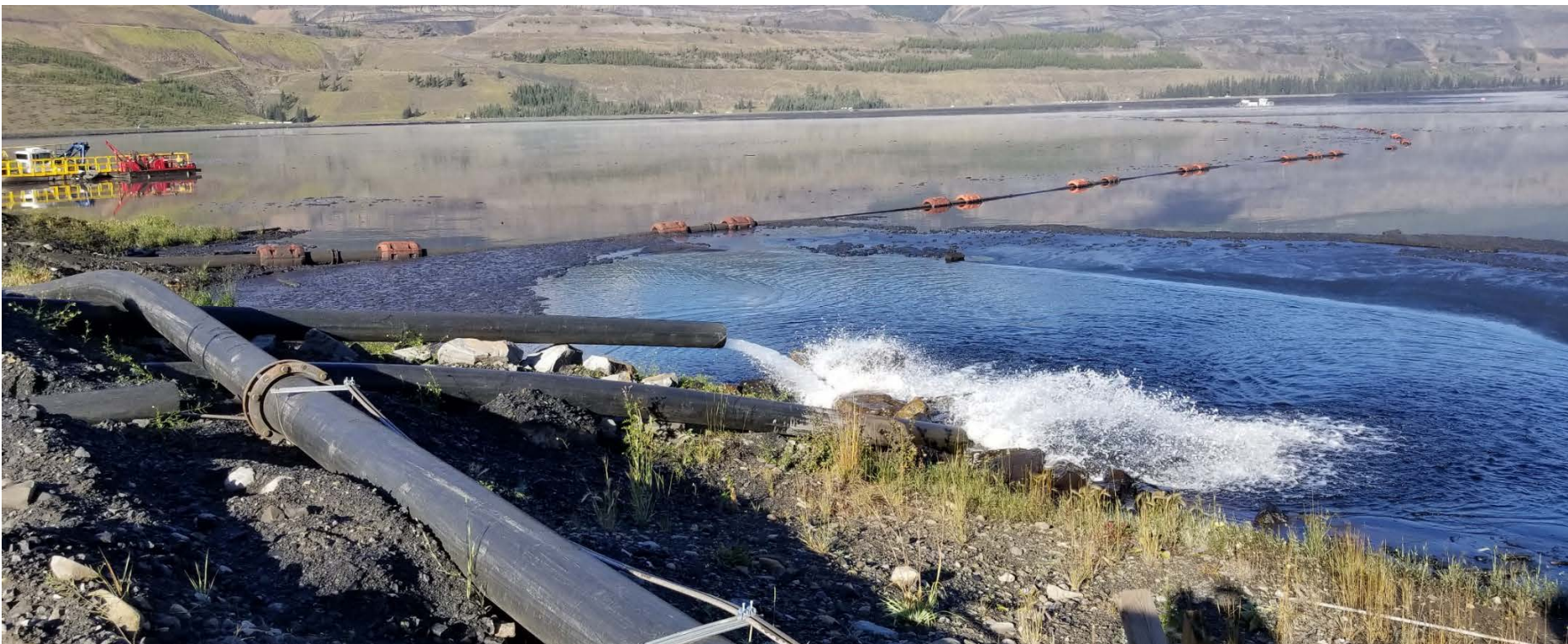
Photograph A-20: STP south abutment till blanket area, makeup waterlines from Kilmarnock Pond with riprap protection on blanket, looking northwest, 11 September 2018.
