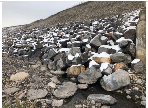
Photo 12: Looking upstream at STP riprap tie-in to pipe bridge abutment (approx. Sta. 0+650 to 0+685)
