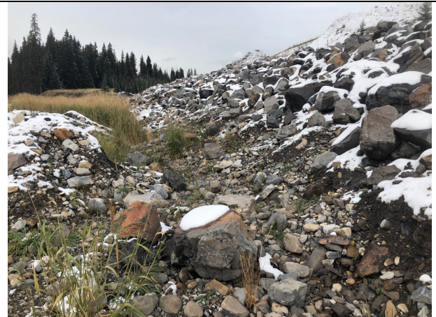
Photo 8: Looking upstream at STP riprap with minor erosion of gravel at the toe of the slope (approx. Sta. 0+300 to 0+325), no impact to riprap stability
