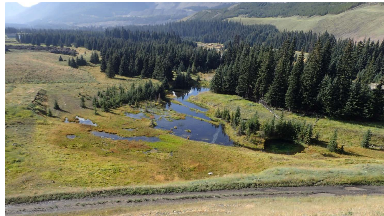
Photograph A-29: STP Main Dam, persistent ponding downstream of toe in old river channel, looking southwest, 11 September 2018.
