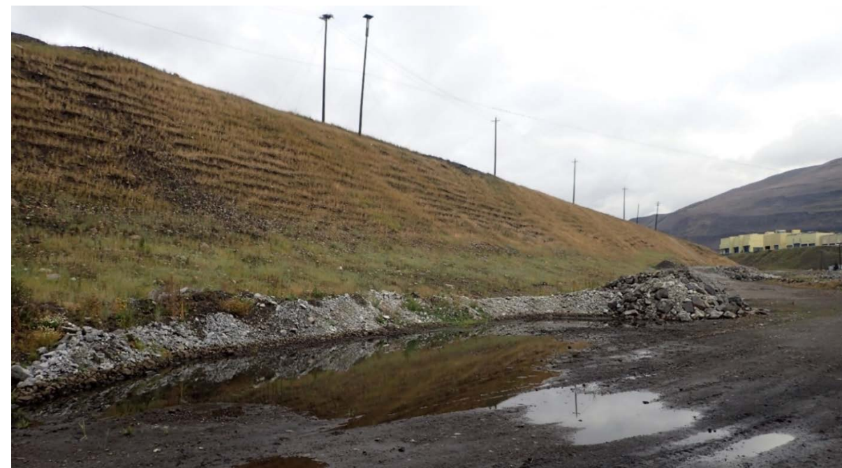
Photograph A-6: NTP dam downstream slope with stepped erosion and minor area of ponded water observed at the toe near Stn 0+970, looking northeast, 12 September 2018.
