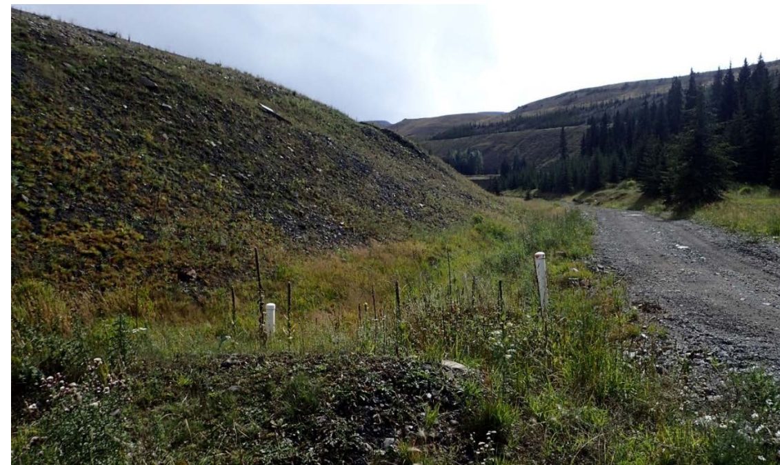
Photograph A-41: STP West Dam downstream slope with vegetation and ditch at downstream toe, looking south, 11 September 2018.
