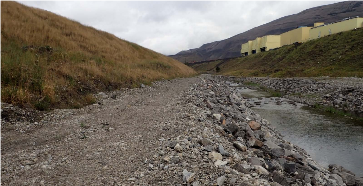
Photograph A-9: NTP downstream slope and toe near Stn 0+700, riprap along Fording River, looking northeast, 12 September 2018.
