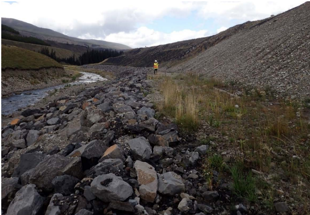
Photograph A-36: STP West Dam, riprap along dam toe, looking northwest, 11 September 2018.
