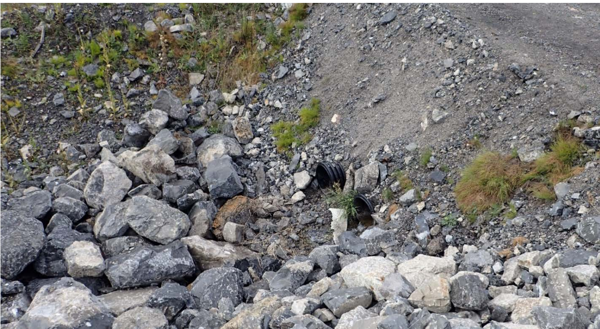
Photograph A-42: STP West Dam, twin culverts beneath access road at toe, looking east, 11 September 2018. The flow rate at the time of inspection was approximately 1.4 L/sec from the eastern pipe (closest to the page). The other pipe (further into the page) was dry.
