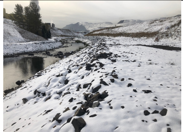
Photo 2: Looking downstream at NTP riprap covered by gravel (approx. Sta. 0+175 to 0+350)
