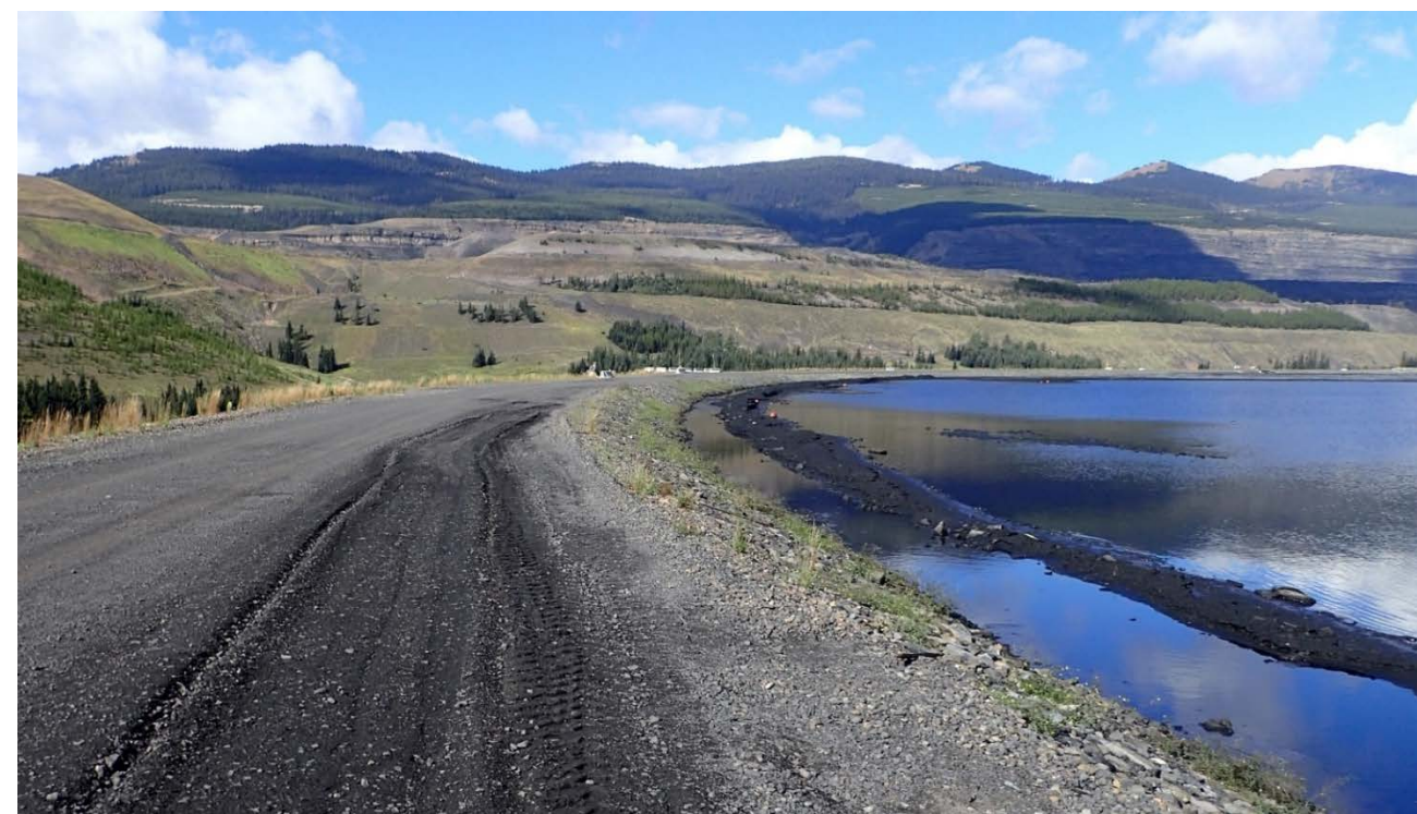
Photograph A-23: STP West Dam, crest and upstream slope with riprap, looking northeast, 11 September 2018.
