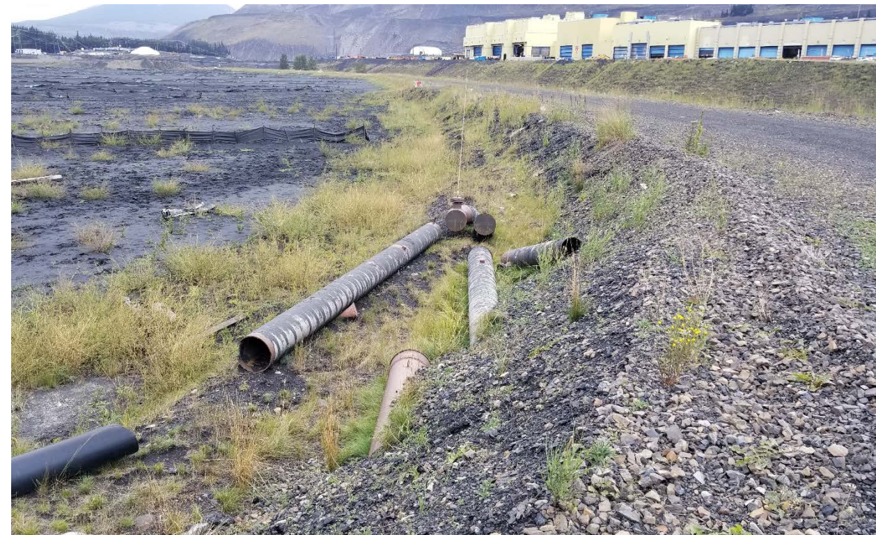
Photograph A-4: NTP unused reclaim pipelines on upstream slope, capped pipelines that go into dam section and crossing under crest, looking north, 12 September 2018.
