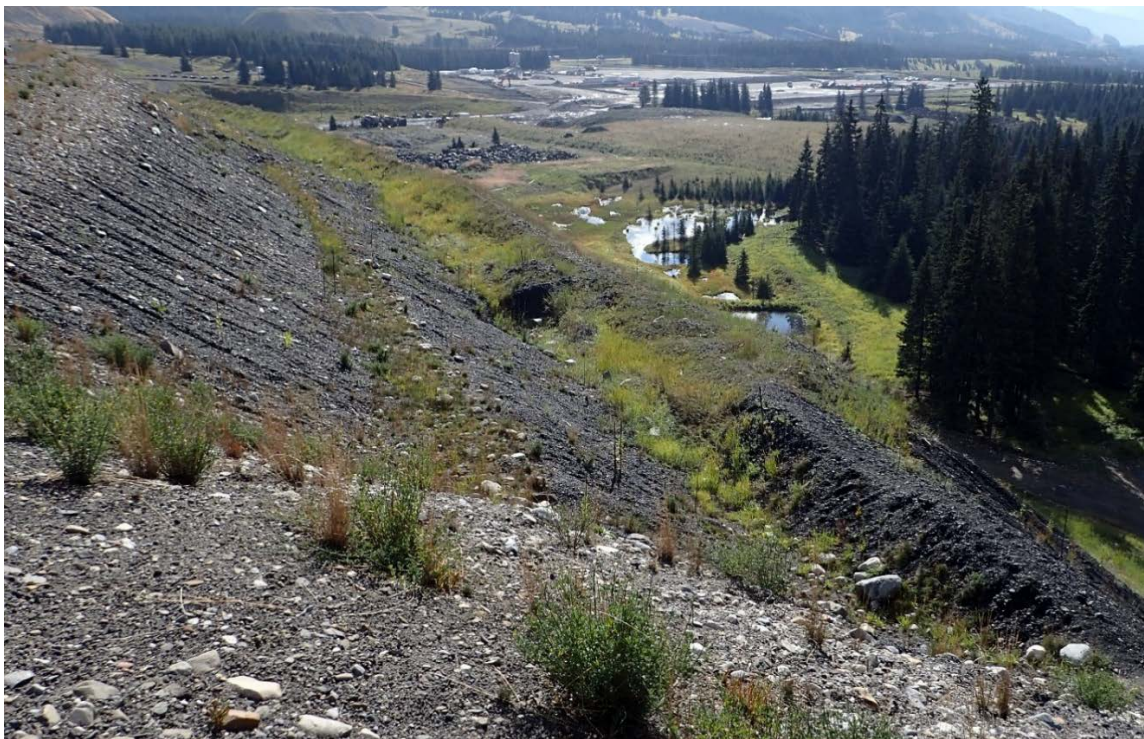
Photograph A-30: STP corner of West and Main dams, looking southeast. Vegetation not taking root in CCFR in this area, 11 September 2018.
