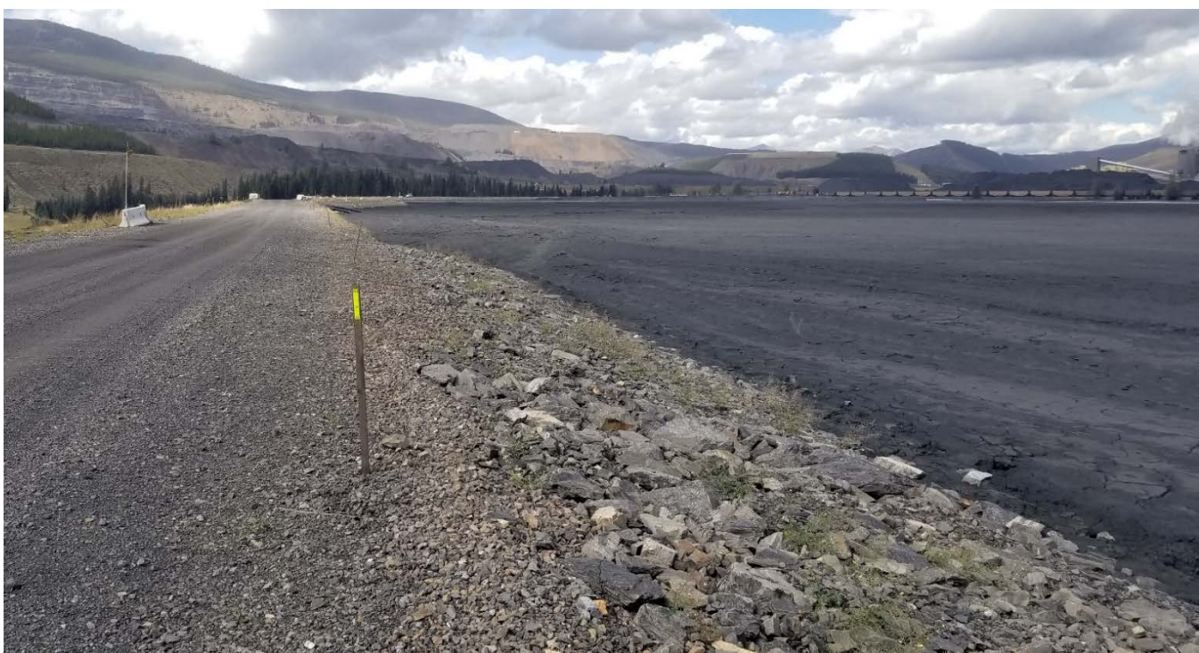
Photograph A-22: On STP Main Dam, upstream slope and riprap 1.4H:1V, looking west, 11 September 2018
