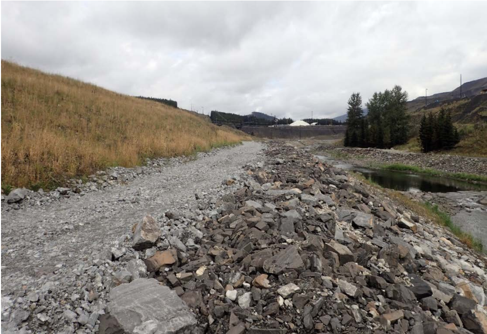
Photograph A-10: NTP downstream slope and riprap along Fording River, looking north, 12 September 2018.
