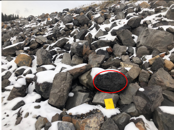
Photo 9: Riprap degradation due to weathering on a surface of a piece of riprap (red outline)
