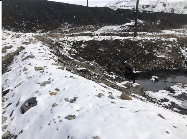
Photo 1: Looking upstream along alignment of NTP riprap that is buried (approx. Sta. 0+100)
