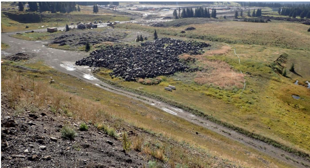
Photograph A-28: STP Main Dam, looking south at riprap emergency stockpile and Fording River flood plain, 11 September 2018.
