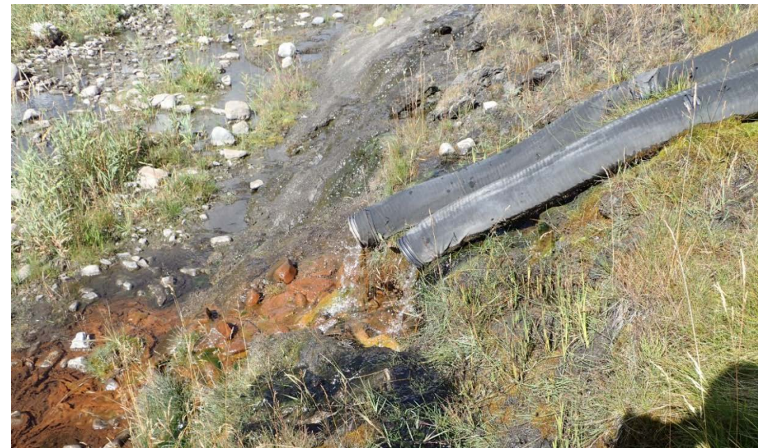
Photograph A 33: On slope of STP West Dam access road, seepage collection point along the downstream slope (Stn. 1+000). Seepage collection points monitor flow. Note discolouration. The flow rate at the time of inspection was approximately 0.21 L/sec from the south pipe (closer to the page) and 0.26 L/sec from the north pipe (further into the page). 11 September 2018.
