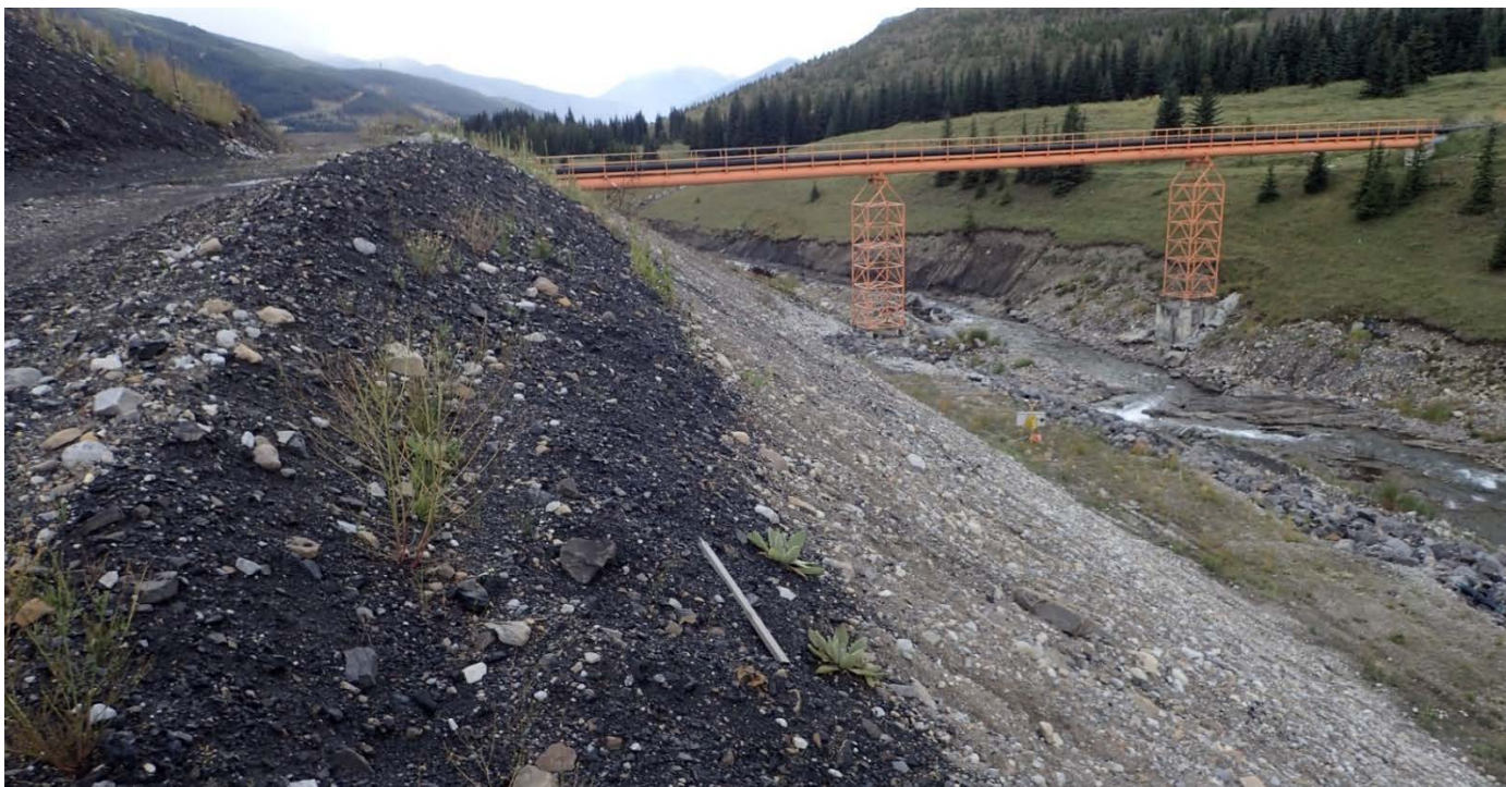
Photograph A-40: STP unused dredge pipeline to 2P-3P TSA on pipe bridge and West Dam access road's downstream slope, looking southeast, 11 September 2018.
