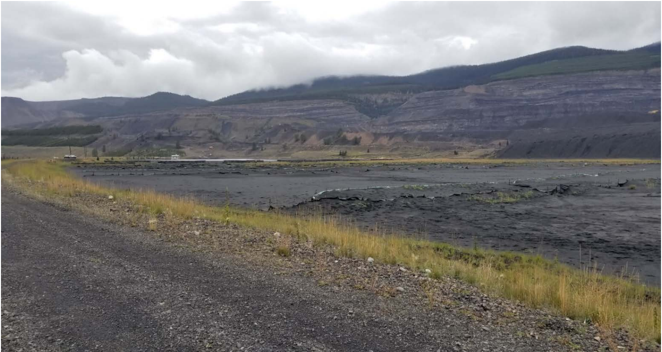
Photograph A-8: NTP, tailings surface with silt fencing for dust control, looking southwest, 12 September 2018.
