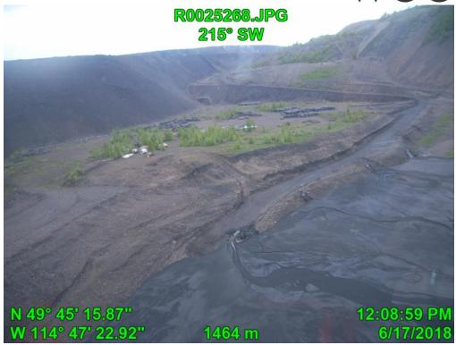
Photograph F - 3: Showing an aerial view of tailings pipelines and tailings beaching at the WTFT, looking west.
