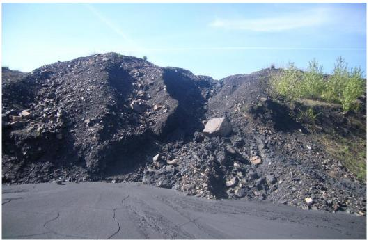
Photograph F - 11: Showing an erosion gully on upstream slope due to tailings discharged from spigot 1 pipe located close to the Adit dump, looking south. (Photo R0018422, 06/06/2017)
