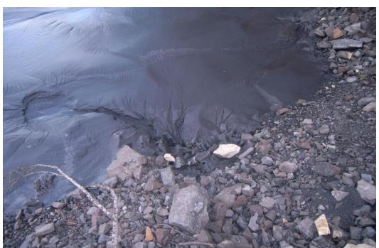
Photograph F - 15: Showing seepage at the east abutment against the 2013 raised, looking north. (Photo R0018375, 06/06/2017)
