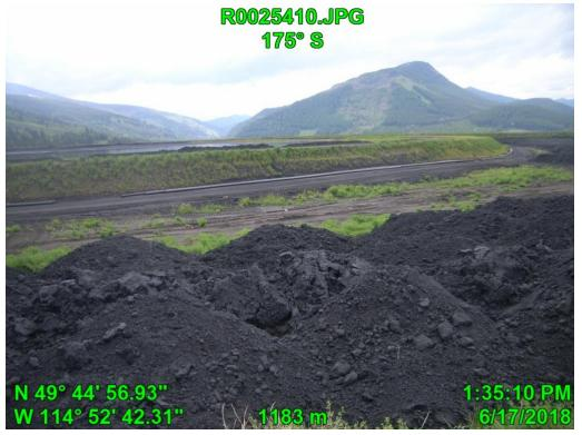
Photograph J - 23: Showing surface of the west corner of Lagoon D, looking south. Noted active tailings deposition on the surface
