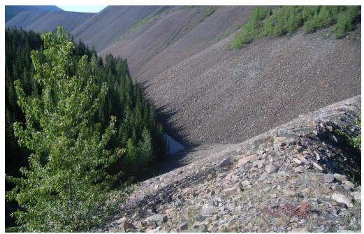
Photograph F - 20: Showing toe of Cowboy dump looking south. Note toe is located approximately 450 m downstream of crest centerline. (Photo R0018407, 06/07/2017)
