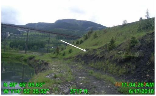
Photograph J - 15: Showing the toe and lower section of north slope of Lagoon D, looking northeast. Note erosion at the toe.
