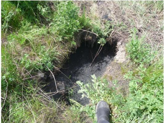
Photograph J - 27: Showing a sinkhole at south west crest of Lagoon D, looking east. (Photo P1100730, 2017/06/06).
