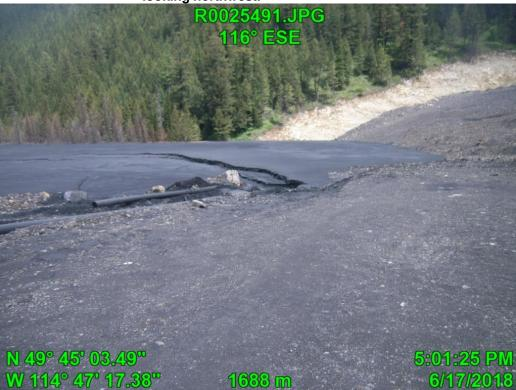
Photograph F - 8: Showing beach tailings on upstream, looking southeast from west abutment.
