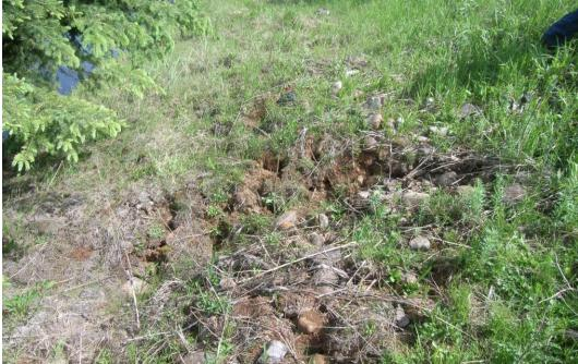
Photograph J - 20: Showing an animal activity at the toe of the north slope of Lagoon D, looking northwest. (Photo R0018710, 06/07/2017
