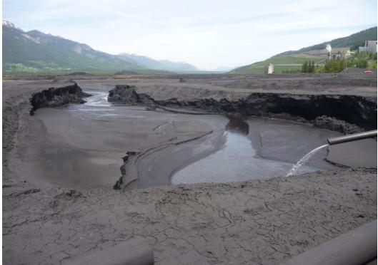
Photograph J - 34: Showing a tailings cell at southeast section of Lagoon D, looking northeast. (Photo P1100742, 2017/06/07)
