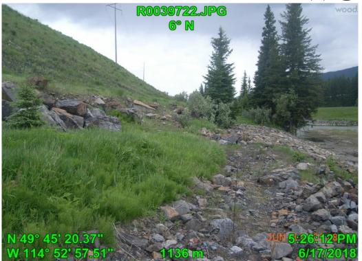
Photograph I - 23: Showing erosion riprap along the shoreline of the Elk River, at the west toe of Lagoon C, looking southwest.
