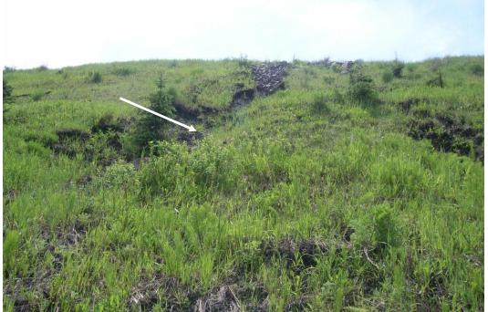
Photograph J - 13: Showing erosion gully at lower north slope, looking south up from the toe. (Photo R0018766, 06/07/2017)
