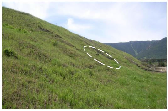
Photograph J - 10: Showing the toe and the 2<sup>nd</sup> seep area at the east end of North toe of Lagoon D, looking west. (Photo R0018807, 06/07/2017)
