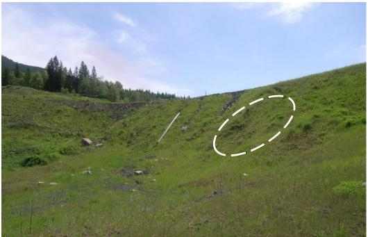
Photograph J - 11: Showing a close-view of the first seep area on the north slope, looking southeast. (Photo R0018808, 06/07/2017)
