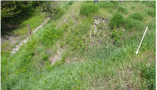
Photograph H - 8: Showing a pipeline at the toe at south end of the west embankment and an erosion gully, looking north. (Photo No. P1100775, 2017/06/07)
