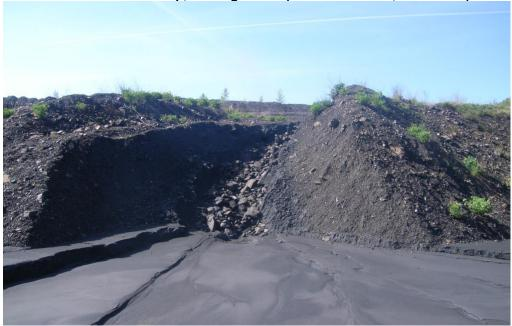
Photograph F - 12: Showing an erosion gully on upstream slope due to tailings. (Photo R0018425, 06/06/2017)
