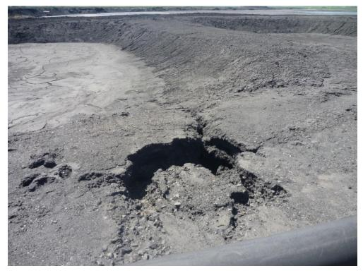
Photograph J - 8: Showing a close-view of a sinkhole within the tailings cell of Lagoon D, looking south.
