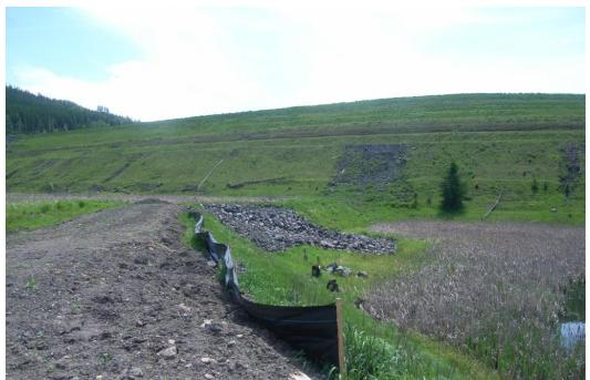
Photograph G - 4: Showing west berm and the spillway, looking southeast. (Photo R0018844, 06/07/2017)
