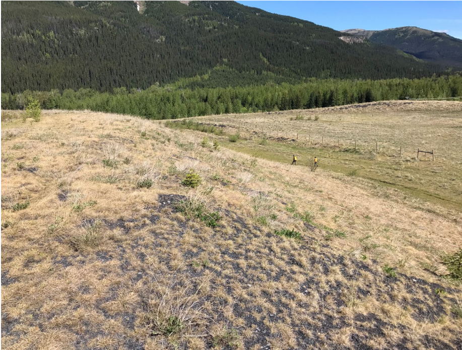
Photo II-14 Overview of the lower downstream slope – looking north. Photo was taken standing on the mid-slope bench. No signs of distress (BTD-2018-11)
