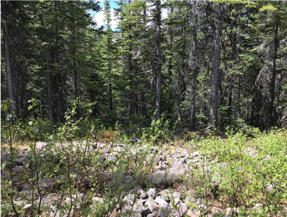
Photo II-34 End of riprap along channel at spillway outfall – looking downstream. Spillway discharges over a natural steep slope (BTD-2018-26)
