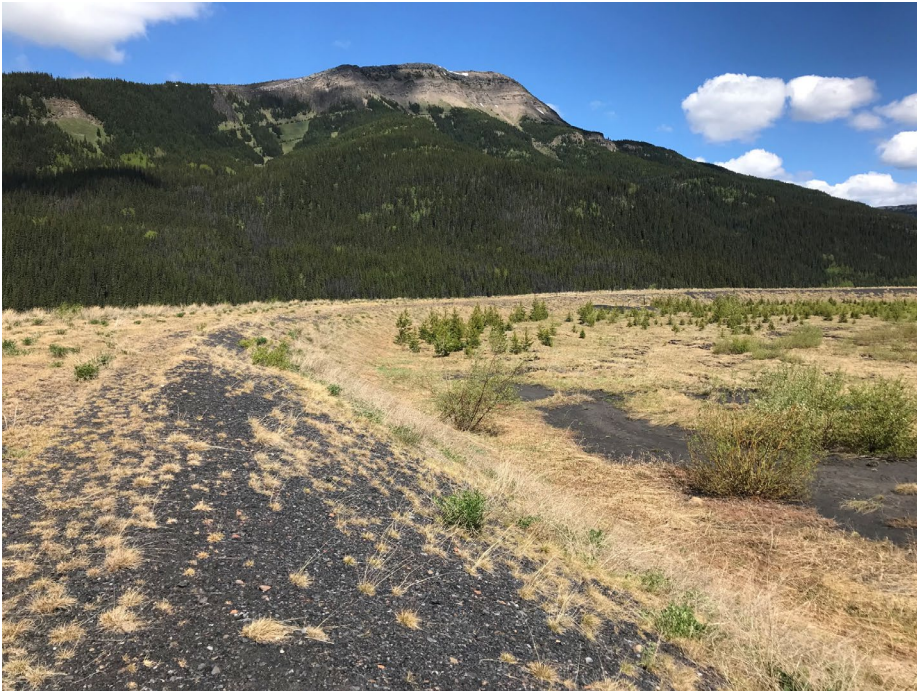
Photo II-23 Upstream slope – looking north. Slope is in good condition with no signs of erosion or movement (BTD-2018-18)
