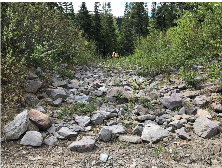
Photo II-33 Spillway channel looking downstream after transition from bedrock to riprap. Channel is armoured with riprap on the invert and side slopes (BTD-2018-25)
