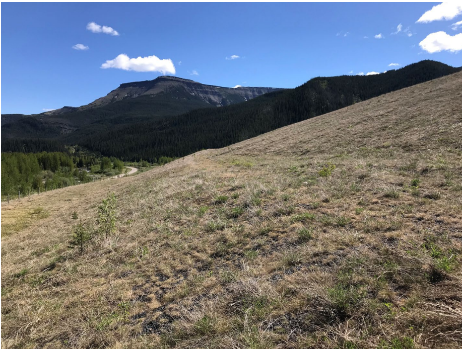
Photo II-19 Overview of the downstream slope – looking east. Slope is in good condition with no signs of erosion or movement (BTD-2018-14)
