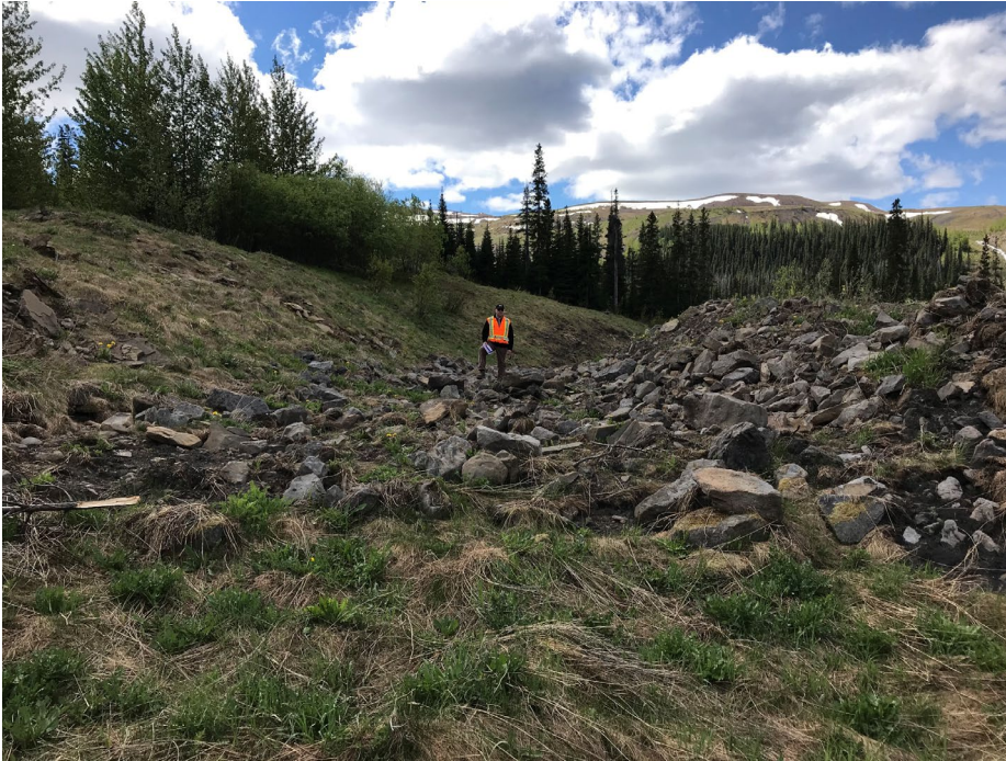
Photo II-26 Spillway inlet – looking southwest. Vegetation was removed in 2017; no major obstruction (BTD-2018-21)
