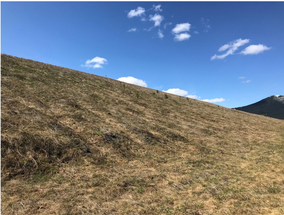
Photo II-17 Upper portion of the downstream slope – looking north. Slope is in good condition with no signs of erosion or movement (BTD-2018-13)
