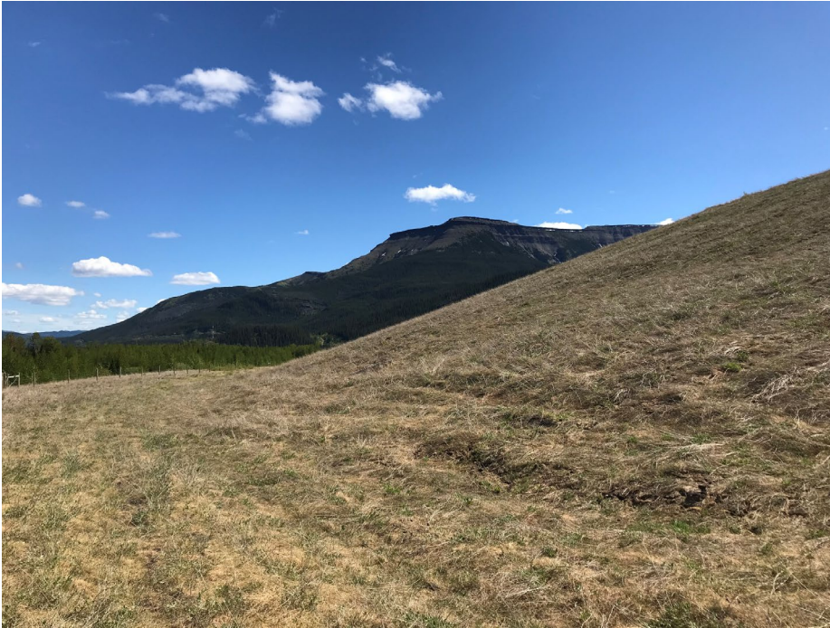
Photo II-22 Downstream slope – looking east. Slope is in good condition with no signs of erosion or movement (BTD-2018-17)
