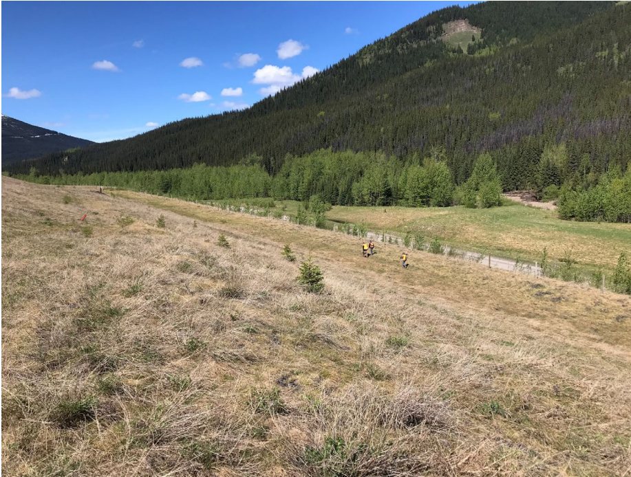
Photo II-18 Lower portion of the downstream slope – looking west. Slope is in good condition with no signs of erosion or movement (BTD-2018-14)
