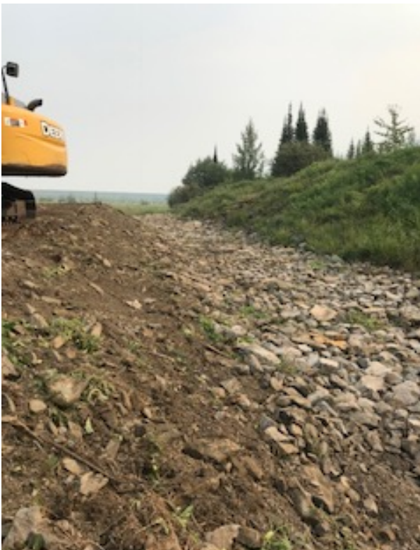
Photo II-37 Teck repaired disturbed riprap on August 15, 2018 – looking northeast
