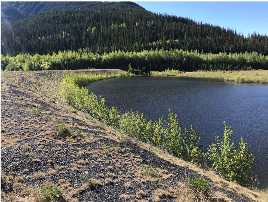
Photo II-5 Overview of ponded area. Pond level appears to be elevated due to spring freshet - higher than previous year observation (not a dam safety concern) (BTD-2018-03)
