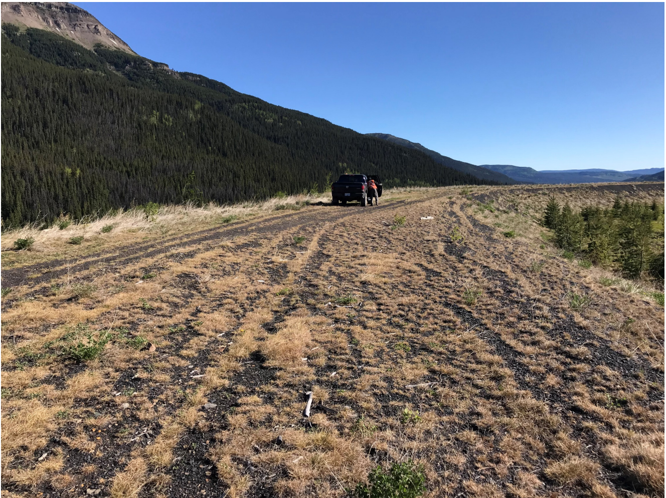
Photo II-1 Overview of BTD crest – looking east. Slope is in good condition and no signs of erosion, settlement or cracking (BTD-2018-01)
