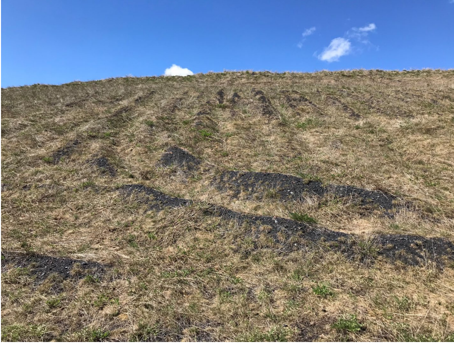
Photo II-16 Overview of the upper portion of the downstream slope – looking southwest. Possible slope break observed likely due to normal soil erosion and rilling (BTD-2018-12)
