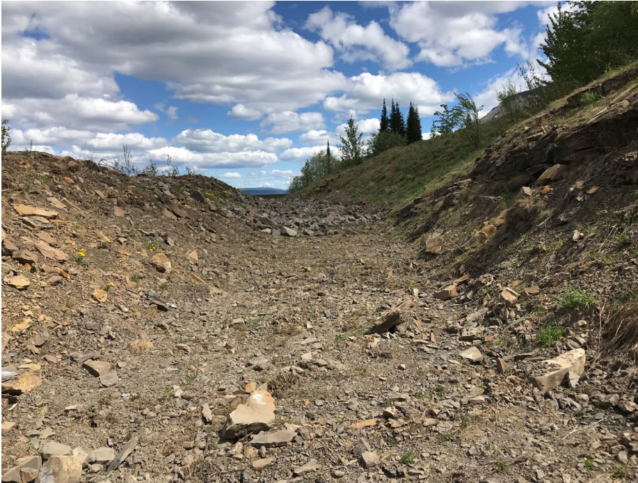
Photo II-30 Spillway channel section founded on bedrock – looking upstream. No obstruction was observed (BTD-2018-24)
