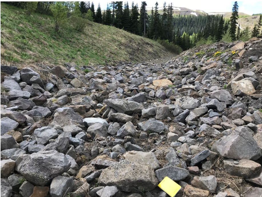
Photo II-27 Spillway channel – looking southwest. Vegetation clearing activity disturbed riprap materials. Photo was taken before repair work was completed (BTD-2018-22)
