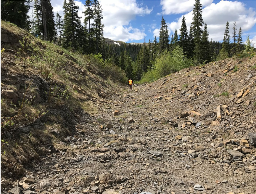
Photo II-32 Spillway channel - looking downstream where channel transitions from riprap lined (invert and right bank) and bedrock (left bank) to channel being entirely in bedrock (BTD-2018-24)
