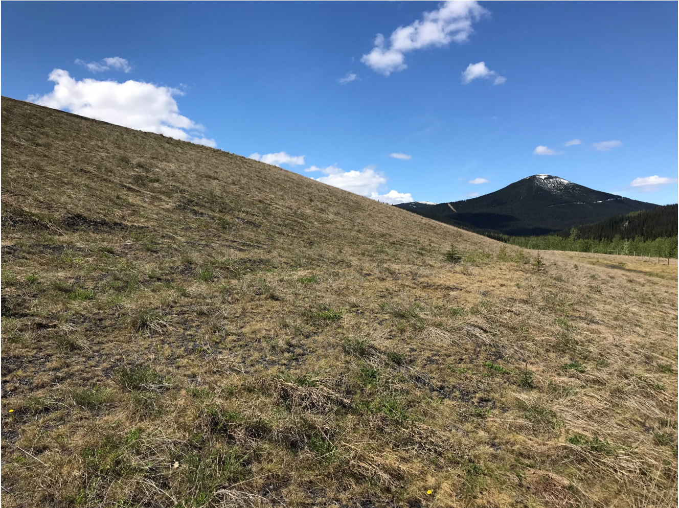
Photo II-20 Overview of the downstream slope – looking west. Slope is in good condition with no signs of erosion or movement (BTD-2018-15)
