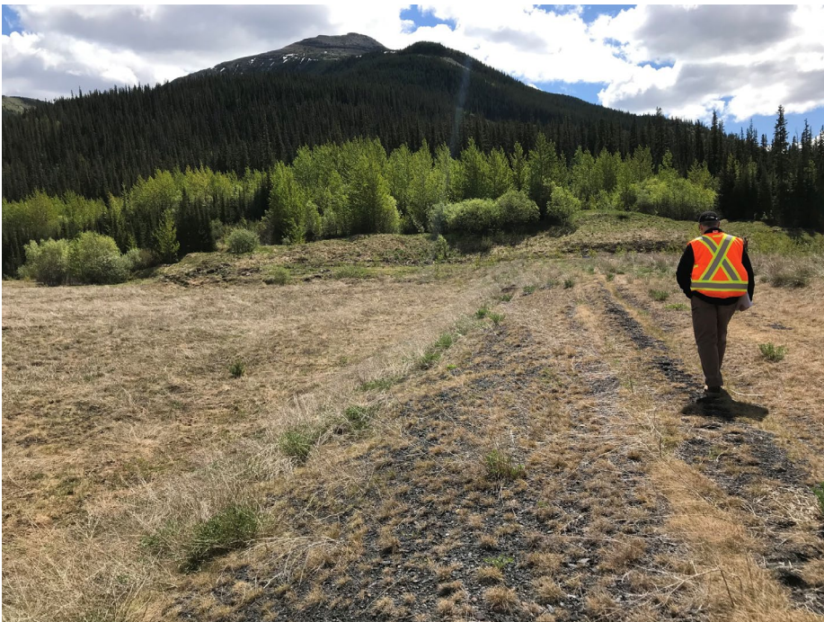
Photo II-25 Upstream slope – looking southeast. Tailings surface elevation is approximately 1.5 m lower than the crest elevation (BTD-2018-20)
