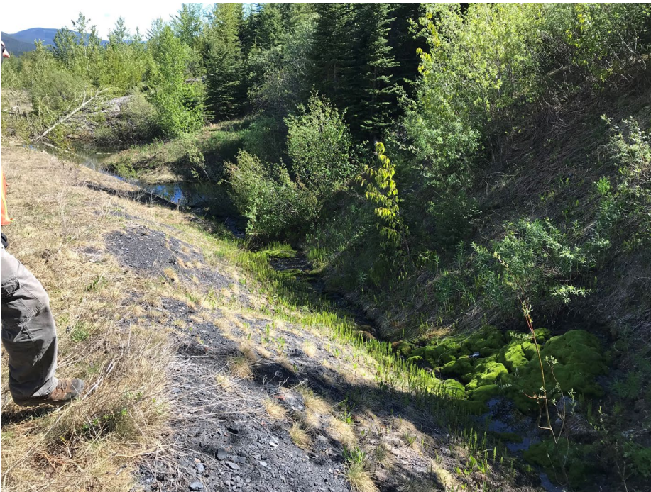
Photo II-11 Side channel which runs downslope from the east abutment – looking northeast. Flow was approximately 1 L/min (BTD-2018-08)
