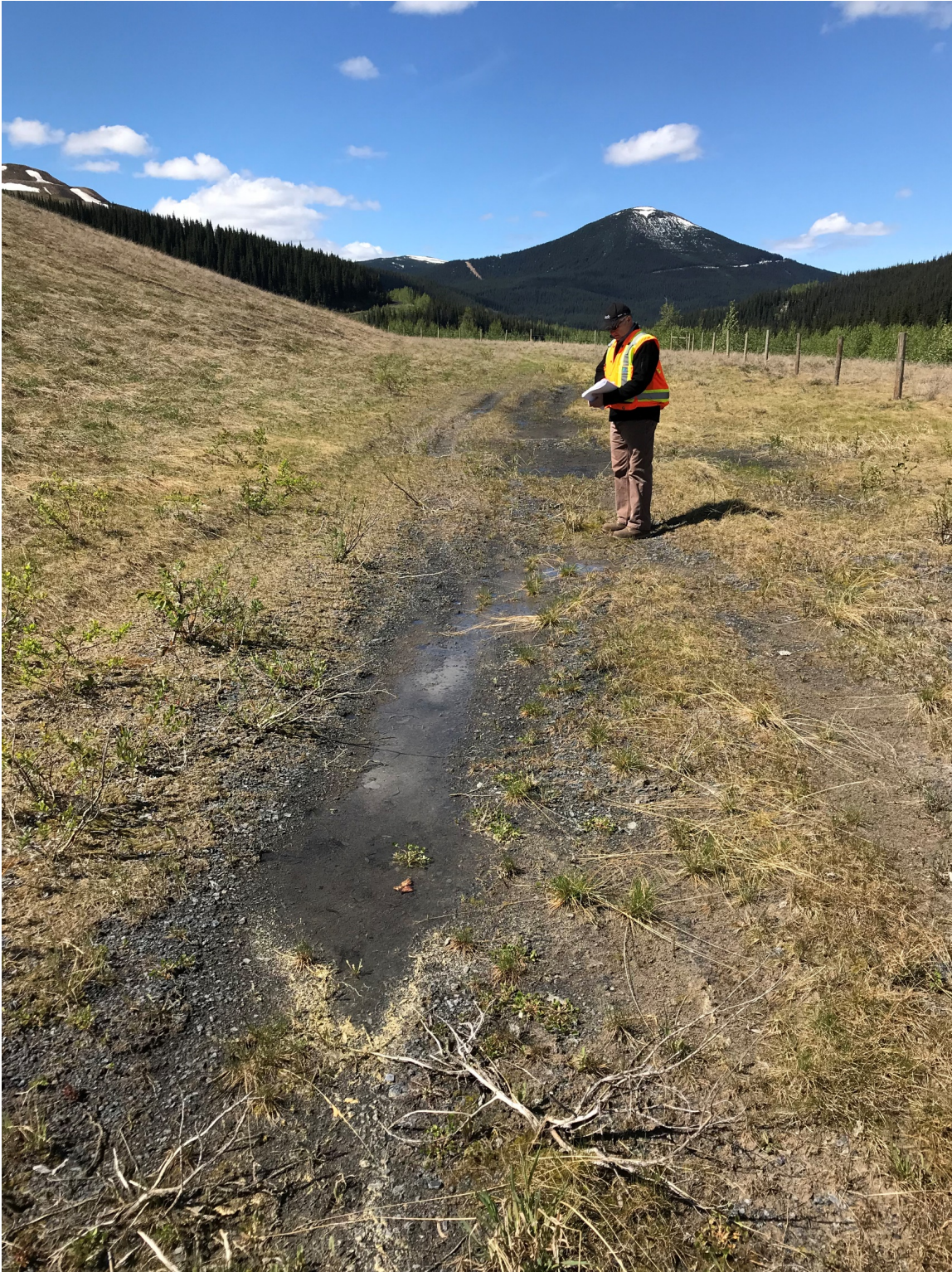
Photo II-21 Boggy area observed at the toe – looking west. Ponded water likely due to recent freshet (BTD-2018-16)
