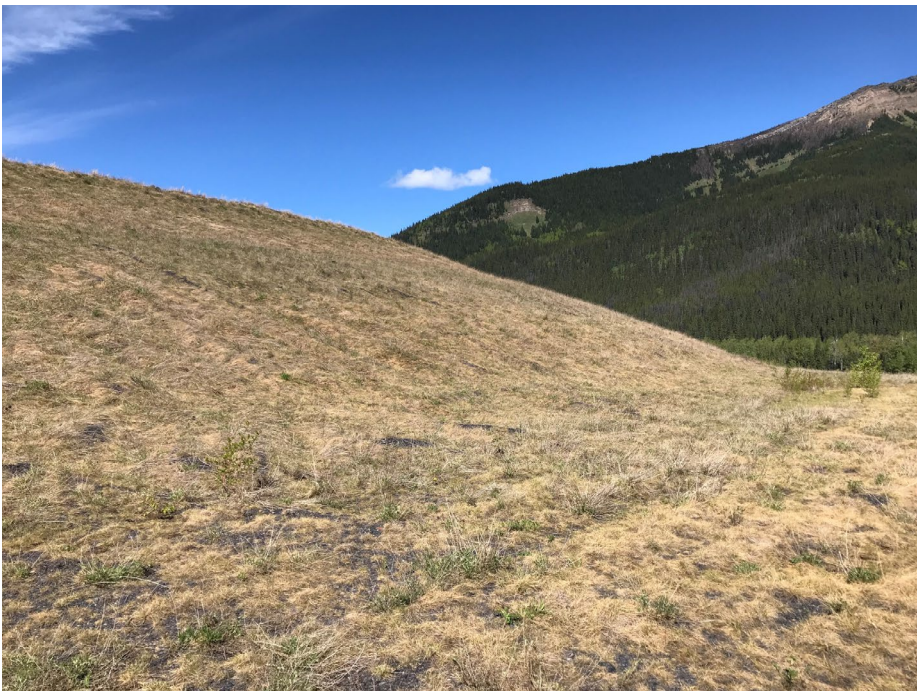
Photo II-15 Overview of the upper downstream slope – looking northwest. Photo was taken standing on the mid-slope bench. No signs of distress (BTD-2018-12)
