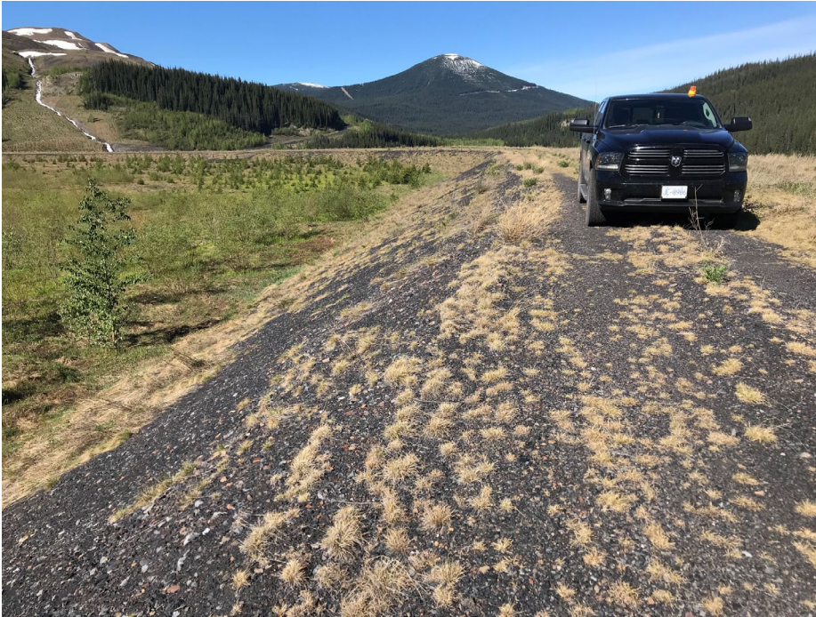
Photo II-4 Overview of upstream slope - looking southwest. Slope is in good condition and no sign of distress (BTD-2018-02)
