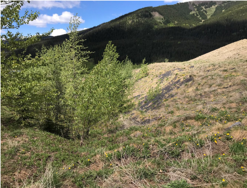
Photo II-36 Toe of the dam along west slope is approximately 1.5H:1V – looking north. The slope appears to be stable with no significant sign of erosion or movement (BTD-2018-28)
