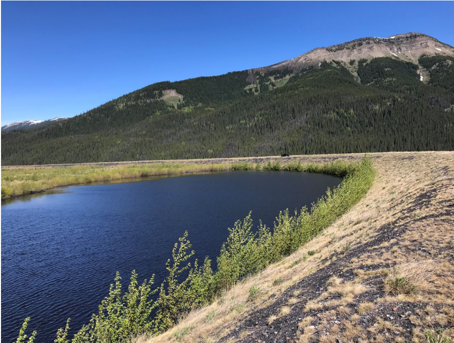
Photo II-8 Overview of upstream slope adjacent to the ponded area - looking northwest. Slope is in good condition and no signs of distress (BTD-2018-05)
