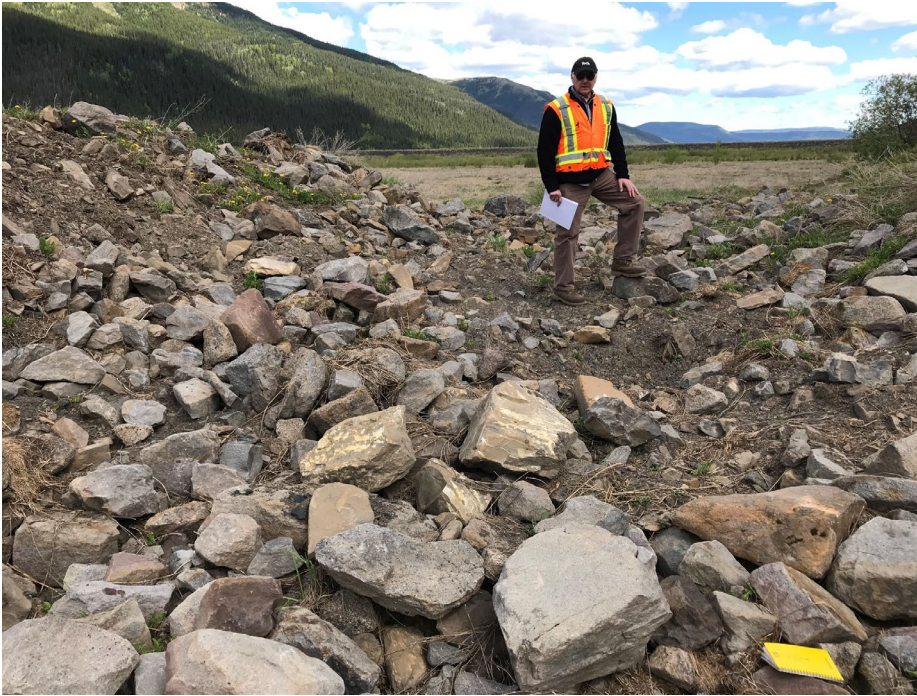
Photo II-28 Disturbed riprap overview – photo was taken during the DSI site visit (BTD-2018-22)
