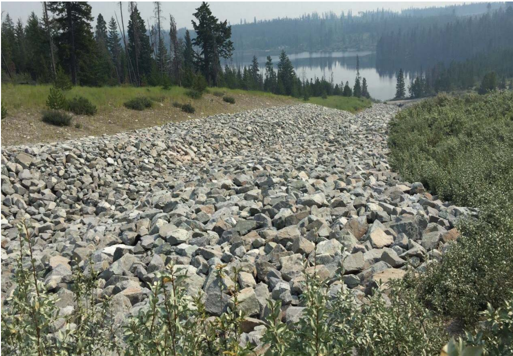
Photo II-B-10 Spillway channel, looking northwest (upstream) at Bose Lake Dam (BTH-2018-14)
