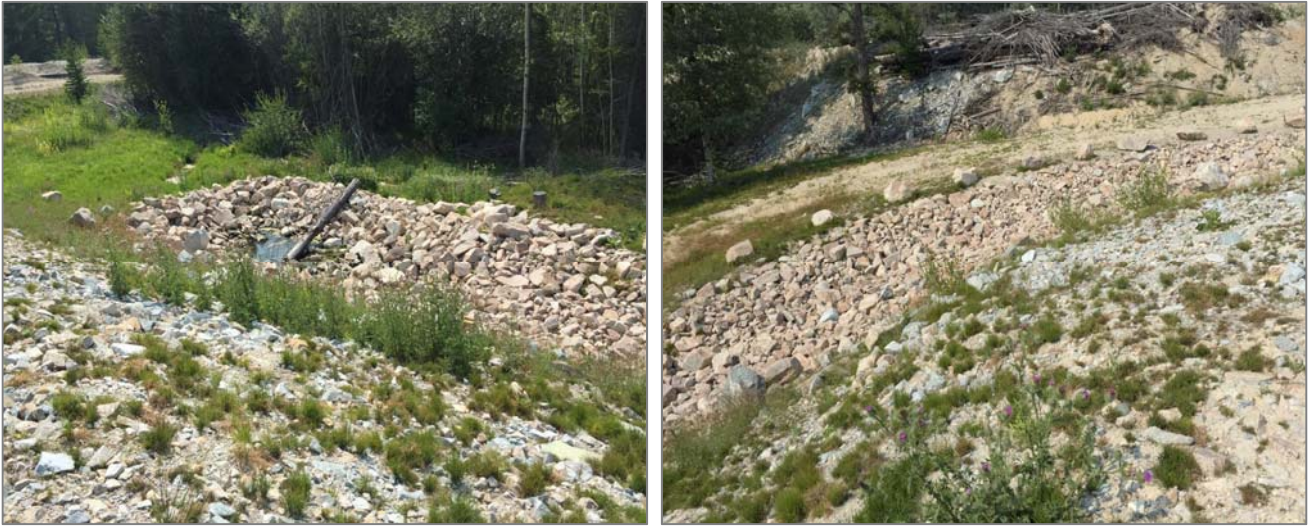
Photo II-C-4 Pond and debris fence for low-level outlet (BTH-2018-21)
