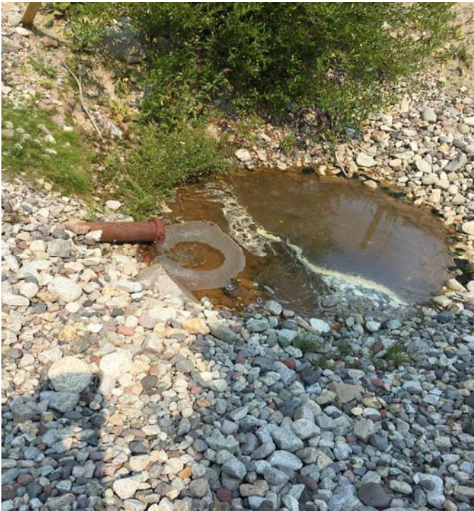
Photo II-B-15 Seepage outflow to riprap lined infiltration basin (BTH-2018-17)
