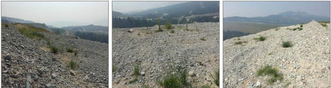
Photo II-A-7 Cracks (two separate instances shown in pictures below) on crest of rockfill placed in September 2015 as part of erosion gully repair. (BTH-2018-07)
