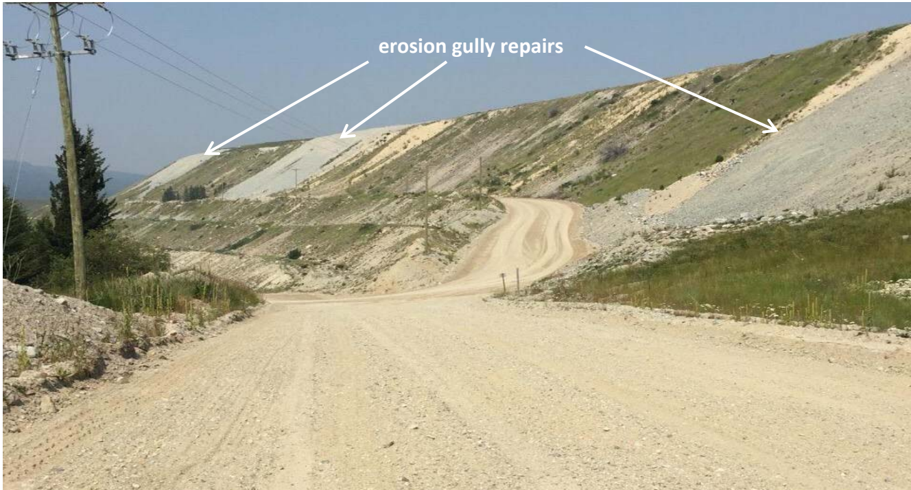
Photo II-A-5 Downstream slope of Dam No. 1, looking west from R3 Seepage Pond. (BTH-2018-05)
