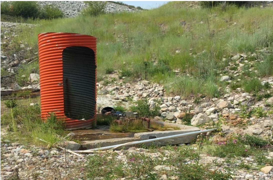
Photo II-B-14 Old gauge-house and decommissioned pump-well (BTH-2018-17)
