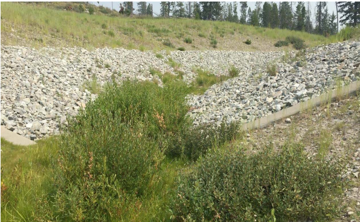
Photo II-B-8 Spillway channel at transition point between inlet and riprap-lined segment, looking southeast (downstream) towards Bose Lake (BTH-2018-12)
