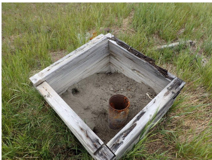
Photograph 15: South TSF, Cell 5, backfilled decant tower, looking northeast. 14 June 2018.
