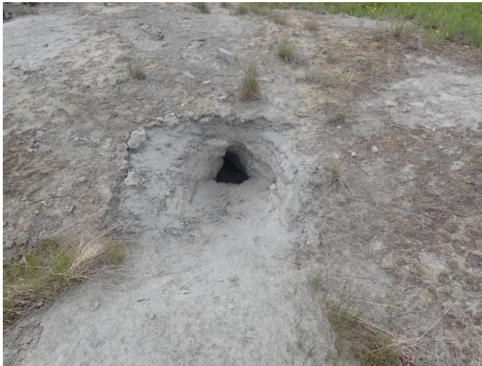
Photograph 47: North TSF, Cell 6, animal burrow in tailings surface, looking east. 14 June 2018.
