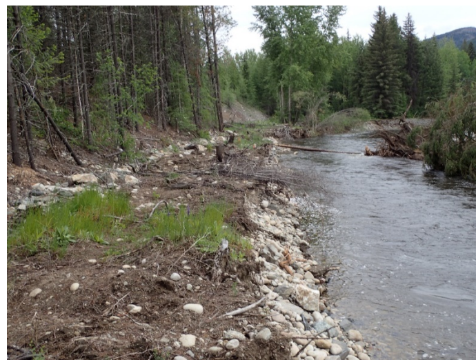
Photograph 12: South TSF, Cell 5, buried riprap at toe of TSF downstream slope, looking northeast. 14 June 2018.
