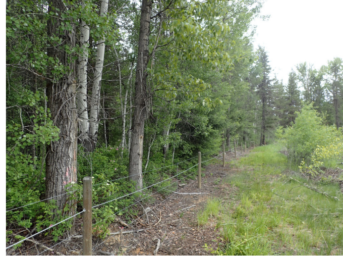
Photograph 30: South TSF, Cell 3, mature trees on dam crest, looking southeast. 14 June 2018.
