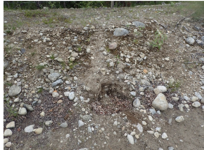
Photograph 36: North TSF, Cell 6, minor erosion in north embankment, looking northeast. 14 June 2018.
