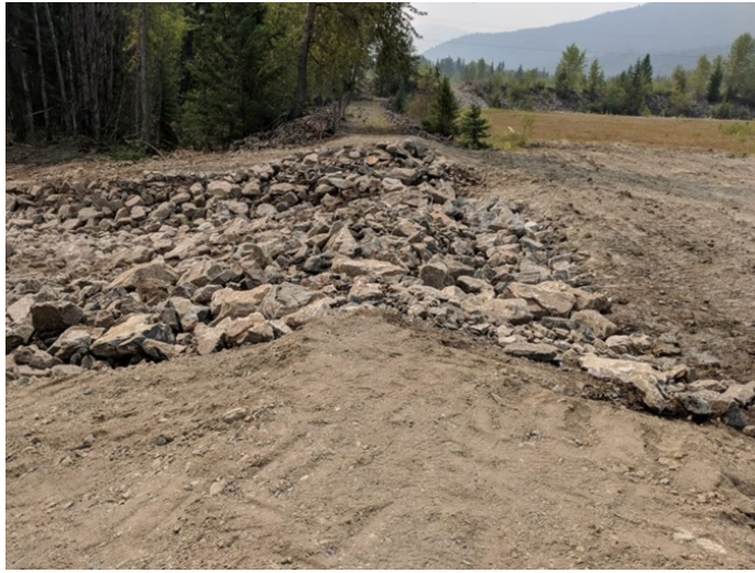
Photograph 25: South TSF, Cell 3, As-Built Spillway Crest., looking south 16 August 2018.
