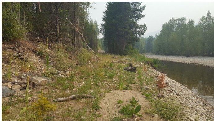
Photograph 11: South TSF, Cell 5, buried riprap at toe of TSF downstream slope, looking northeast. Low river flow. 8 August 2017.
