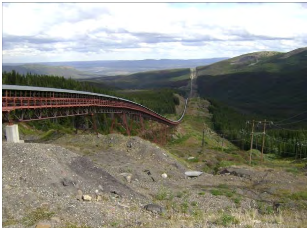
The existing overland conveyor at Quintette
