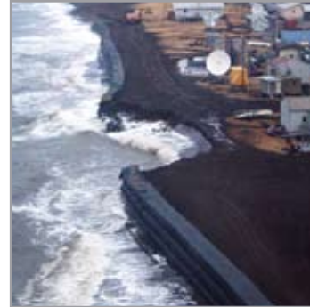
Emergency erosion control effort in the Village of Kivalina.
