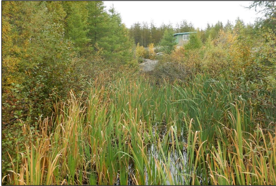
Photo 13 : Dam 4B – Vegetative growth in the final effluent channel to be monitored.
