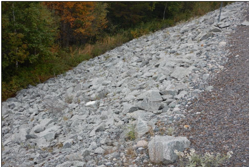
Photo 8 : Dam 1A – General view of vegetative growth at the toe of the embankment.
