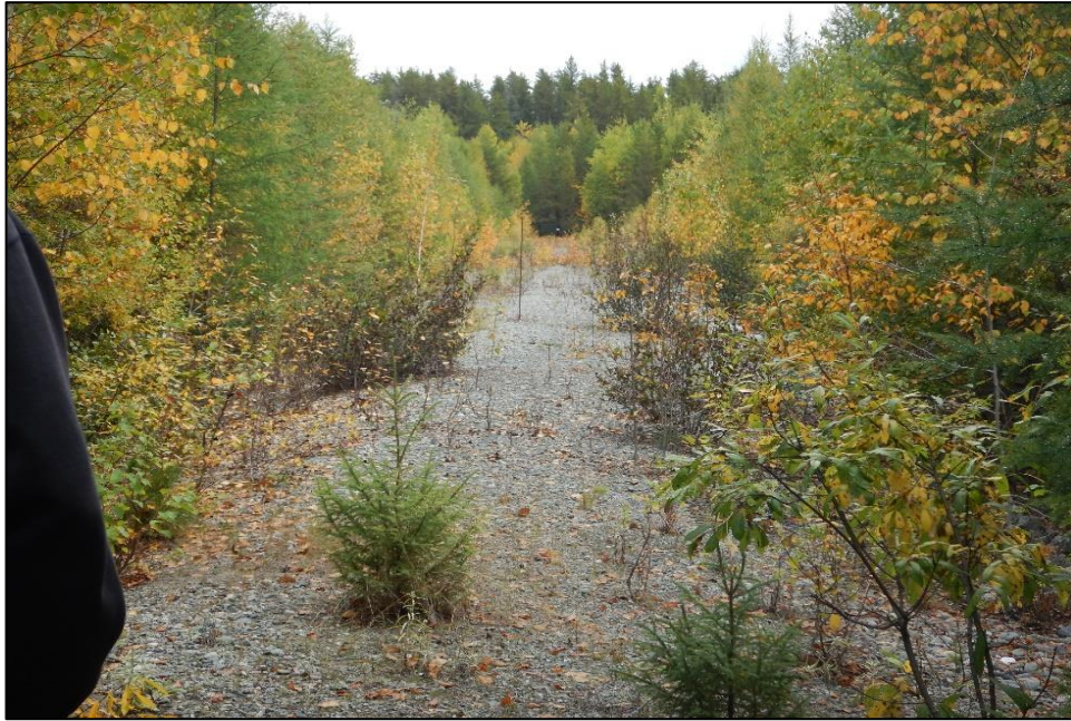
Photo 11 : Dam 4A - Crest of dam, looking East. Note significant vegetative growth on the sideslopes of the dam.
