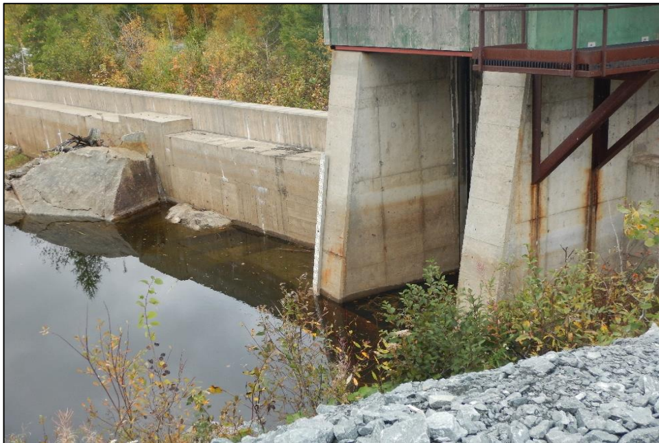
Photo 12 : Dam 4B – View of main spillway control structure and concrete overflow section adjacent to it. Concrete appears intact.
