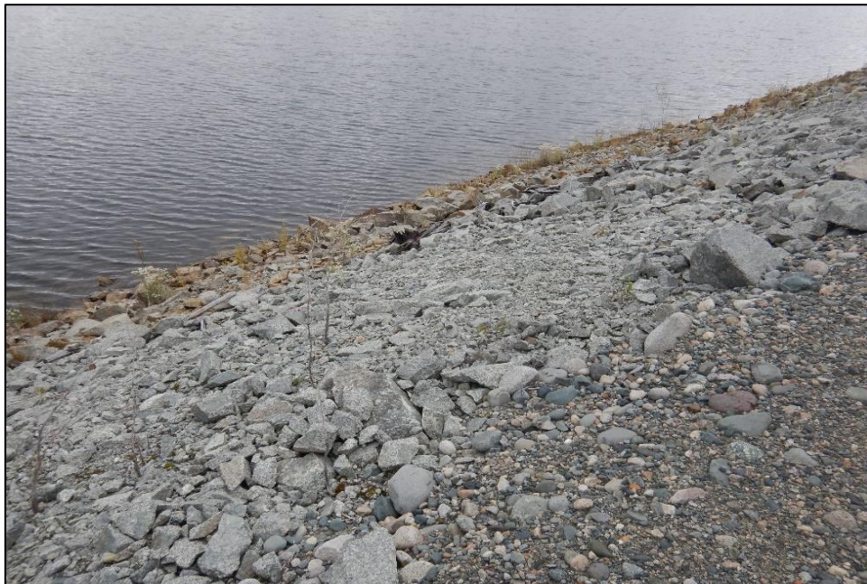
Photo 2 : Dam 1C – Photo of degraded rip rap area on the upstream slope. View looking South.
