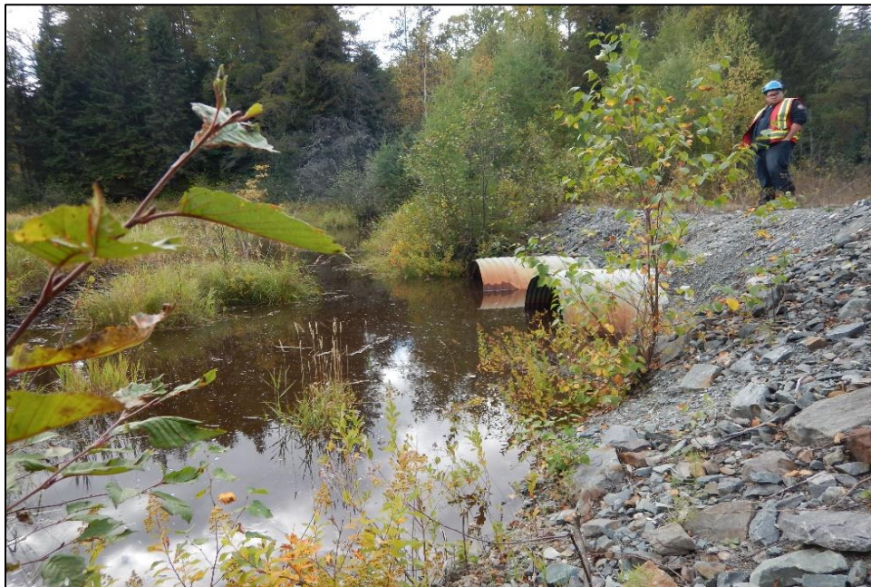
Photo 10 : Dam 2B - Photo of culverts located northwest of the TSF. The culverts are partially blocked by beaver activity.
