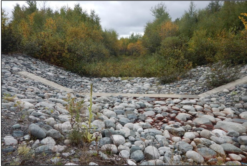
Photo 5 : Dam 1D – Photo of concrete sill and upstream spillway channel at the TSF emergency spillway. Vegetation was cleared in 2018.
