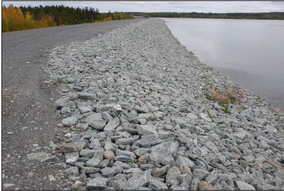
Photo 1 : Dam 1B - Photo of new rip rap placed on upstream slope. View looking East.
