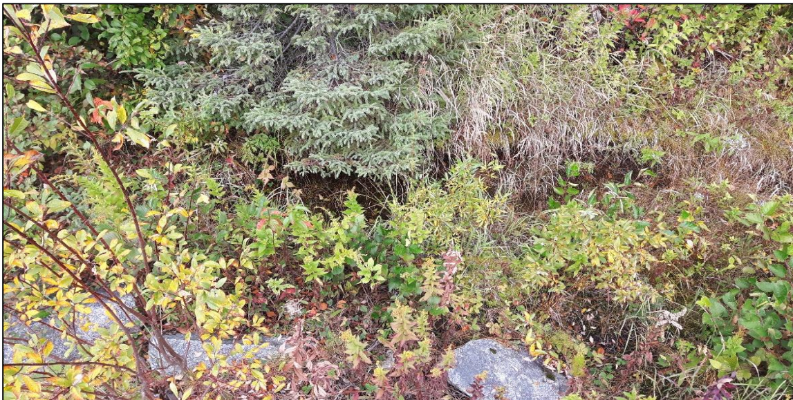
Photo 4 : Dam 1B – Photo of seepage area at the toe of the embankment. No visible flow, area is slightly damp.
