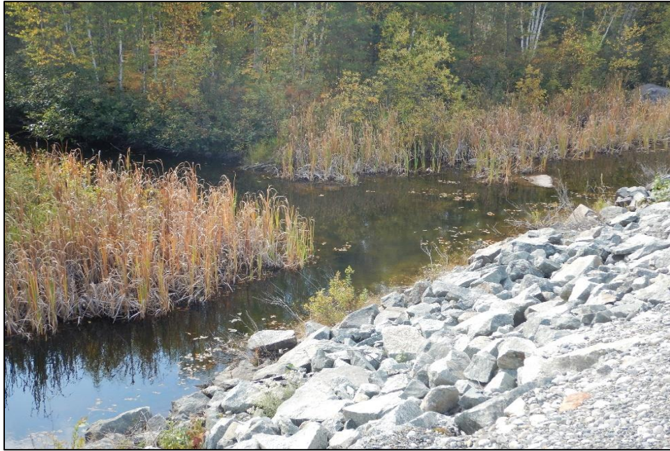
Photo 9 : Dam 2A – water ponding at the downstream toe of the dam, similar to previous years. This is a natural topographic low, however beaver activity nearby exacerbates the ponding.
