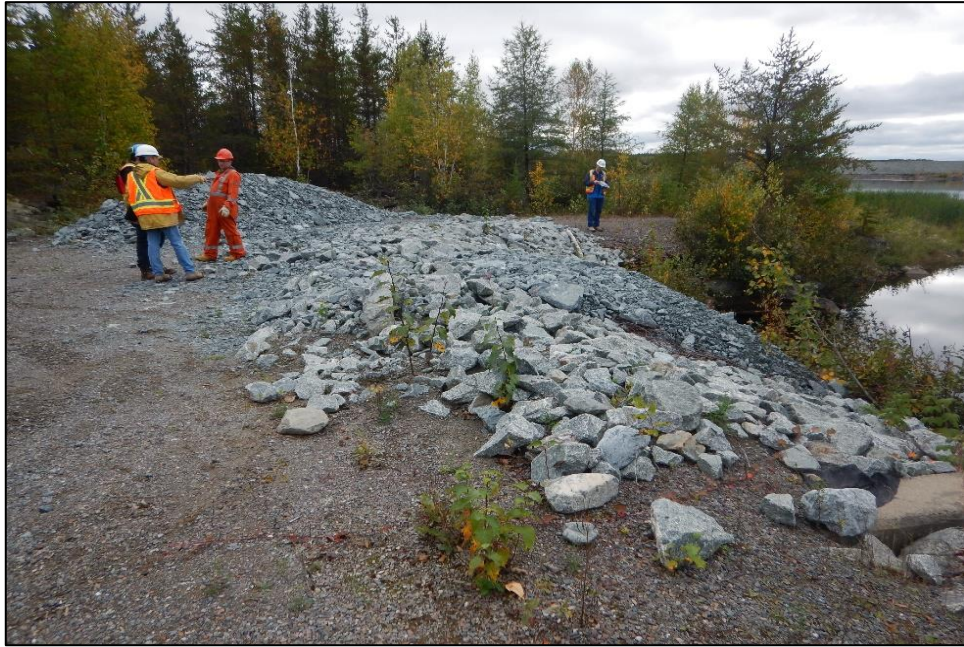
Photo 15 : Dam 4B – granular fill placed across part of the emergency spillway.
