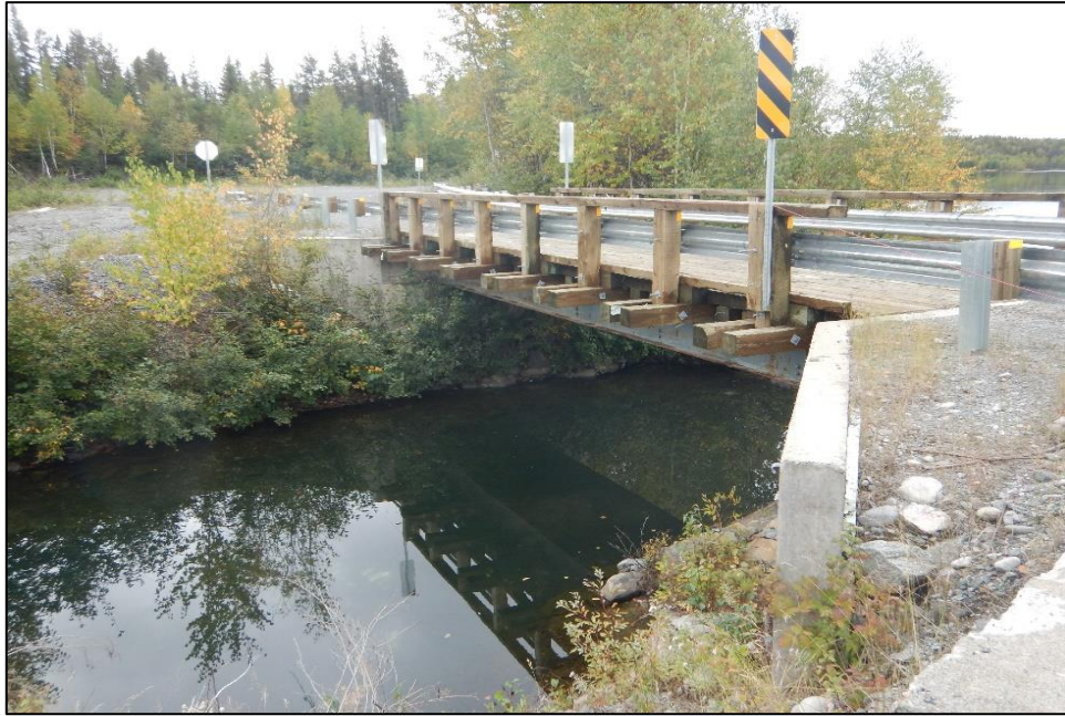
Photo 7 : Dam 1E – Spillway bridge in good condition.
