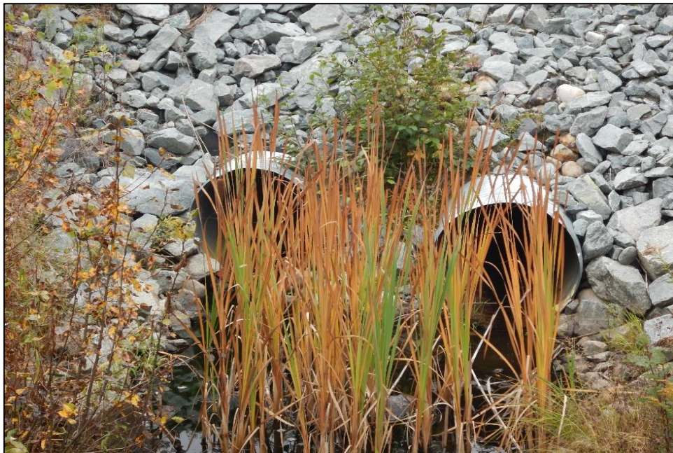
Photo 14 : Dam 4B – final outflow culverts are clear and unobstructed by sediment. Vegetative growth to be monitored.
