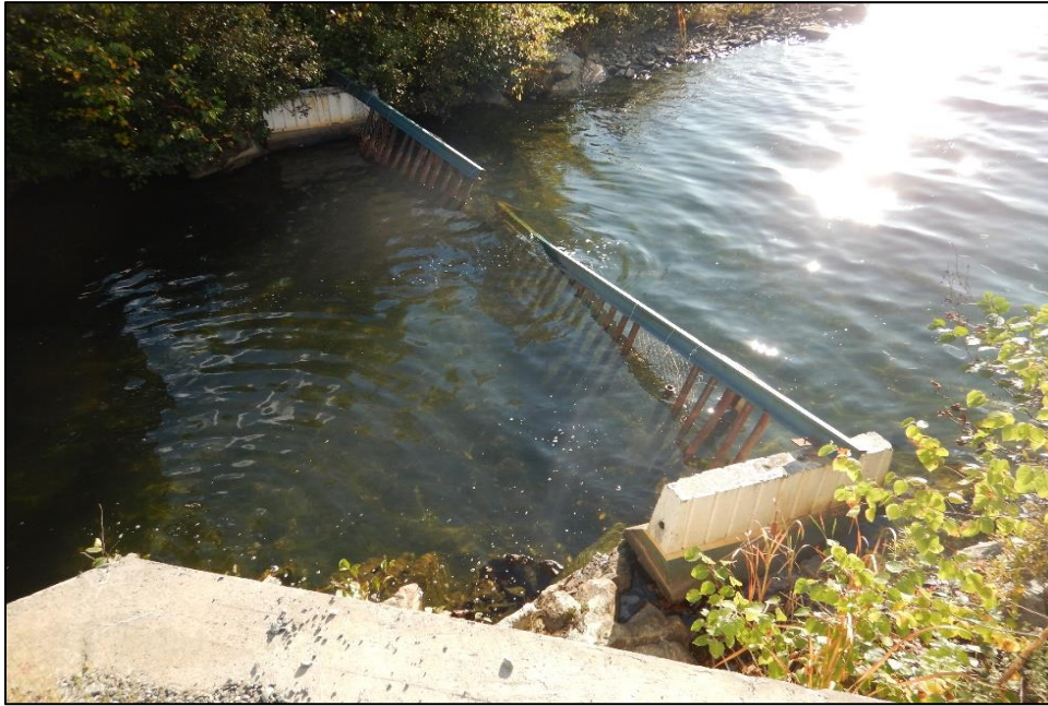
Photo 3 : Dam 1E – Photo of damaged trash rack structure.
