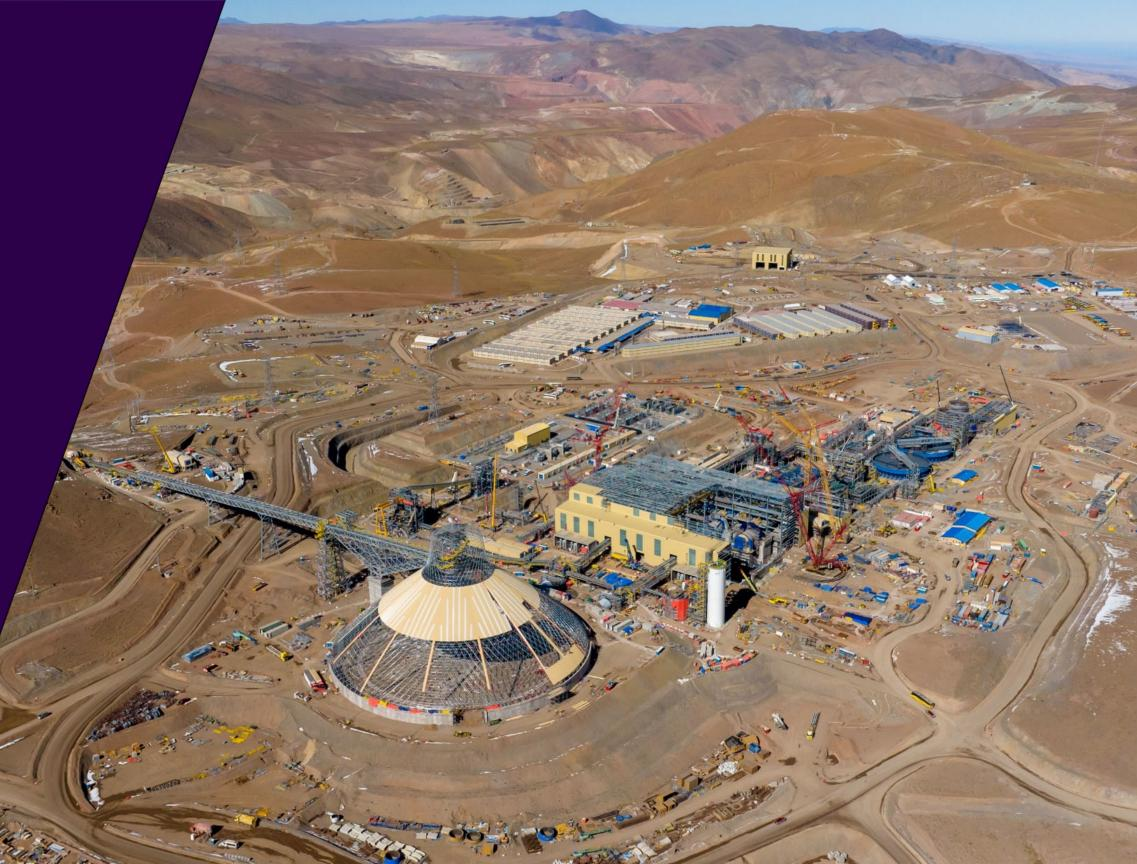
Grinding building and SAG feed conveyors
