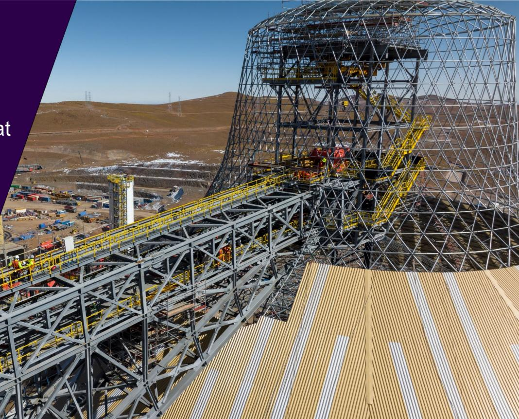
Concentrator area overview including stockpile dome, grinding building, and flotation area. Camp and truck shop in background.
