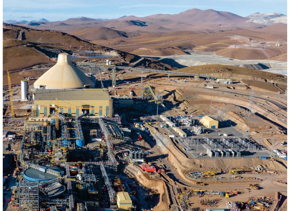
Concentrator flotation area, grinding building, and ore stockpile.
