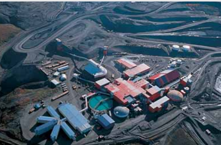
Aerial view of the Red Dog plant site.
