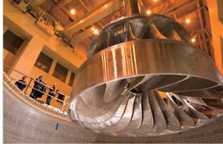
Lowering a new turbine into the generator at Waneta Dam.
