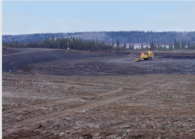
Mining to support pilot work at the Fort Hills oil sands project – Alberta.
