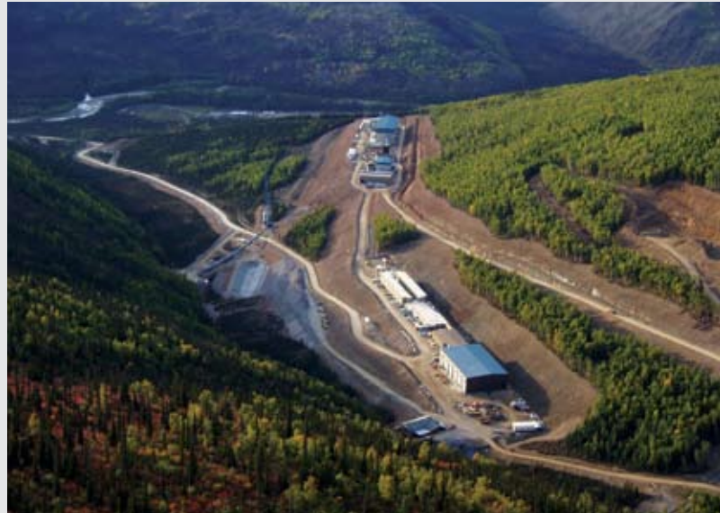
Surface facilities at Pogo gold mine – Alaska.
