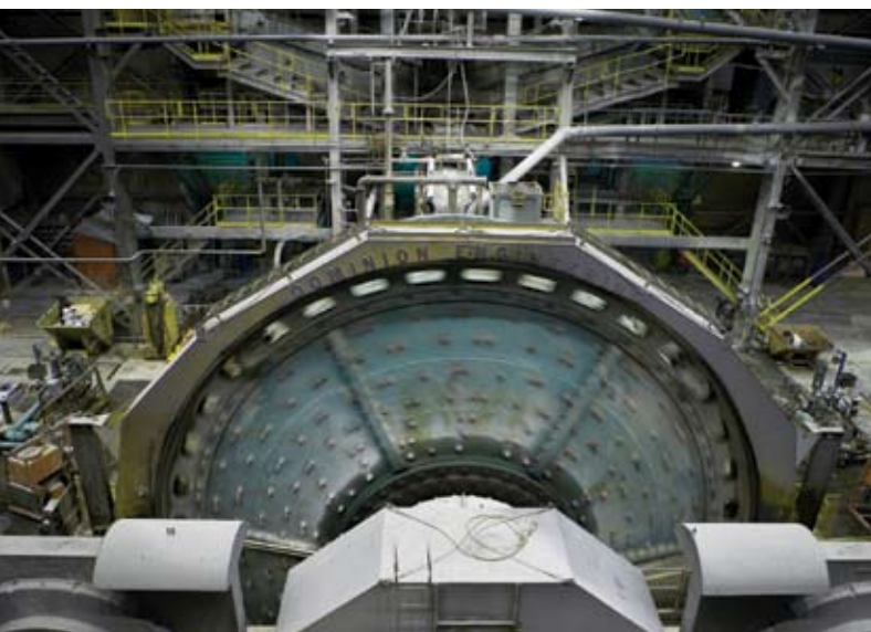
One of the five primary SAG mills – Highland Valley Copper, BC.
