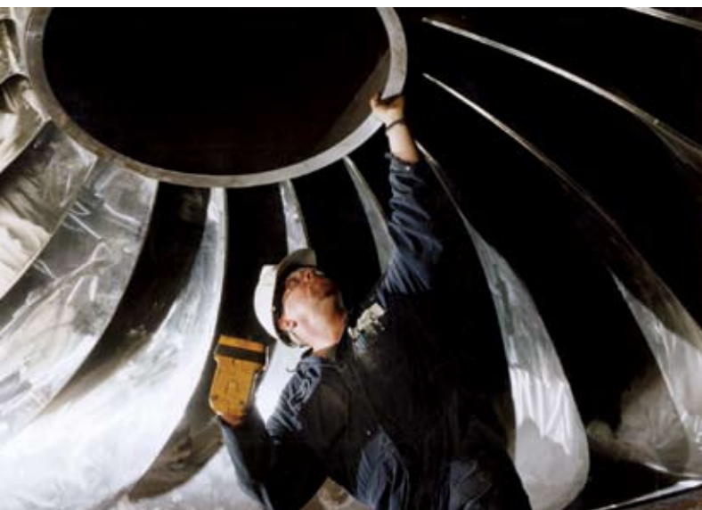
Walter Kutzner, a FortisBC Inc. Welder – Waneta Dam, BC.
