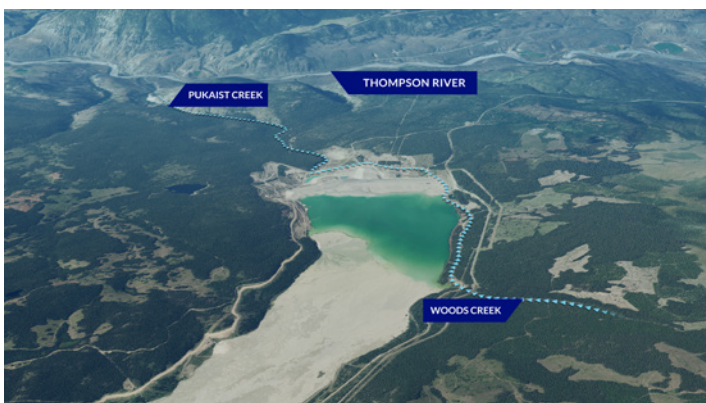
Historical flows from Woods Creek to Pukaist Creek have been re-established through the installation of the Woods Creek Diversion, enhancing groundwater control for downstream land users and ecosystems.
