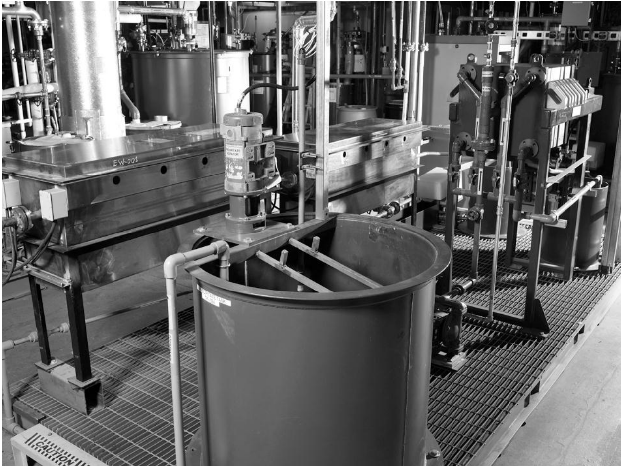
Figure 4 – CESL demo plant gold electrowinning
