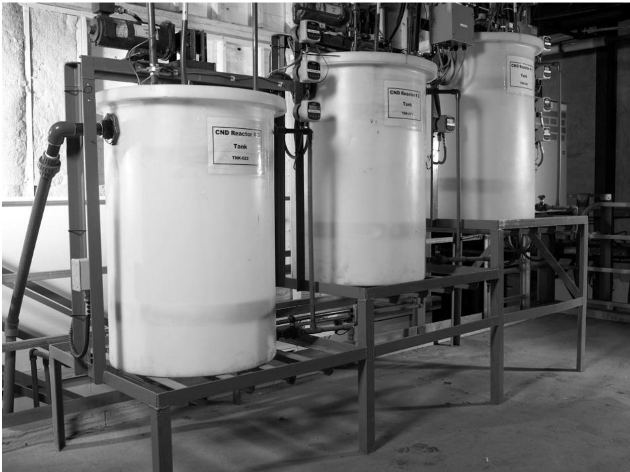
Figure 6 – CESL demo plant cyanide destruct reactors
