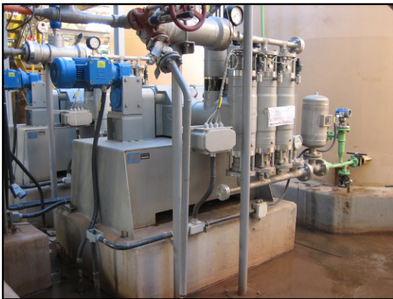
Figure 7. Autoclave slurry feed pumps.
