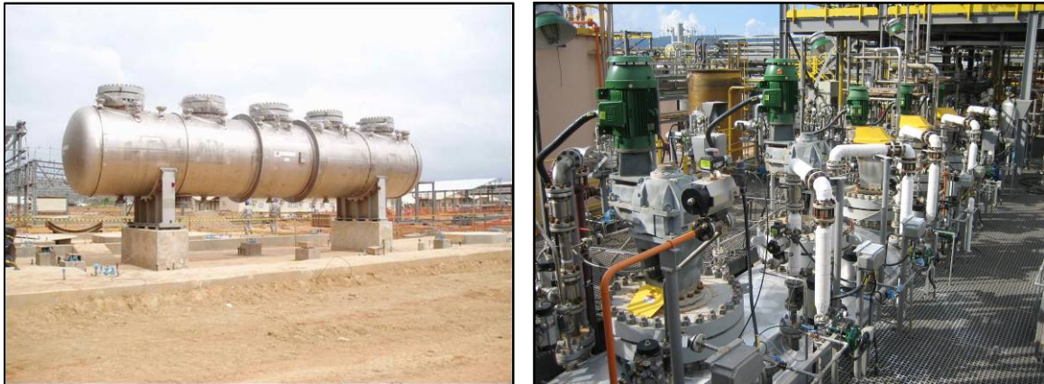
Figure 2. UHC autoclave (2.1 m ID, Grade 12 titanium).
