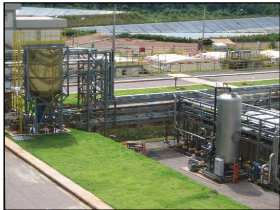
Figure 8. Electrolyte filter & back flush tank.
