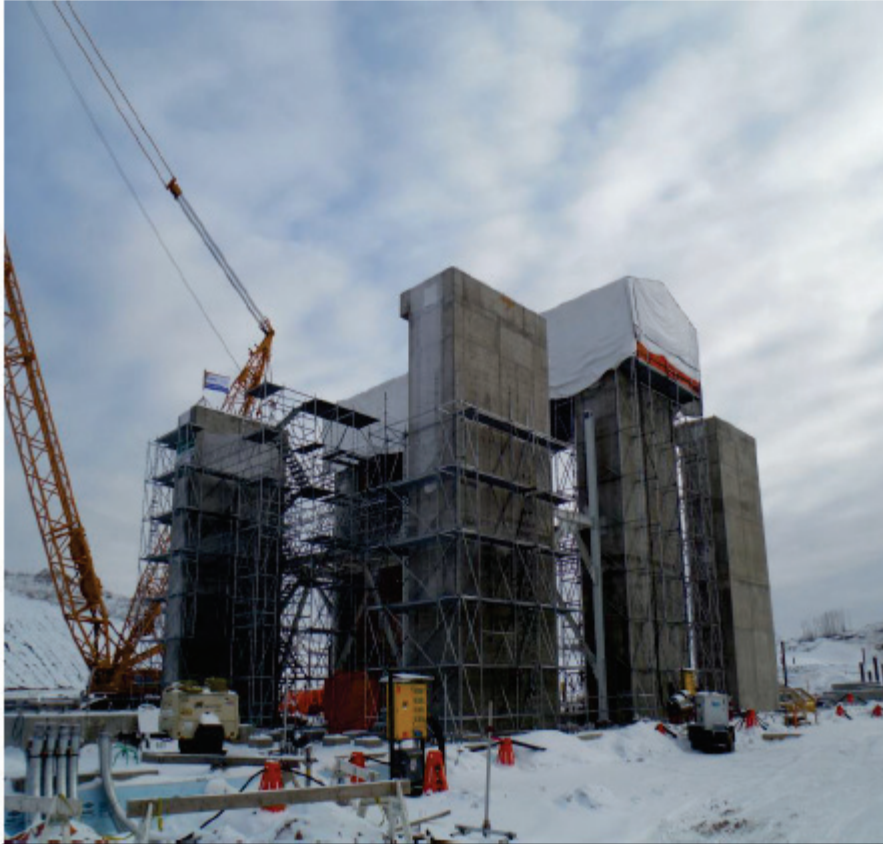
Ore Preparation Plant – trunnion installation
