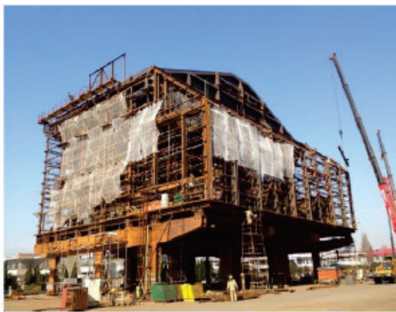
Surge Bin with Hopper pre-assembly in China.
