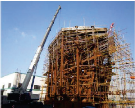
Crusher Plant Hopper & Support Structure for Train 1.
