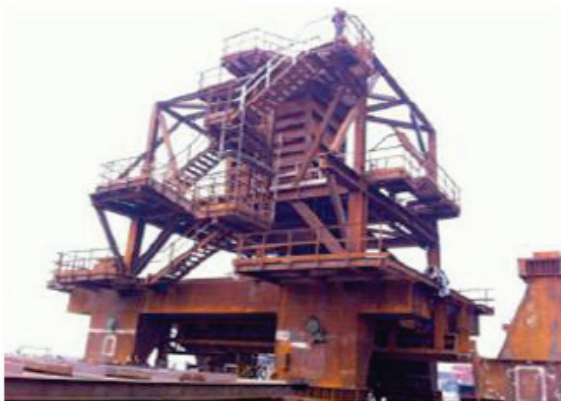
Crushing Plant Sizer module train 2 was being assembly
