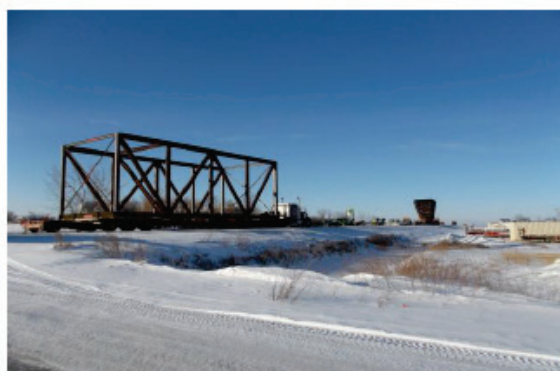
610D-2003 Lower Pumpbox and Cradle Mid-Section is on the road. 05-Feb-15
