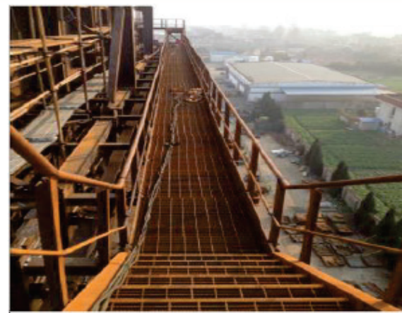
Stairs & Platforms have been shipped from other China shops for full pre-assembly on Surge Bin.
