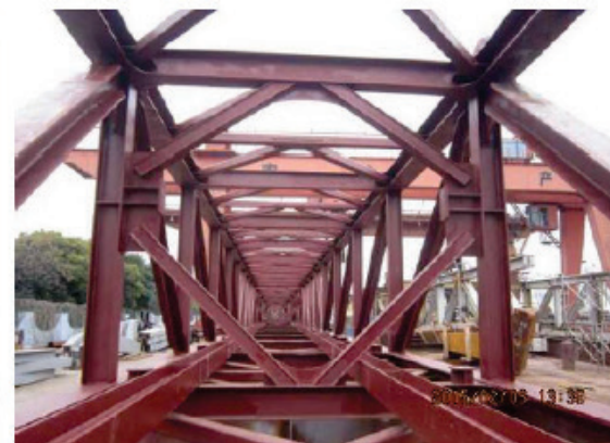
Conveyor Bridges being assembled by SBC
