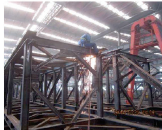
Conveyor bridges progressing.
