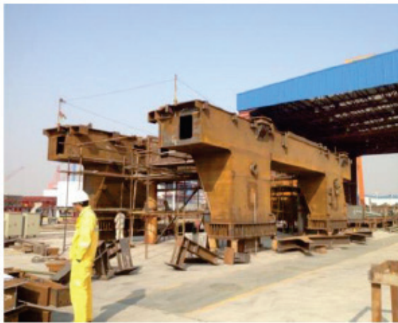
Sizer support structure pre-assembly.
