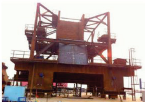
Crushing Plant Sizer module train 2 was being assembly
