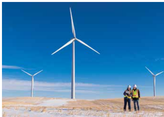
Our Wintering Hills Wind Power Facility near Drumheller, AB
