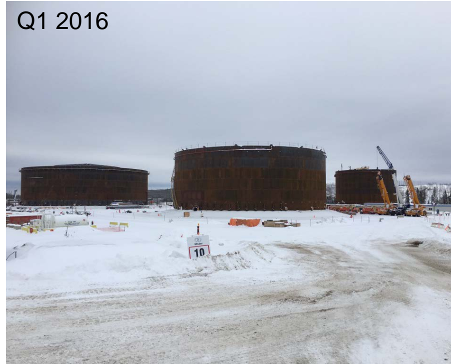
Pipeline start at the Fort Hills tank farm
