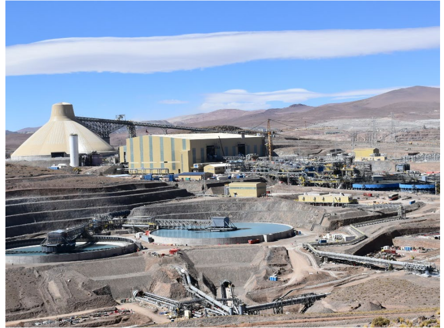
QB Operations site overview, October 2023.
