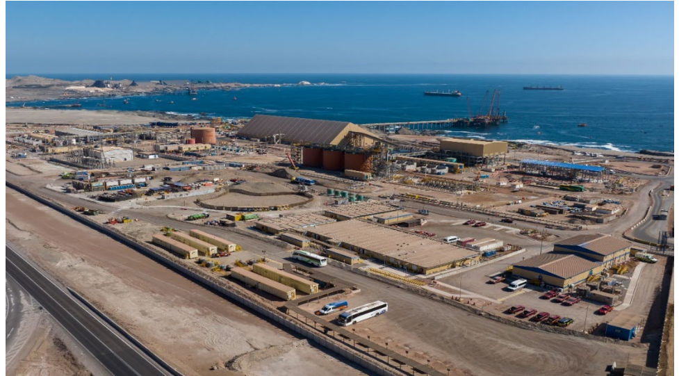
QB desalination plant.
