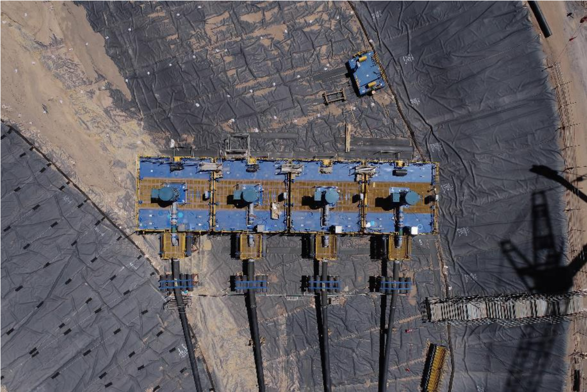
Pump barge setups
