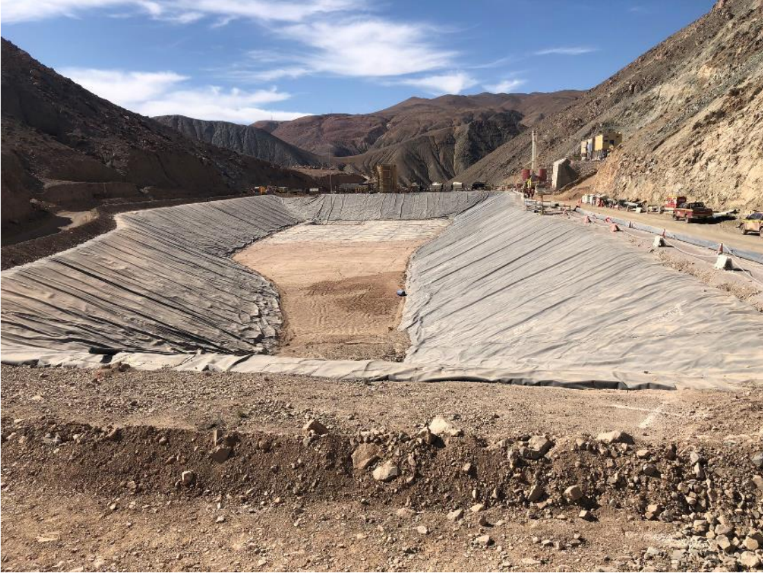
Seepage Collection Pond 1
