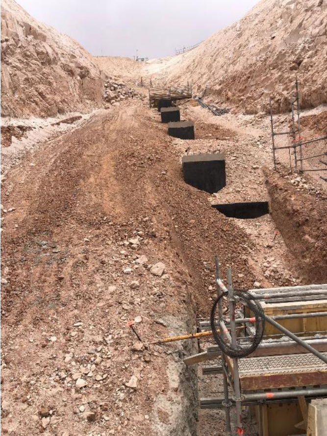
East abutment above starter dam crest
