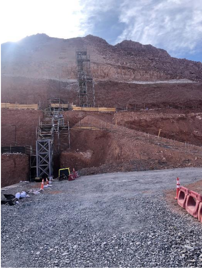
East abutment viewed from starter dam crest
