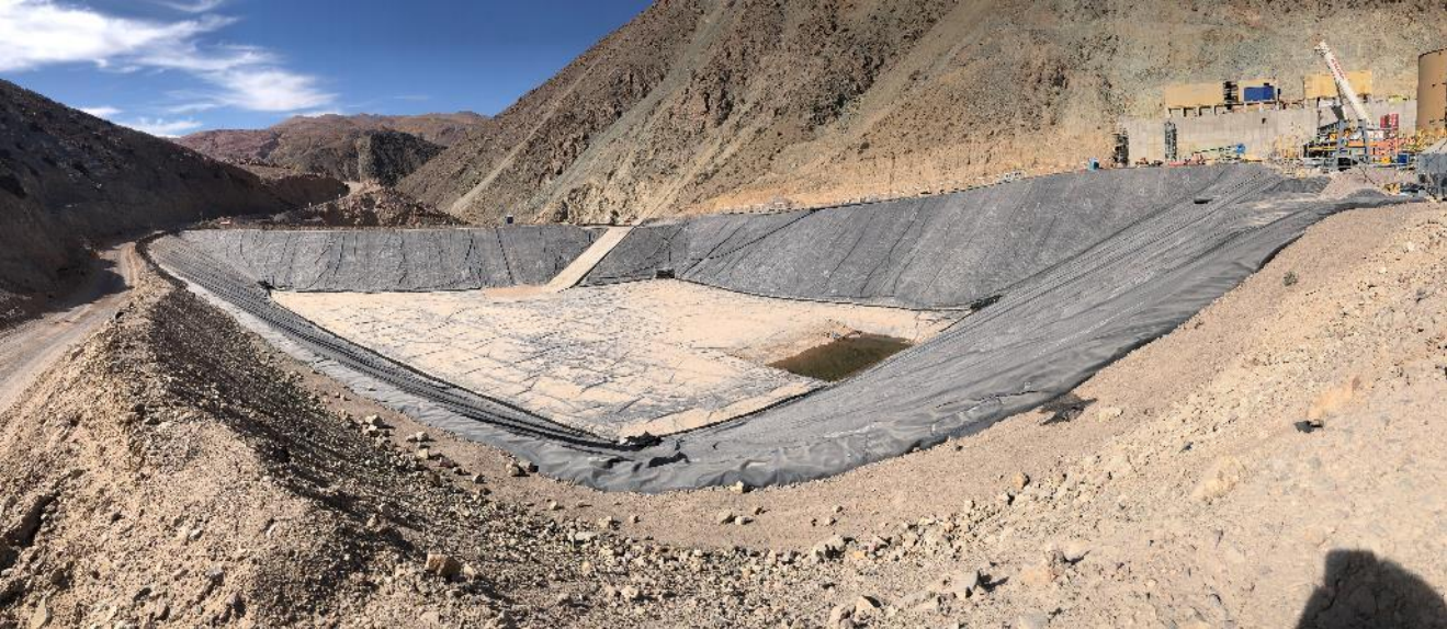
Seepage Collection Pond 2
