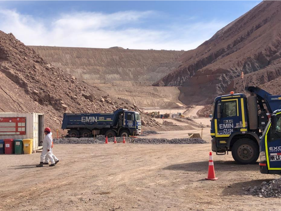
Looking upstream towards starter dam along dam drain
