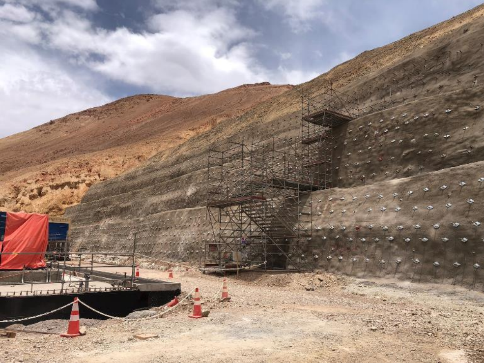
Slope reinforcement measures
