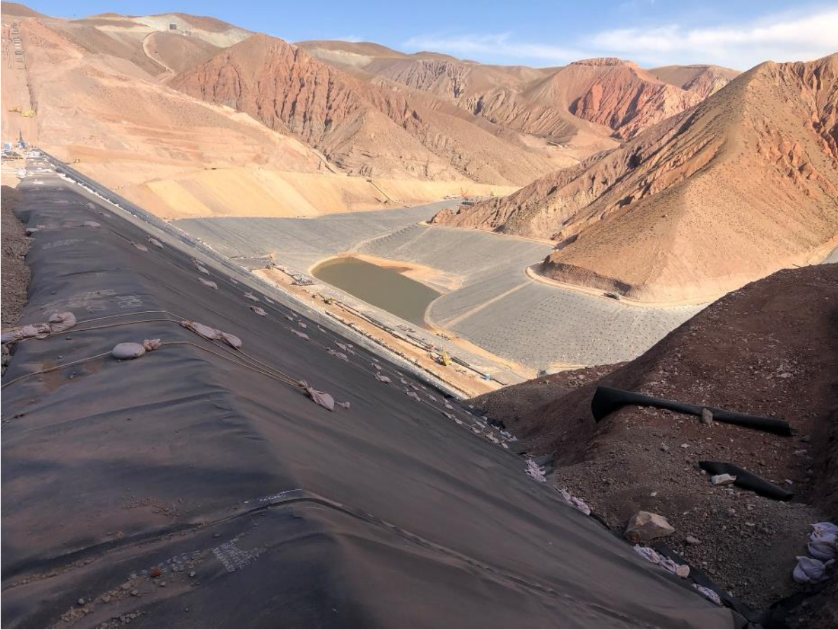
View from west abutment of starter dam crest
