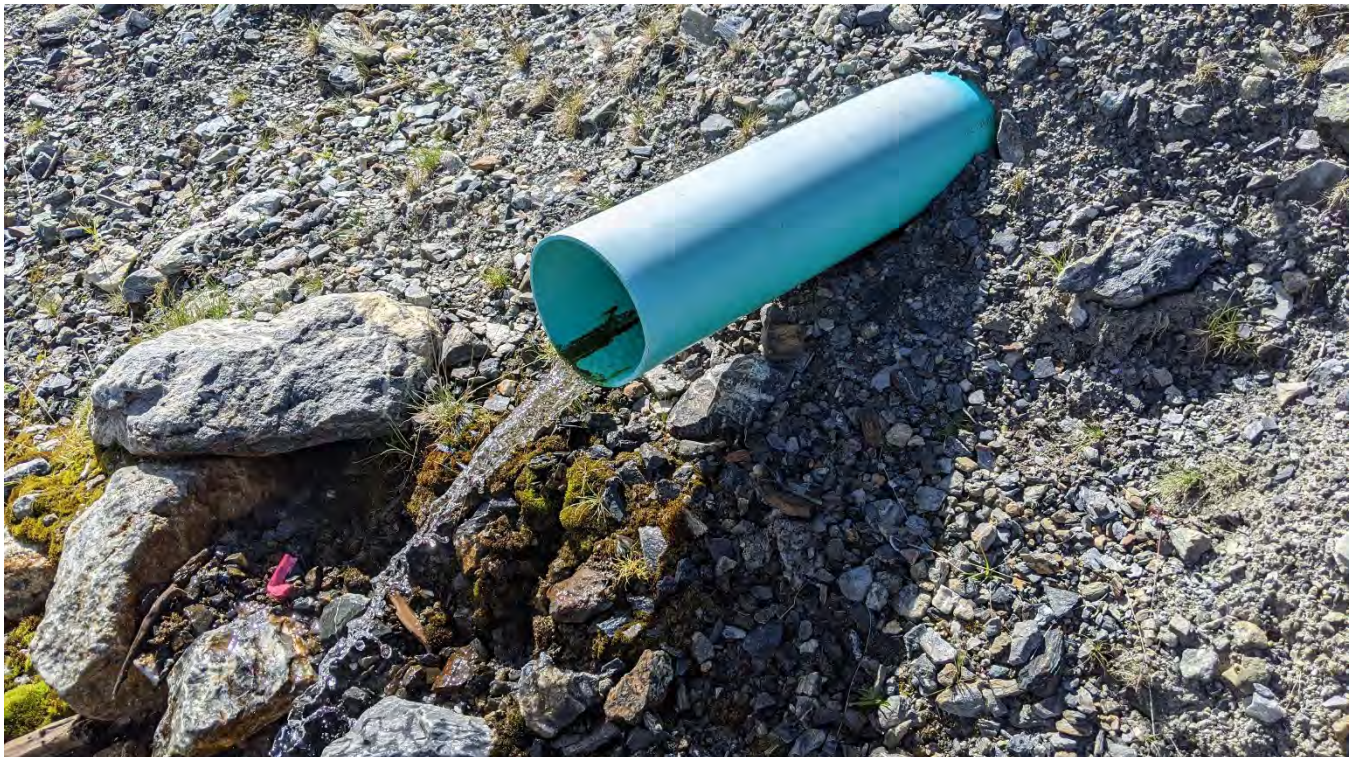
Photo WR-18: 1200 Portal drainpipe.
