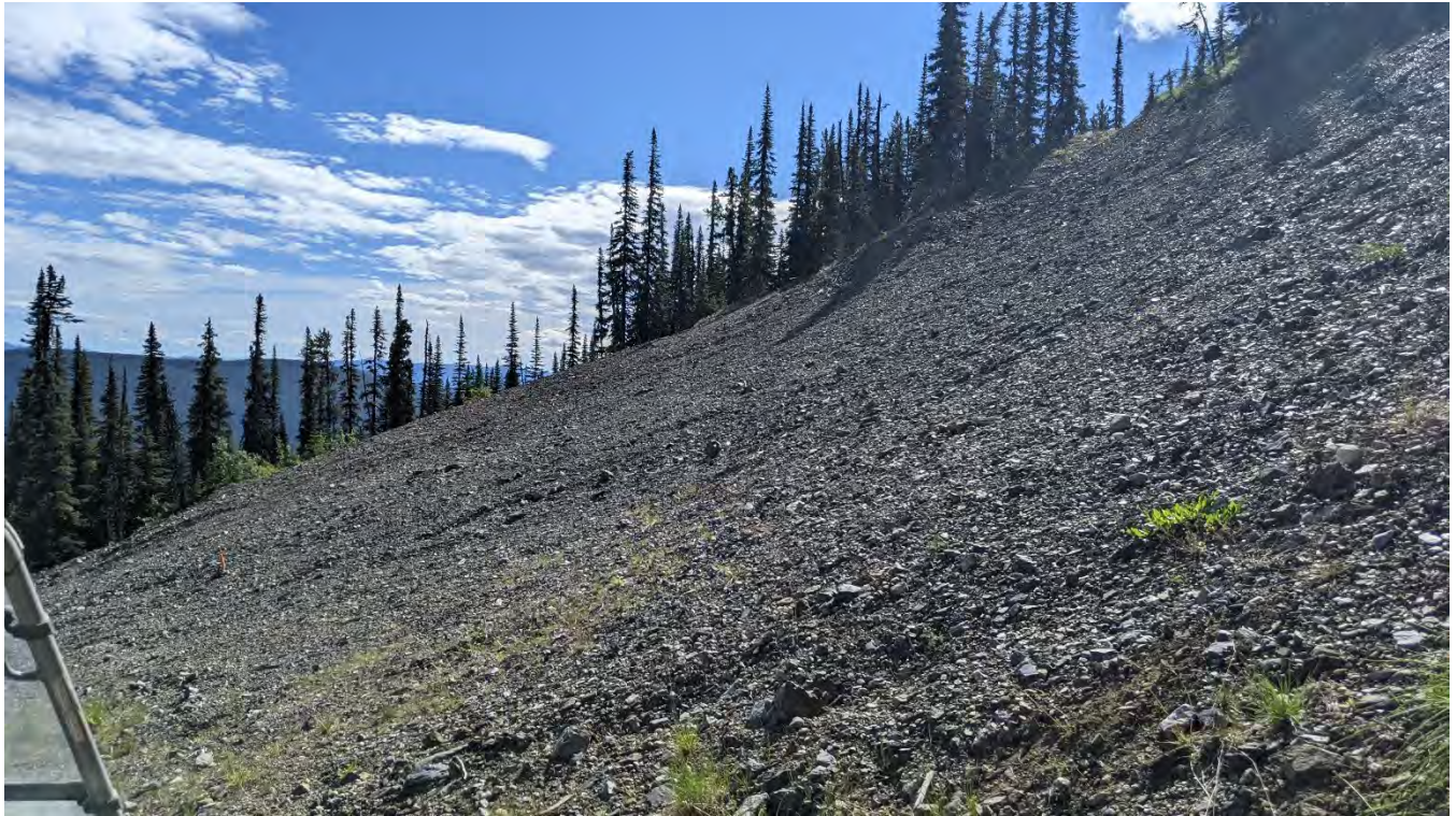
Photo WR-19: Regraded 1300 Portal Waste Rock Dump and 1300 Portal area
