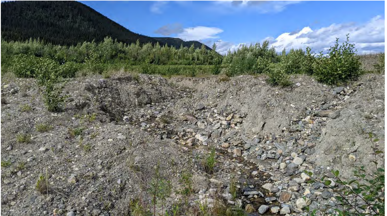
Photo TC-07: Upstream end of the erosion gully in the tailings cover south of the SRS Pond.
