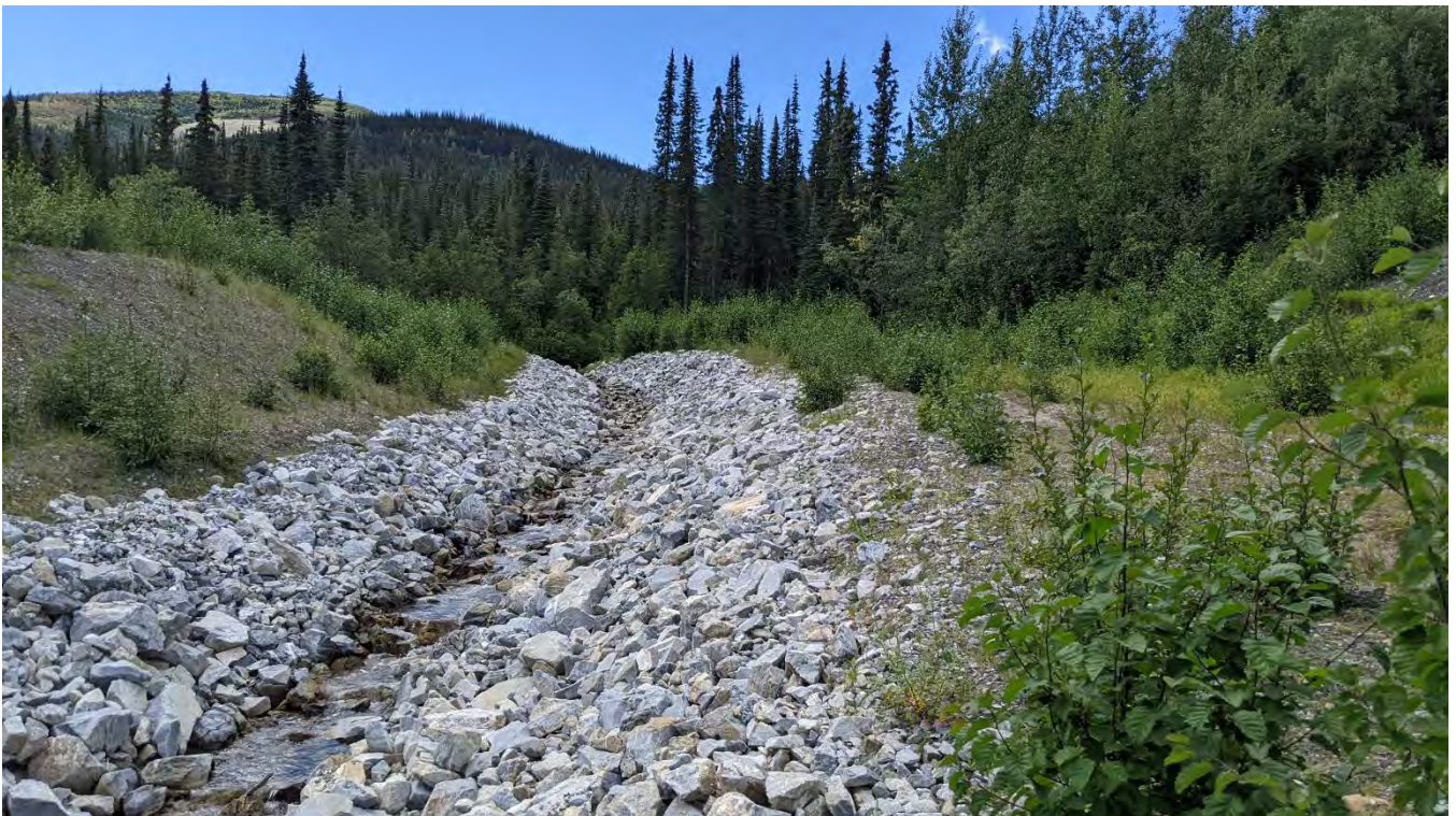
Photo DC-02: Camp Creek looking upstream.
