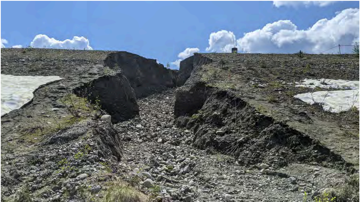
Photo 2: Erosion Gully looking upslope (June 21, 2022).
