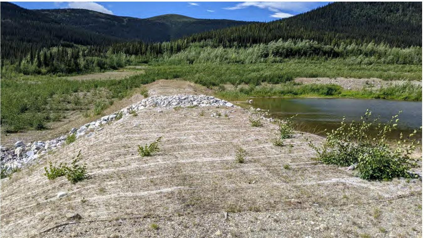
Photo SRS-04: SRS crest looking west from the east abutment.
