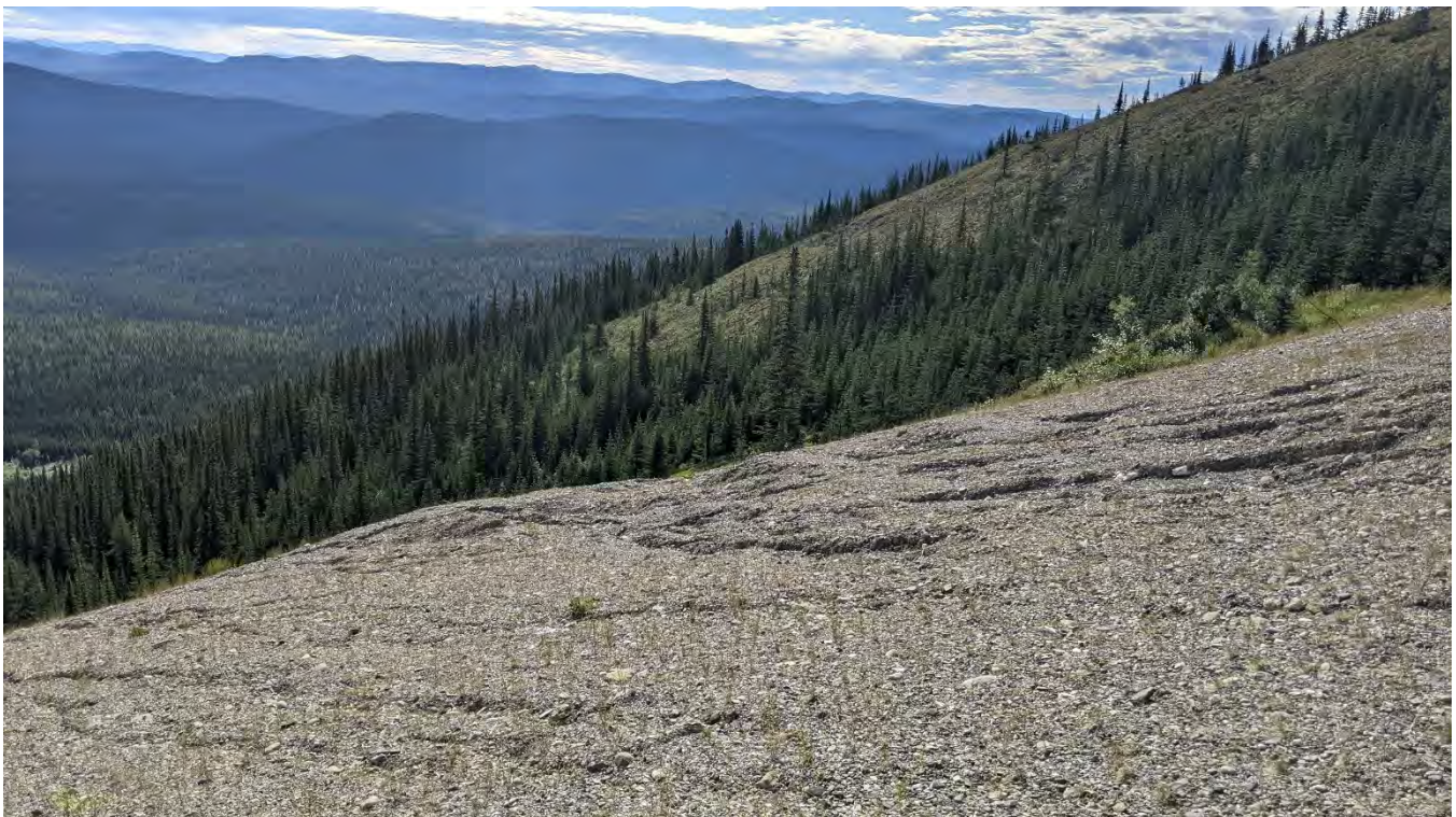
Photo WR-08: Surficial slumping near the south end of the 1408 Portal Waste Rock Dump
