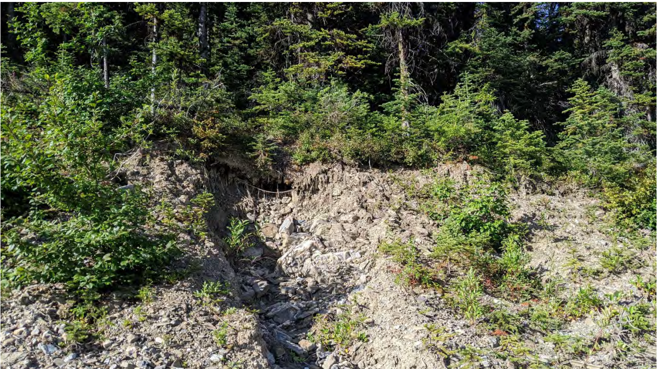
Photo WR-02: Erosion gully across the decommissioned access road to the Jewelbox Waste Rock Dump.
