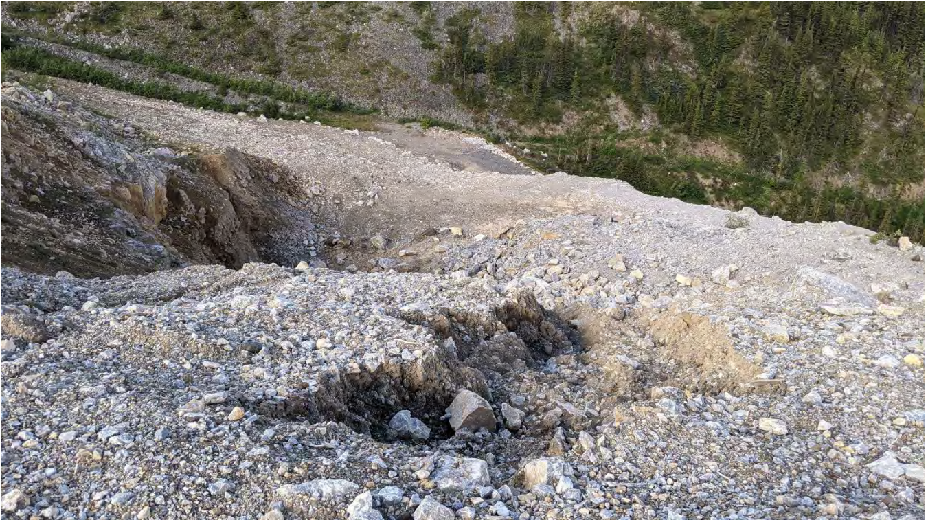
Photo WR-15: Erosion gully down the Main Zone Waste Rock Dump above the 1380 Portal.
