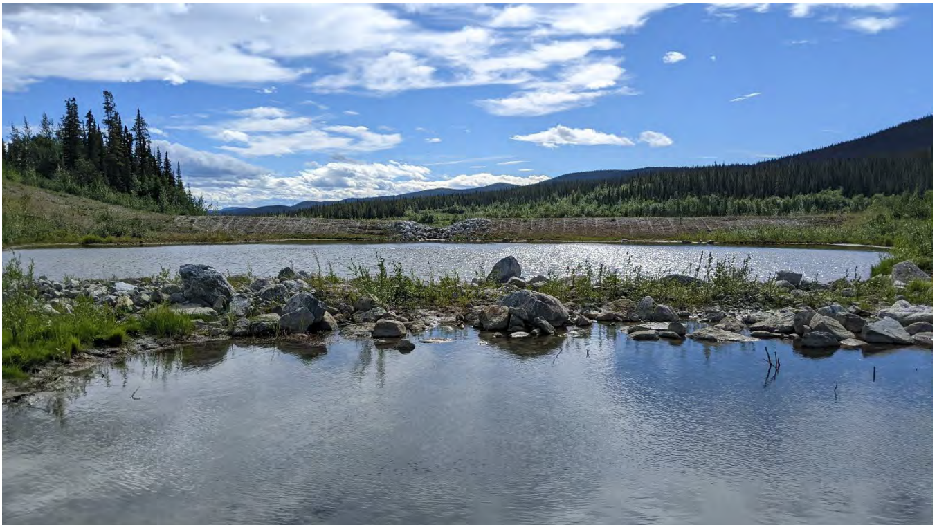
Photo SRS-02: SRS in distance, with the coffer dam in the foreground of the photo.
