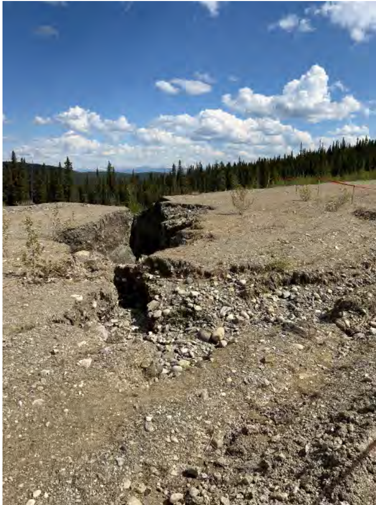
Photo 3: Erosion of the dam crest and tailings cover at the upstream end of the erosion gully (June 21, 2022).
