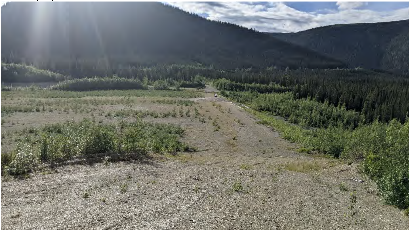
Photo ND-04: North Dam looking west.
