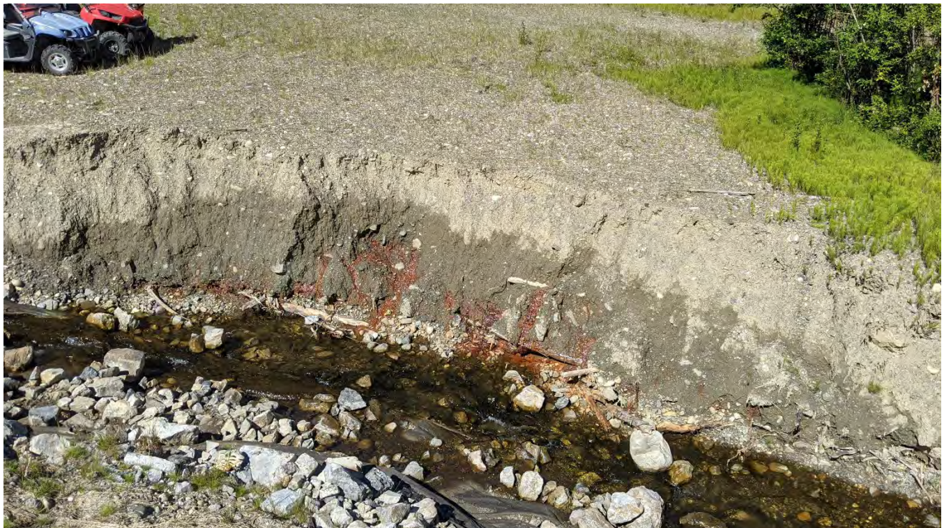
Photo NC-02: Channel Erosion at North Creek across the decommissioned access road to Burnick Zone. Seepage observed entering channel leaving a rusty-reddish coloured stain on the soils.
