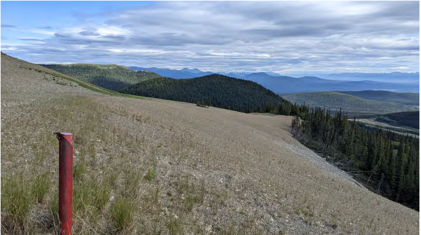
Photo WR-07: 1408 Portal Waste Rock Dump looking north.
