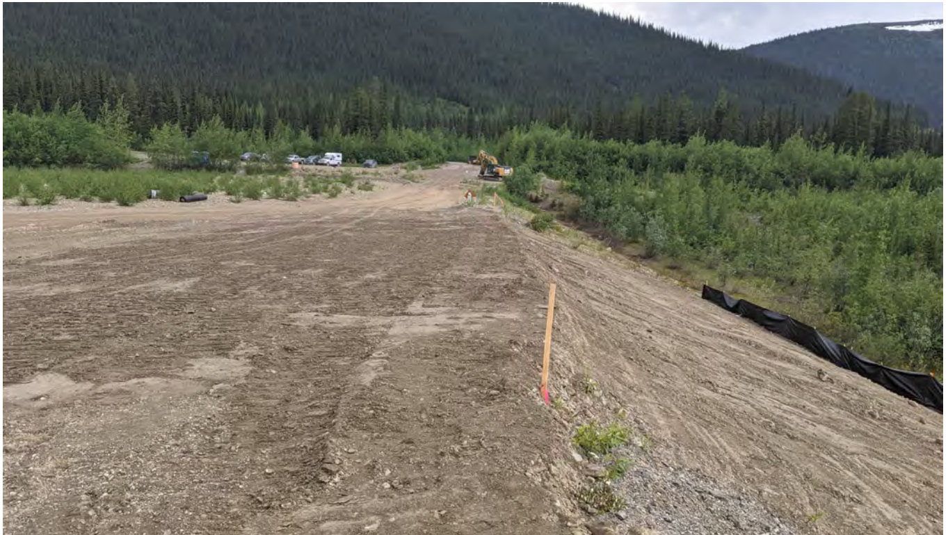
Photo 10: Completed repairs looking west (June 28, 2022).
