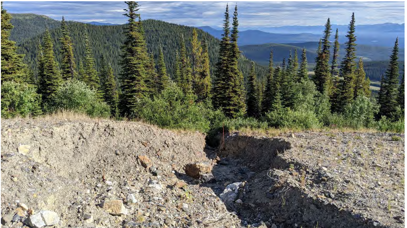
Photo WR-04: Erosion gully at the base of the Jewelbox Waste Rock Dump looking downslope. The gully has eroded down to bedrock.
