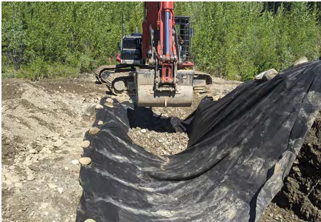
Photo 6: French Drain installation at the base of the gully (June 24, 2022).
