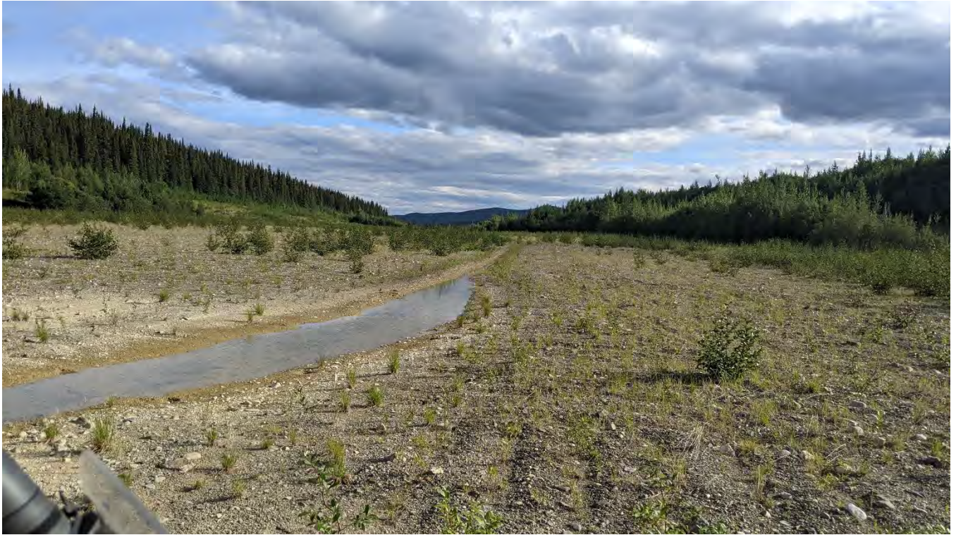
Photo TC-03: Main drainage swale that flows south through the middle of the tailings cover.
