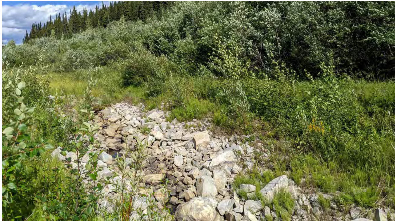
Photo DC-04: North Diversion Channel looking upstream.
