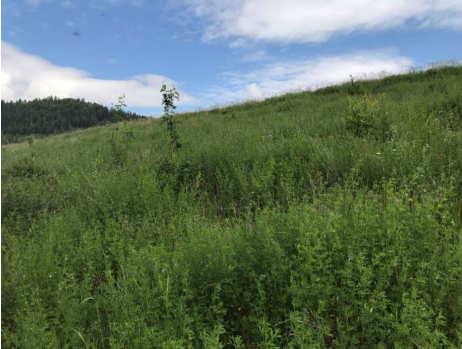
Photo II-15 TSF Embankment – Southwest leg, looking northwest along the downstream slope
