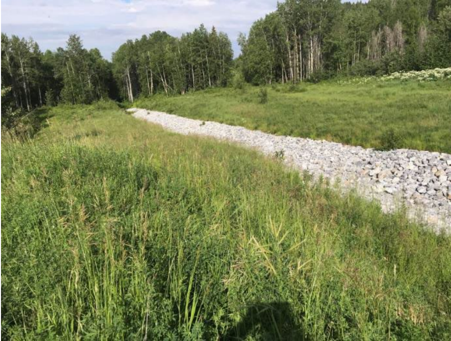
Photo II-21 Closure Spillway – looking downstream from embankment crest
