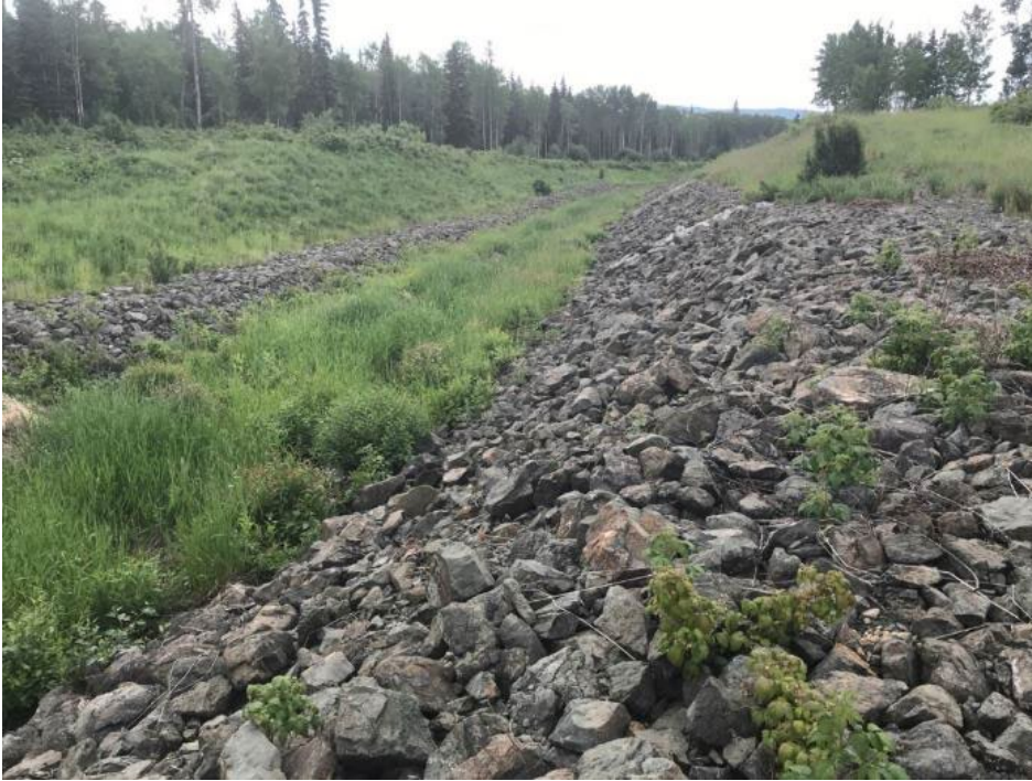
Photo II-39 Ed Creek Diversion Channel – Looking downstream from near first bend
