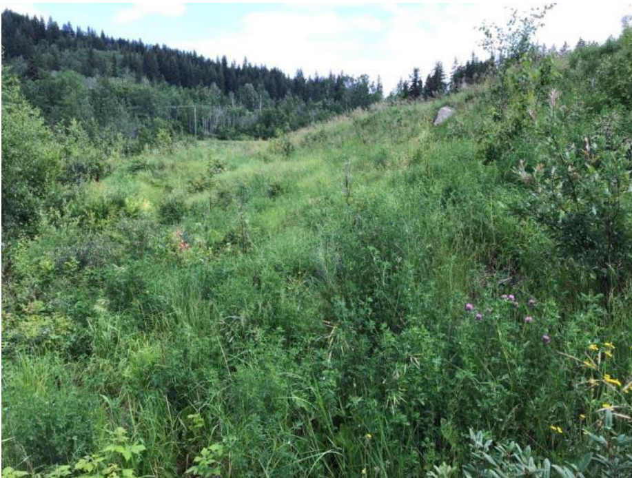
Photo II-16 TSF Embankment – West leg, looking north along downstream slope
