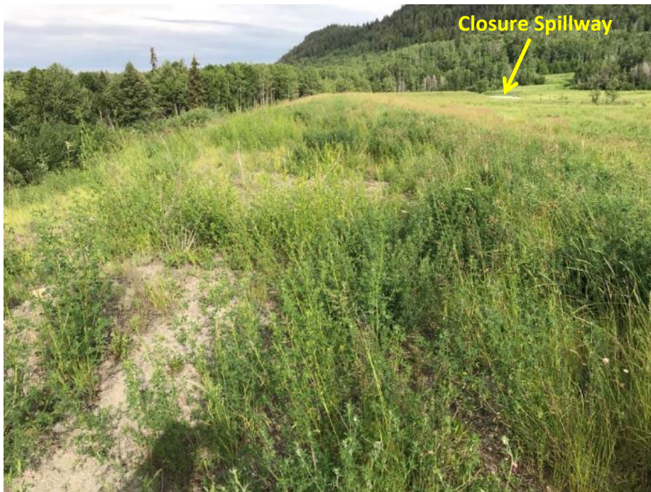
Photo II-12 TSF Embankment – Southwest leg, looking northwest along the crest
