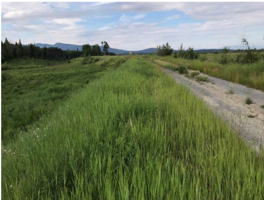
Photo II-6 TSF Embankment – East leg looking south
