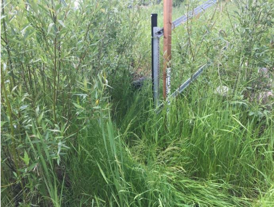
Photo II-25 Outlet Channel – Culvert inlet and flow monitoring station
