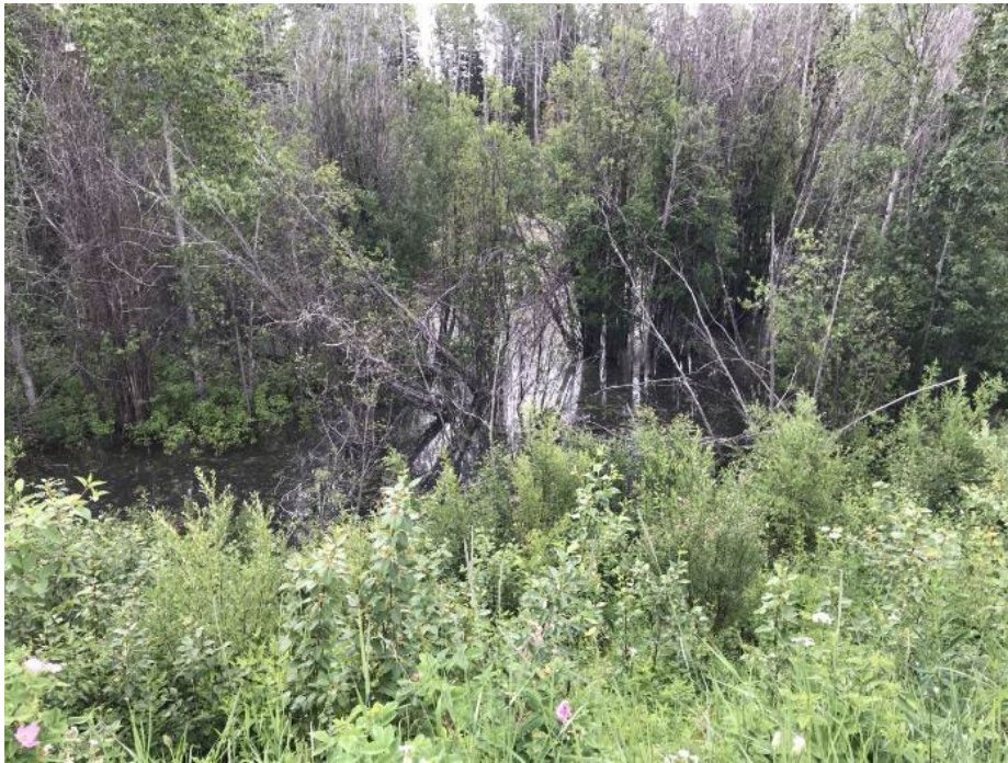
Photo II-5 TSF Embankment – Pond near toe of east leg
