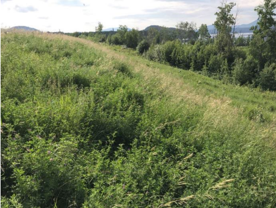
Photo II-13 TSF Embankment – Southwest leg, looking southeast along downstream slope
