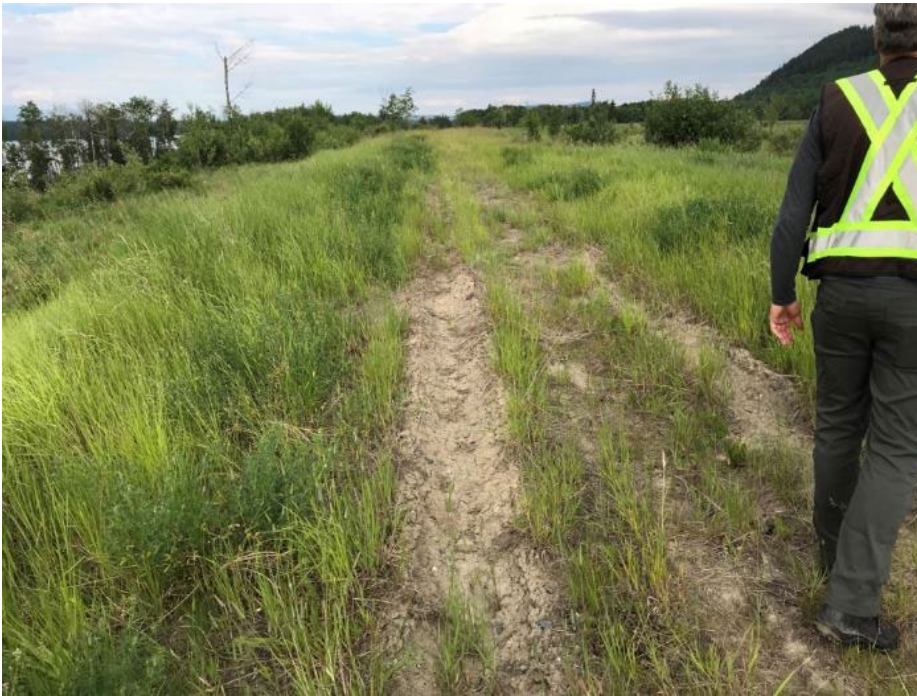
Photo II-11 TSF Embankment – South leg, looking west
