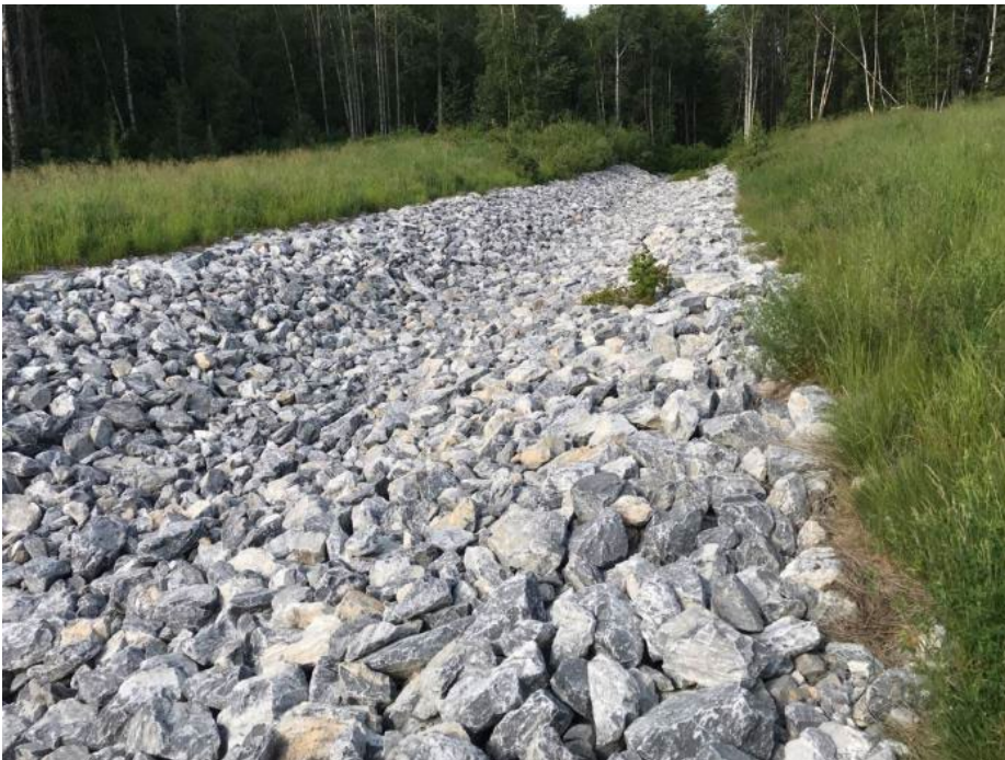
Photo II-22 Closure Spillway – looking downstream
