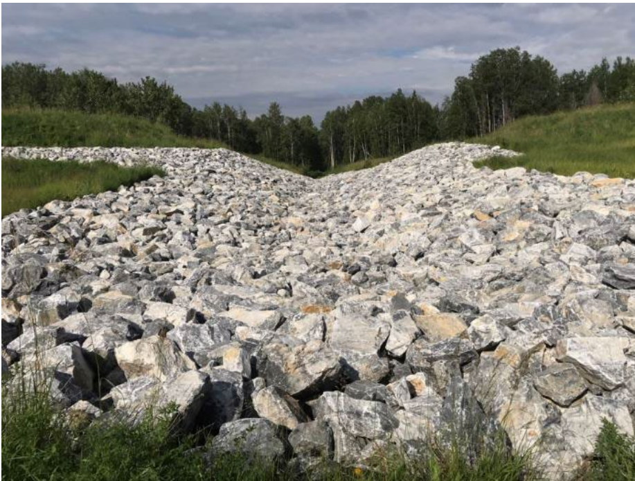
Photo II-20 Spillway inlet looking downstream
