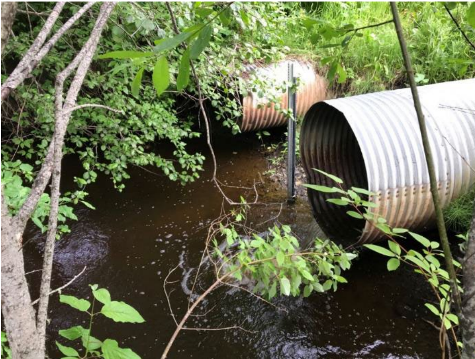
Photo II-48 Outlet of Ed Creek culverts under Pinchi Lake Road
