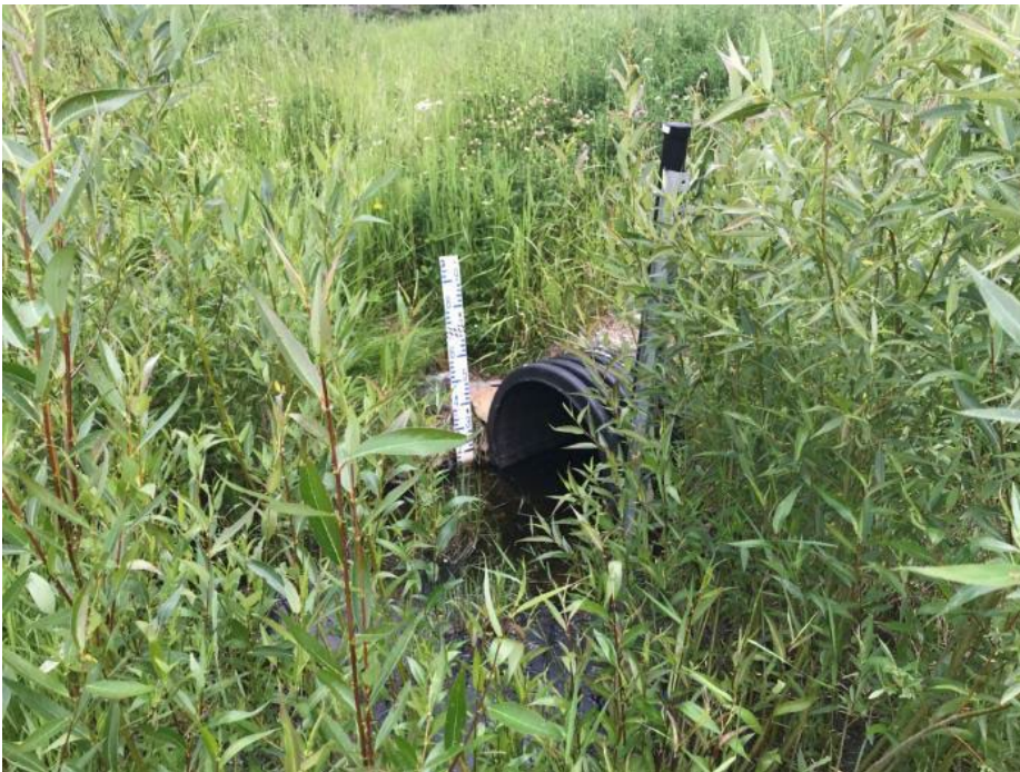
Photo II-26 Outlet Channel – Culvert outlet and flow monitoring station
