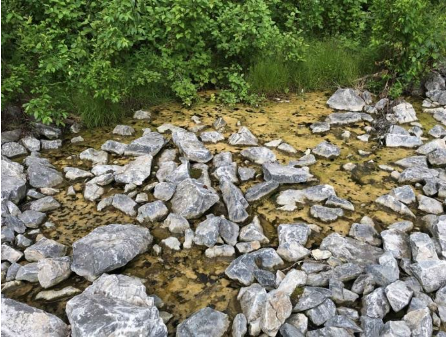
Photo II-23 Closure spillway – Pond at downstream end of riprap
