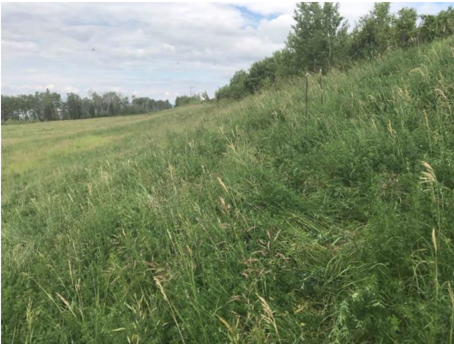
Photo II-28 Borrow Area A – crack monitoring rod location 203
