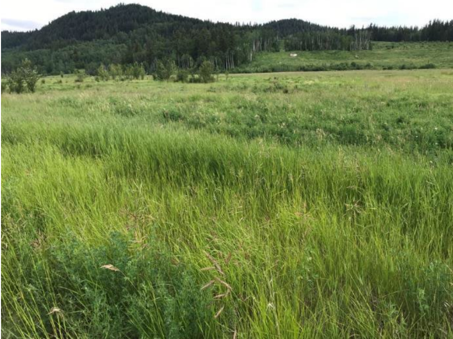
Photo II-10 TSF Embankment – South leg, looking north at the covered tailings surface
