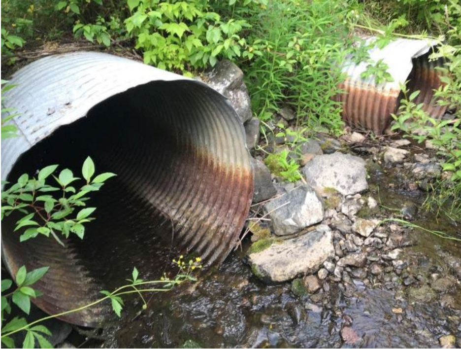
Photo II-45 Inlet of Ed Creek culverts under Pinchi Lake Road
