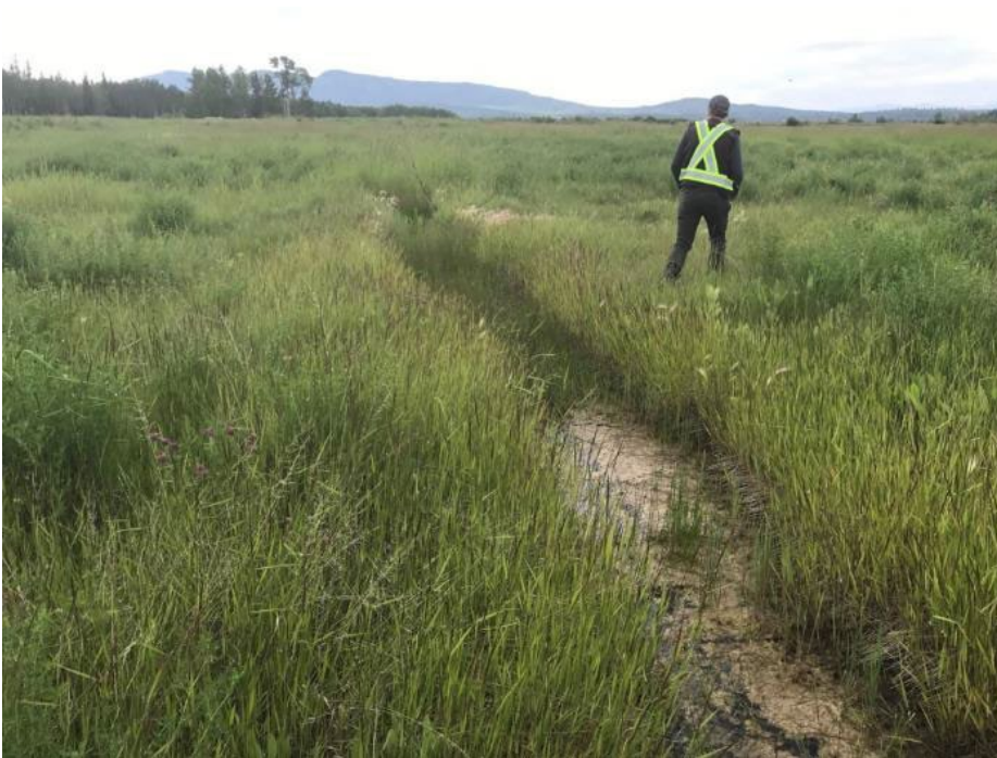
Photo II-3 Tailings Impoundment – Looking south along drainage channel in cover, ~70 m west of TSF Embankment East Leg. Note standing water
