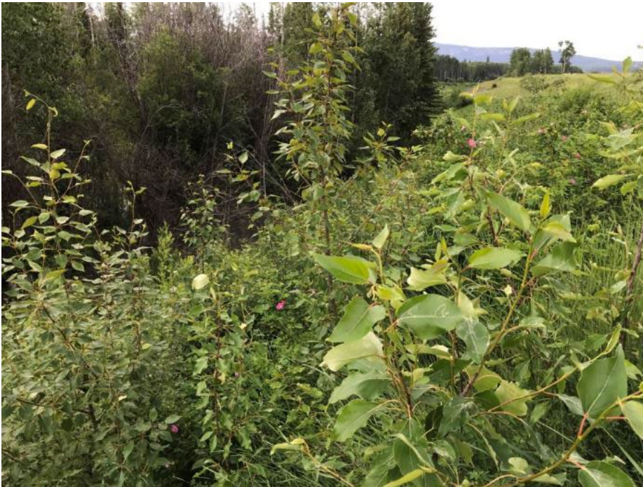
Photo II-4 TSF Embankment – East leg, looking south. Note vegetation
