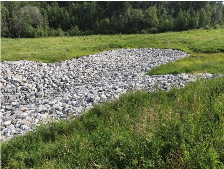
Photo II-18 Closure Spillway – Inlet apron
