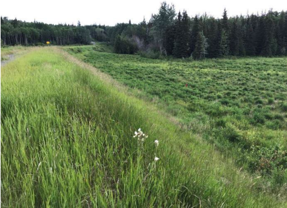
Photo II-7 TSF Embankment – East leg, looking north
