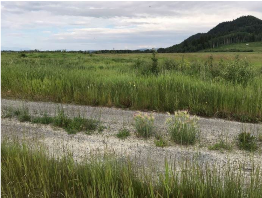
Photo II-8 TSF Embankment – East leg, looking west at the covered tailings surface
