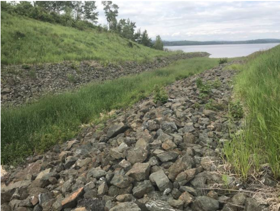
Photo II-32 Ed Creek Diversion Channel – looking downstream towards outlet
