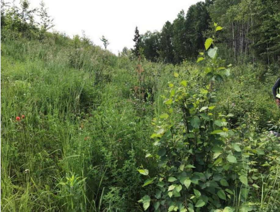
Photo II-17 TSF Embankment – West leg, looking south along downstream slope
