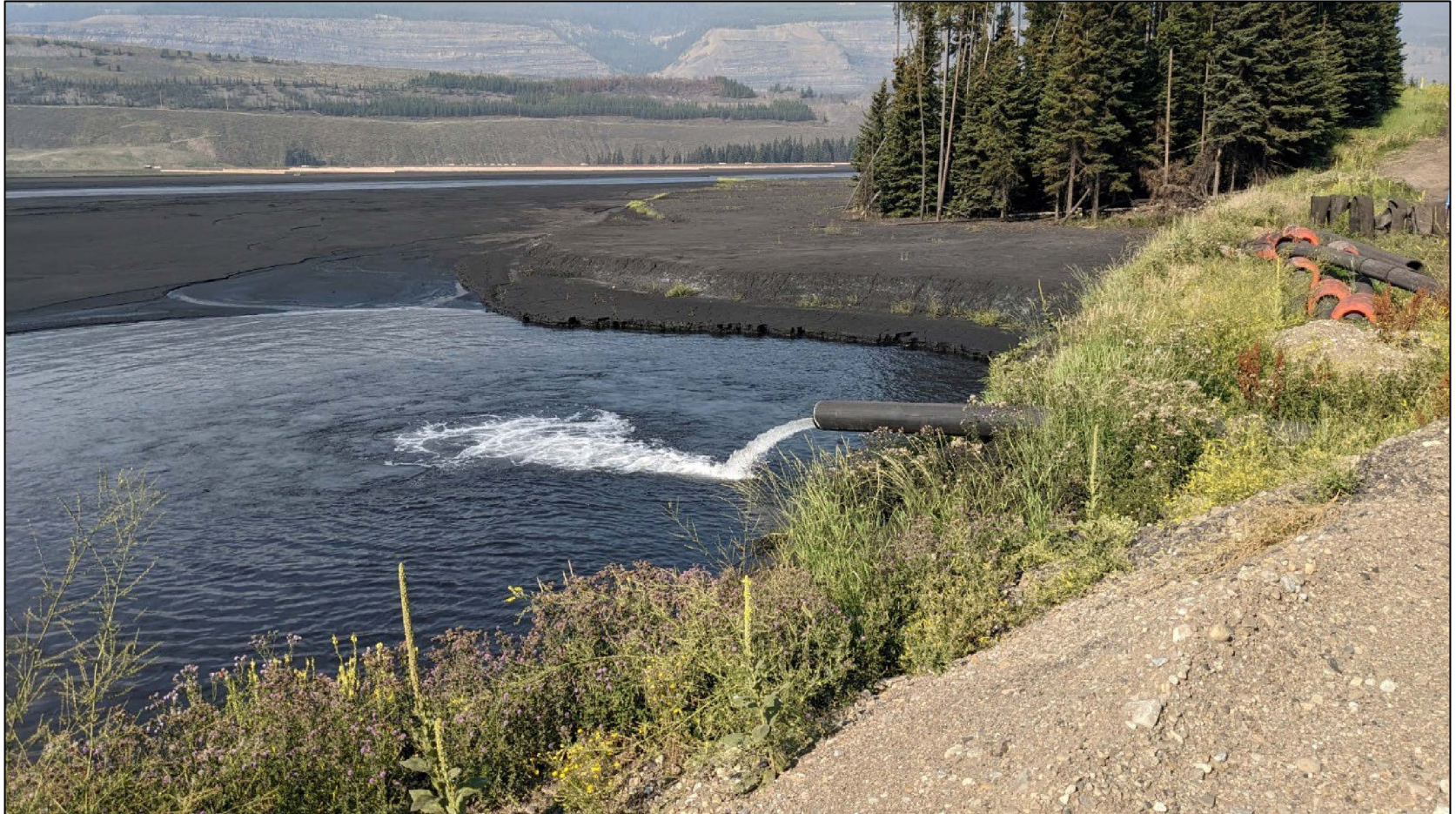
STP reclaim water pipeline from Turnbull TSF, looking northwest.
