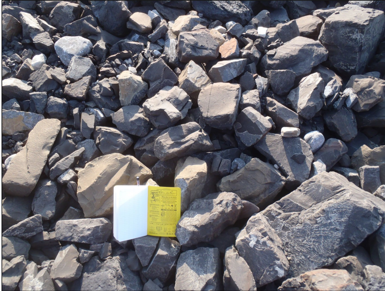
STP spillway channel Class 10 kg riprap at approximately spillway Sta. 0+025.
