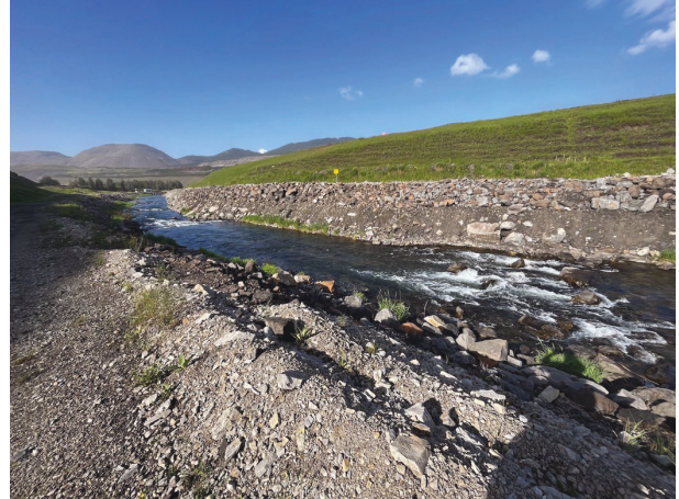
Photo 6: Looking downstream at NTP riprap (from approx. Sta. 0+550)
