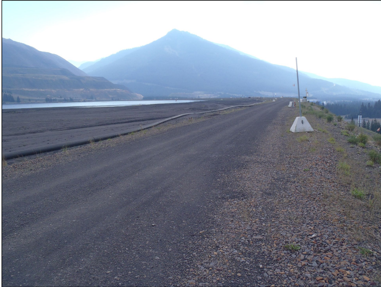
STP West Dam crest, looking southeast from approximately Sta. 0+950.
