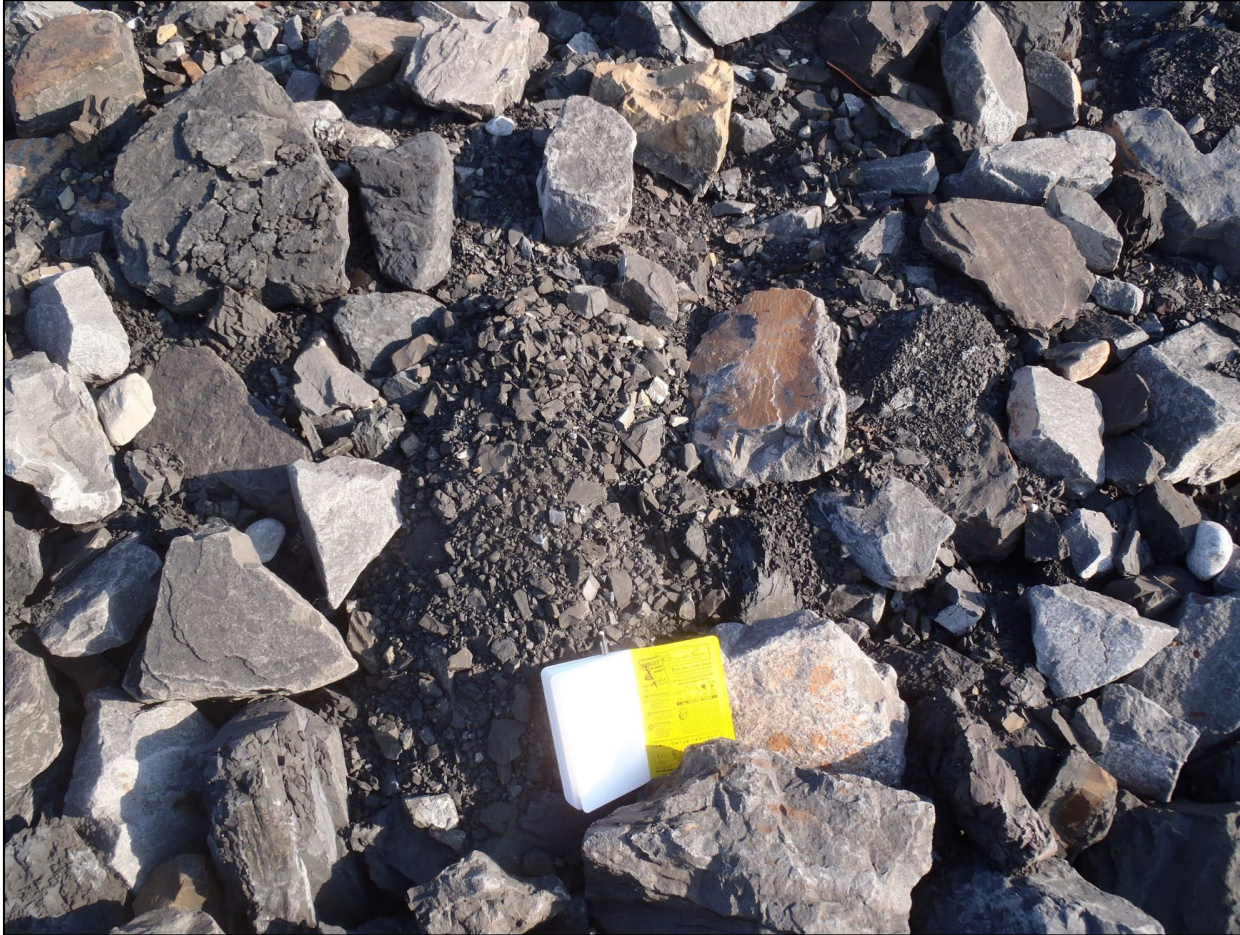
STP spillway channel Class 50 kg riprap at approximately spillway Sta. 0+090.
