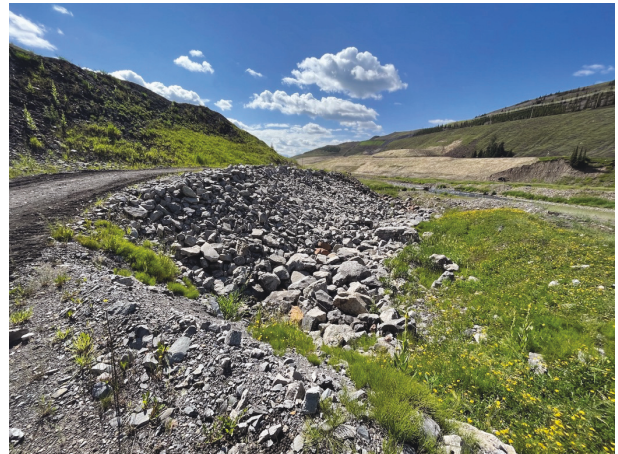
Photo 8: Looking downstream at start of STP riprap (from approx. Sta. 0+250)
