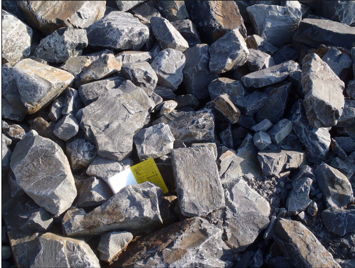
STP spillway channel Class 250 kg riprap at approximately spillway Sta. 0+350.
