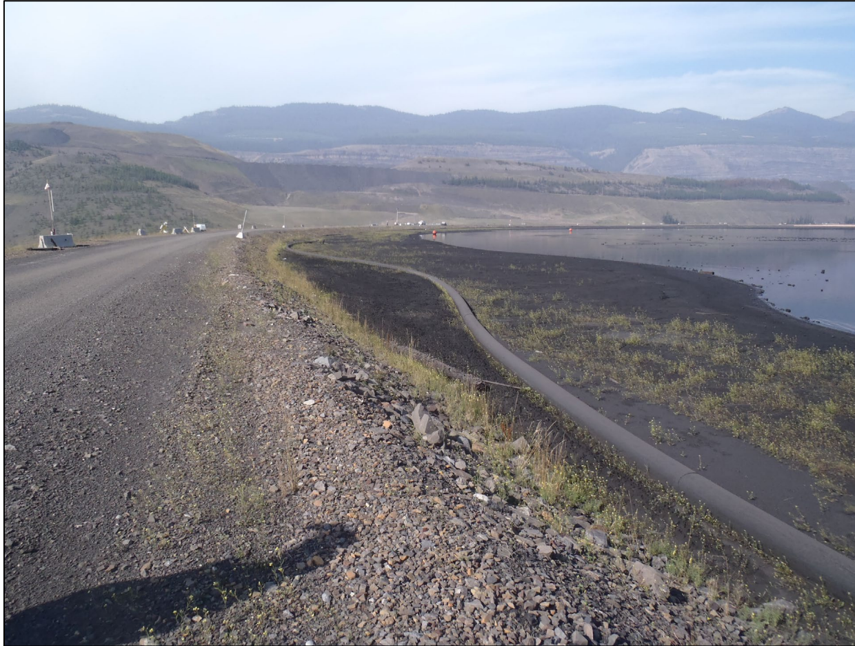
STP Main Dam crest and upstream beach, looking southwest from approximately Sta. 1+450.
