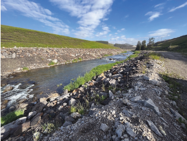
Photo 5: Looking upstream at NTP riprap (from approx. Sta. 0+550)
