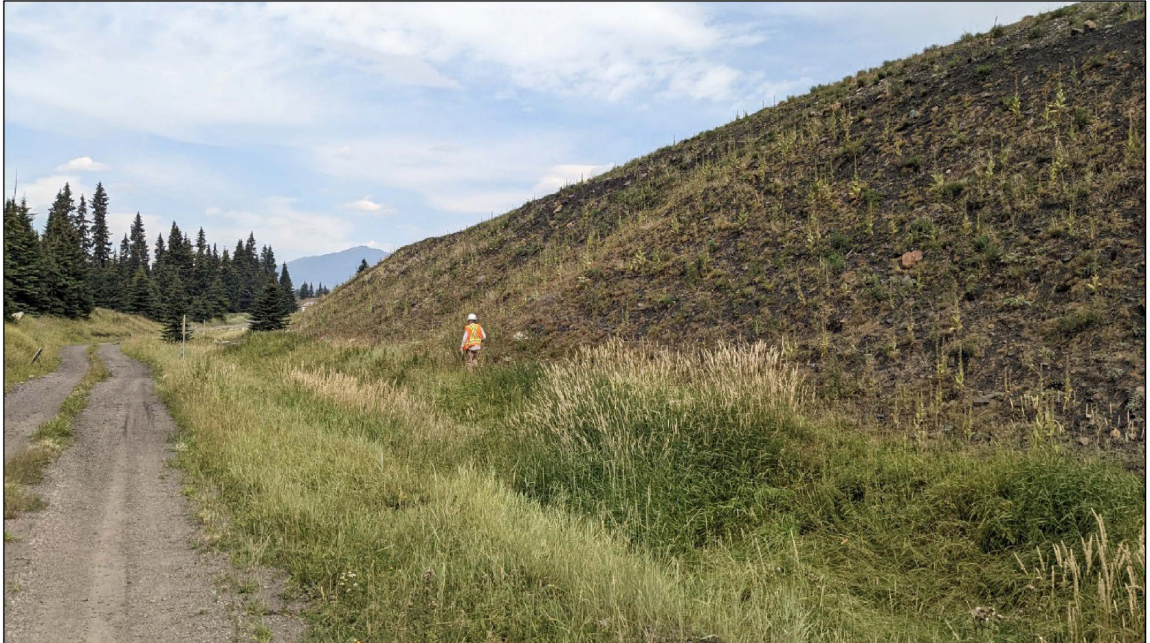
STP West Dam downstream slope, looking northeast from approximately Sta. 0+050.
