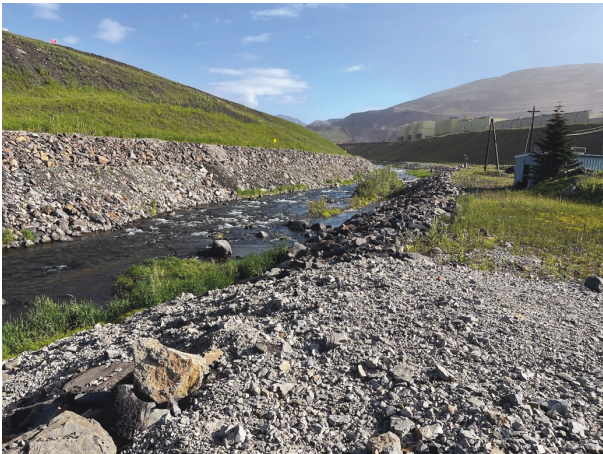
Photo 7: Looking upstream at NTP riprap (from approx. Sta. 0+900)
