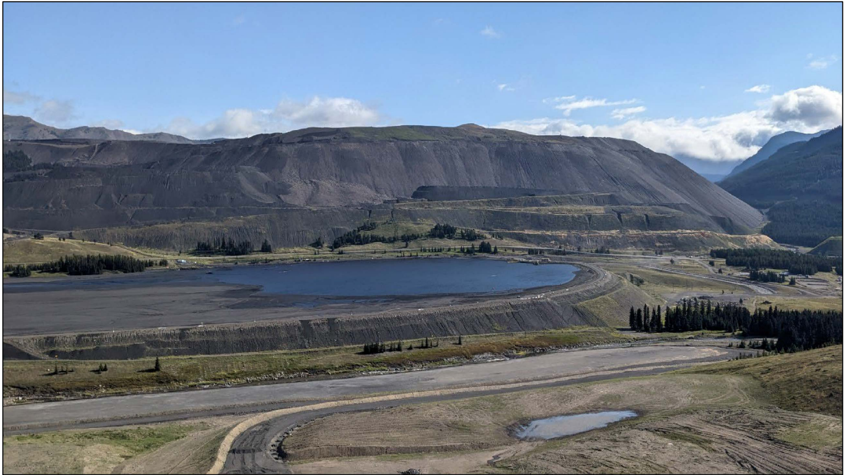
South Tailings Pond (STP) overview, looking east.
