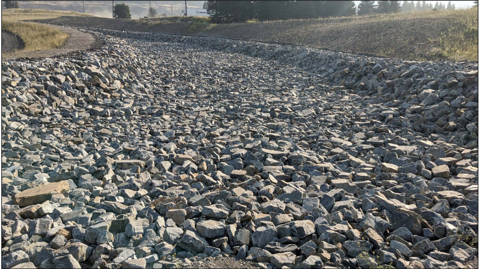
STP spillway channel outlet, looking northeast.
