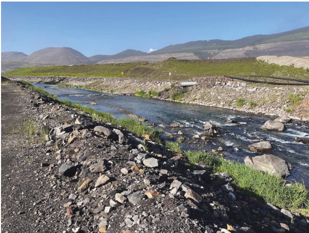
Photo 3: Looking downstream at riprap along right bank (Sta. 0+125)
