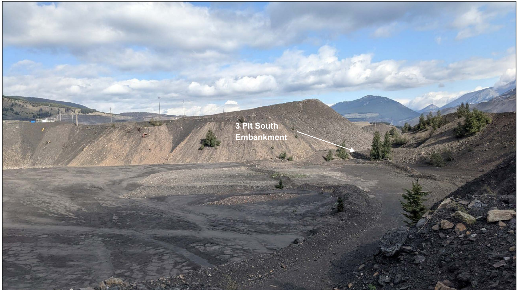
3 Pit South overview, looking north.
