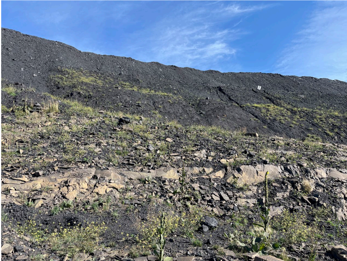
Blake spoil: west slope with minor vegetation, minor erosion rilling, and bedrock outcrop, looking east.
