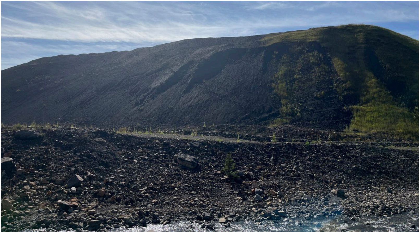
Impact Berm spoil: eastern slope and toe, looking southwest from Kilmarnock Creek.
