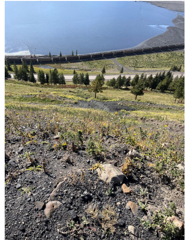
Kilmarnock / Toe Berm spoil: view of the erosion gully and runout that formed following the 2022 precipitation event.
