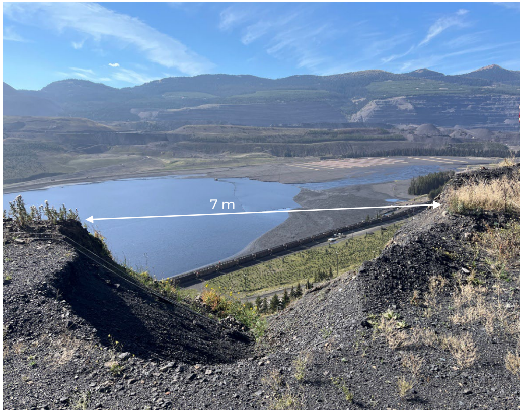
Kilmarnock / Toe Berm spoil: view of the erosion gully and runout that formed following the 2022 precipitation event.
