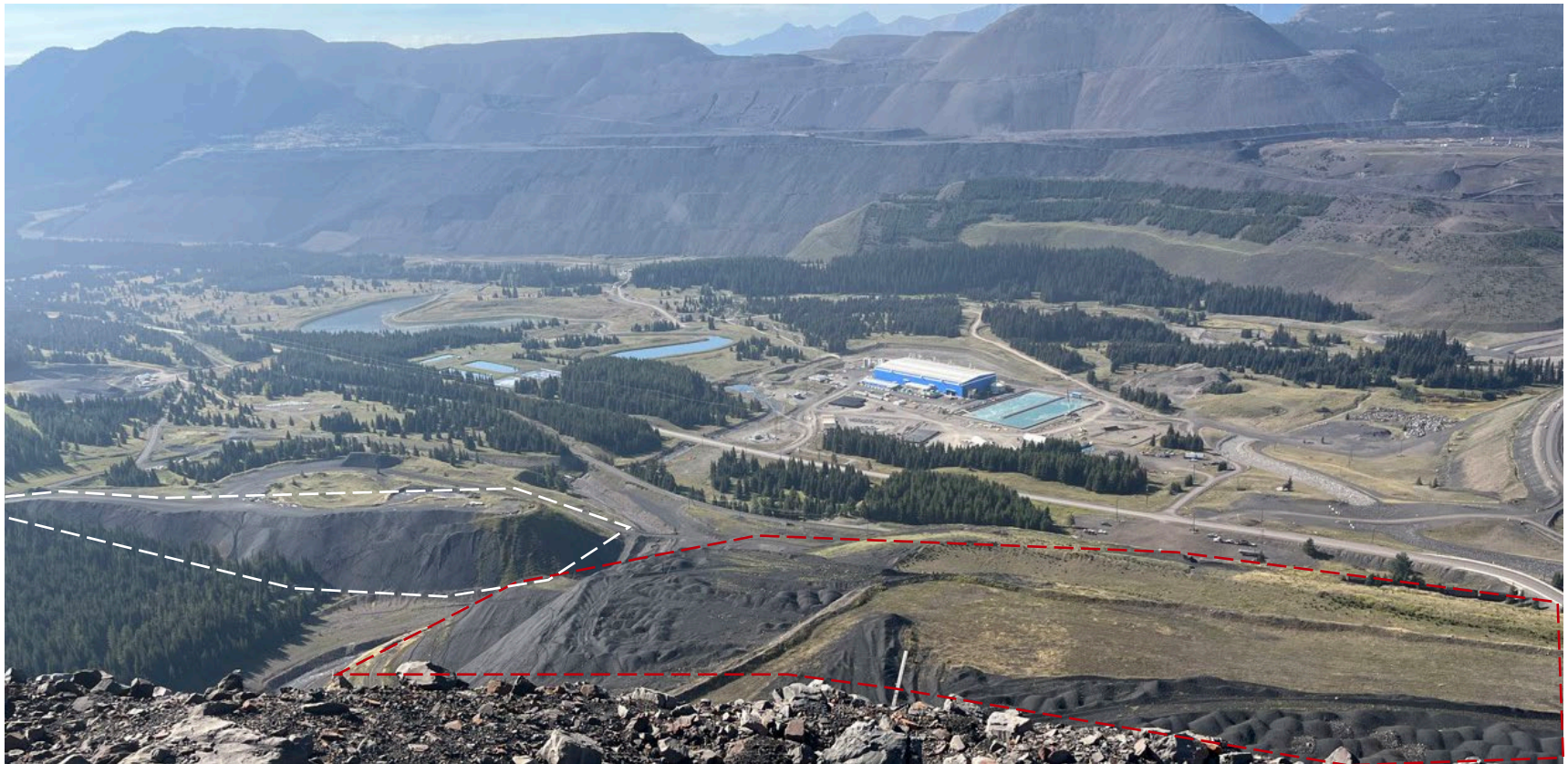
Kilmarnock / Toe Berm spoil (red dash) and Impact Berm spoil (white dash), looking southwest from the Old South spoil.
