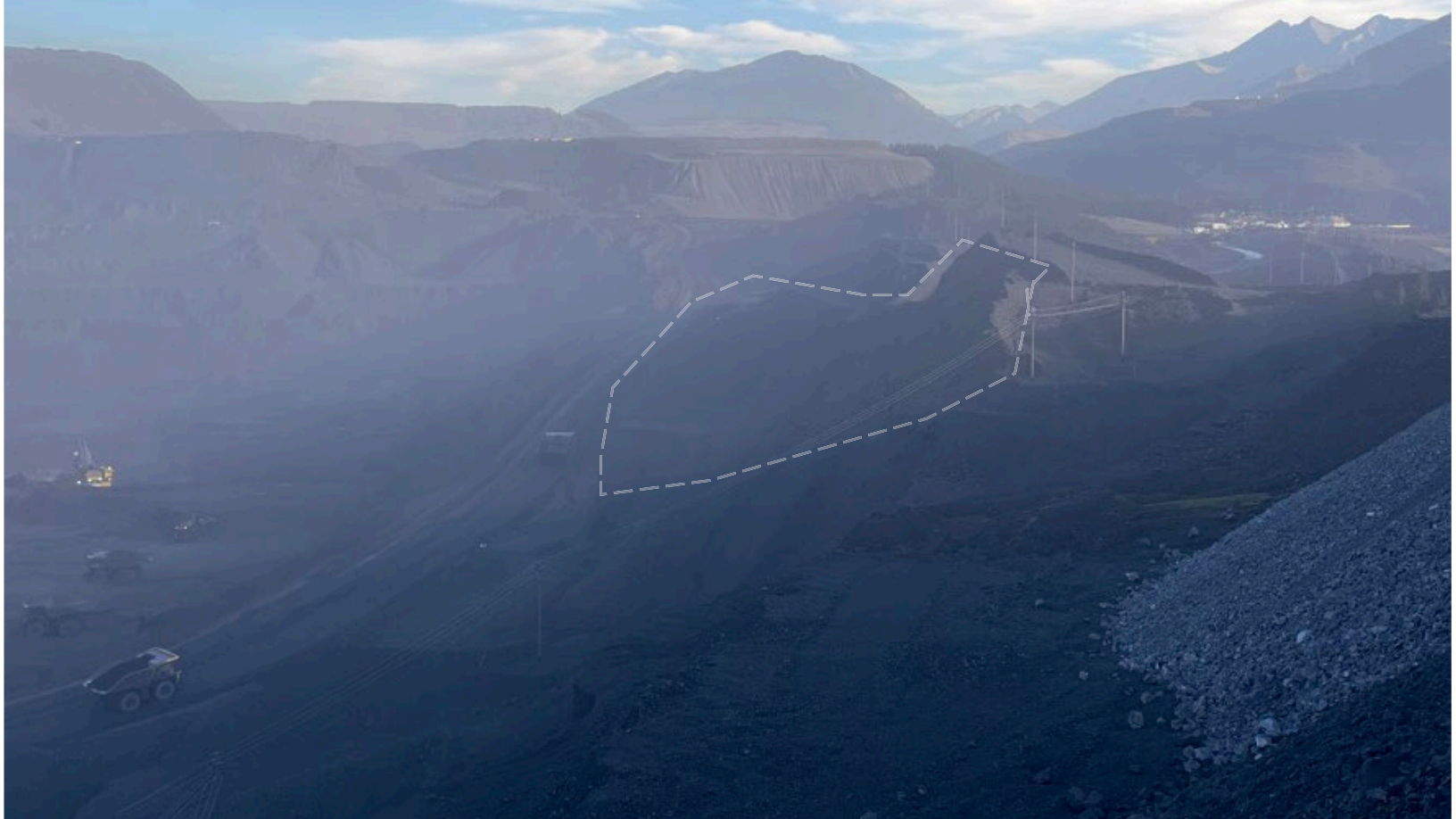
Box Yard spoil: view of excavated spoil remnant (white dash), looking north.
