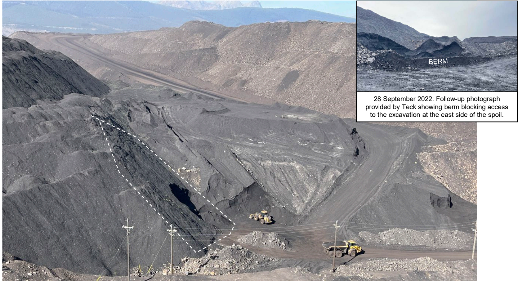
Eagle 4 South Backfill spoil: east side spoil at the toe, looking west at unauthorized operations at the toe and deformation above and adjacent to the excavated slope (white dashed area).
