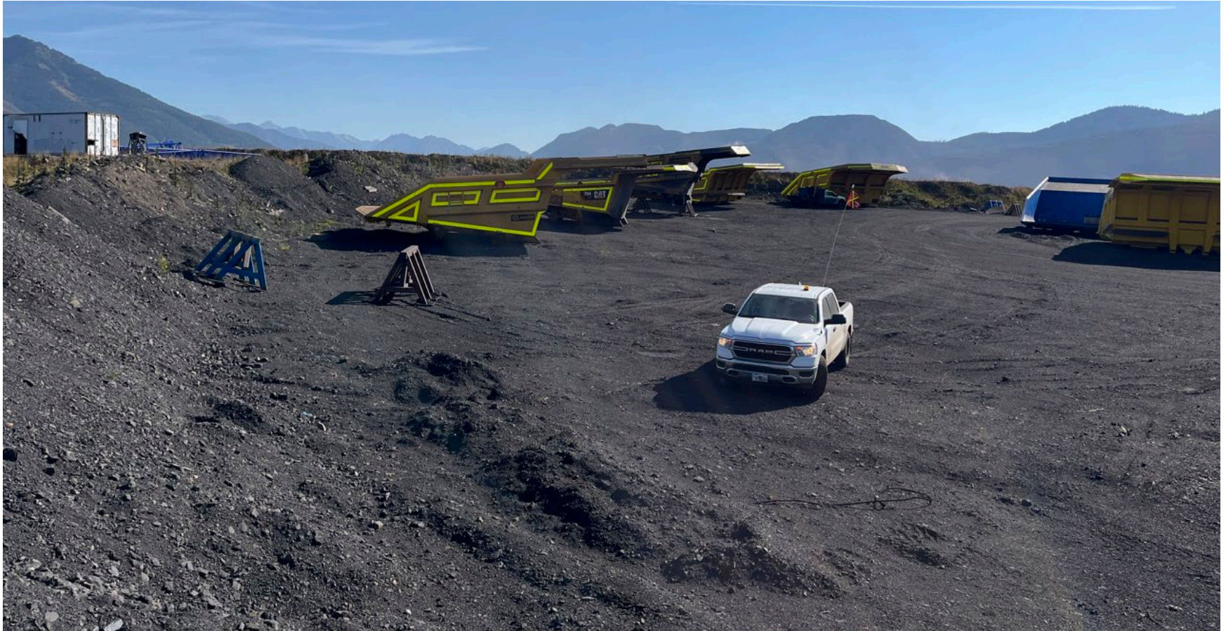
A-Spoil: overview of the crest, including equipment storage, looking north.
