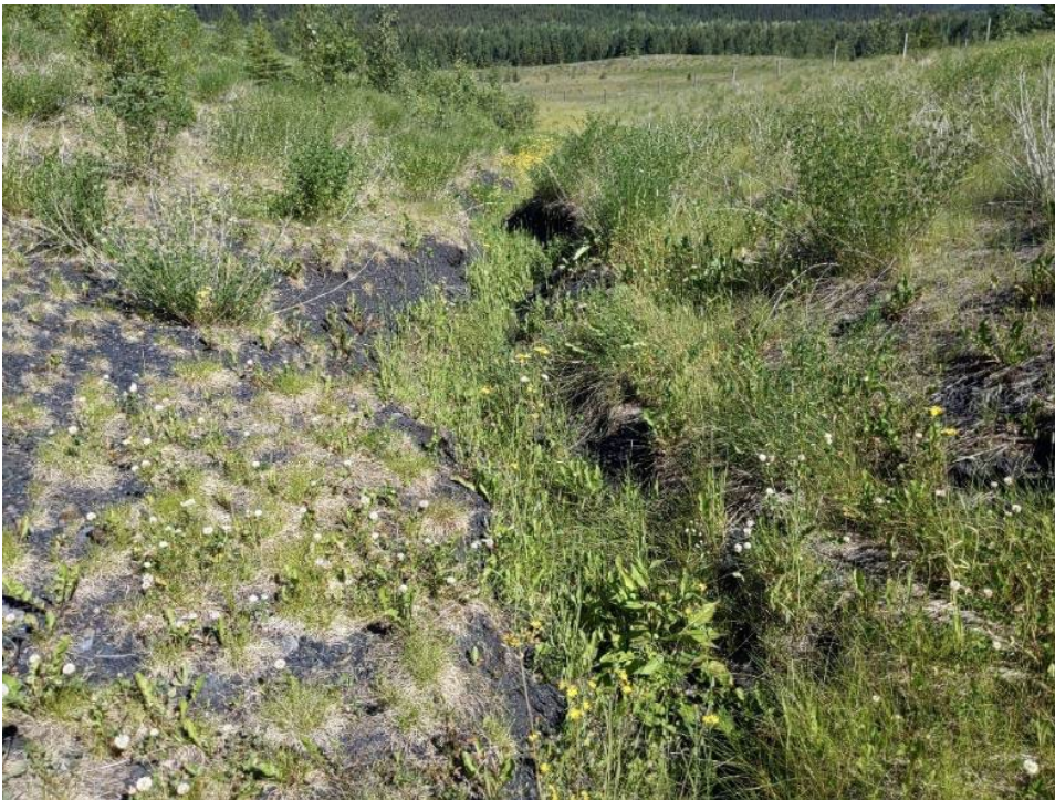
Photo II-13 Erosion gully near the toe of BTSF. No visible change from previous site visits. (BTSF-2022-08)
