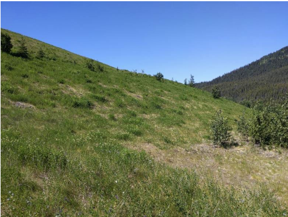
Photo II-15 BTSF downstream slope looking west (BTSF-2022-09)
