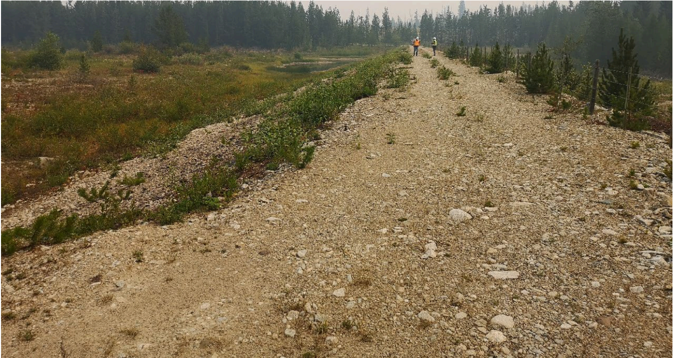
Photo I-B-17 S3 Pond: Overview of dam crest from right abutment (HGH-2021-27).
