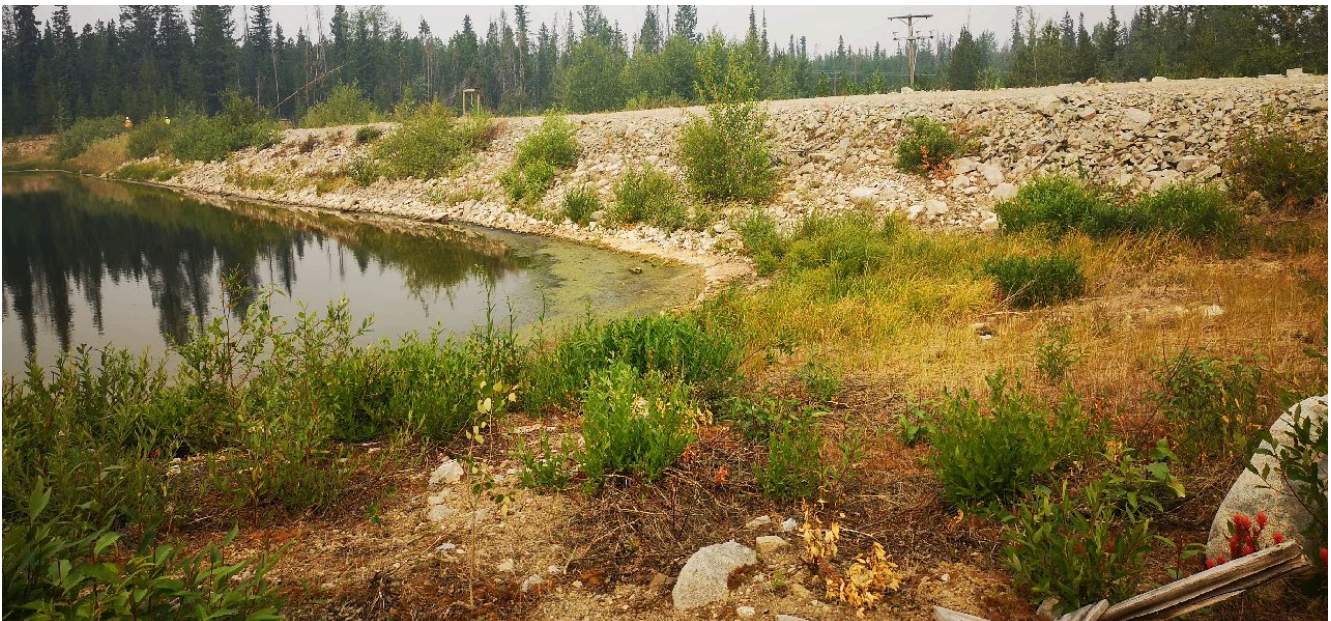
Photo I-B-10 S2 Pond: Overview of upstream slope riprap. Slope is in good condition (HGH-2021-23).
