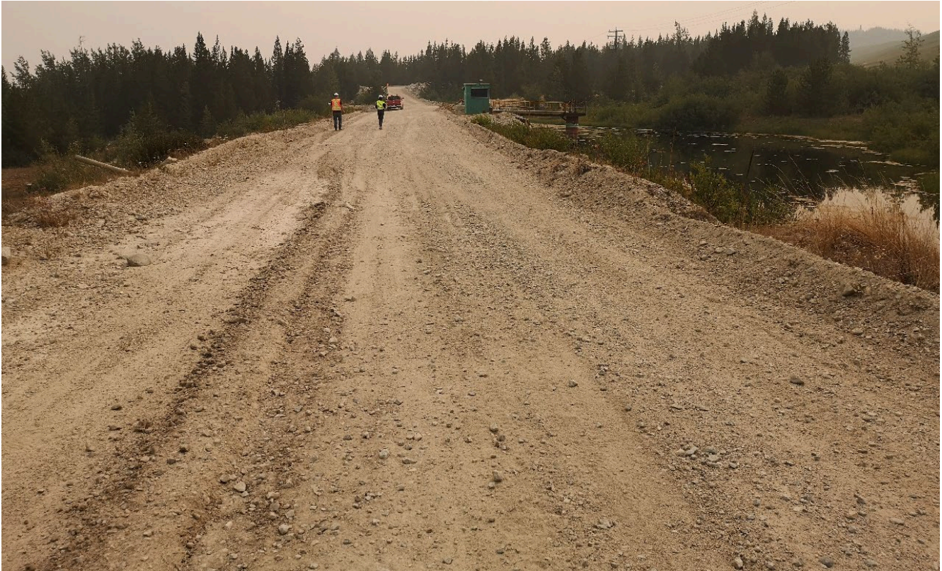
Photo I-B-38 S8 Pond: Overview of crest from left abutment (HGH-2021-38).
