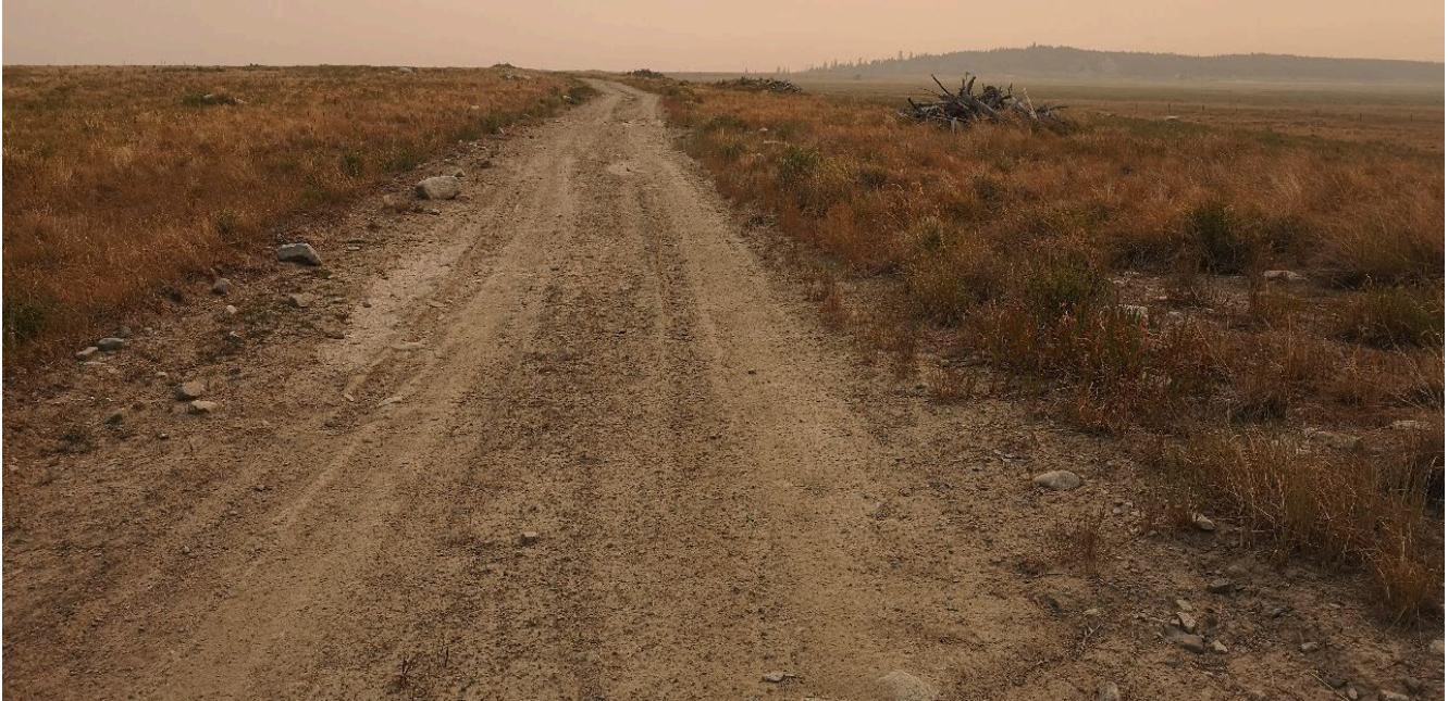
Photo I-A-5 North Dam crest access road to S1 Diversion. Minor rutting observed is managed by HVC as needed (HGH-2021-04)
