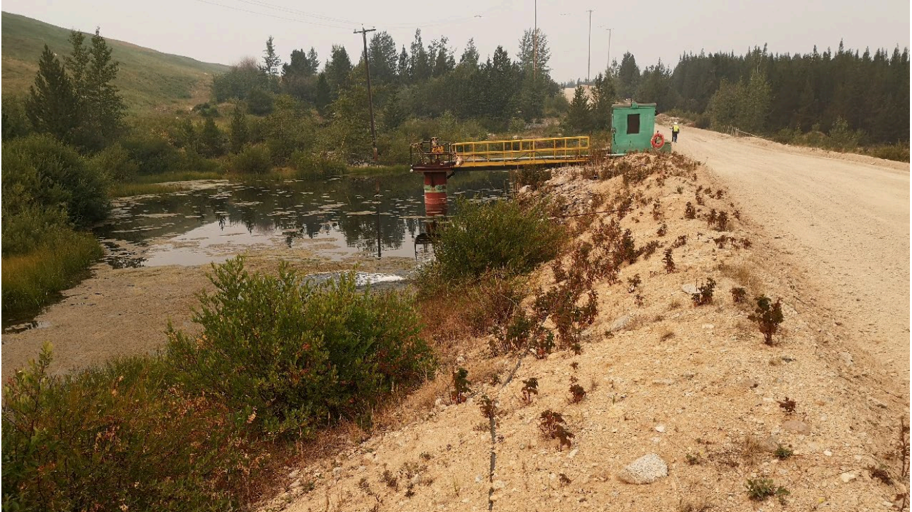
Photo I-B-41 S8 Pond: View of impoundment, catwalk and outlet pump to S1 Pond (HGH-2021-40 and HGH-2021-41).
