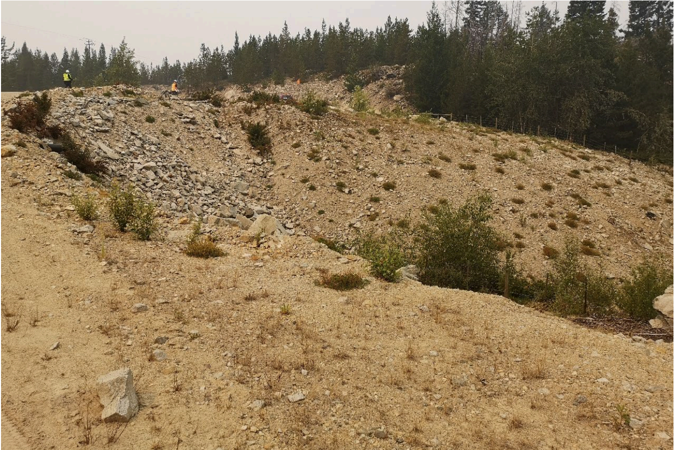
Photo I-B-2 S1 Pond: S1 Pond dam downstream slope (HGH-2021-19).
