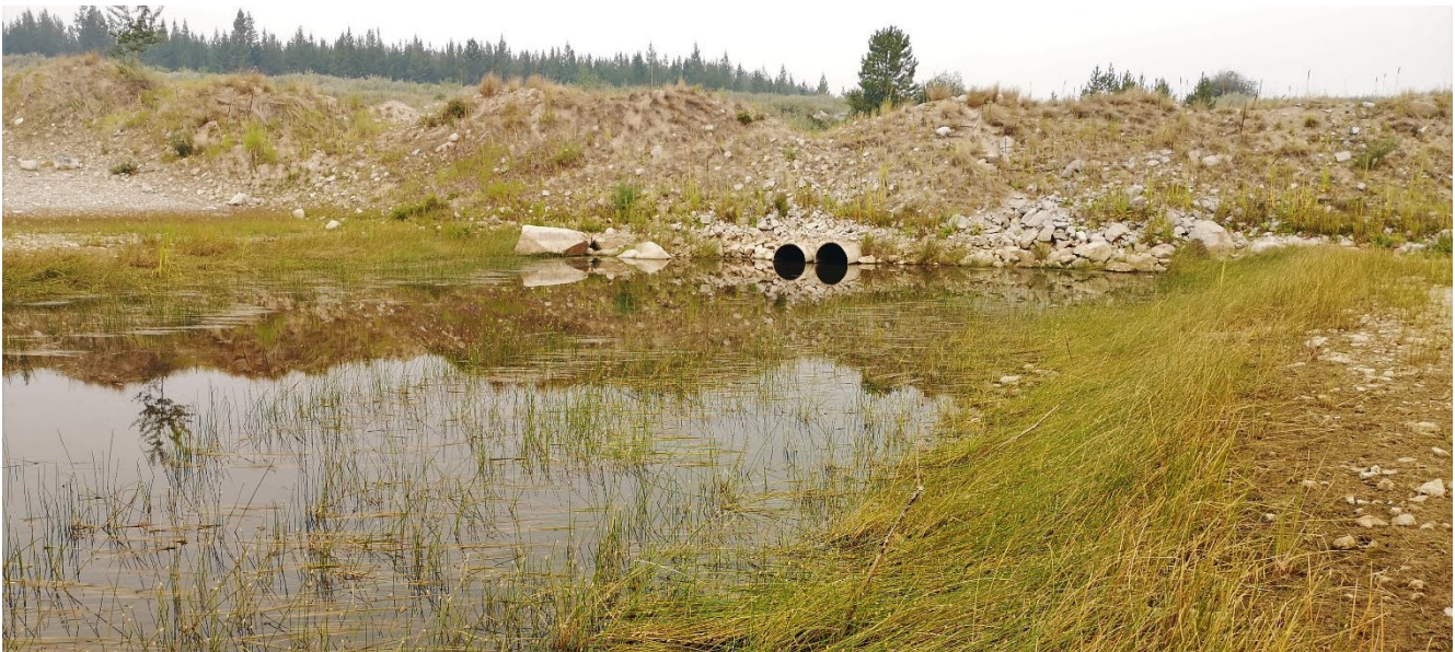
Photo I-A-19 Approach channel. Road culverts are partially submerged, section upstream of culverts is clear of debris and vegetation (HGH-2021-10)
