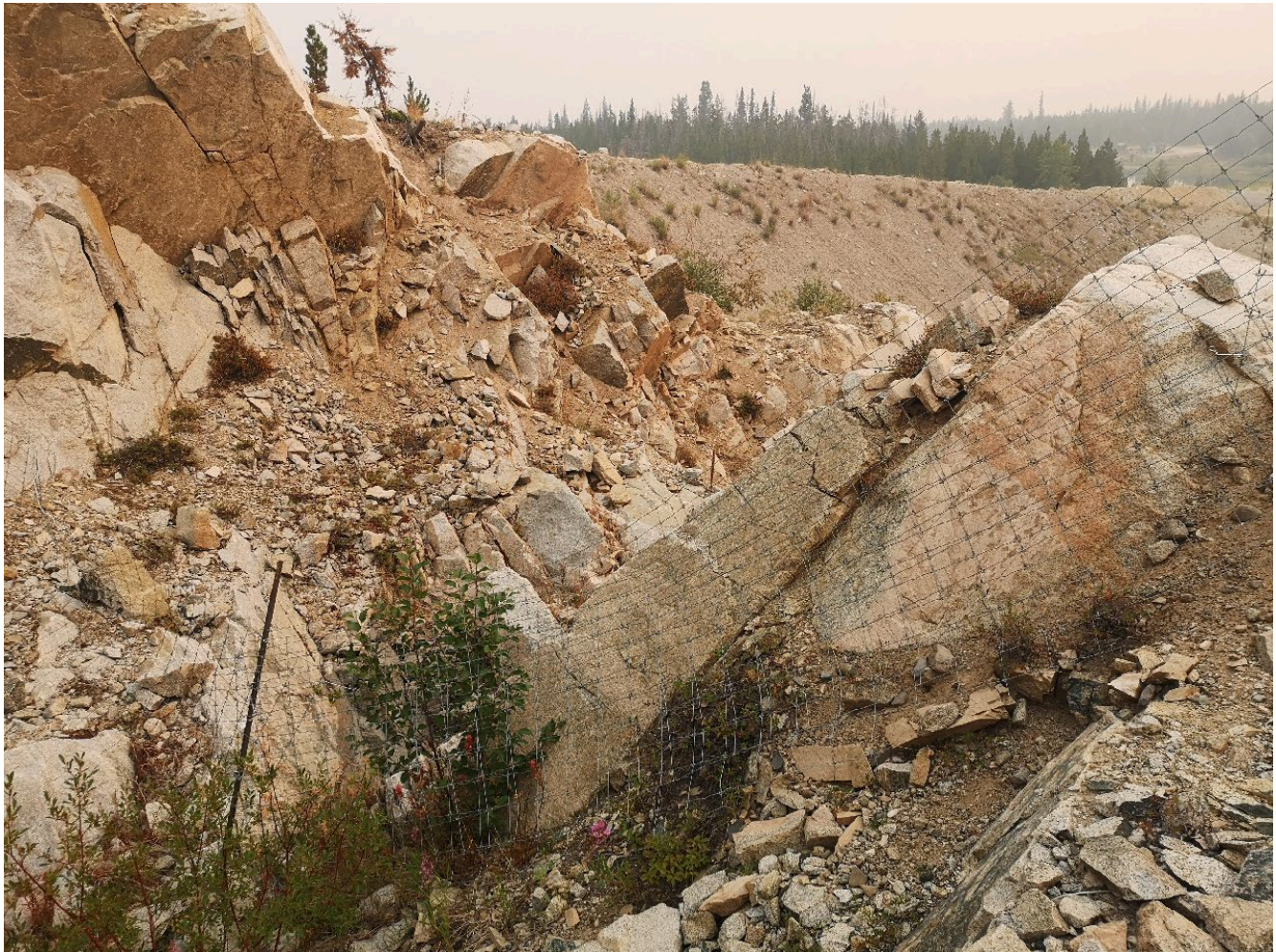
Photo I-A-26 Highmont Spillway channel upstream of spillway drop (HGH-2021-15)
