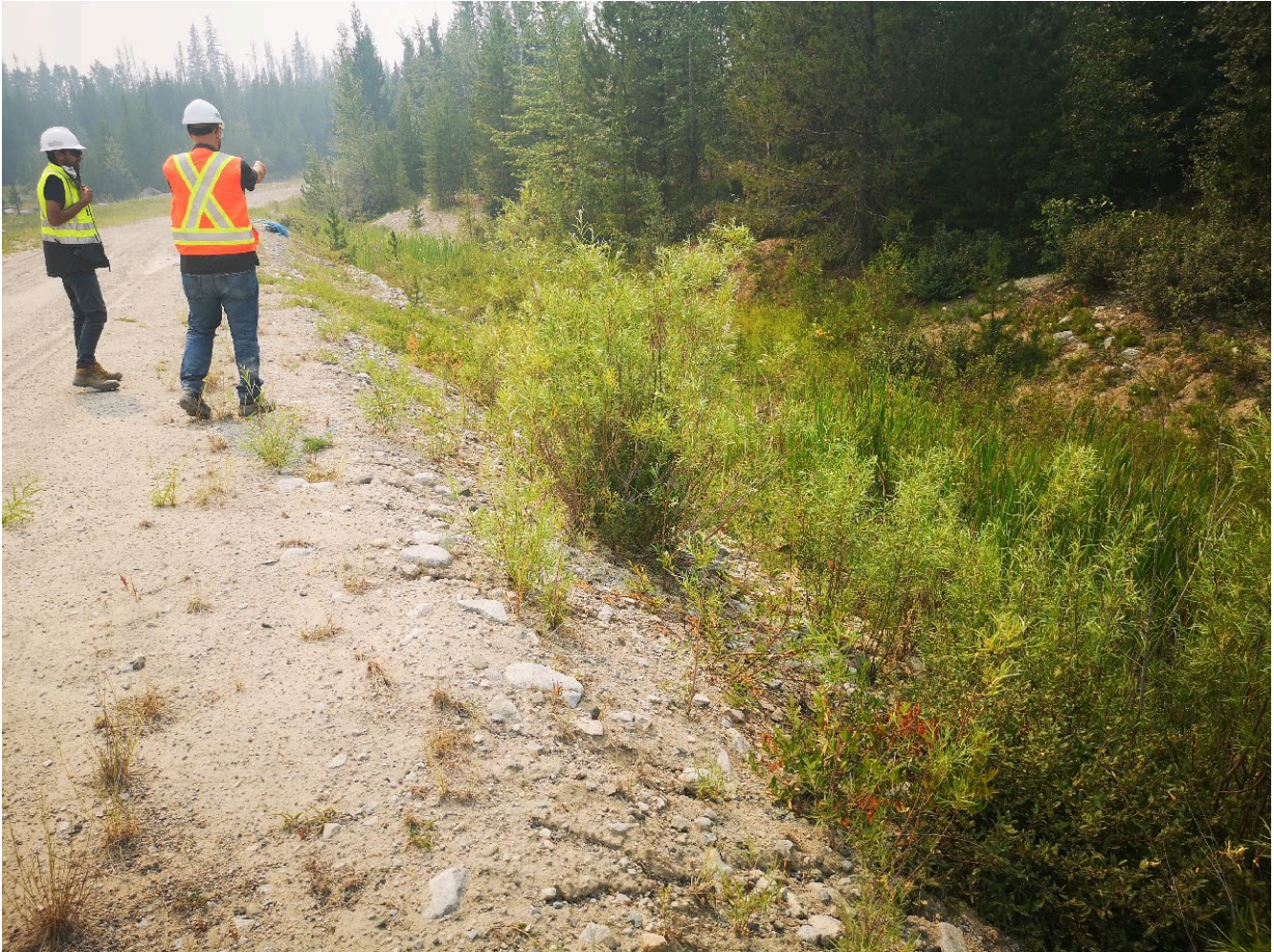
Photo I-B-32 S5 Pond: Pumping Sub-cell spillway channel (HGH-2021-34).
