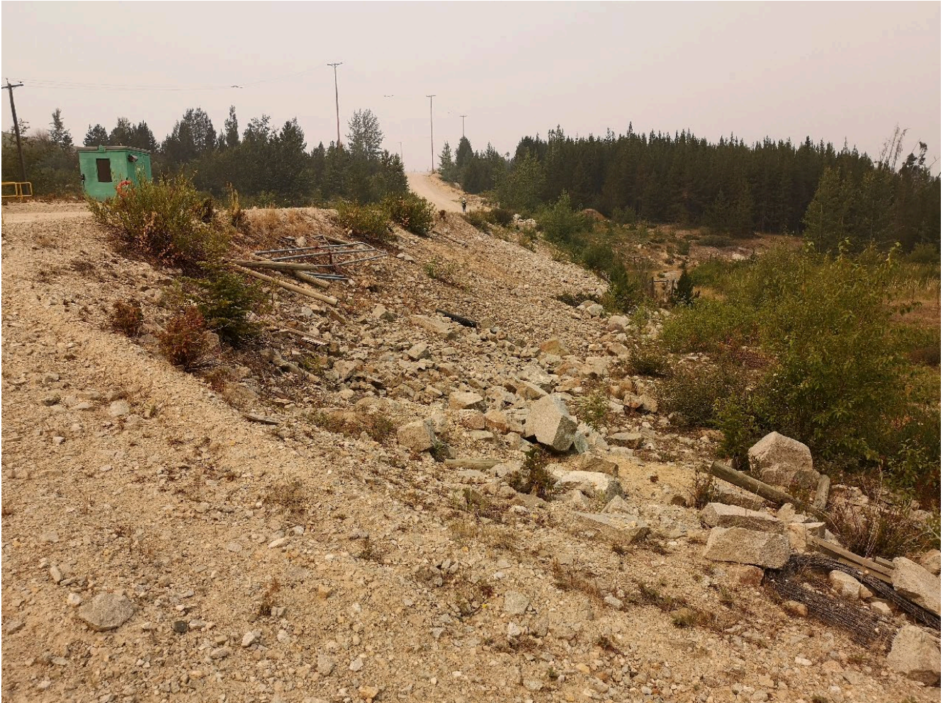
Photo I-B-39 S8 Pond: View of downstream slope (HGH-2021-39).
