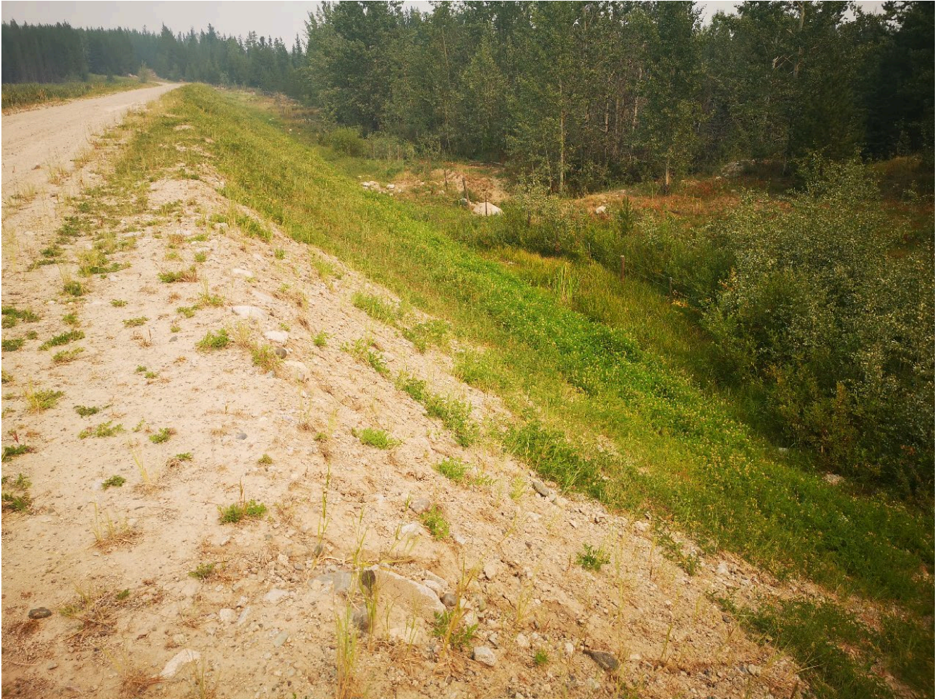
Photo I-B-28 S5 Pond: Downstream slope of perimeter crest, looking north (HGH-2021-31).
