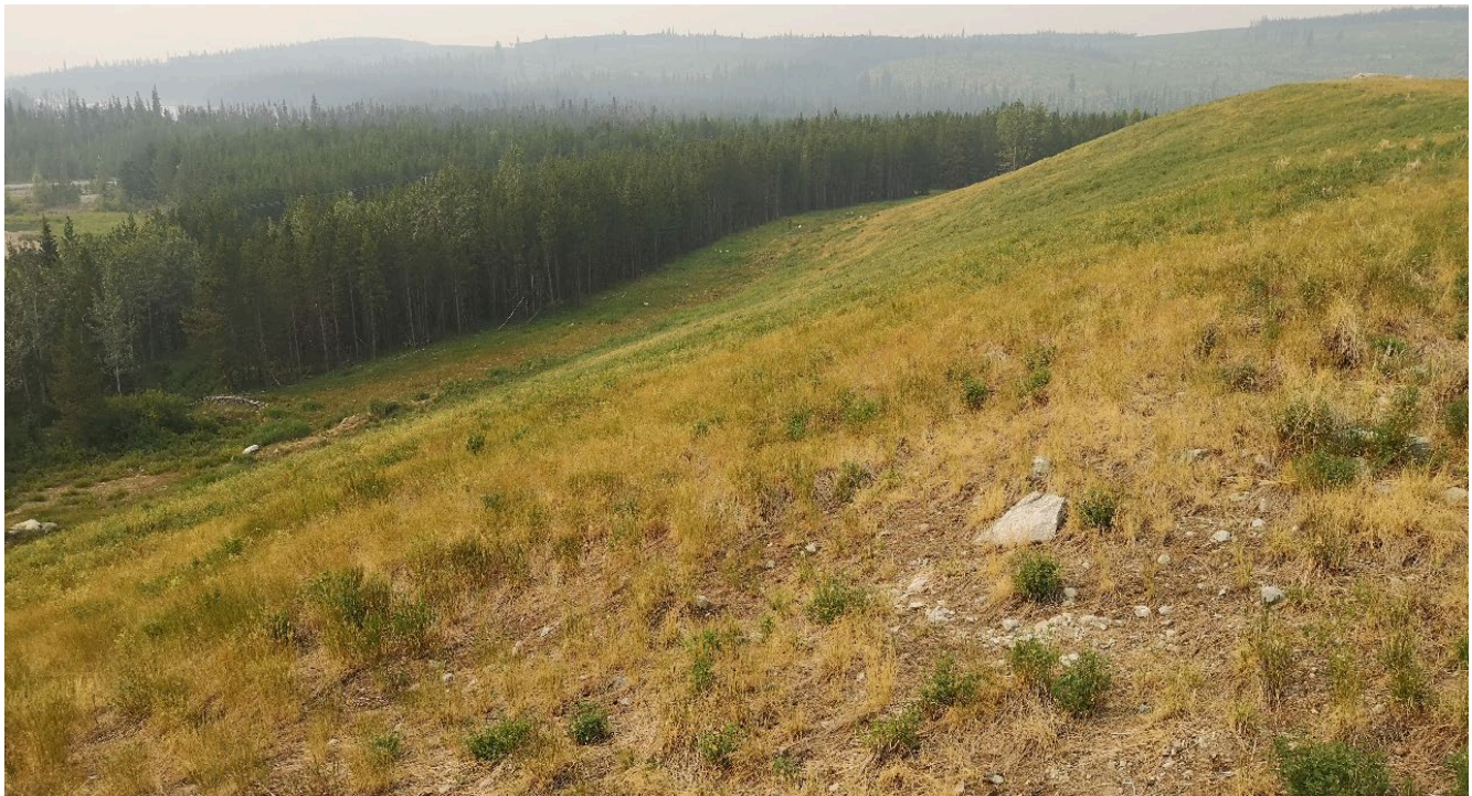
Photo I-A-14 View of South Dam downstream slope looking southwest. Slope is vegetated and in good condition (HGH-2021-08)
