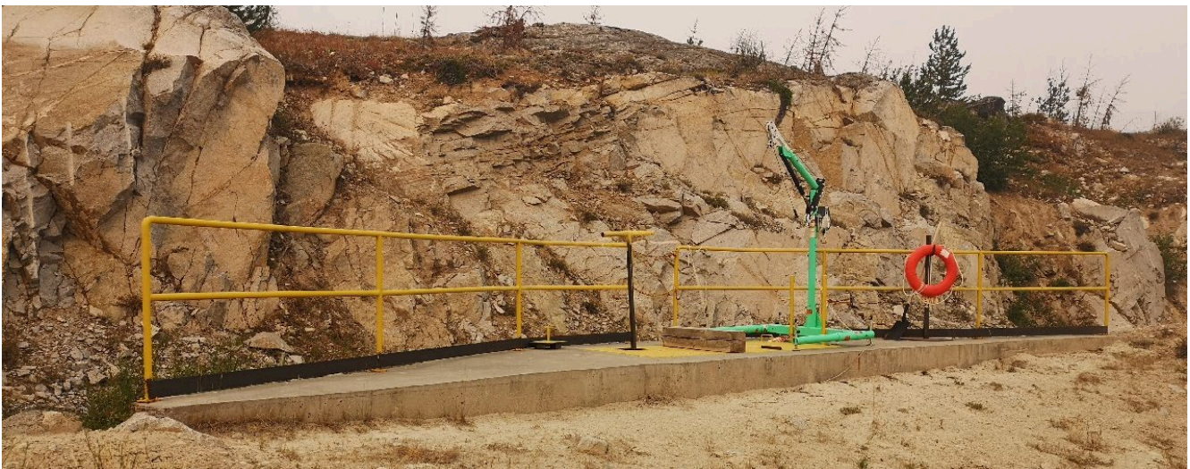
Photo I-A-24 Highmont Spillway channel, S1 Pond diversion control (HGH-2021-14)
