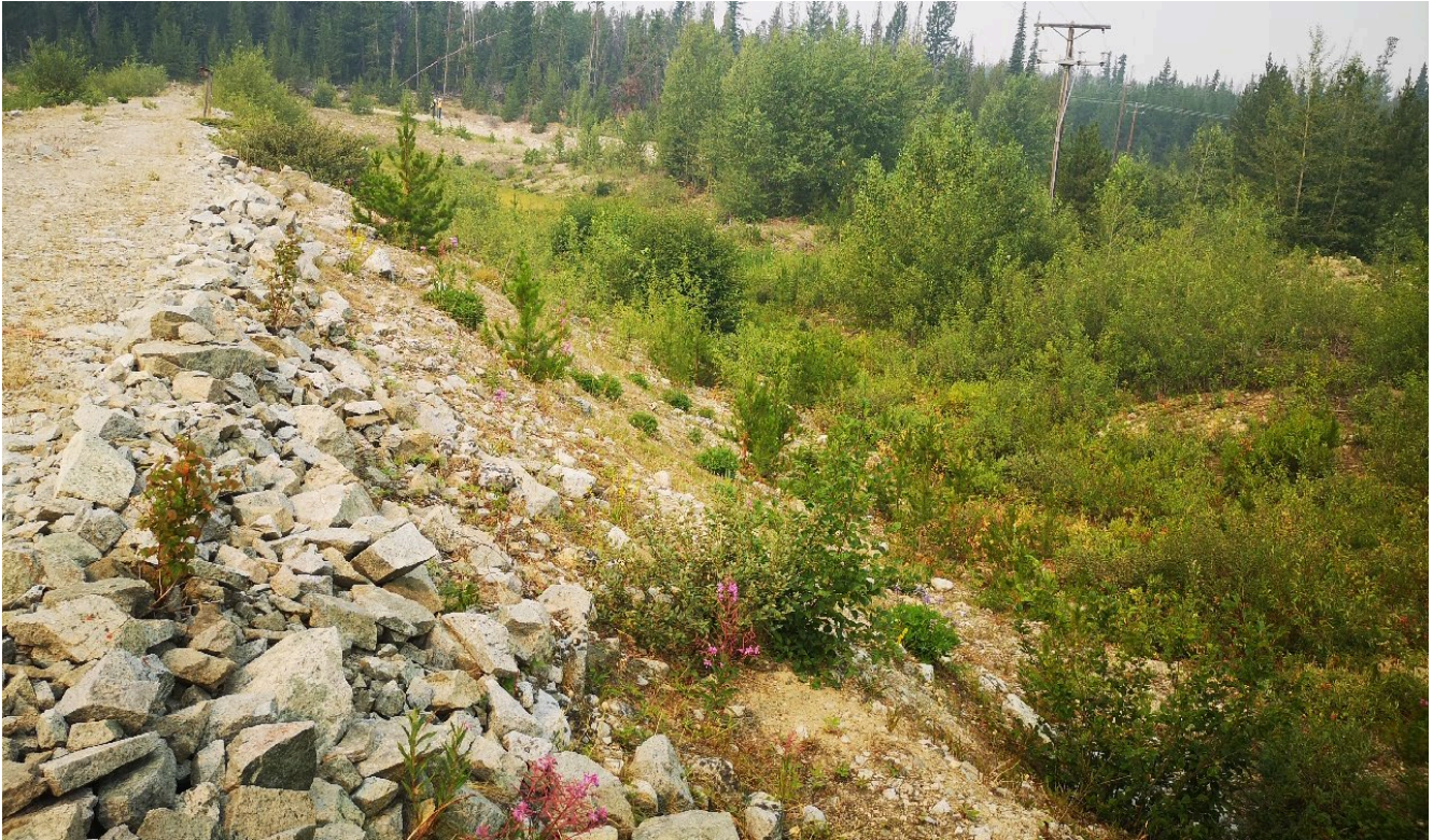
Photo I-B-10 S2 Pond: Overview of upstream slope riprap. Slope is in good condition (HGH-2021-23).
