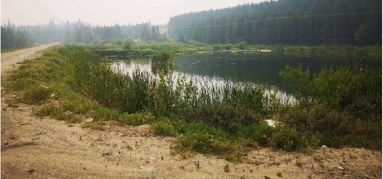
Photo I-B-29 S5 Pond: S5 Pond north outlet pipe, permanently sealed. Metal plates placed at intake and pipes filled with till in 2015 (HGH-2021-32 and HGH-2021-33).
