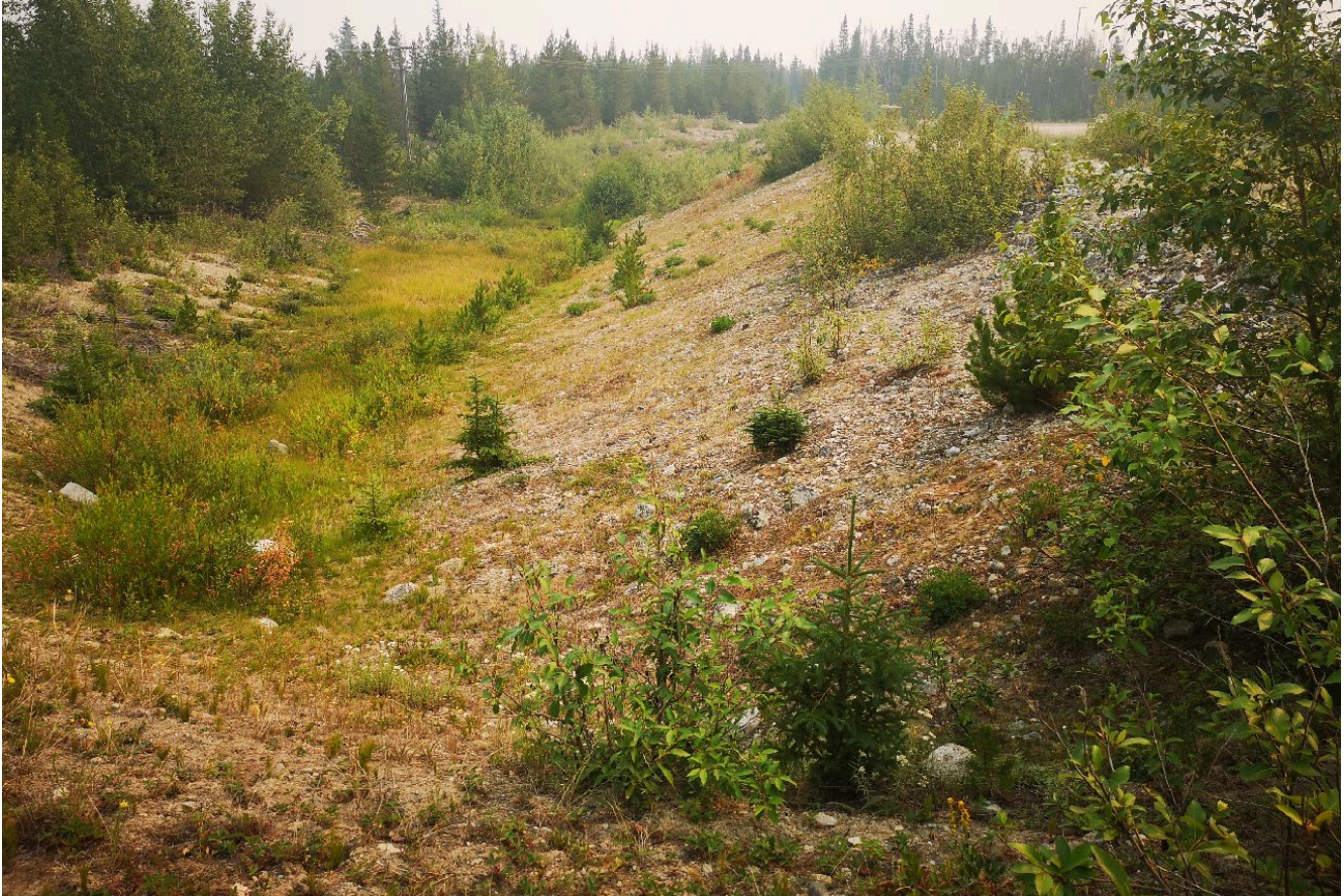
Photo I-B-16 S2 Pond: Vegetation and signs of recent ponded water at downstream toe (HGH-2021-26).
