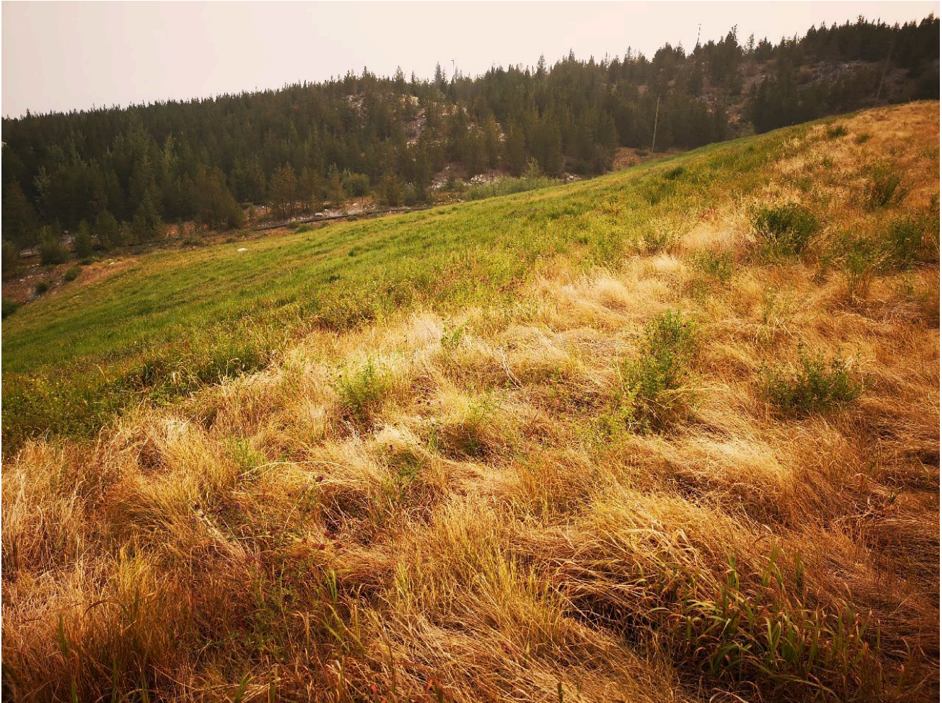
Photo I-A-10 View of North Dam downstream slope looking east (HGH-2021-06)
