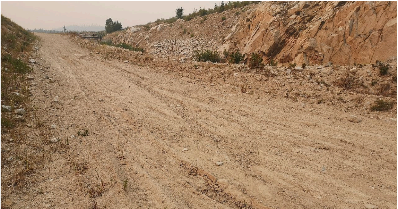
Photo I-A-5 North Dam crest access road to S1 Diversion. Minor rutting observed is managed by HVC as needed (HGH-2021-04)
