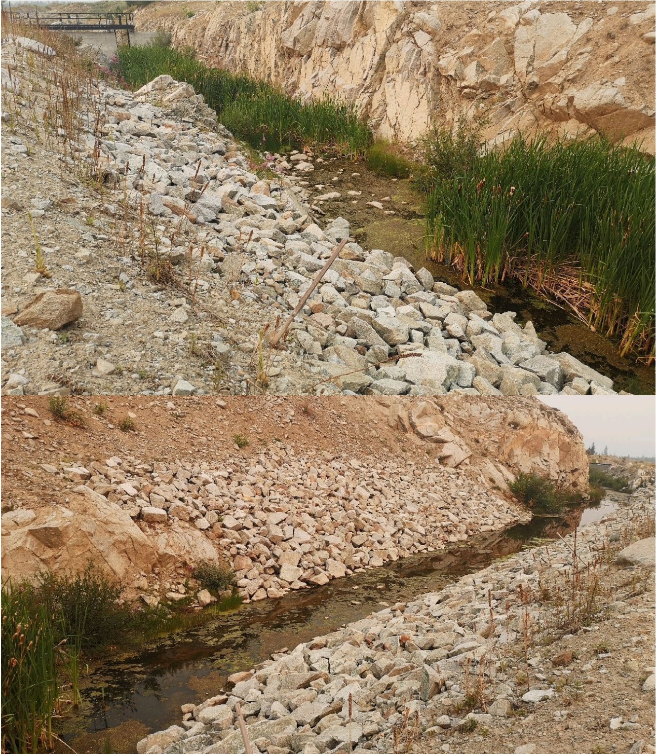
Photo I-A-22 Downstream area of spillway flow control gate (HGH-2021-13)
