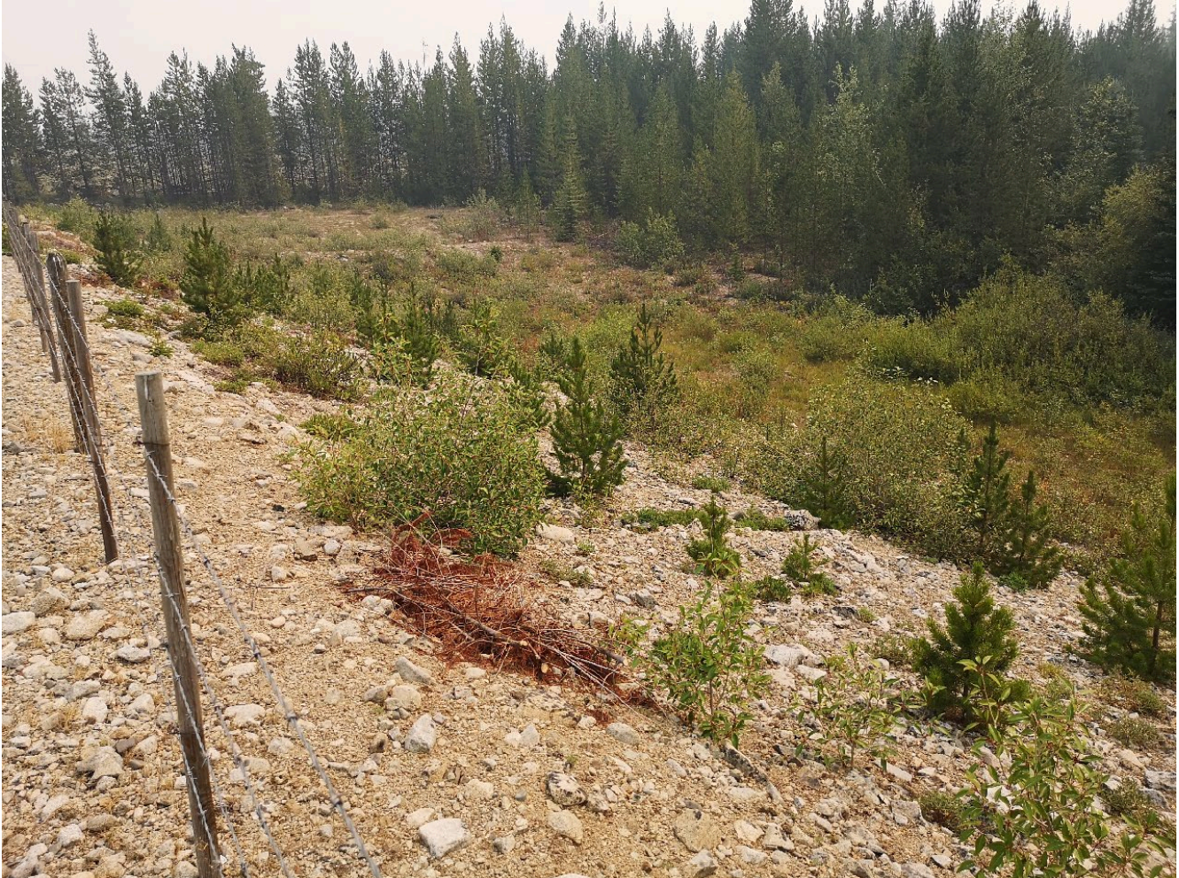
Photo I-B-21 S3 Pond: Overview of downstream slope with small trees from mid dam (HGH-2021-28).
