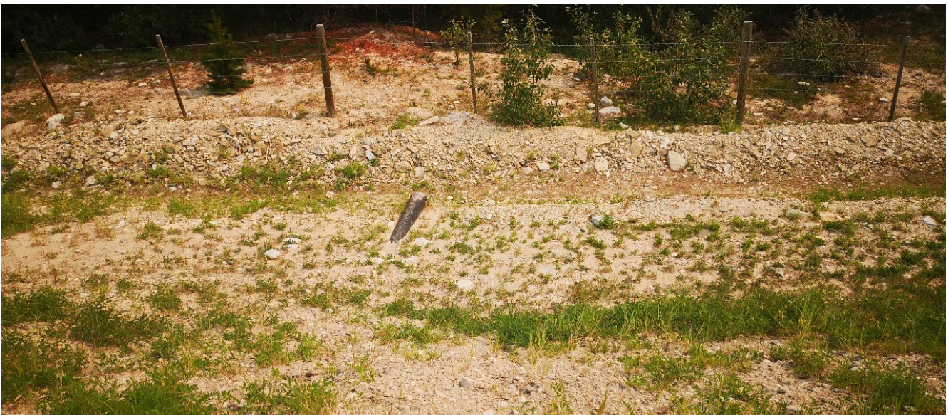
Photo I-B-34 S5 Pond: Overview of downstream slope and Outlet #2 pipe daylighting at toe, looking east (HGH-2021-35).
