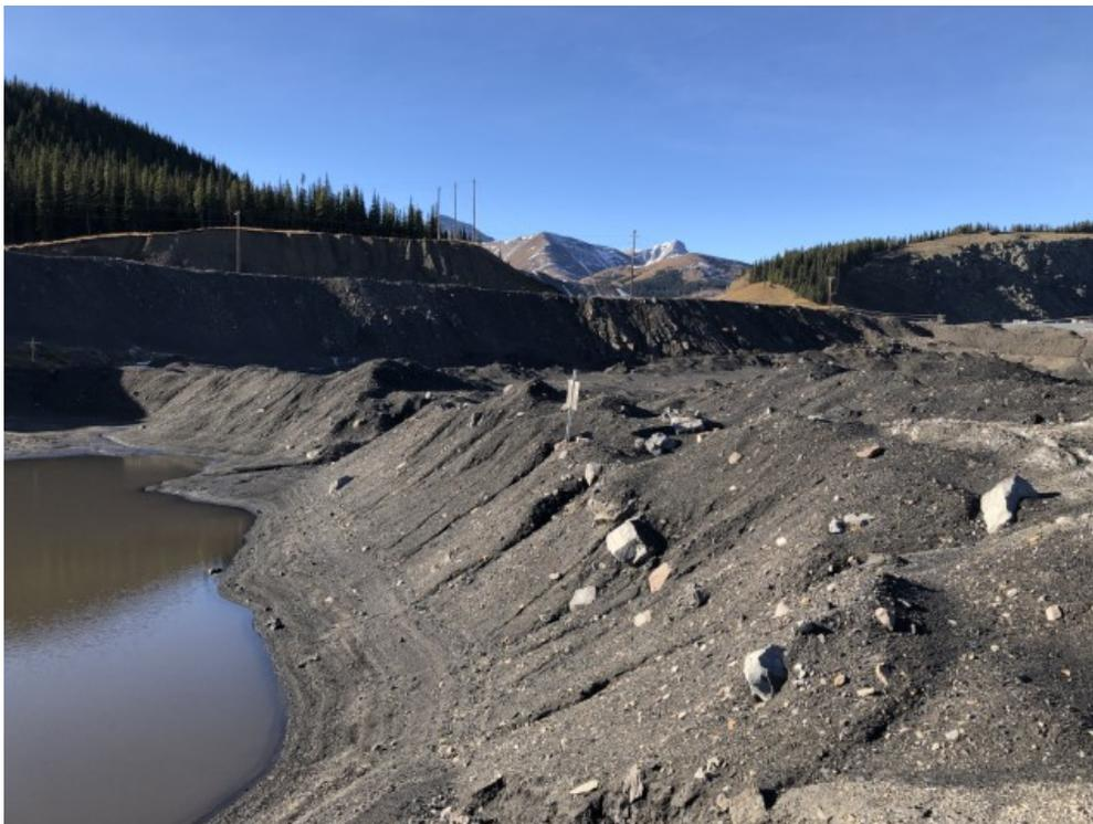
Photo A-22: Looking west near WP14 at CCR surface placed above tailings in 50-B9 (WP14, IMG\_7016)
