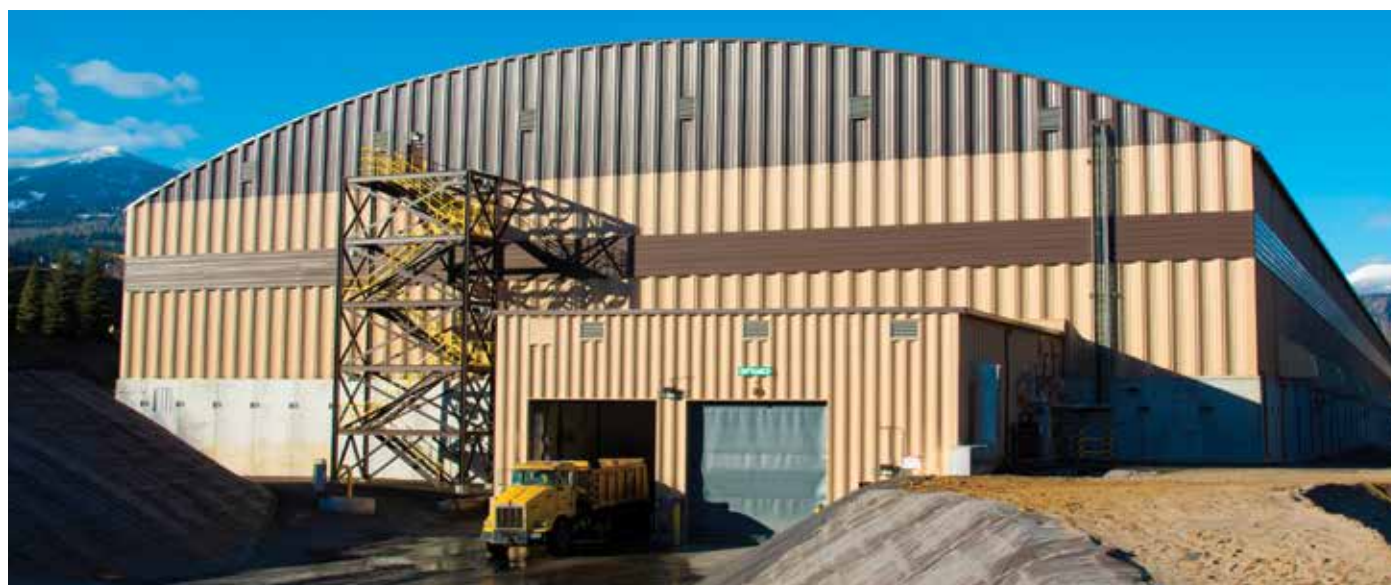
Pictured Above: Trail Operation’s new Smelter Recycle Building. The building is a key component of Trail’s Fugitive Dust Reduction Program, and is helping improve air quality.
